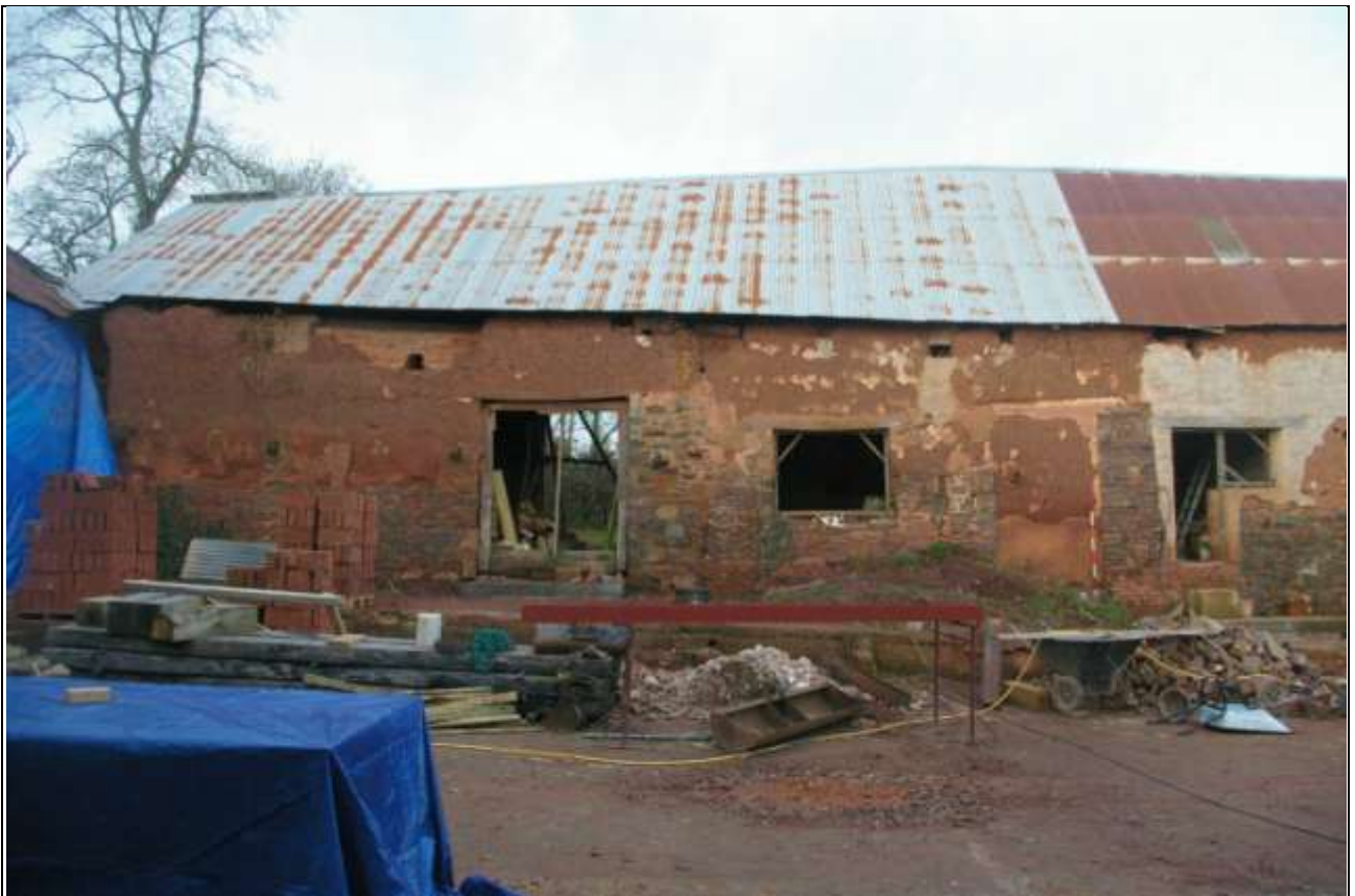
The south-east elevation, at the south-end; from the south-east (2m scale).
