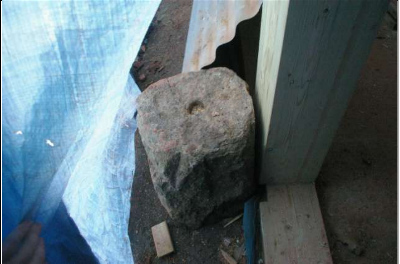
Detail of one of the stone plinths for the oak posts to the front of the western linhay; from the west.
