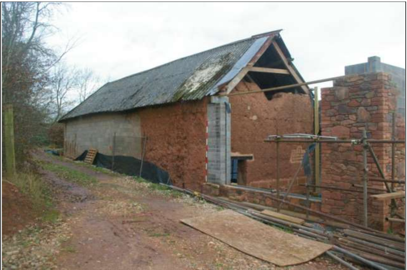
The south-west elevation the west linhay, surviving cob on a stone plinth to the south end and base, but largely rebuilt in concrete block sometime in the 20 th century; from the south (2m scale).
