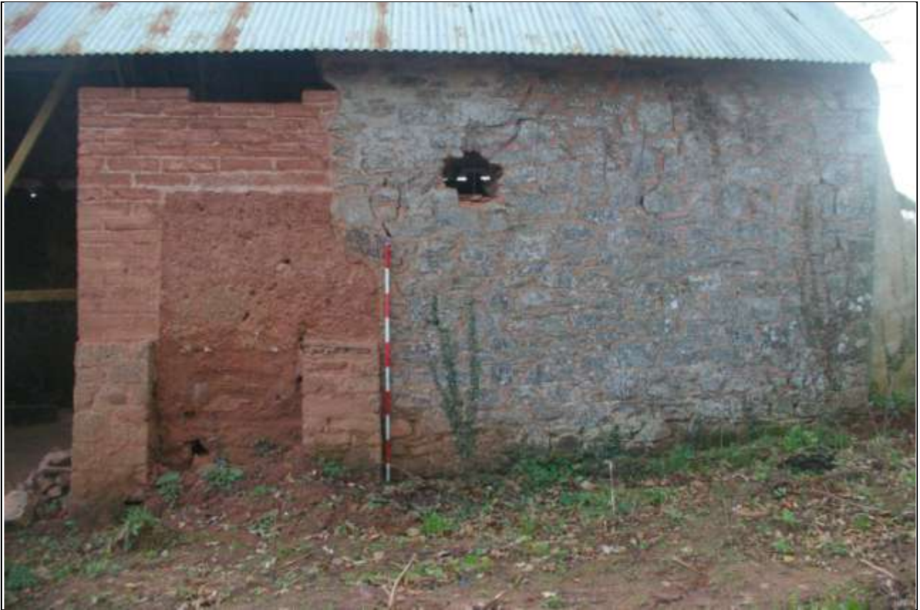
The south end of the barn, later 17 th or 18 th century, showing a 19 th century rebuild; from the north-west (2m scale).
