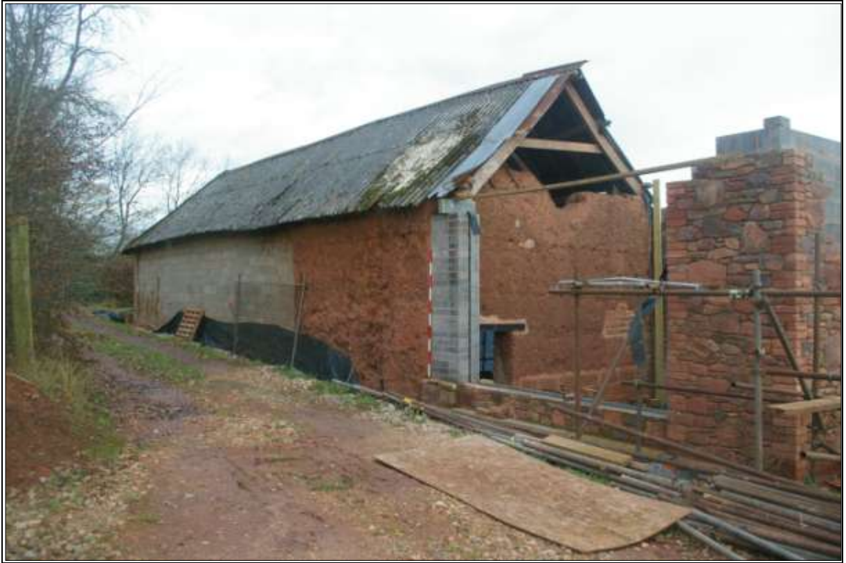
Figure 6: The south and west elevations of the western linhay, surviving in cob to the south end but largely rebuilt in concrete block sometime in the 20 th century; from the south (2m scale).
