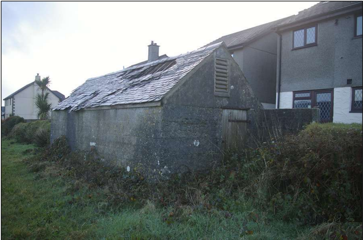
STRUCTURE IN THE SOUTHERN BOUNDARY OF THE SITE; LOOKING SOUTH-EAST.
