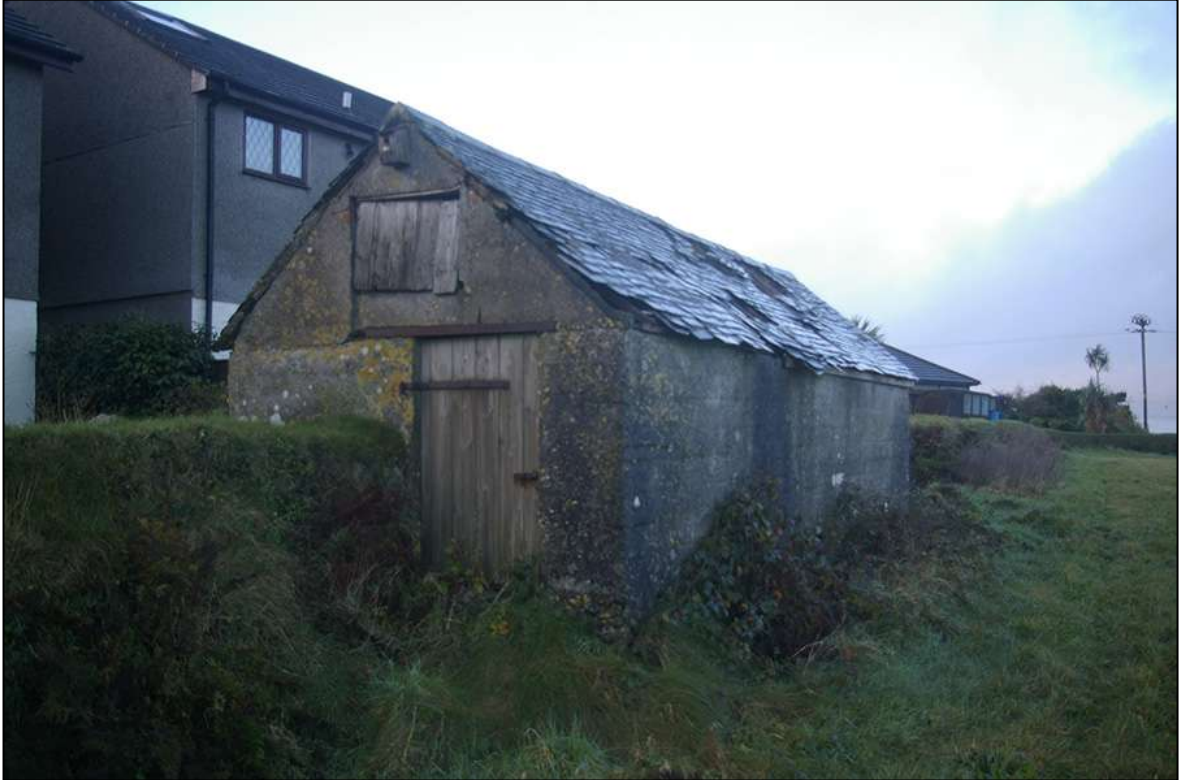
STRUCTURE IN THE SOUTHERN BOUNDARY OF THE SITE; LOOKING SOUTH-WEST.
