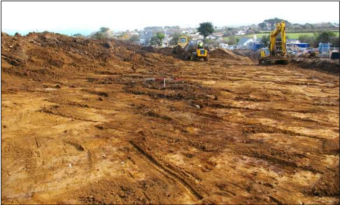
FIGURE 9: DITCH [113]; VIEWED FROM THE EAST (SCALE 2M).
