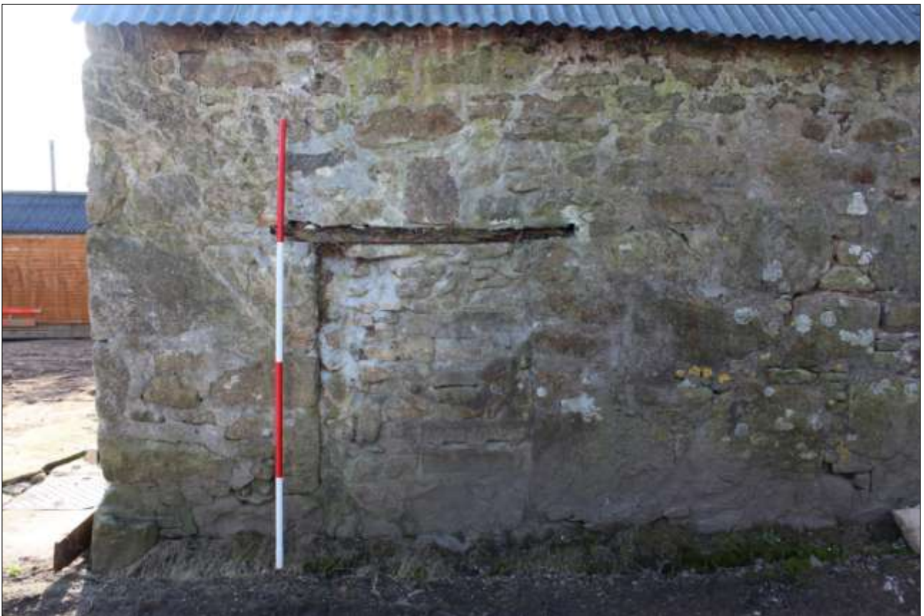
DETAIL OF THE BLOCKED NORTH DOOR IN THE WEST ELEVATION (SCALE 2M).
