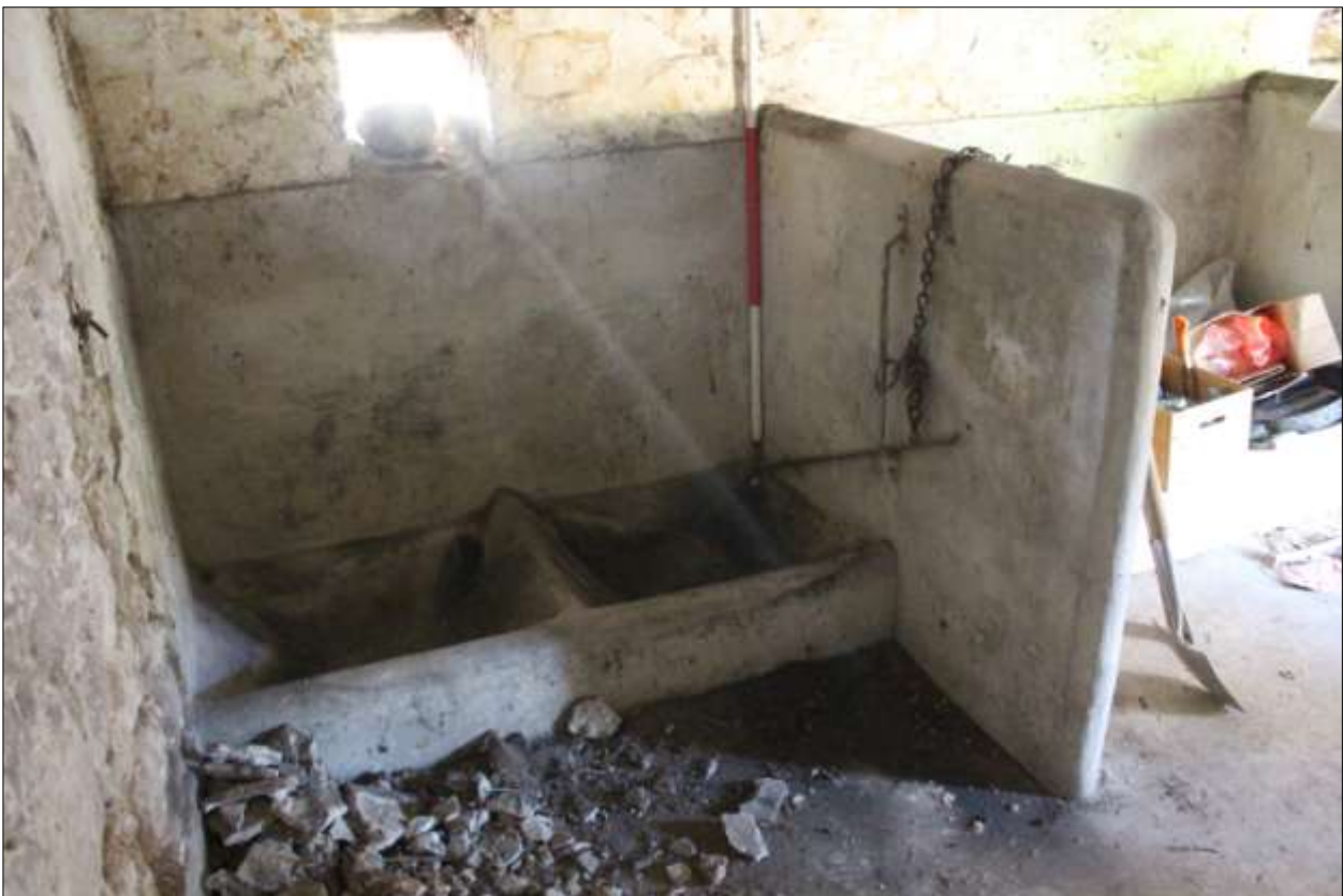
DETAIL OF THE CATTLE STALLS (NORTH END), SHOWING THE INTEGRAL FEED TROUGHS; VIEWED FROM THE WEST (SCALE 2M).
