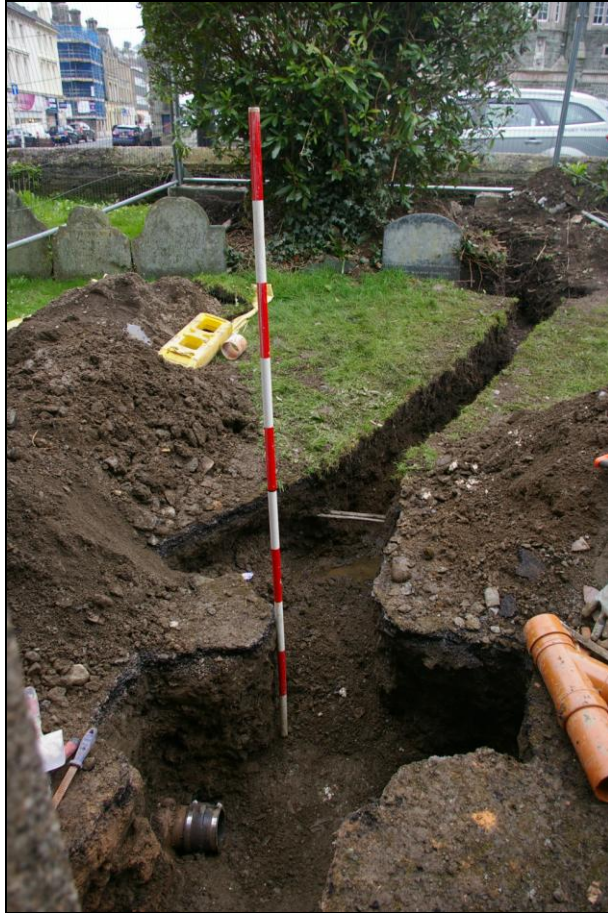
FIGURE 2: POST-EXCAVATION VIEW OF PIPE TRENCH; FROM THE WEST, SOUTH-WEST (2M SCALE).
