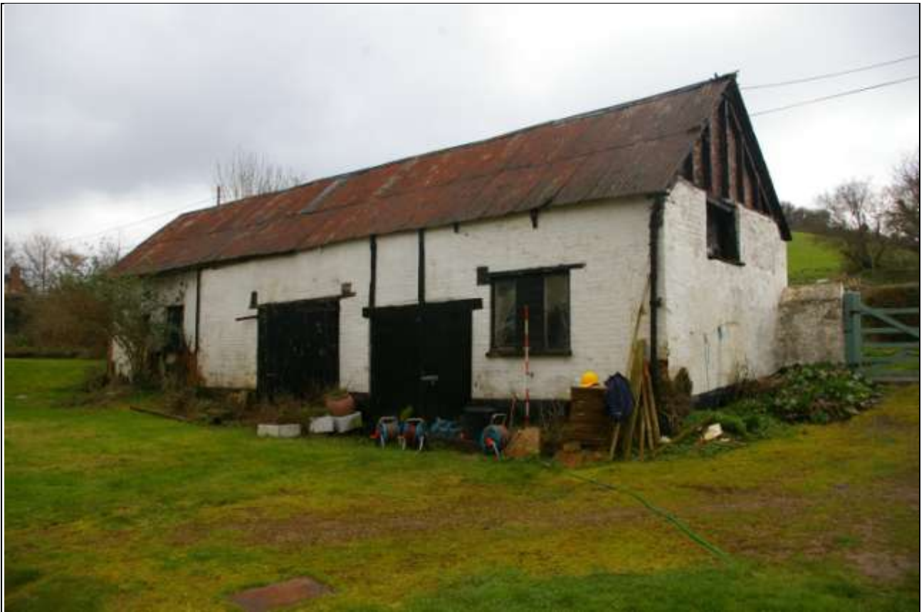
The north and west elevation of the barn; from the north-west.
