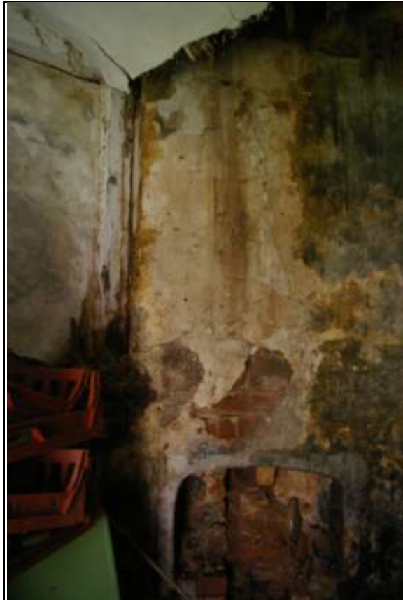
The brick stack and fireplace in room 1; from the north
