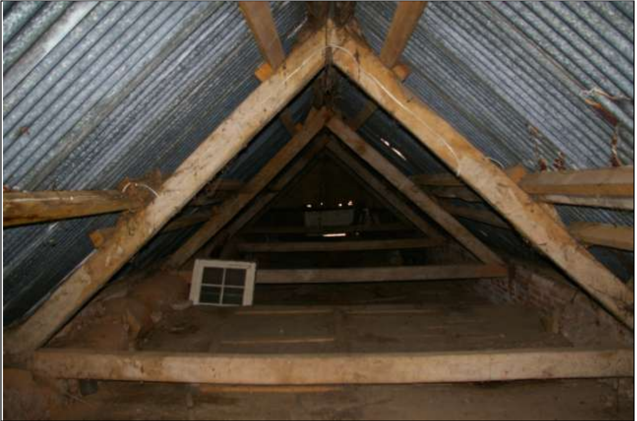
View of the roof structure from the east.
