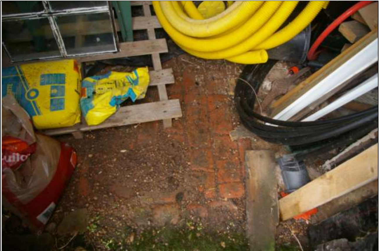
The brick pavers in the west end; from the north.
