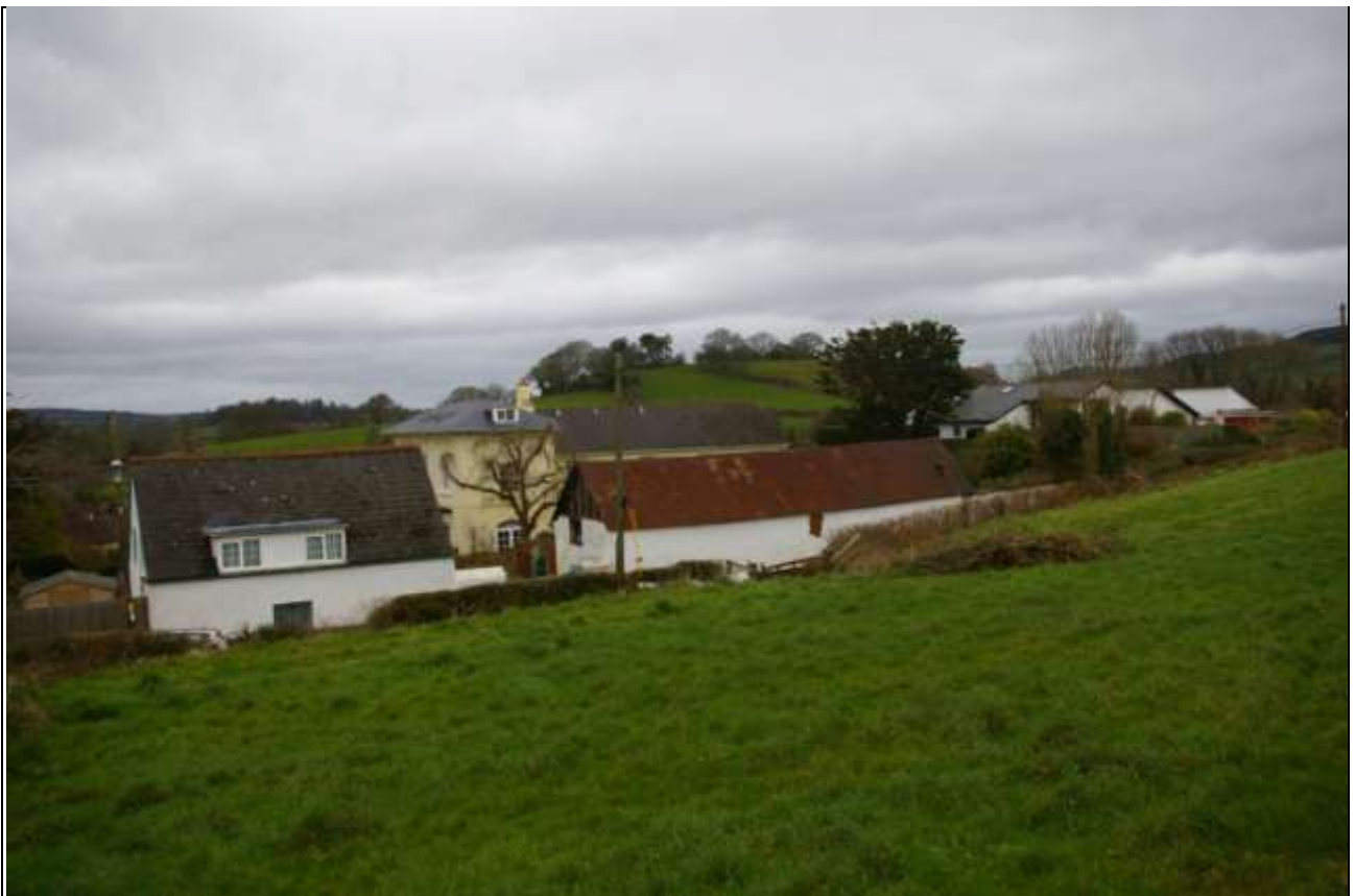
View of the former barns and Coleshayes, The Old Vicarage; from the south-west.
