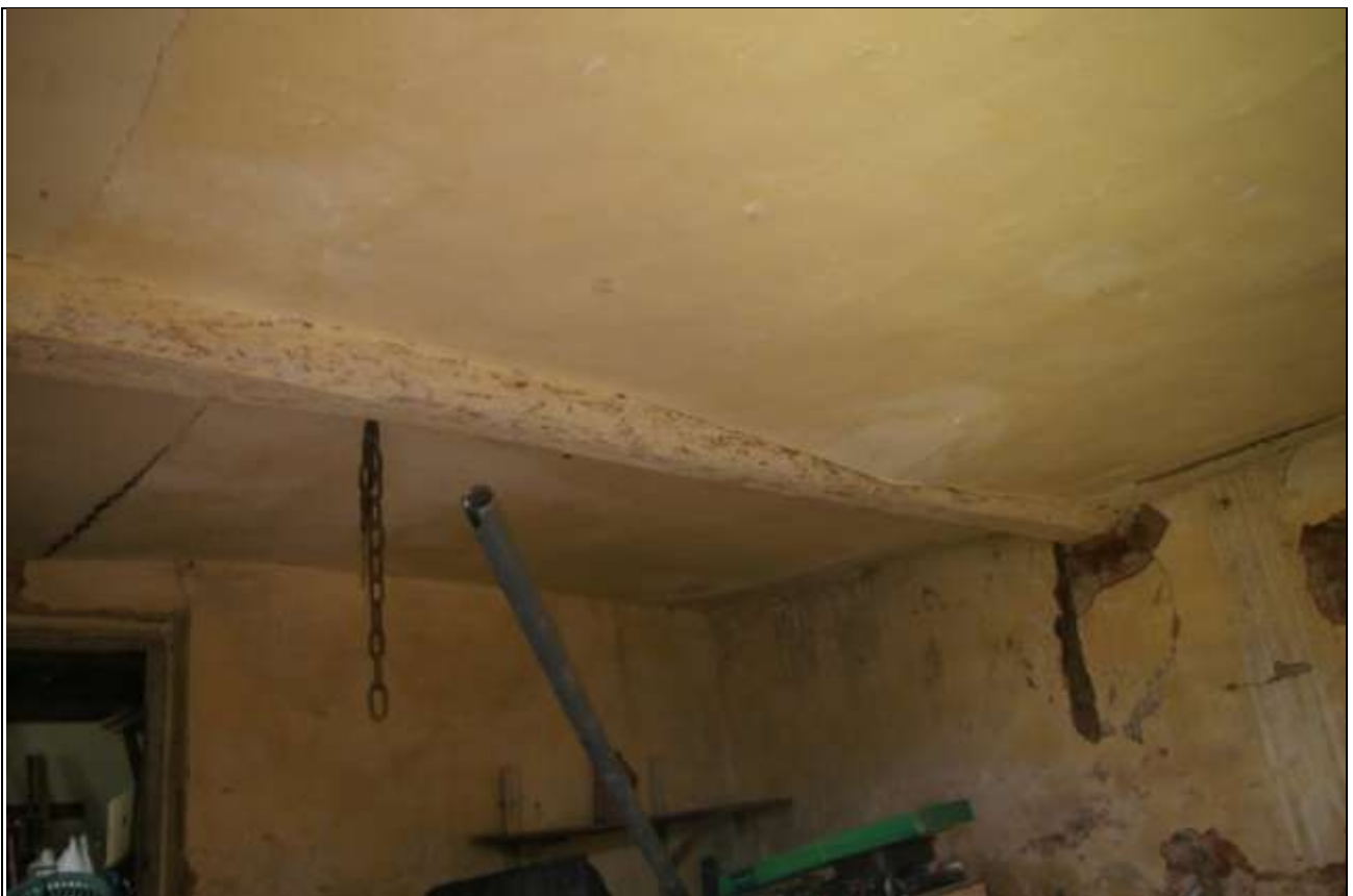
The ceiling beam in room 4, has a narrow chamfer, with run out stops, the base cruck can be seen in the wall to the east side of the beam; from the north-west.
