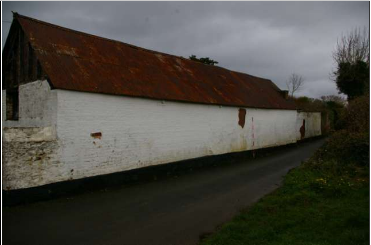
The south elevation along Behind Hayes Lane; from the south-west.
