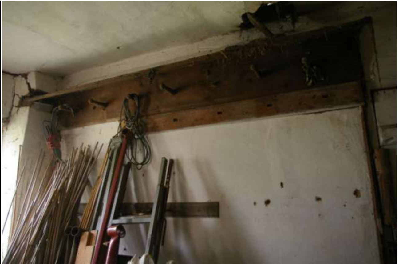
Detailed view of one of the planks, bolted to the wall, with turned pegs, for reins or harness; from the south-west.
