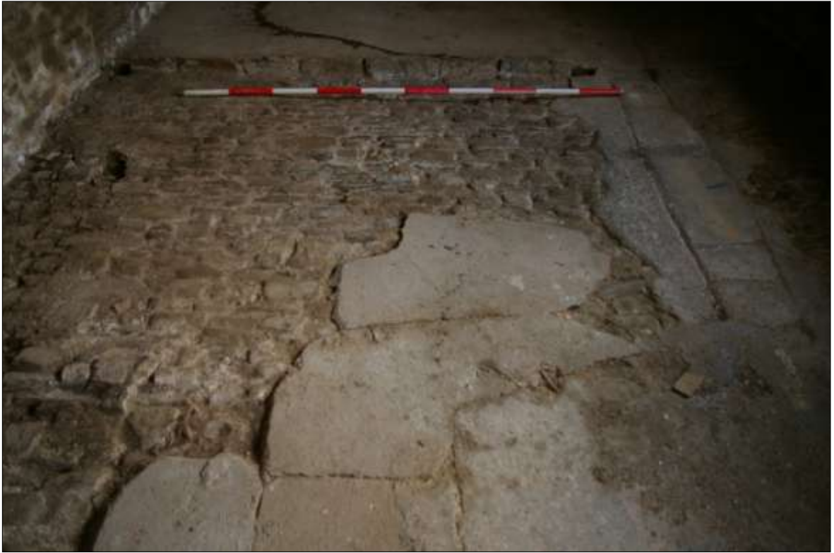
31. DETAIL OF THE CONCRETE SCREED AND ORIGINAL GOOD QUALITY COBBLE FLOORS TO THE EAST OF B1, SHOWING PARTITION SLOTS AND SOCKETS; VIEWED FROM THE WEST (2M SCALE).
