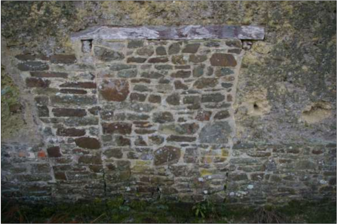
11. DETAIL OF THE BLOCKED DOOR OFF-CENTRE IN THE NORTH EXTERNAL ELEVATION OF B1; VIEWED FROM THE NORTH (NO SCALE).
