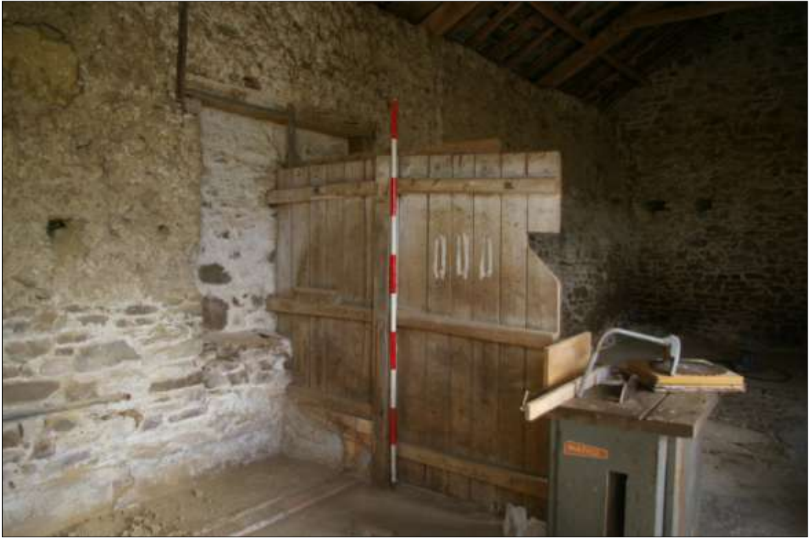
23. DETAIL OF THE TWO PHASES OF BLOCKING OF THE DOOR WITHIN THE NORTH WALL OF B1, AND THE TIMBER PARTITION SCREEN CURRENTLY DIVIDING THE INTERIOR SPACE WITHIN THE OUTBUILDING; VIEWED FROM THE WEST (2M SCALE).
