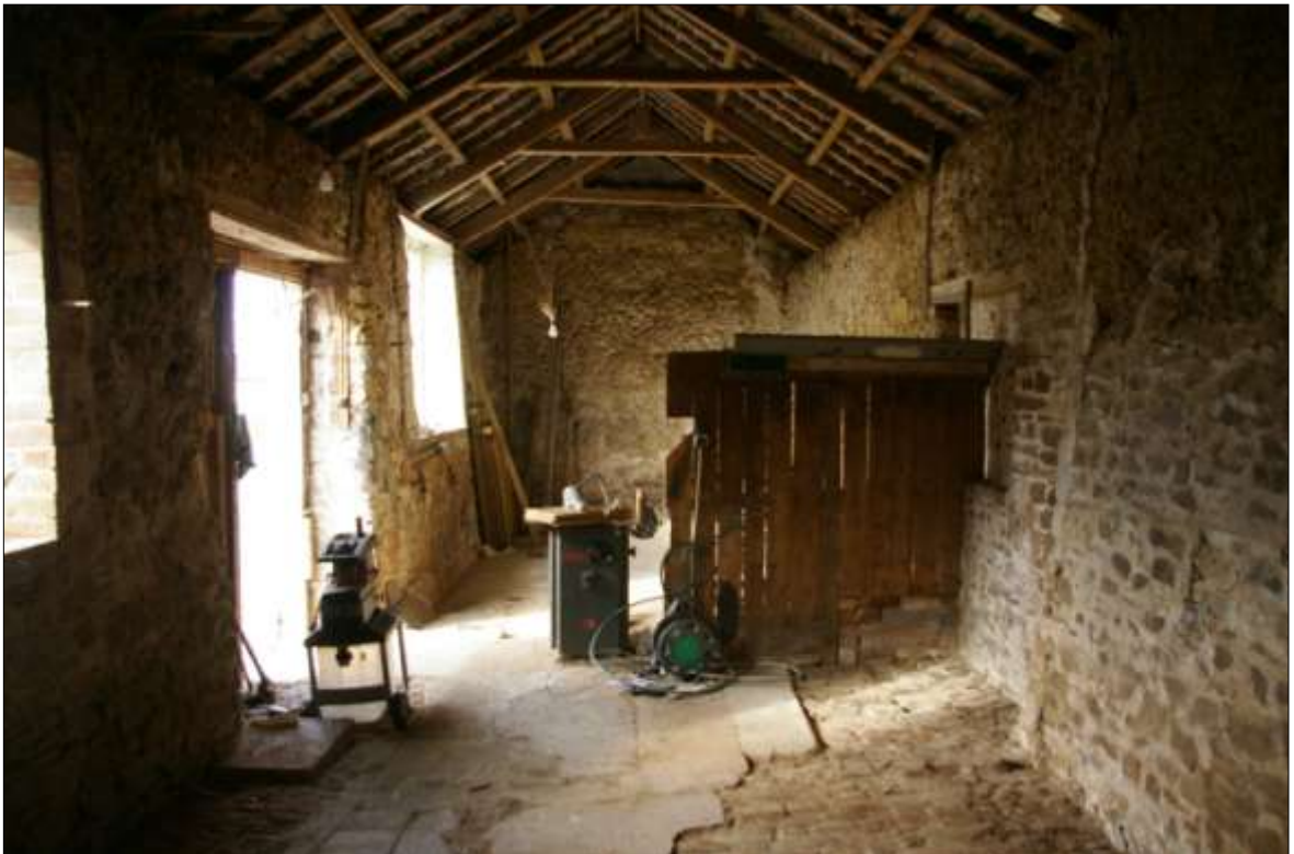
14. THE INTERIOR OF B1; VIEWED FROM THE EAST (NO SCALE).
