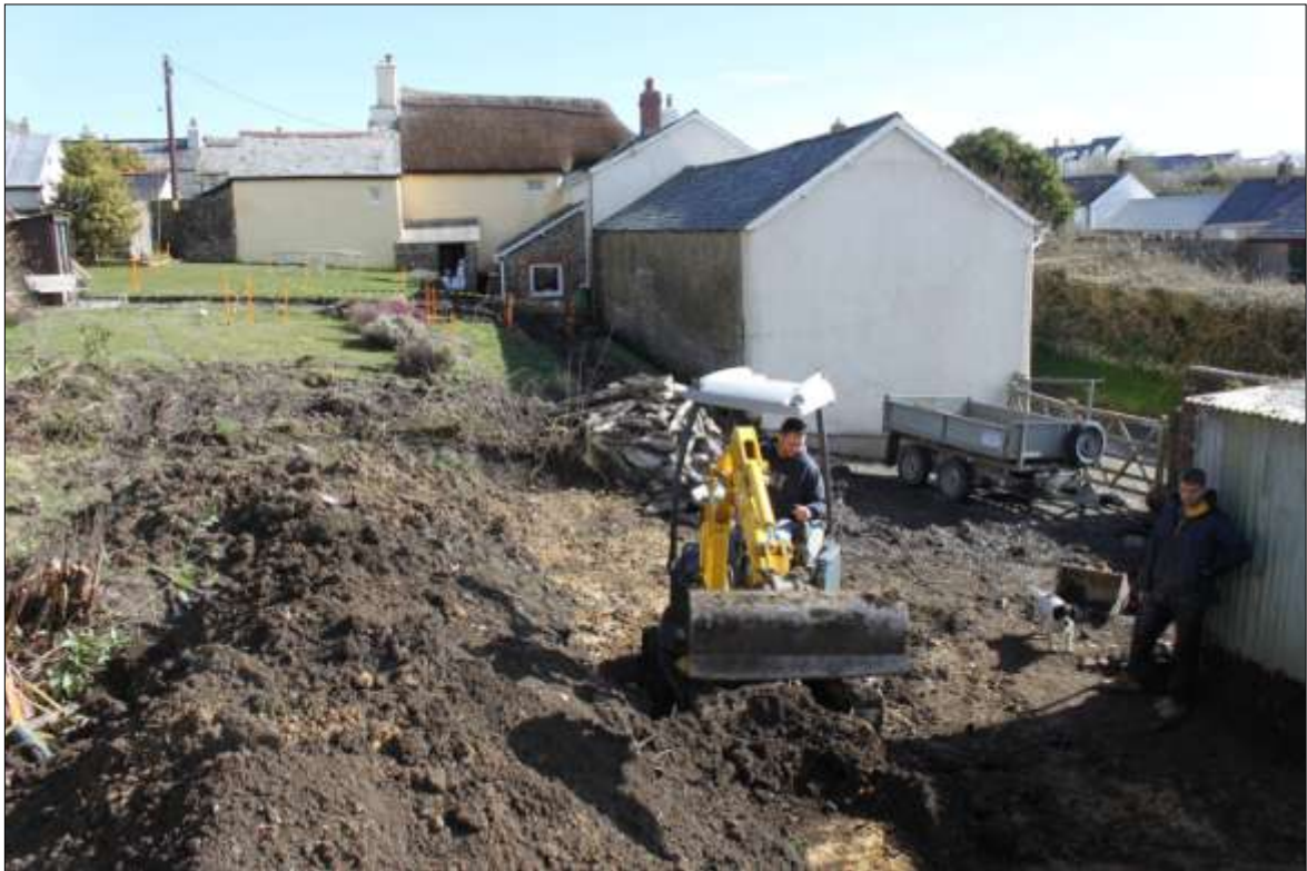
1. GENERAL SITE WORKING SHOT; VIEWED FROM THE WEST (NO SCALE).
