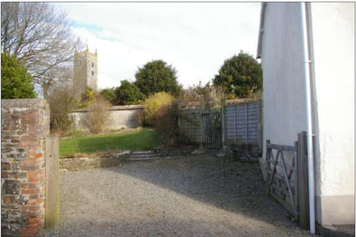
2. VIEW SHOWING B1 IN CONTEXT, WITH THE CLOSE PROXIMITY OF CHURCH BEHIND THE GARDEN WALL; VIEWED FROM THE SOUTH (NO SCALE).
