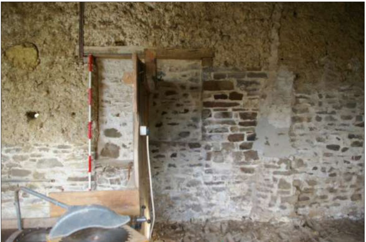
24. DETAIL OF THE BLOCKED DOORWAY IN THE NORTH WALL OF B1, SHOWING DETAIL OF THE TAPERED OPENING, WIDER TO BOTTOM; VIEWED FROM THE SOUTH (2M SCALE).
