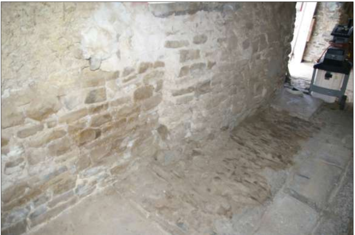
28. DETAIL OF THE CLEAR BUILD LINE IN THE INTERNAL ELEVATION OF THE SOUTH WALL OF B1, WHERE THE GOOD BATTERED STONWORK ENDS AND IS ABUTTED BY A SHORT STRETCH OF 19TH CENTURY CHARACTER RUBBLE; VIEWED FROM THE NORTH-EAST (NO SCALE).
