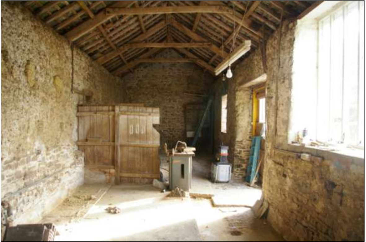
13. THE INTERIOR OF B1; VIEWED FROM THE WEST (NO SCALE).
