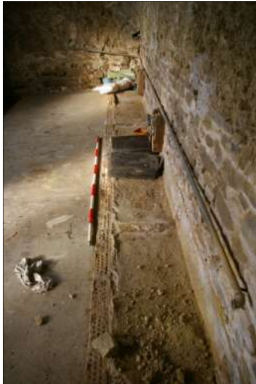
30. DETAIL OF THE BRICK AND LIME/CEMENT MIX BUILT CATTLE TROUGH, USING A MIX OF RECYCLED BRICKS, SOME HANDMADE, WITH RAISED CONCRETE PLINTH INDICATING THE WEST END OF THE OUTBUILDING WAS USED FOR A TIME AS A MILKING PARLOUR IN THE EARLY 20TH CENTURY AND POSSIBLY EARLIER; VIEWED FROM THE EAST (2M SCALE).
