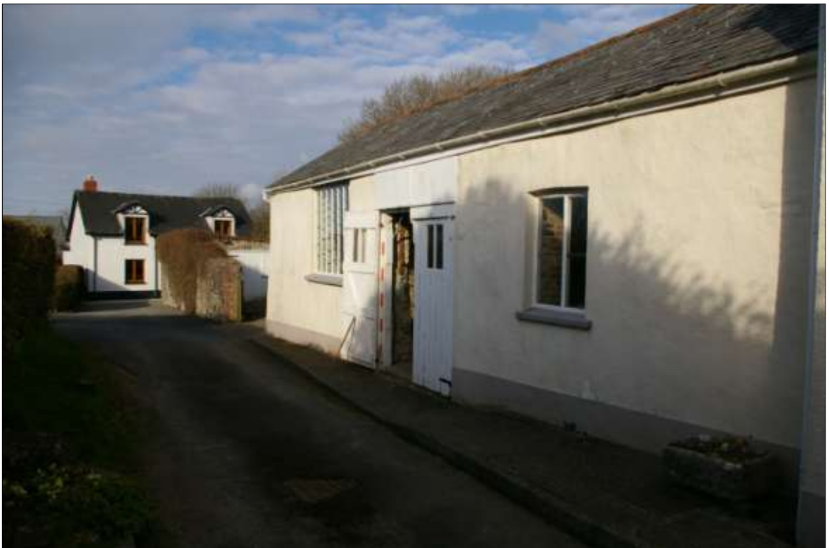
4. THE SOUTH EXTERNAL ELEVATION OF B1; VIEWED FROM THE SOUTH-EAST (2M SCALE).
