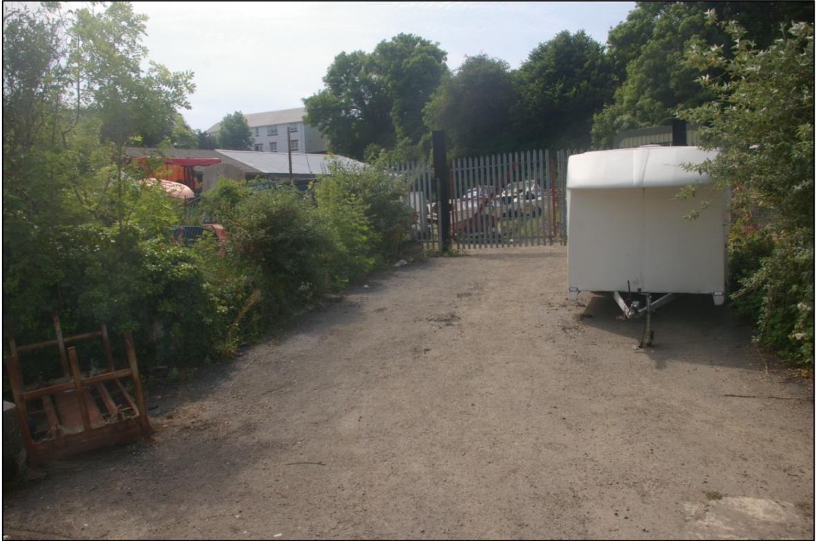
FIGURE 9: VIEW OF THE MAIN COMPOUND OF THE DEPOT SITE, SHOWING SECURITY FENCING AND GATES.
