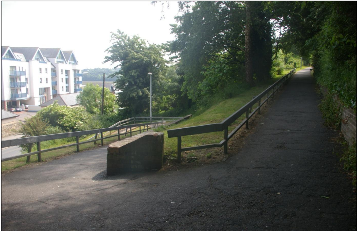
FIGURE 12: VIEW OF THE DENSE FOLIAGE AT THE NORTHERN END OF THE SITE, FROM THE ZIG-ZAG PATH TO DEVONSHIRE PARK; NORTH-WEST.
