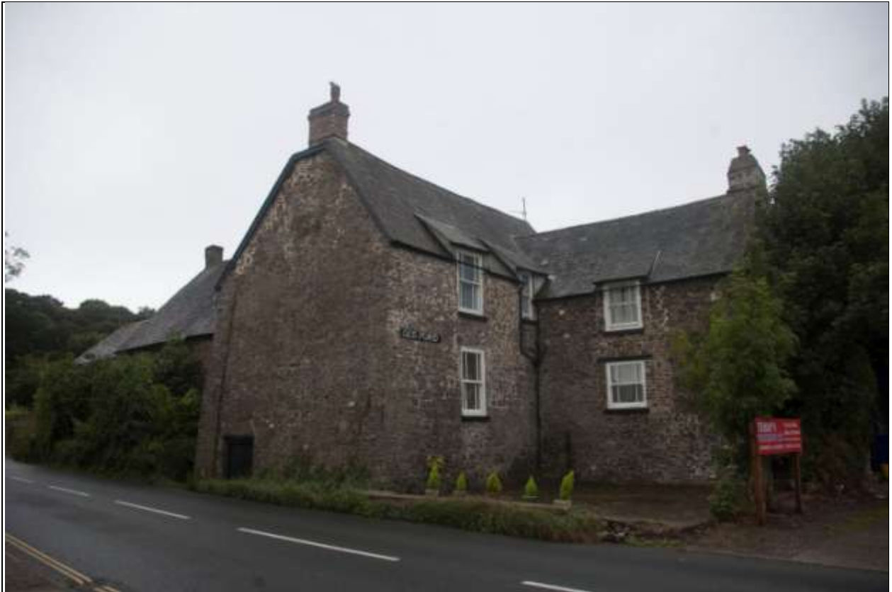
Old Ford house, showing its battered thick medieval stone walls and later 19 th century sash windows; from the north-east.
