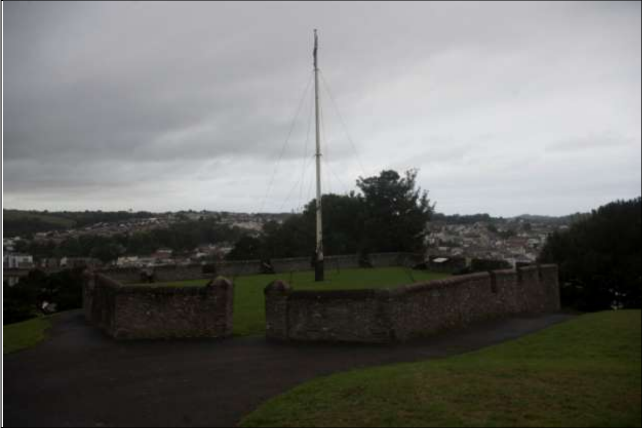
Chudleigh Fort, rebuilt in the 19 th century as a park feature; from the east, south-east.
