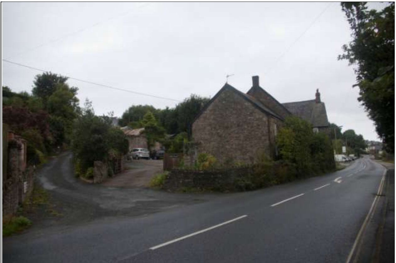
Old Ford from the south, with its small courtyard, small service building and modern houses on the slope above. The busy A386 close to the walls of the building; from the south, south-east.
