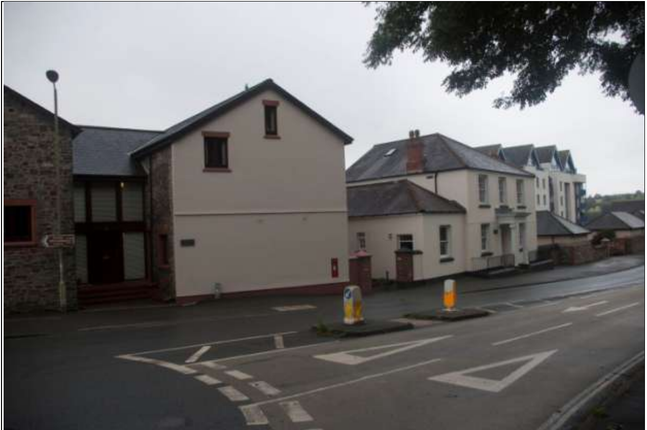
St Davids, from the busy roundabout, showing more warehouse style buildings to the north of the building, with the larger Longbridge Wharf buildings behind; from the north-west.
