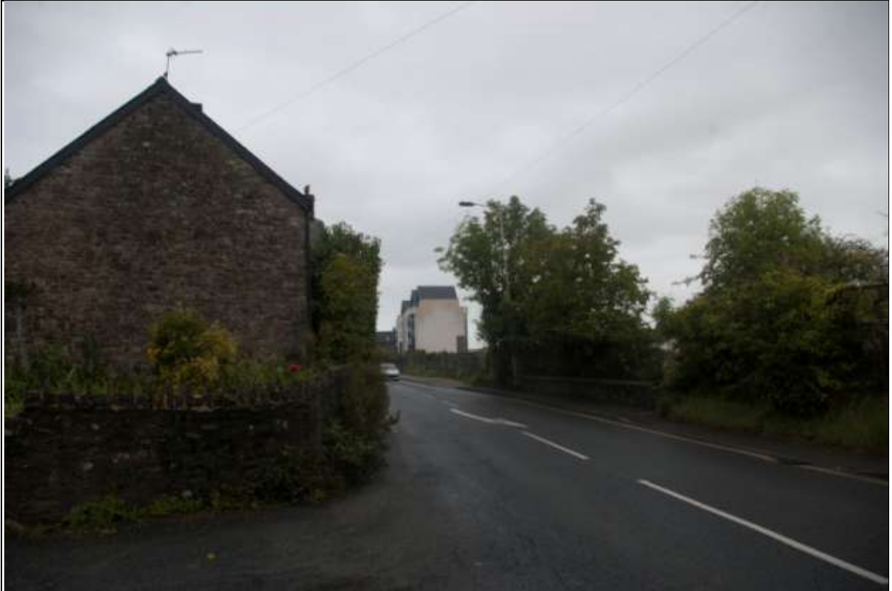
Shot along the A386 towards the Longbridge Wharf building development, showing the open ground between and the relative massing of the buildings; from the south, south-west.
