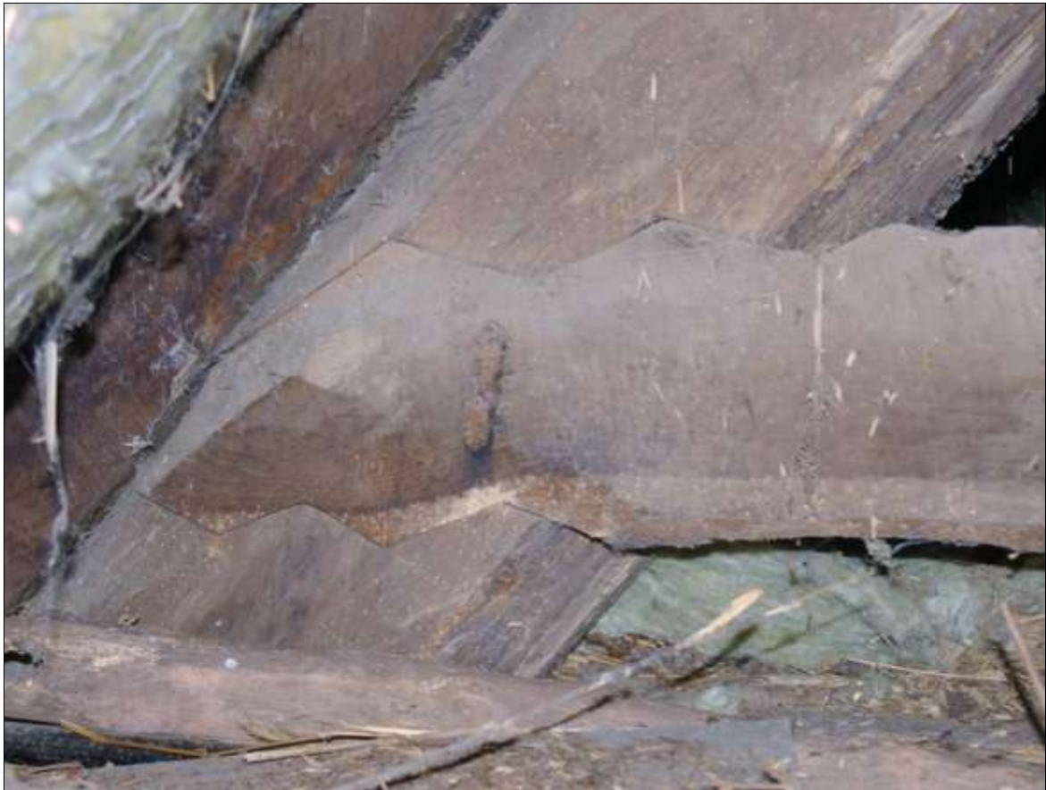
Figure 8 Detail of collar joint with truss blade over central section.
