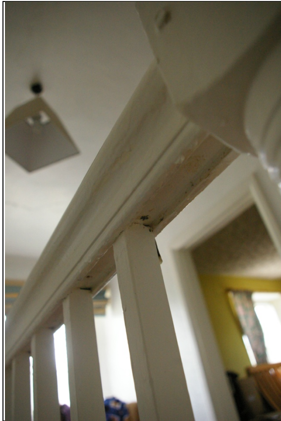
Detail of the balusters, set into the hand rail; viewed from the south-west.
