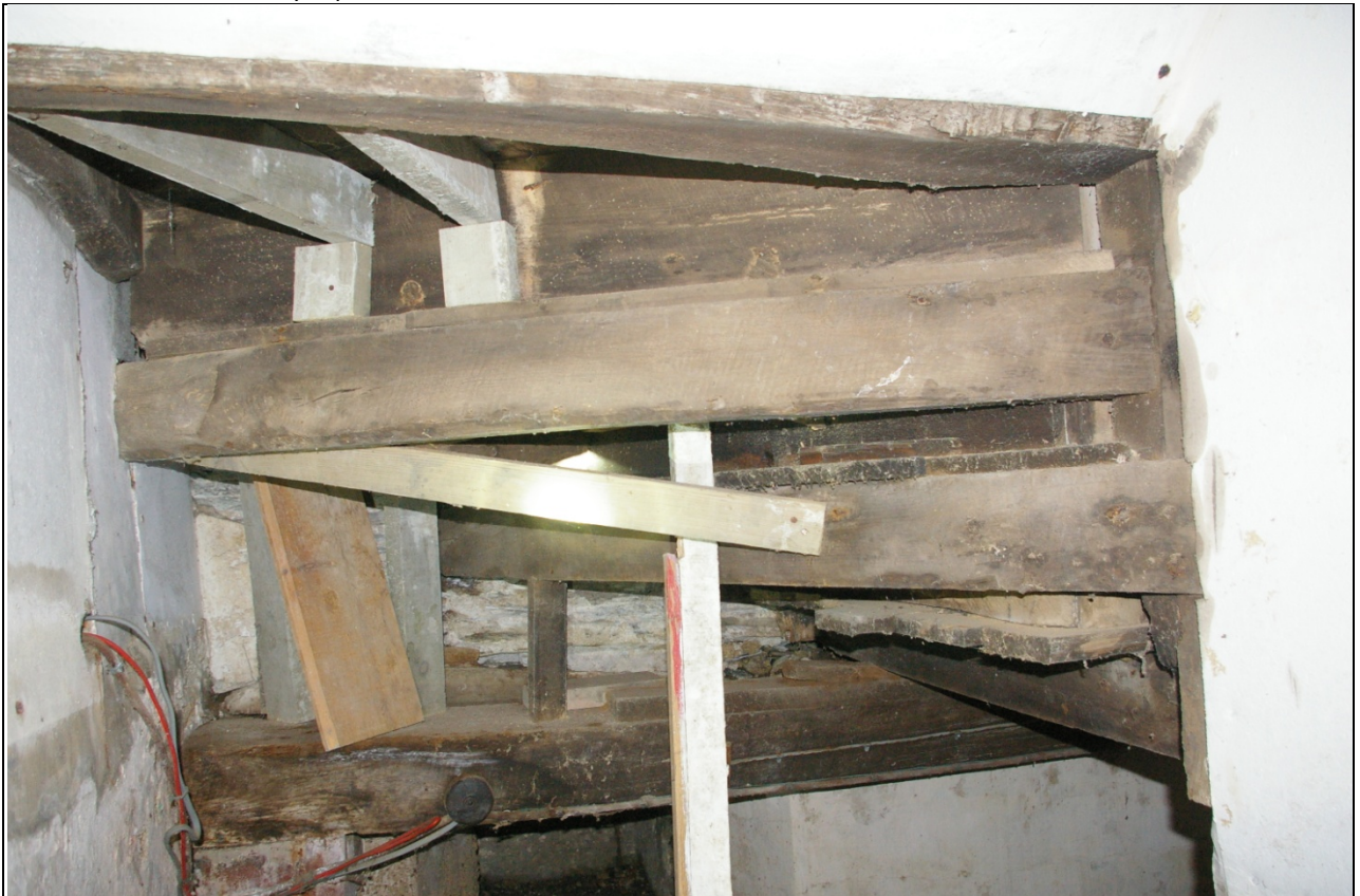
Shot of the base of the stair, the winder steps, showing 20 th century bracing; viewed from the south-east.
