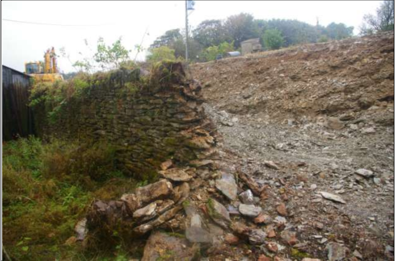
View of Area 1, the rear revetment wall and area excavated behind; from the south-east.
