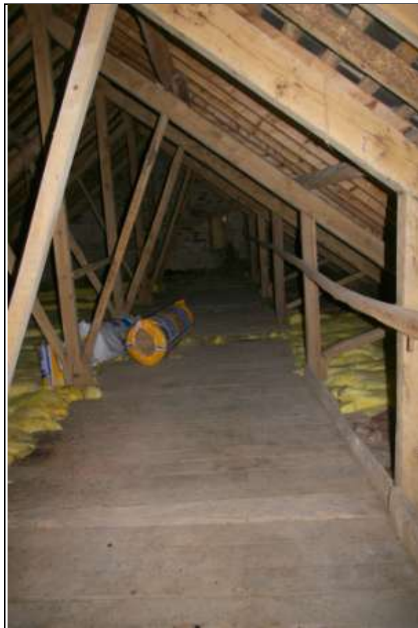
View along the boarded section of flooring; from the west.
