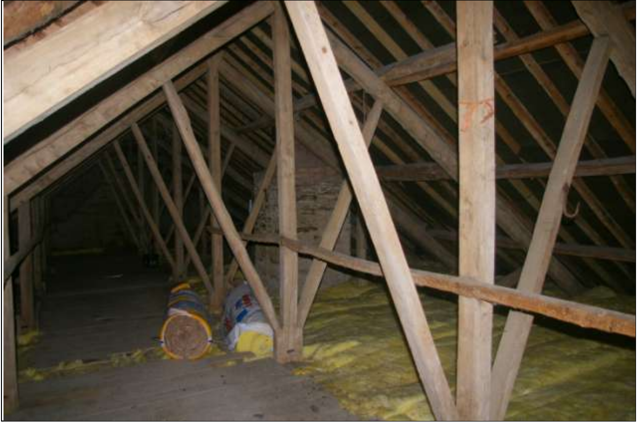
View down the length of the roof; from the east-south-east.
