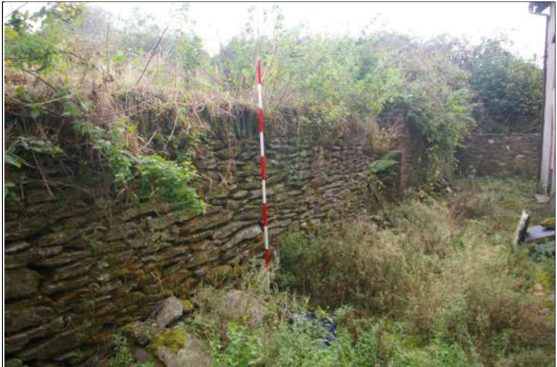
Figure 10: The northern retaining wall before demolition, viewed from the south-west (2m scale).
