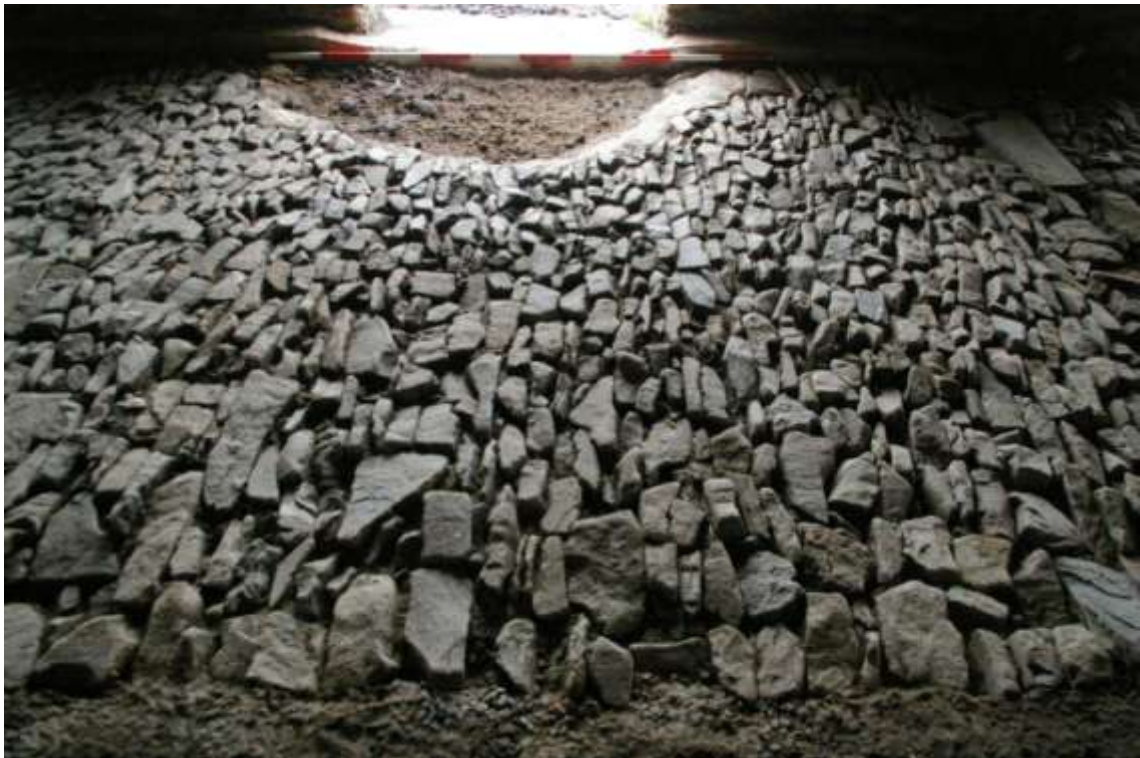
East of centre arch threshold, with 2m scale; from the north.
