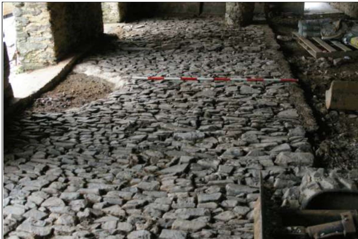
Figure 13: The cobbled floor following power-washing; viewed from the east.
