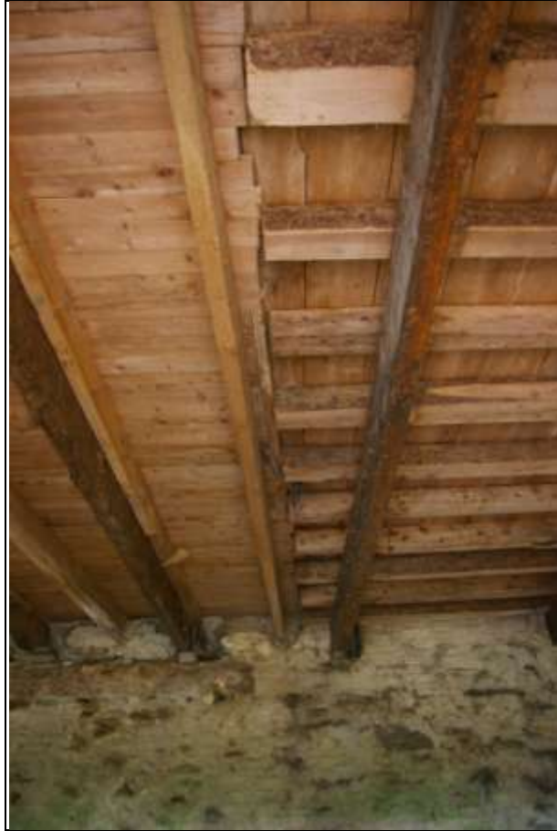
The rough join between the two types of flooring; from the south.
