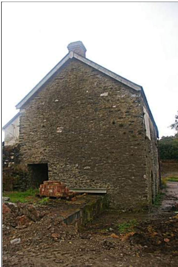
Figure 7: The west elevation of the East Barn; viewed from the south-west.
