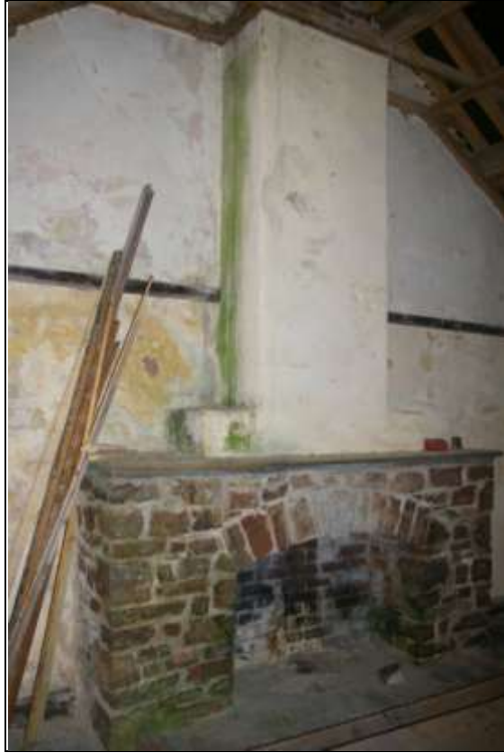
The chimney stack in the living room; from the south-east.
