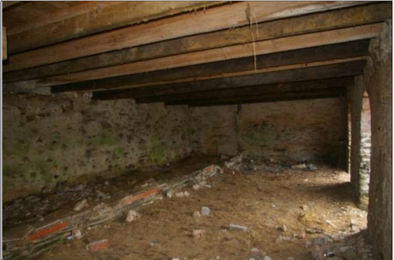
The ground floor interior of the bank barn; from the south-west.
