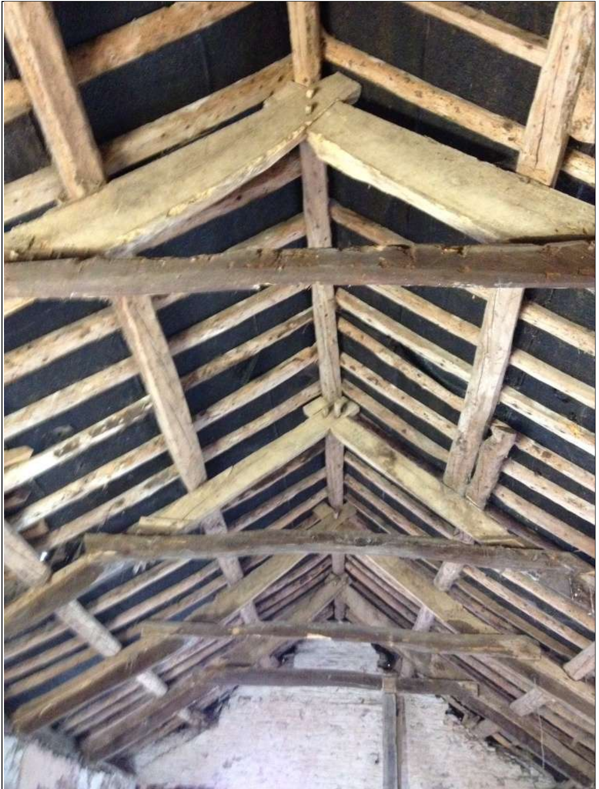
Figure 12: Shot of the roof following the removal of the plaster ceilings.
