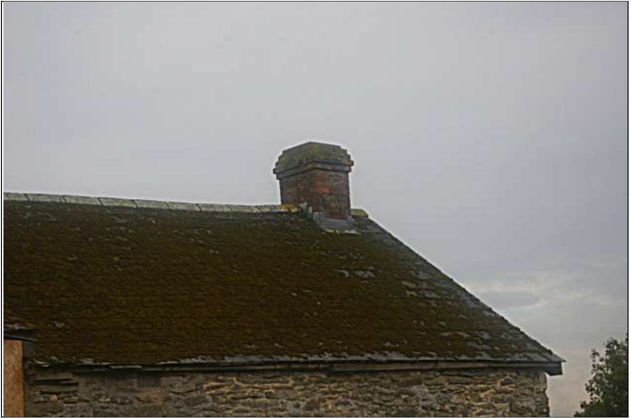
Detailed view of the repaired brick stack; from the north-east.
