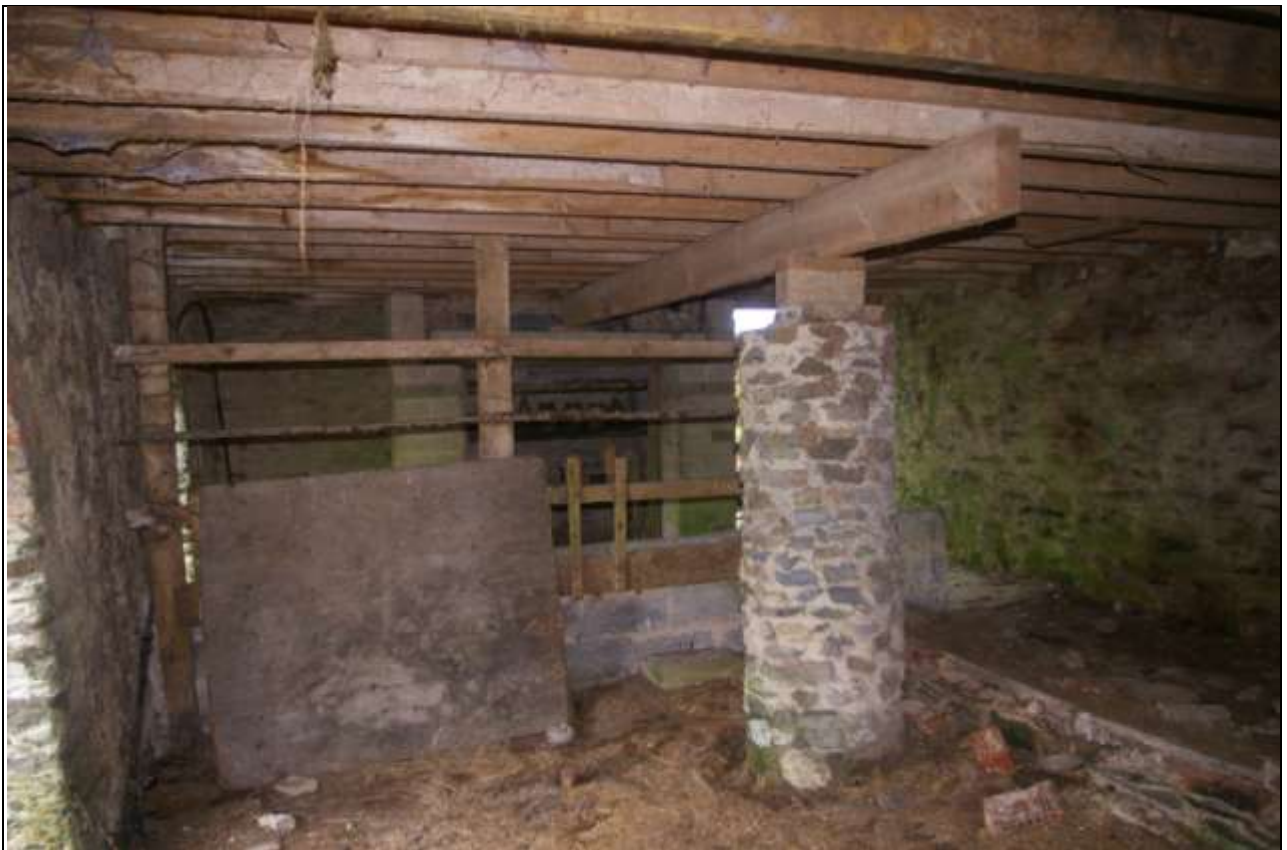
The round pillar supporting the floor to the west; from the south-east.
