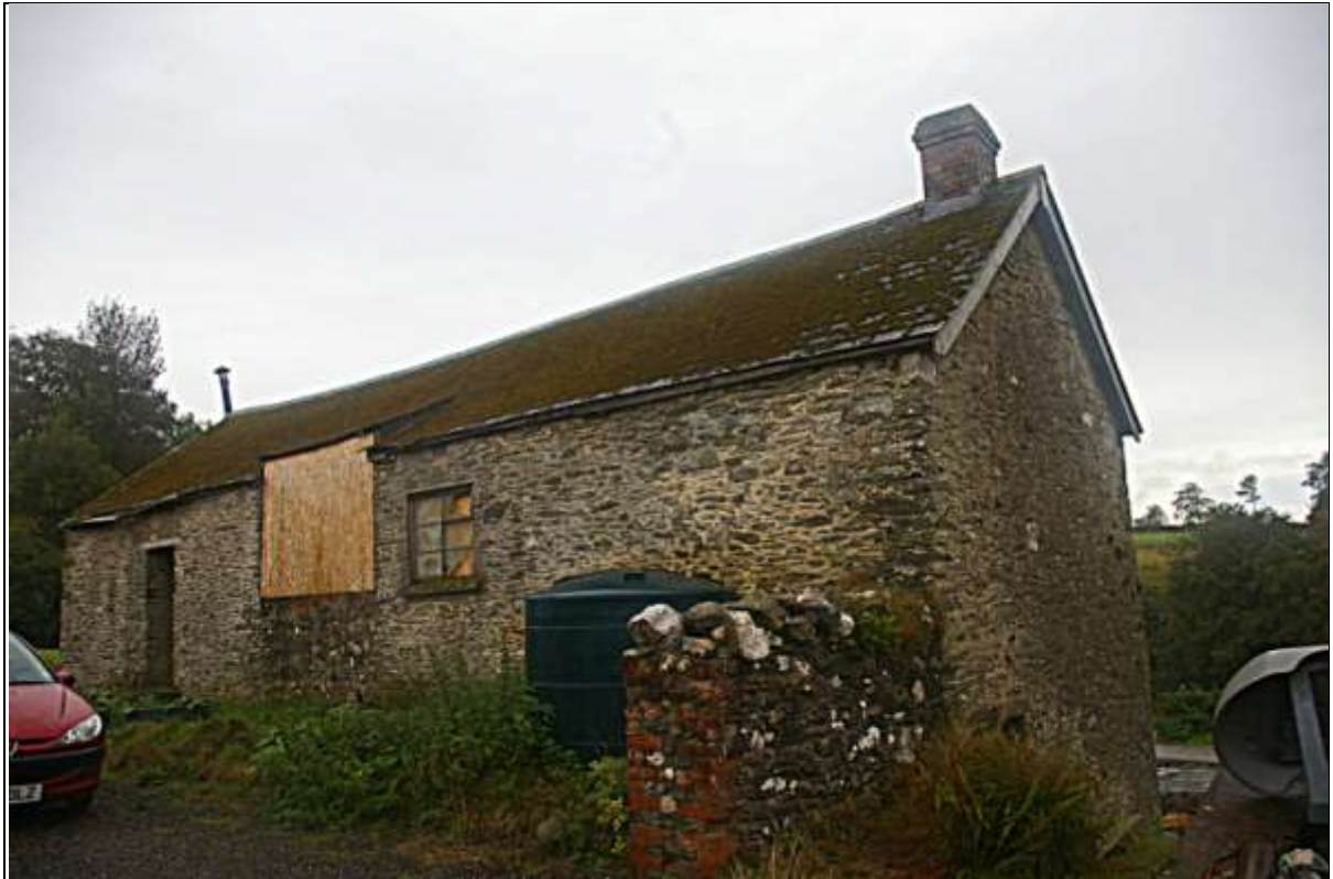
Figure 8: Shot along the north elevation; viewed from the north-west.
