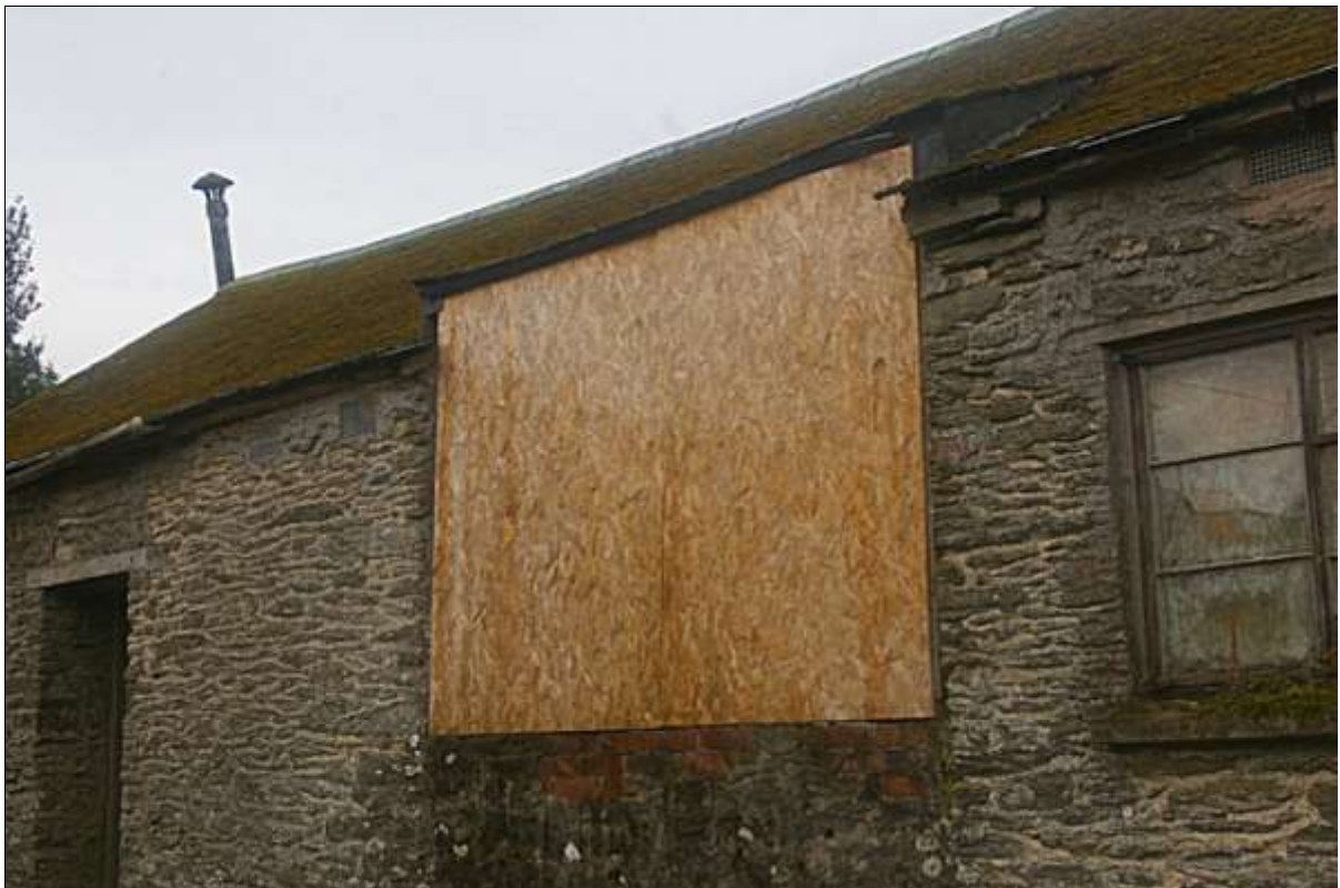
Detail of the 'Somerset' dormer; from the north-west.
