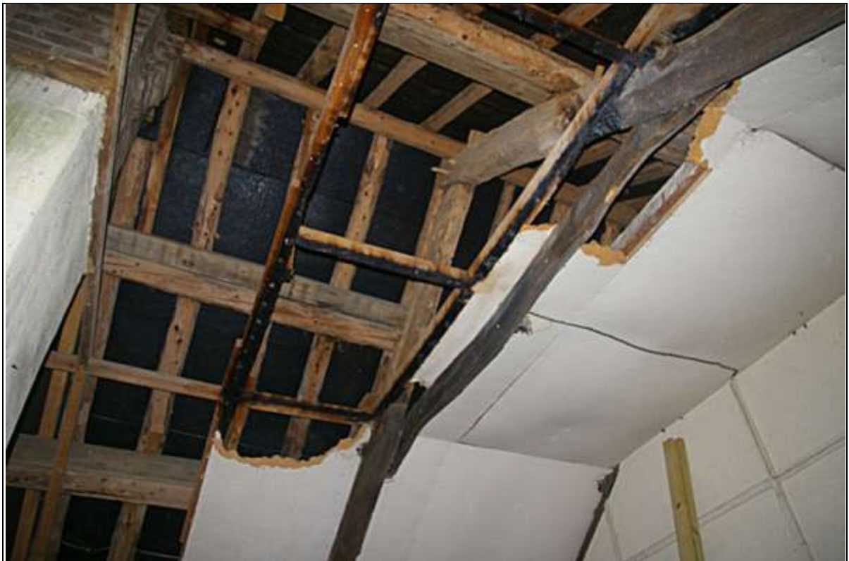
Figure 11: The roof structure; from the south-south-west.
