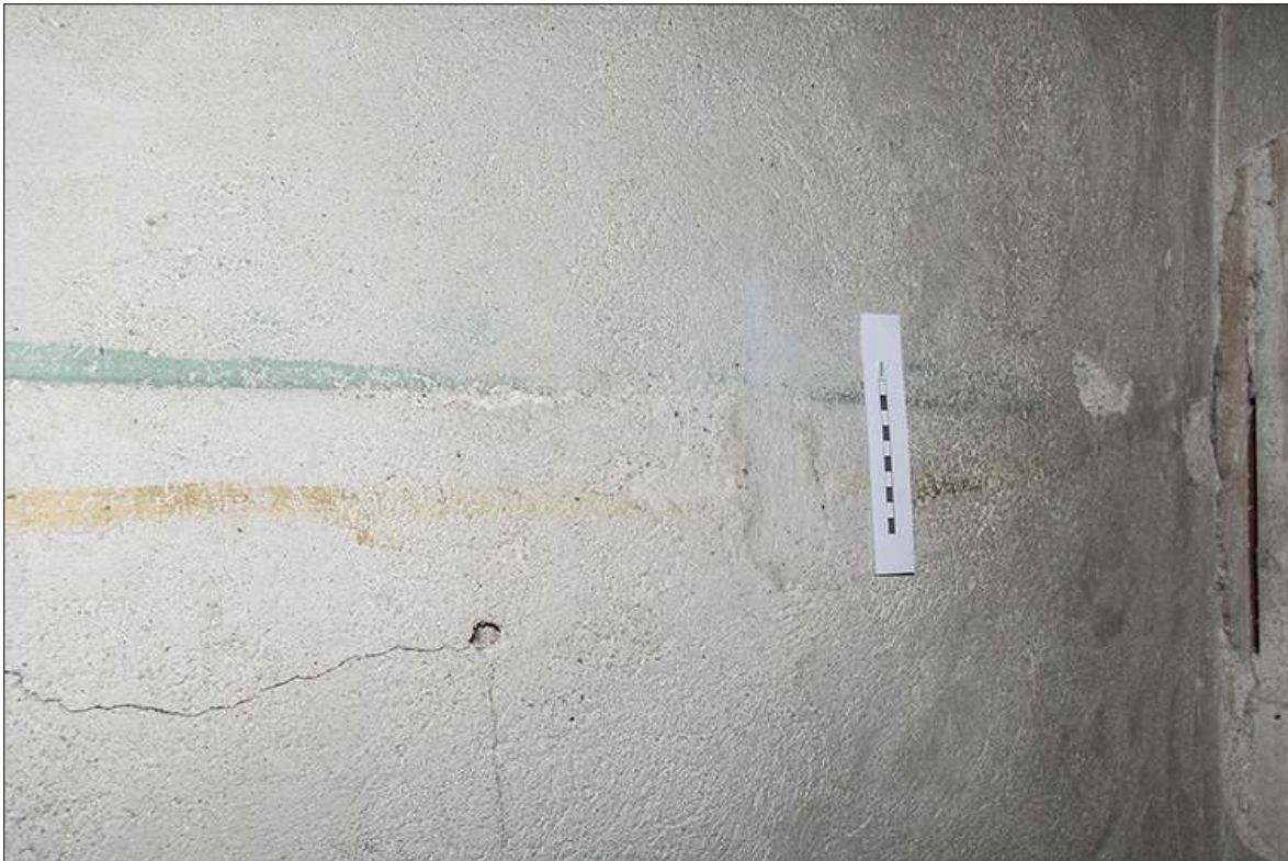
Figure 15: 6041 Detail of the partition marks south of the moulded oak beam; viewed from the north-west (scale 10cm).
