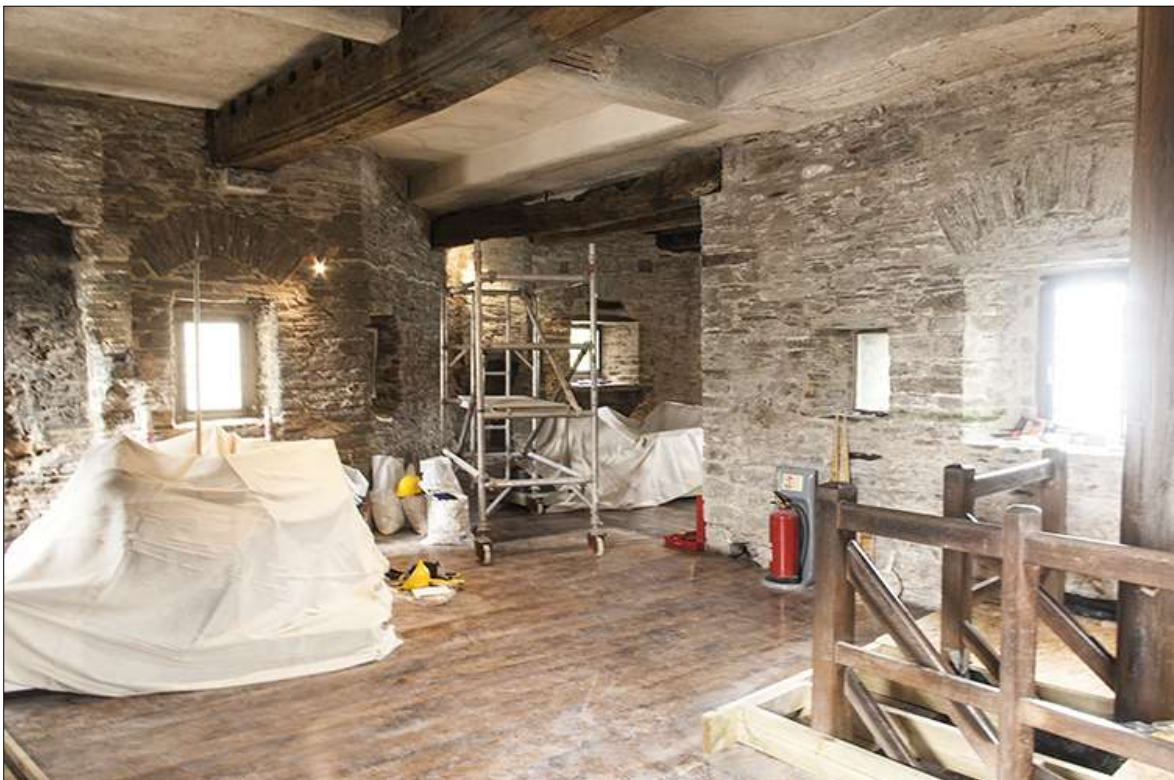
Figure 9: 6022 The north-west corner of the tower; viewed from the south-east.
