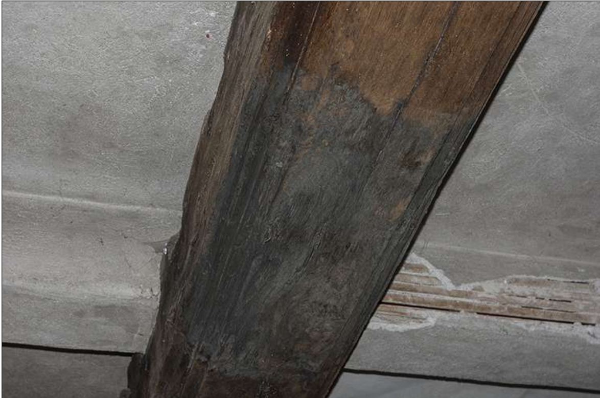
Figure 12: 6011 Detail of the grey paint on the original moulded oak beam, which appears to correspond with the re-established partition marks on the ceiling; viewed from the south-east.
