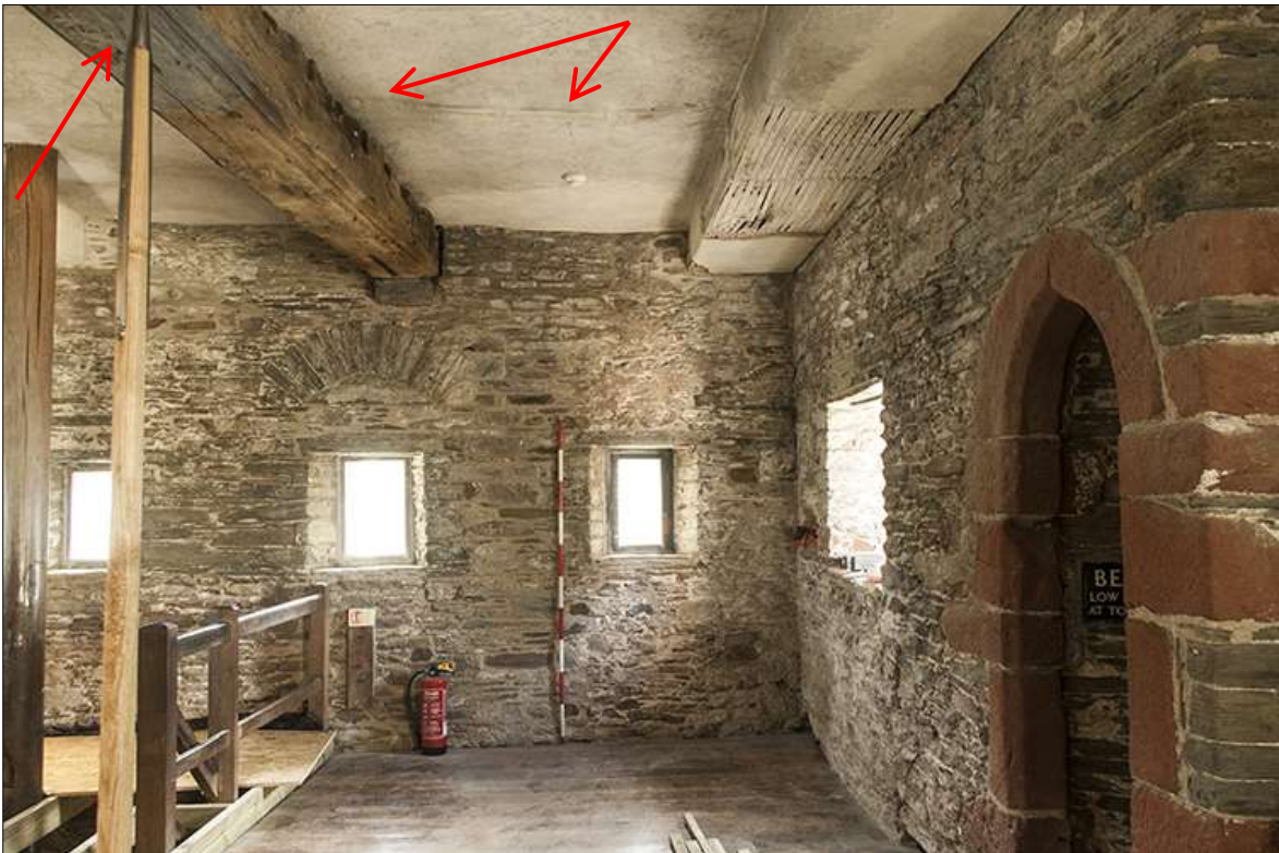
Figure 3: 5991 The south side of the tower; viewed from the south west (scale 2m). The grey paint on the moulded oak beam and partition marks are indicated.
