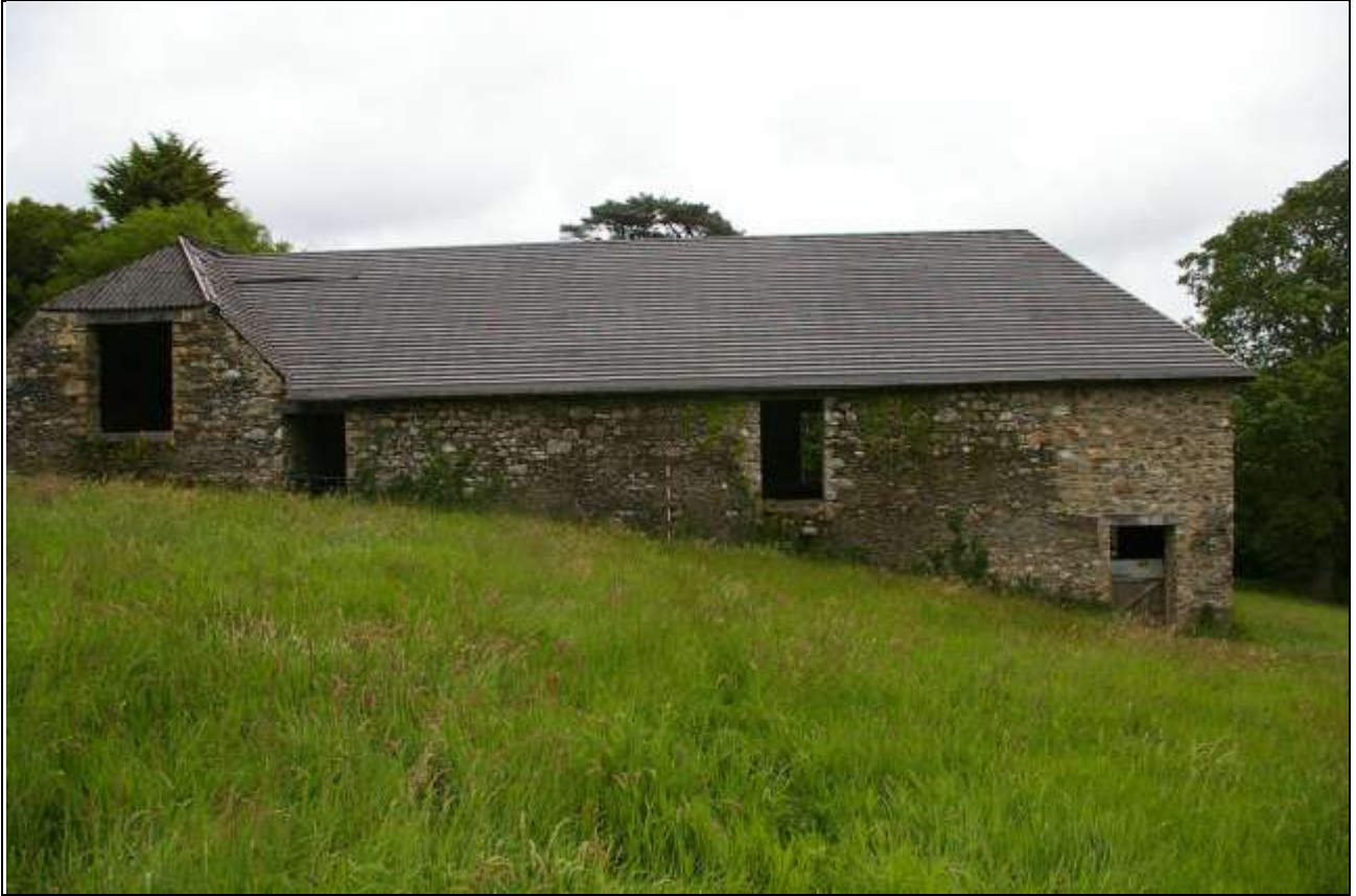
FIGURE 10: WEST ELEVATION BARN A; FROM THE WEST-SOUTH-WEST (2M SCALE).
