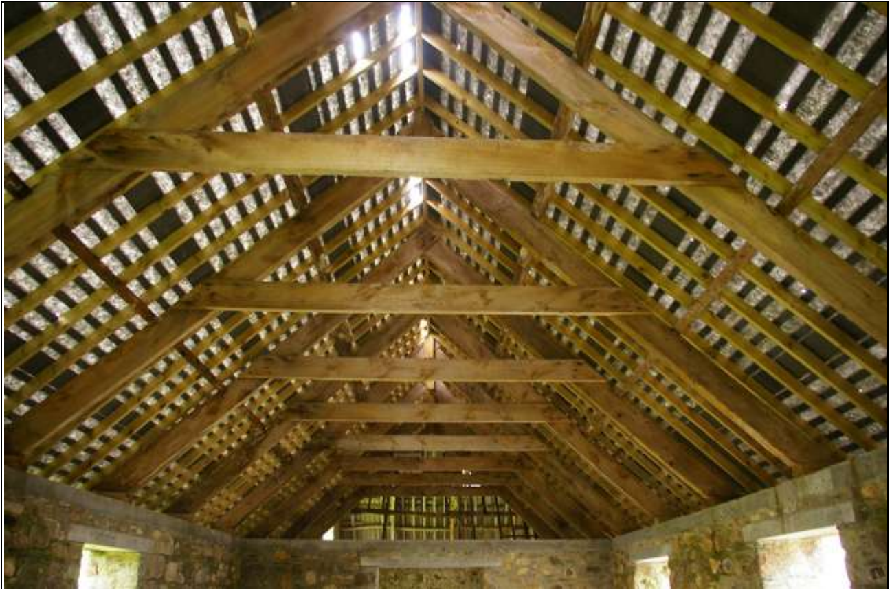
FIGURE 12: ROOF STRUCTURE BARN A; FROM THE SOUTH.
