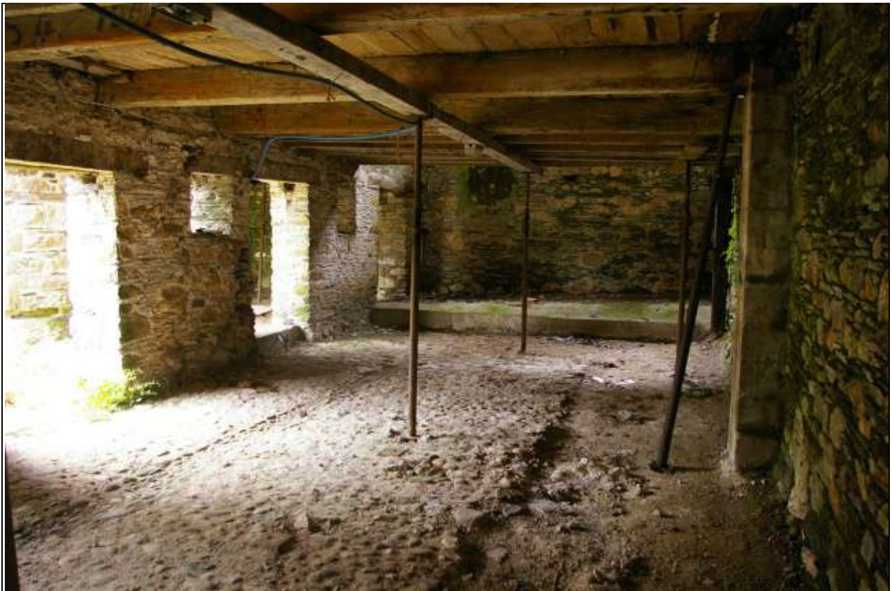
FIGURE 35: THE INTERIOR OF BARN B, FROM THE NORTH-EAST CORNER.
