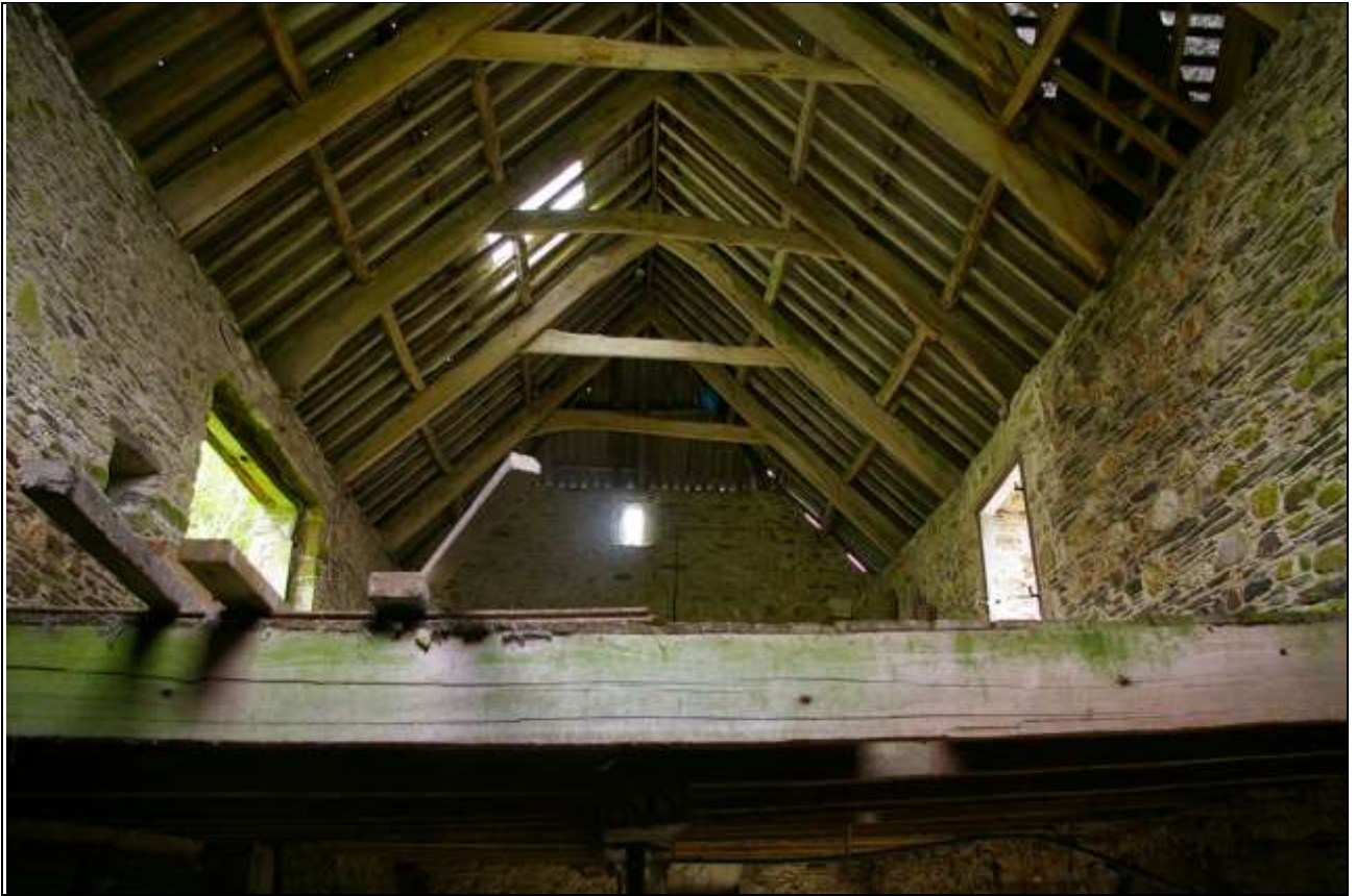
FIGURE 44: VIEW UP TO ROOF IN BARN B; FROM THE WEST.
