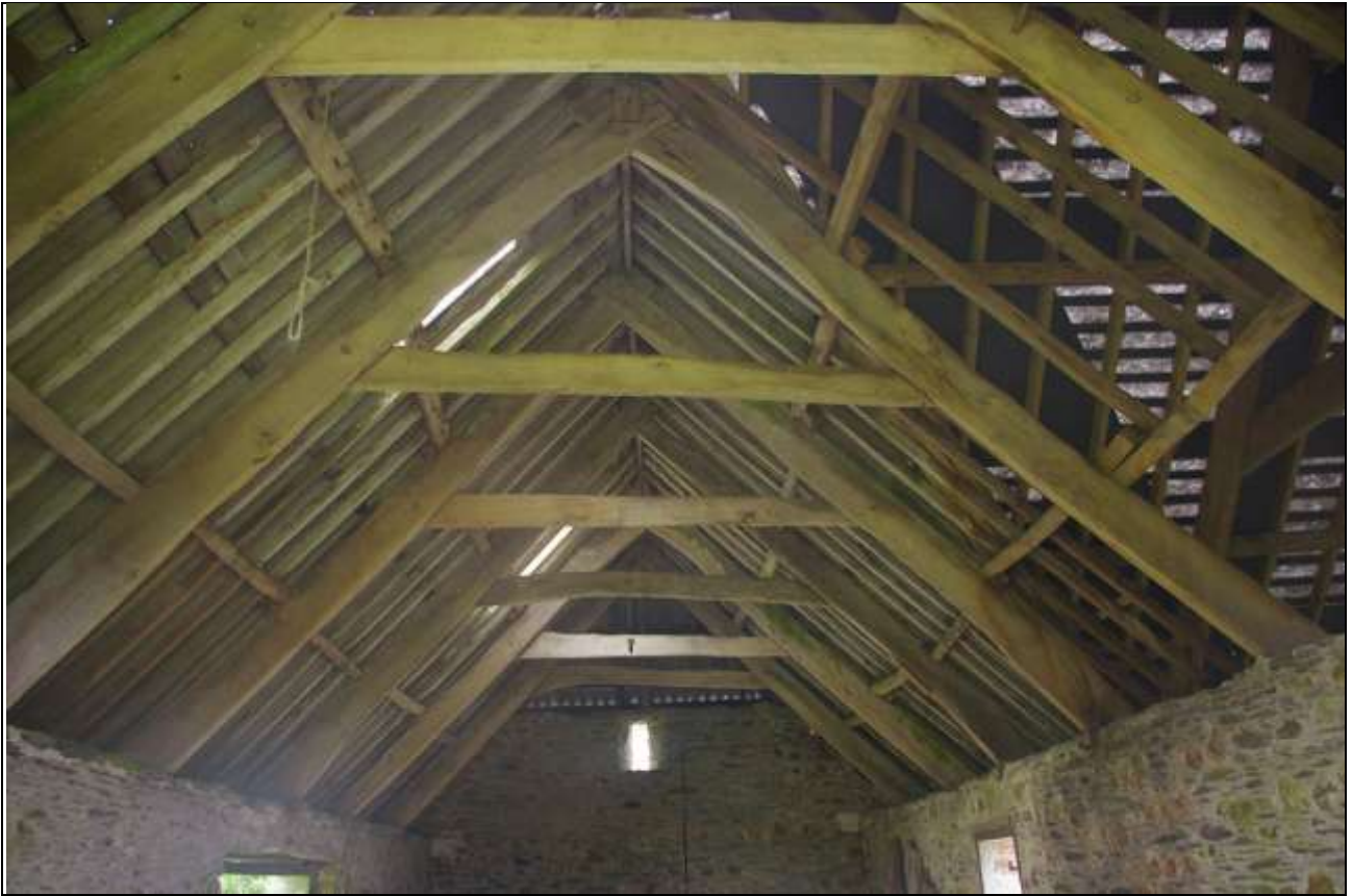
FIGURE 8: GOOD QUALITY ROOF STRUCTURE IN BARN B; FROM THE WEST.
