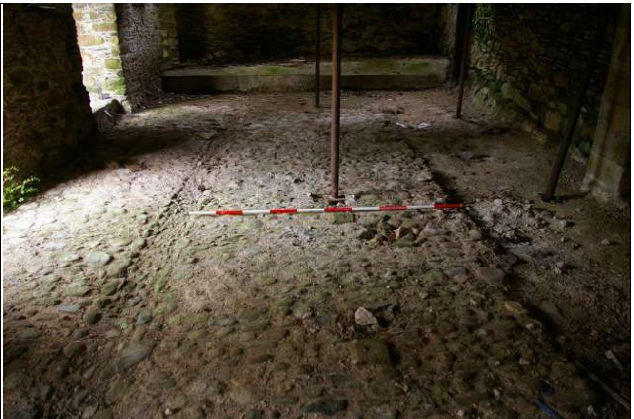
FIGURE 33: THE COBBLED FLOOR IN BARN B; FROM THE EAST (2M SCALE).
