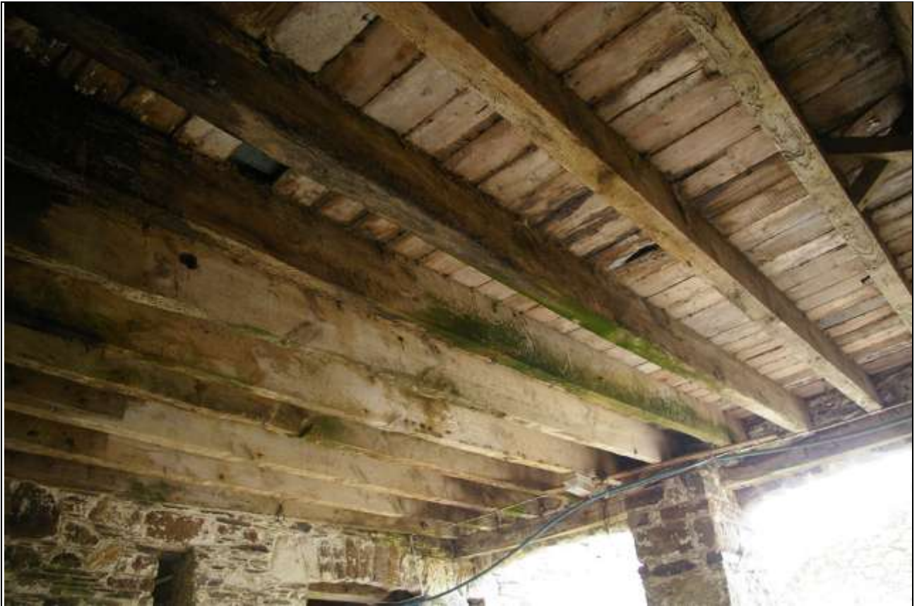
FIGURE 48: THE LOFT FLOOR IN BARN A, NORTH END; FROM THE WEST-SOUTH-WEST.
