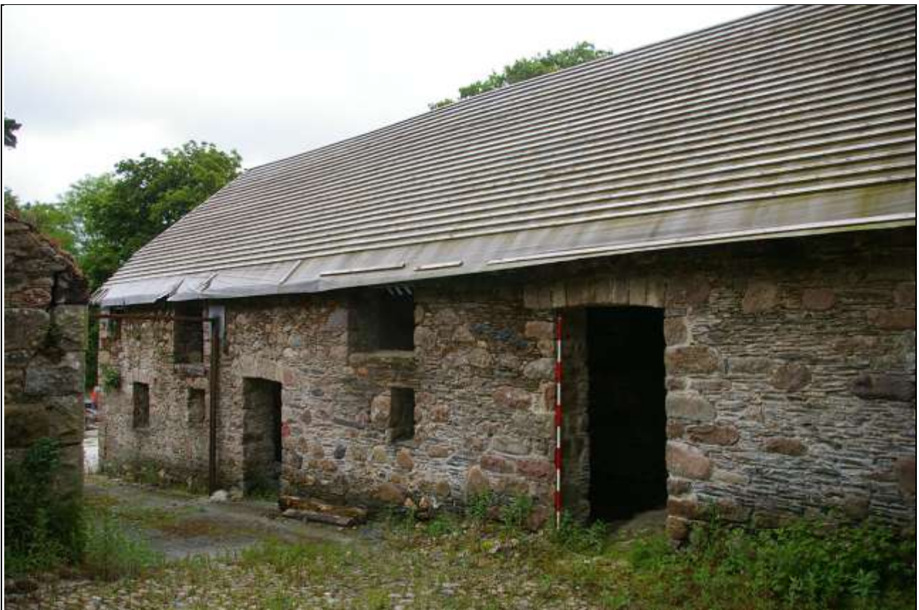
FIGURE 29: BARN C, NORTH ELEVATION; FROM THE NORTH-WEST (2M SCALE).
