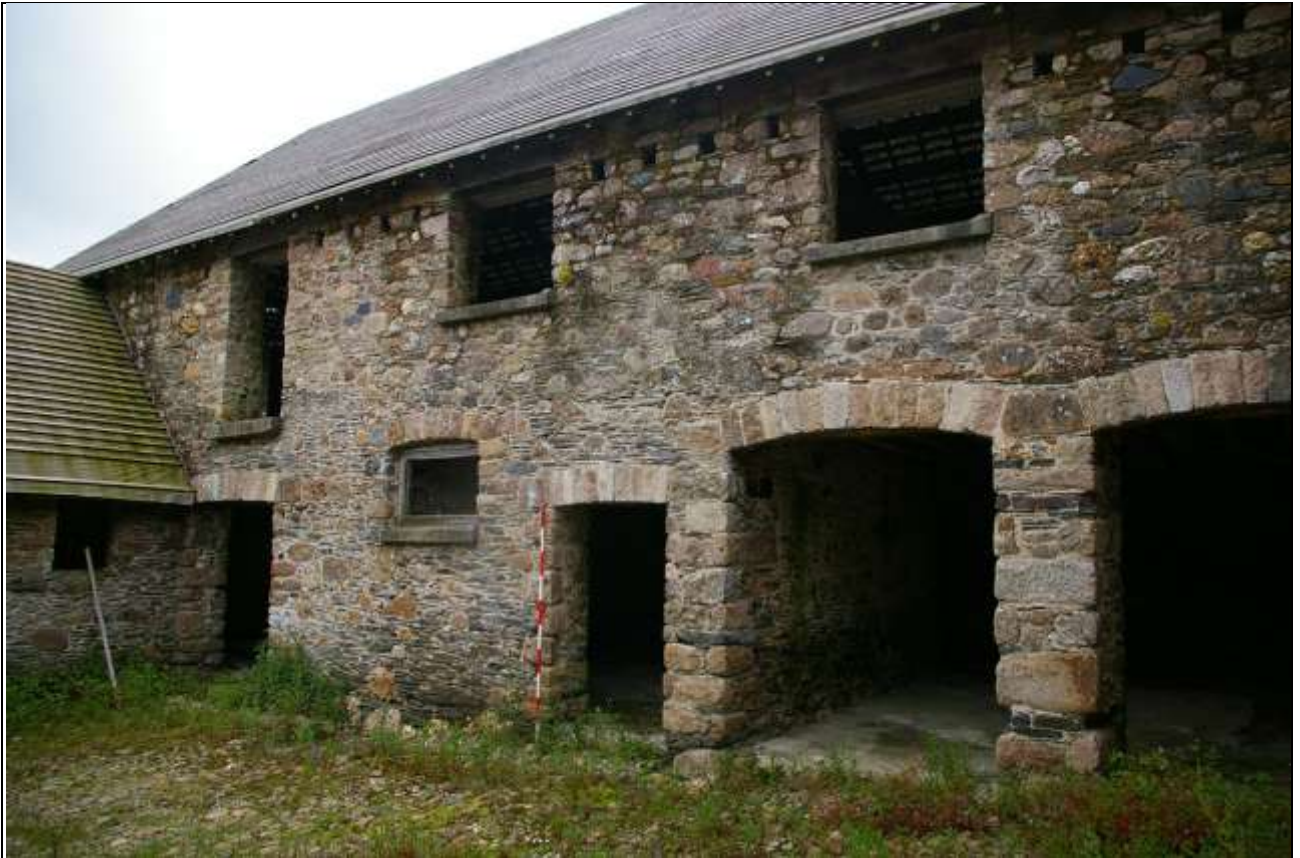
FIGURE 32: BARN A, EAST ELEVATION; FROM THE NORTH-EAST (2M SCALE).
