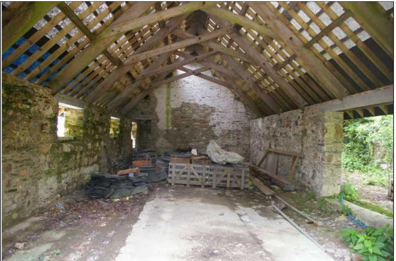
FIGURE 81: THE INTERIOR OF BARN D; FROM THE EAST.
