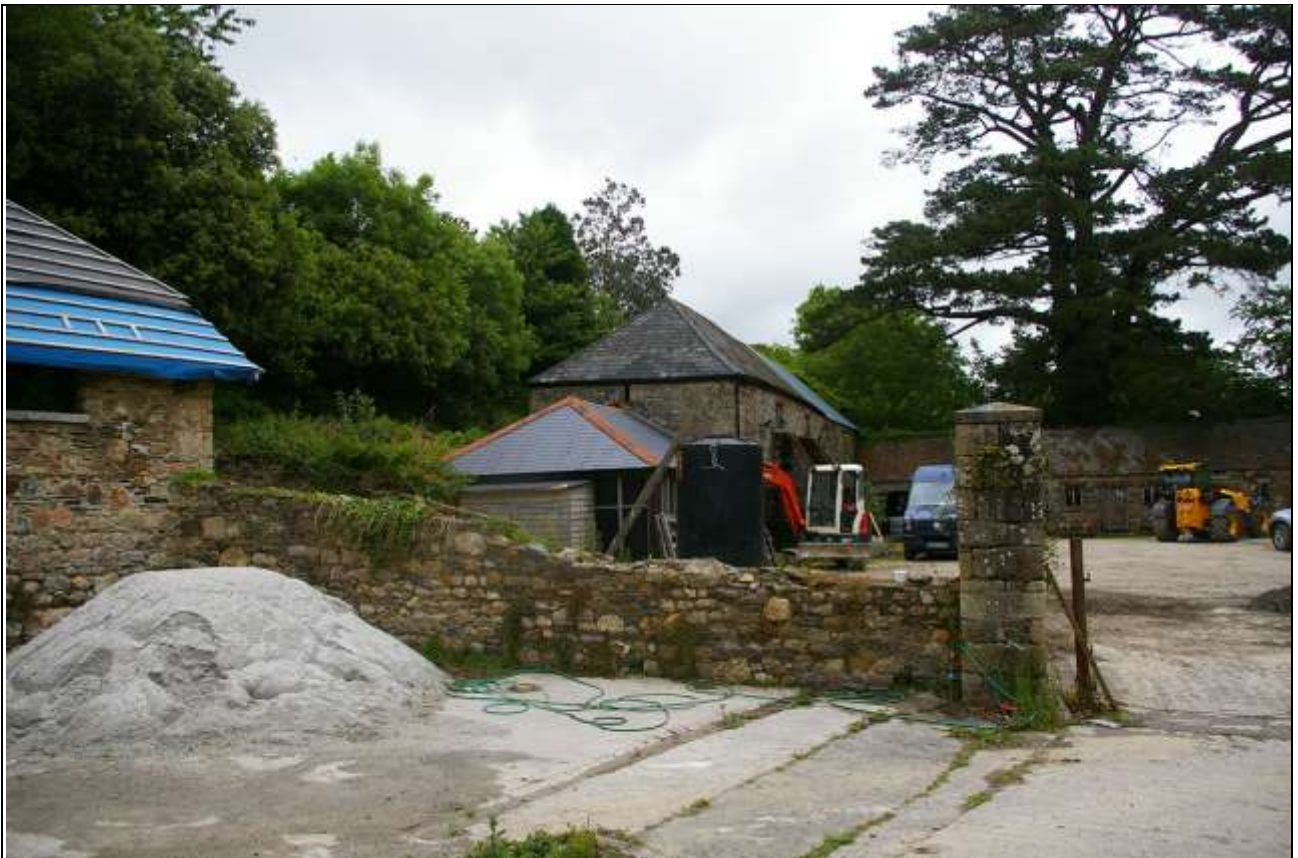
FIGURE 77: VIEW OUT OF THE COURTYARD, OVER THE BOUNDARY WALL, TO THE OTHER BLOCK OF BUILDINGS ACROSS THE DRIVEWAY; FROM THE WEST-SOUTH-WEST.
