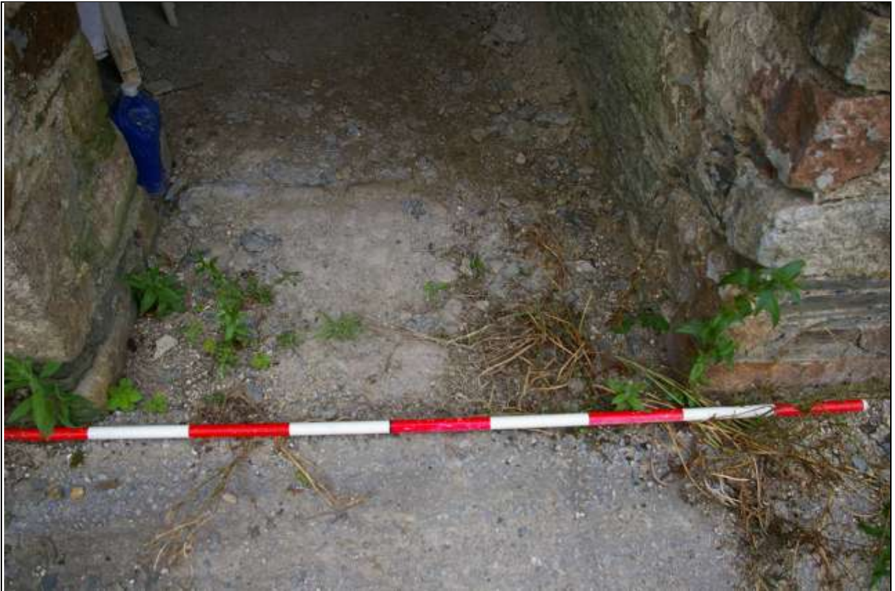
FIGURE 72: COBBLED THRESHOLD SURVIVES IN BARN C DOOR IN EAST ELEVATION; FROM THE EAST (2M SCALE).
