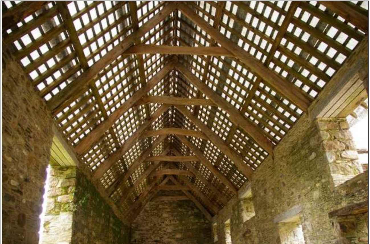
FIGURE 67: THE ROOF STRUCTURE IN BARN C; FROM THE EAST.
