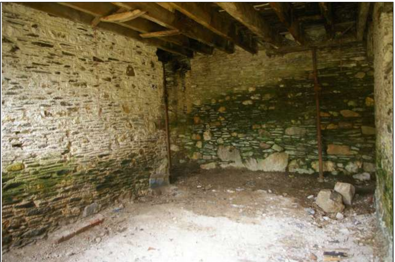
FIGURE 49: THE CENTRAL COMPARTMENT IN BARN A; FROM THE NORTH-EAST.
