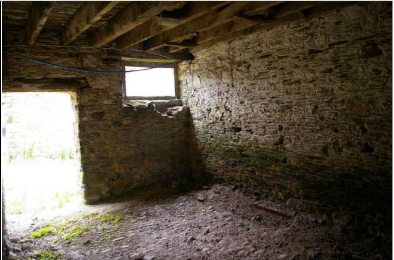
FIGURE 51: THE CENTRAL COMPARTMENT OF BARN A; FROM THE NORTH-WEST.
