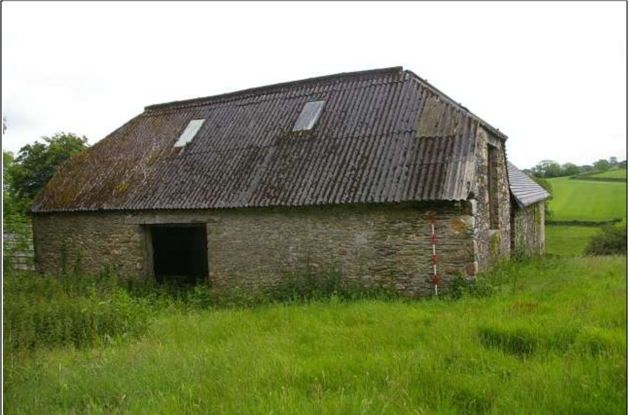
FIGURE 4: NORTH ELEVATION OF BARN B; FROM THE NORTH-WEST (2M SCALE).
