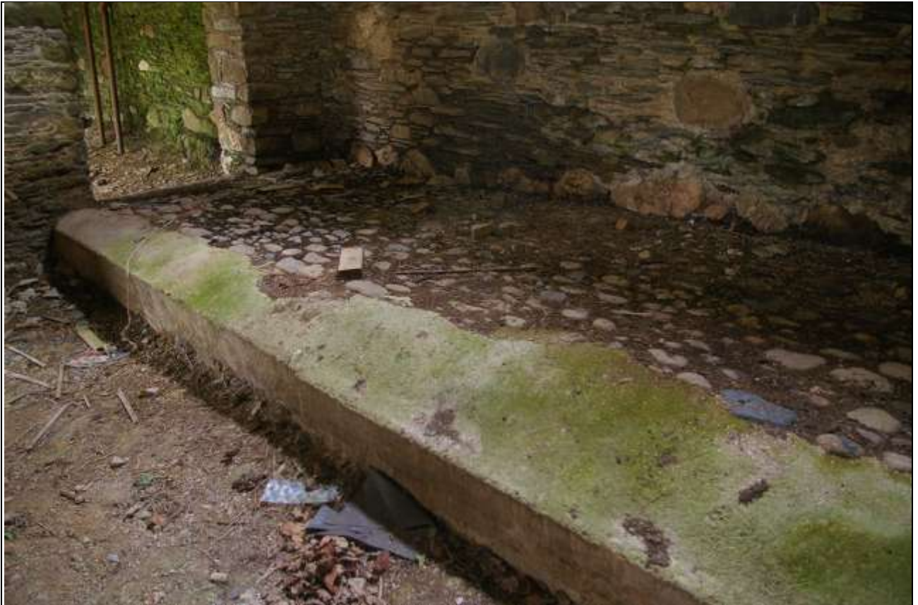
FIGURE 37: THE RAISED FLOOR TO THE WEST OF BARN B; FROM THE NORTH-NORTH-EAST.
