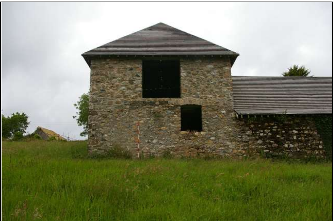
FIGURE 23: BARN A, SOUTH ELEVATION; FROM THE SOUTH (2M SCALE).
