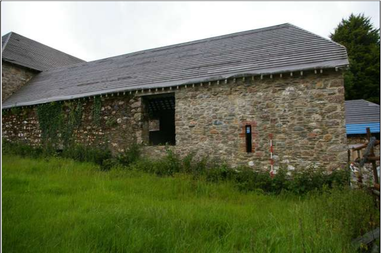
FIGURE 26: BARN C, SOUTH ELEVATION; FROM THE SOUTH-EAST (2M SCALE).
