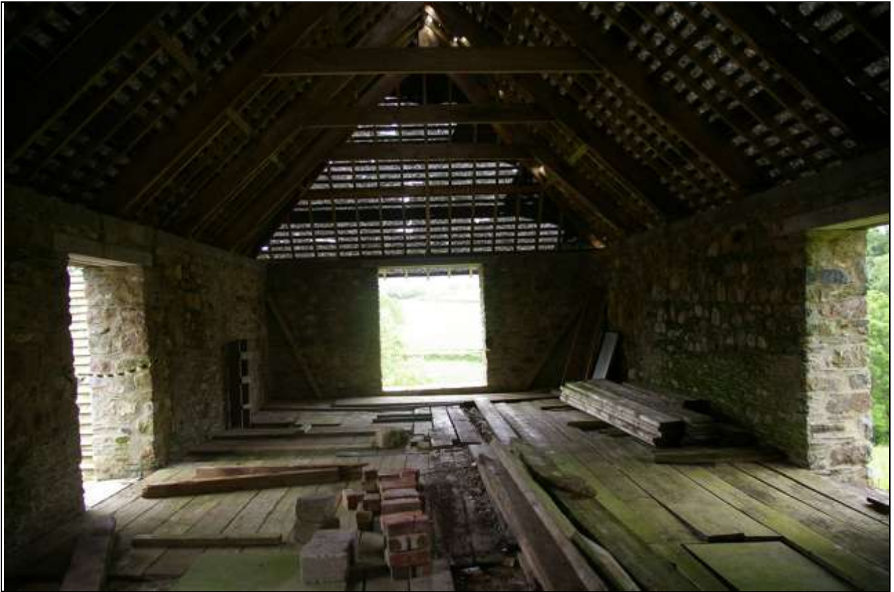
FIGURE 20: BARN A, INTERIOR OF LOFT; FROM THE NORTH.
