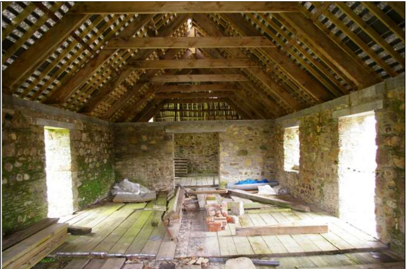
FIGURE 11: INTERIOR OF BARN A, LOFT; FROM THE SOUTH.
