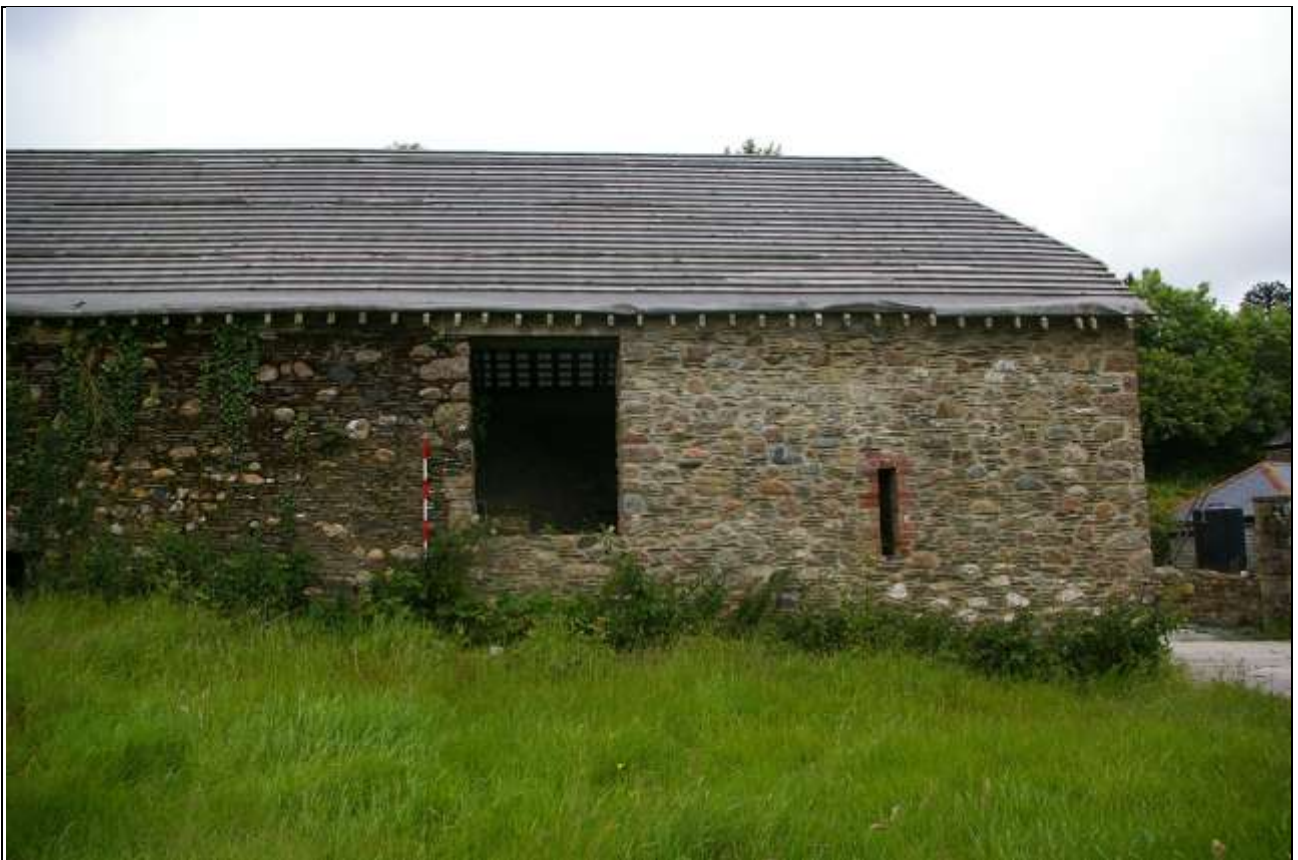
FIGURE 25: BARN C, SOUTH ELEVATION; FROM THE SOUTH (2M SCALE).
