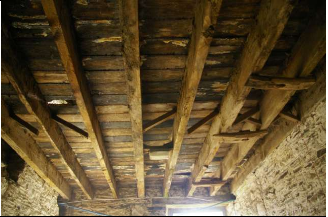
FIGURE 52: THE LOFT FLOOR IN BARN A, CENTRAL SECTION; FROM THE WEST.
