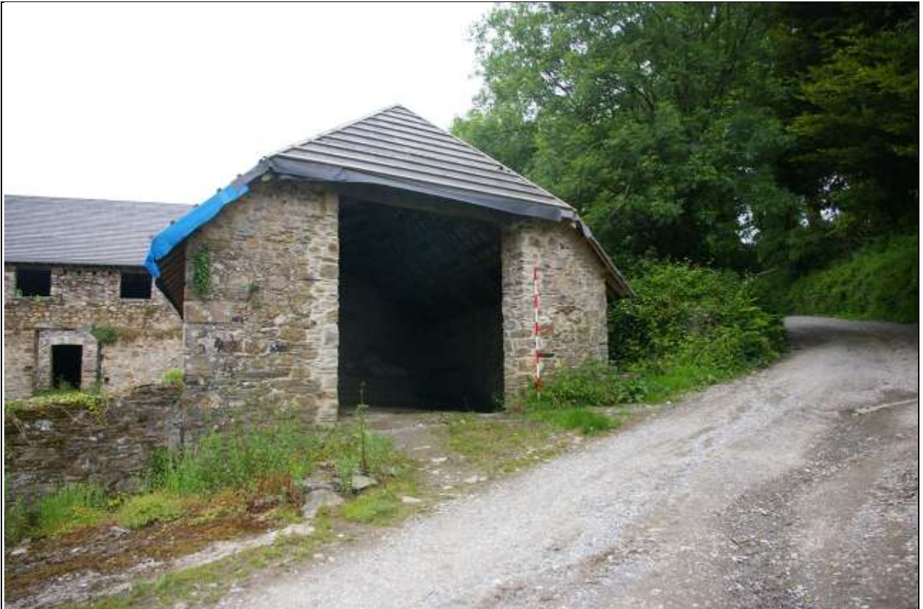
FIGURE 79: THE EAST ELEVATION OF BARN D, SHOWING THE ENLARGED OR WHOLLY FORCED OPENING; FROM THE EAST-SOUTH-EAST (2M SCALE).
