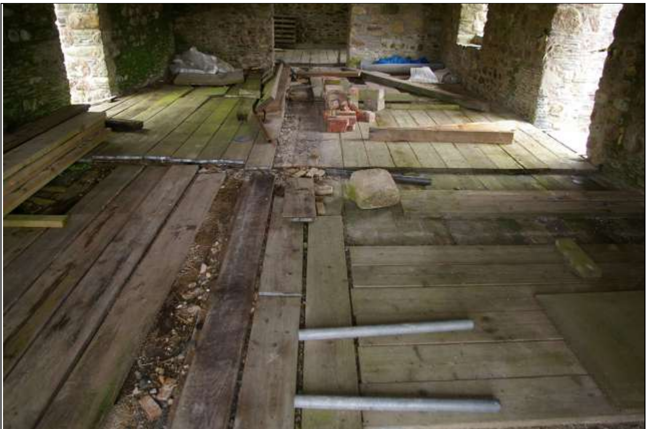
FIGURE 13: LOFT FLOOR, BARN A; FROM THE SOUTH.
