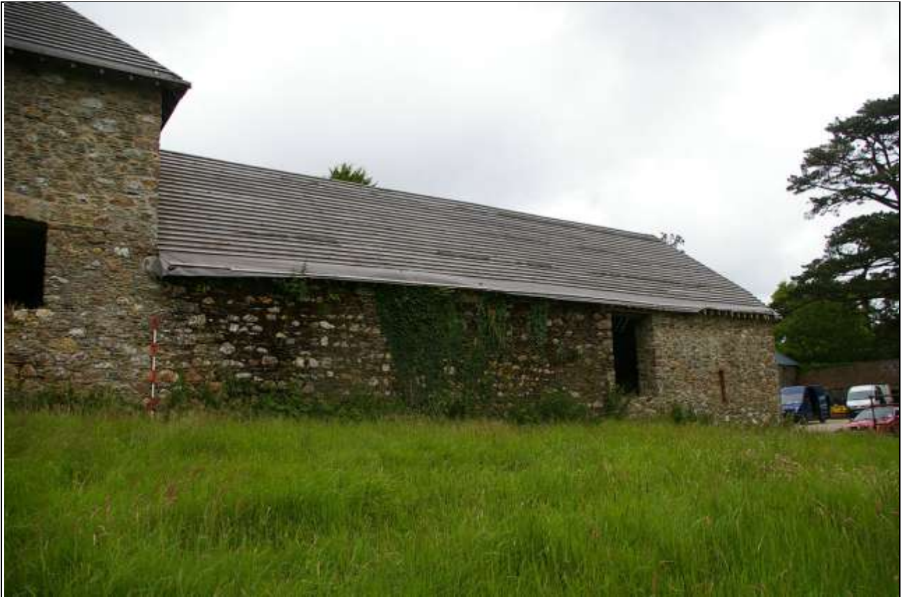
FIGURE 24: BARN A, SOUTH ELEVATION; FROM THE SOUTH (2M SCALE).
