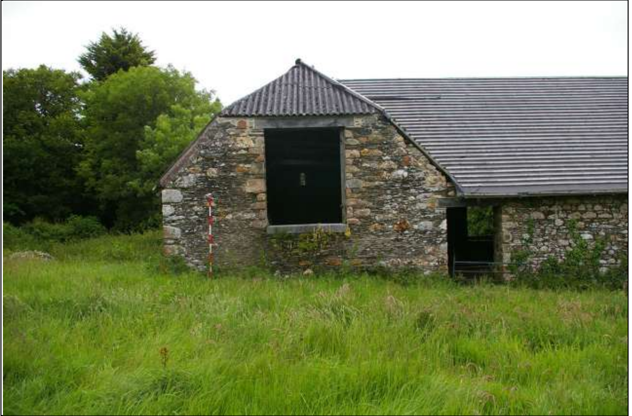
FIGURE 6: WEST ELEVATION OF BARN B; FROM THE WEST (2M SCALE).
