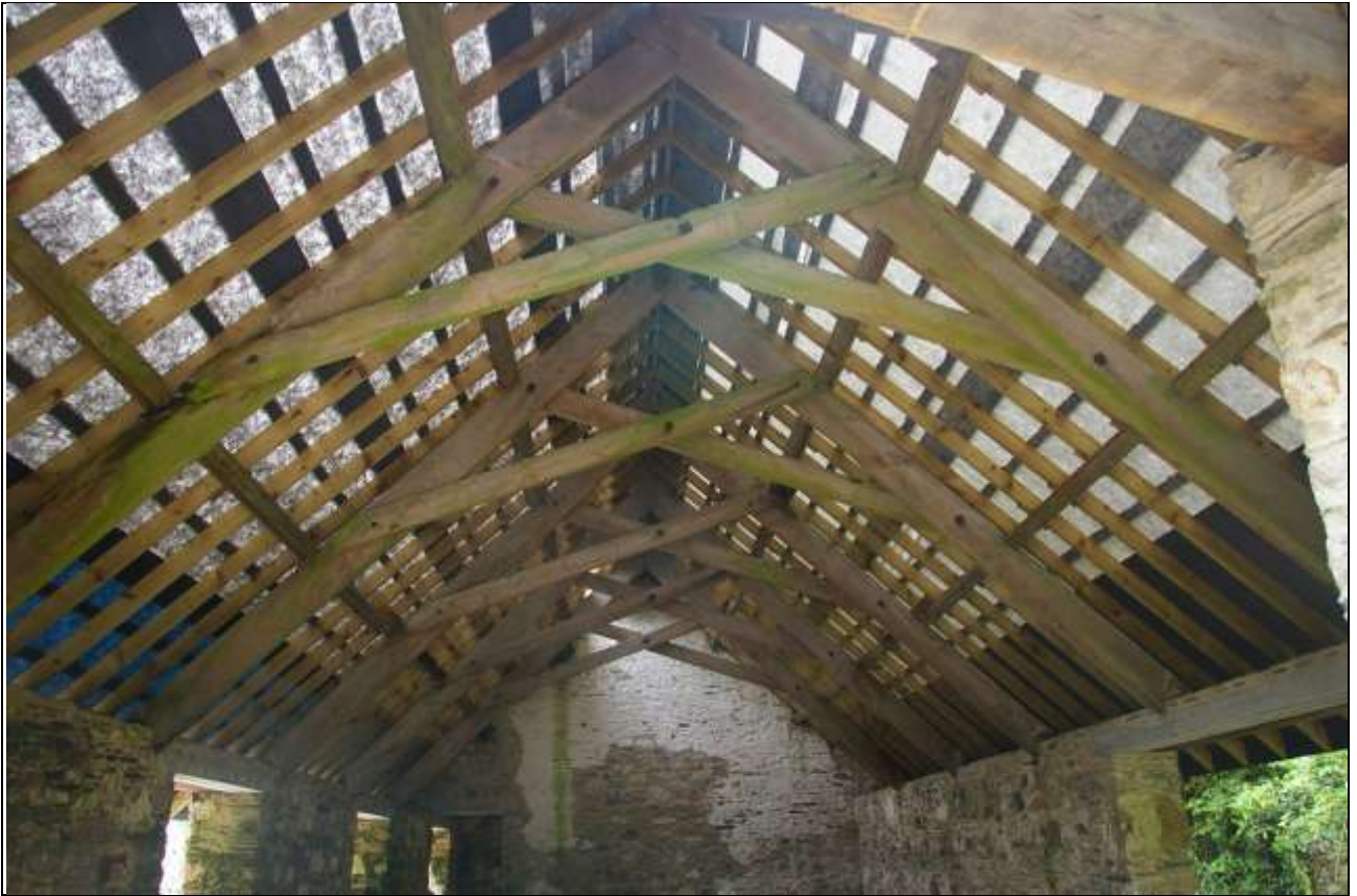
FIGURE 80: THE SCISSOR TRUSS ROOF IN BARN D; FROM THE EAST.
