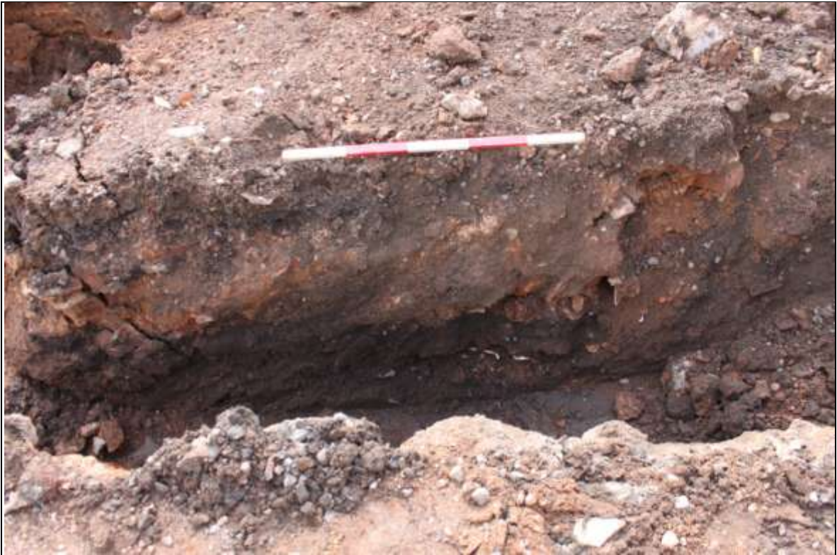
HOUSE PLOT 1, MID FOUNDATION TRENCH, NORTH-EAST FACING SECTION OF SERVICE TRENCH [111]; VIEWED FROM THE NORTH-WEST (1M SCALE).
