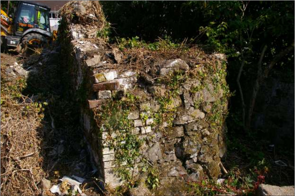
B2: the curving block of masonry that supports the stair on the east side of B2; viewed from the south.
