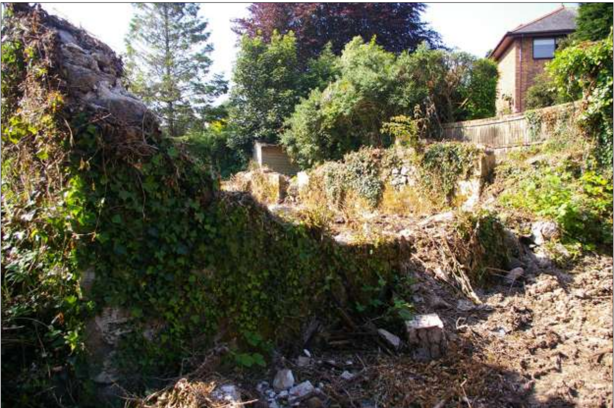
B2: the north wall of B2; viewed from the north-east.
