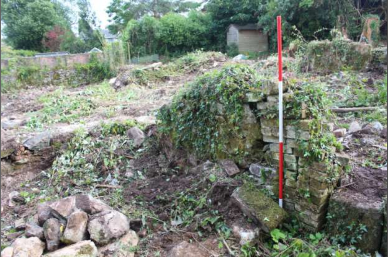
B3: the east wall of B2 where it forms the wall of B3; viewed from the north-east (scale 2m).
