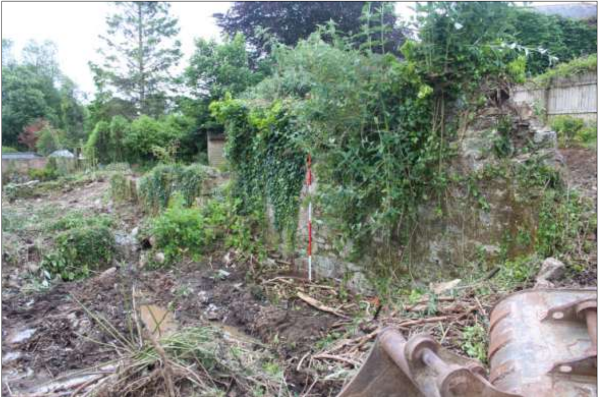
FIGURE 6: THE SURVIVING WEST WALL OF B1; VIEWED FROM THE NORTH.
