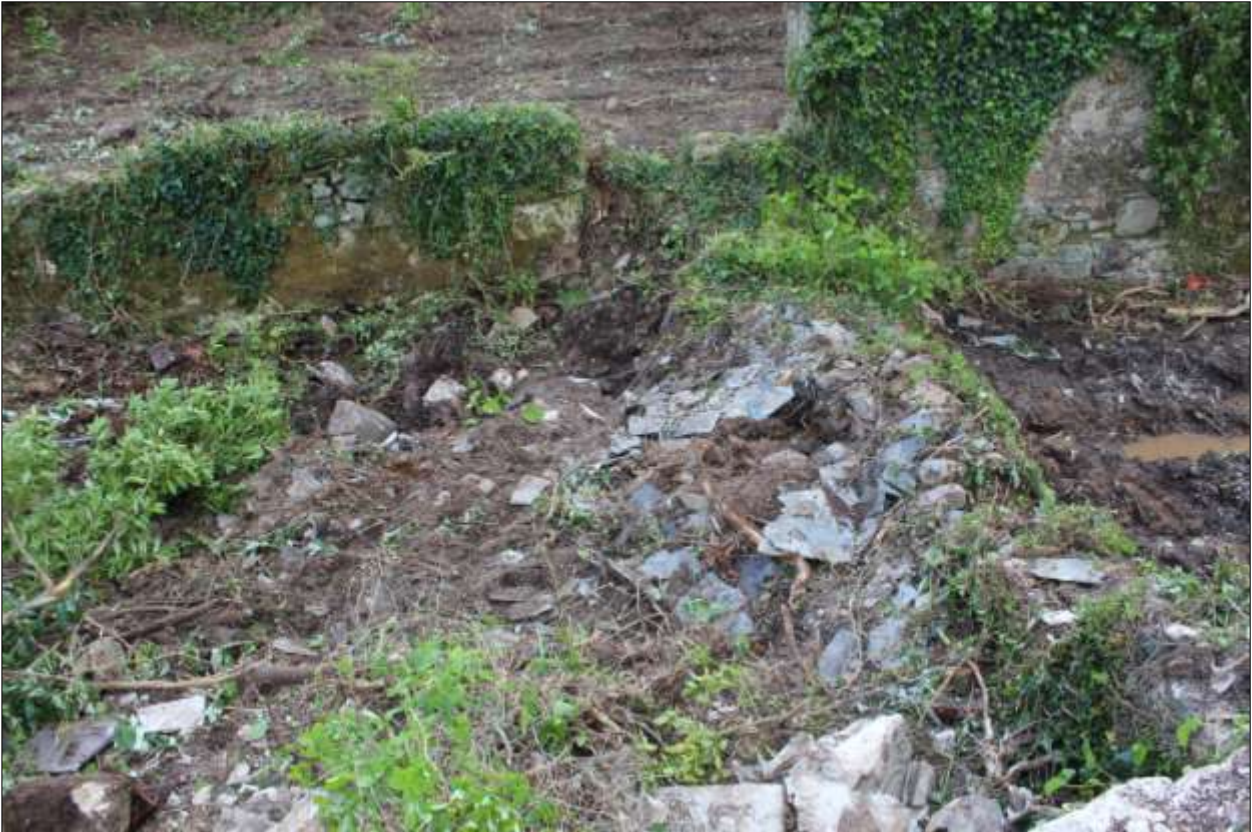
B2: the interior of B2, showing the dump of roof slate; viewed from the east.
