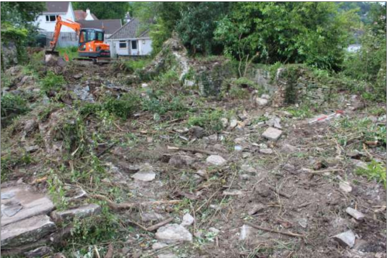
B2: The interior of B2; viewed from the south-west (scale 2m).
