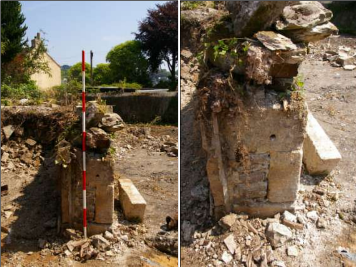
B4: The east side of the western doorway in the south wall of B4, showing the width and profile of the wall, pindle holes, and scar for doorframe; viewed from the west (scale 2m).
