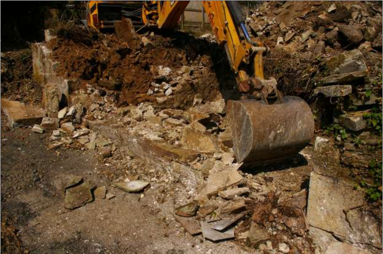
B4: the demolition of the south wall; viewed from the south-east.
