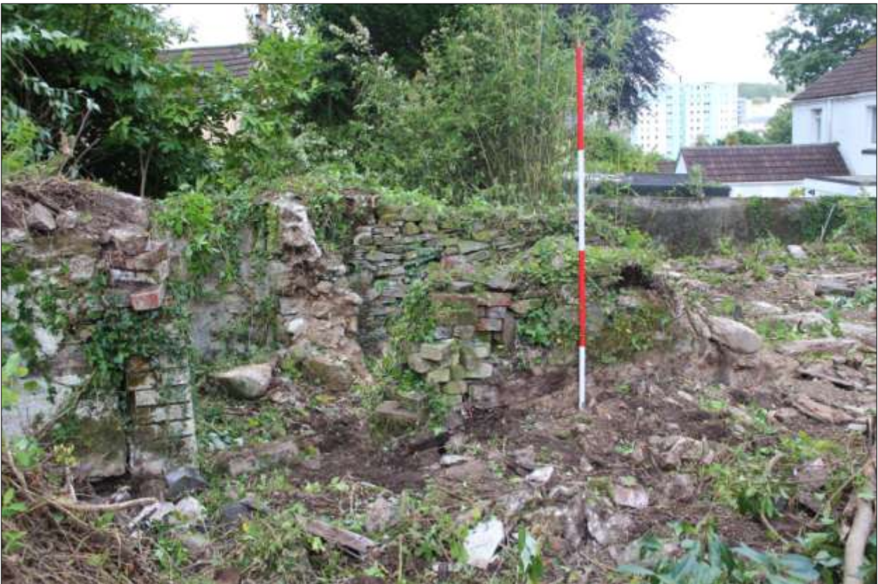
B2: the east wall of B2; viewed from the north-west (scale 2m).
