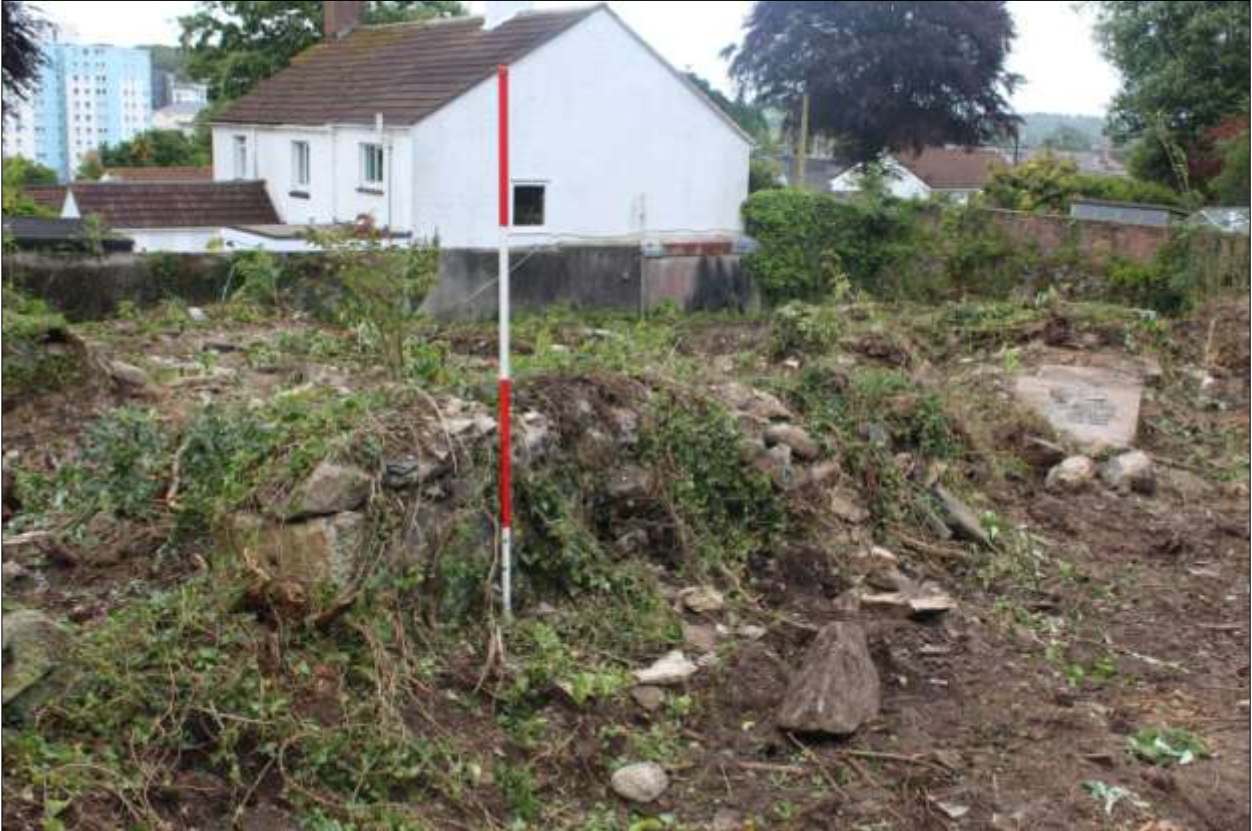
B2: The west wall of B2; viewed from the north (scale 2m).
