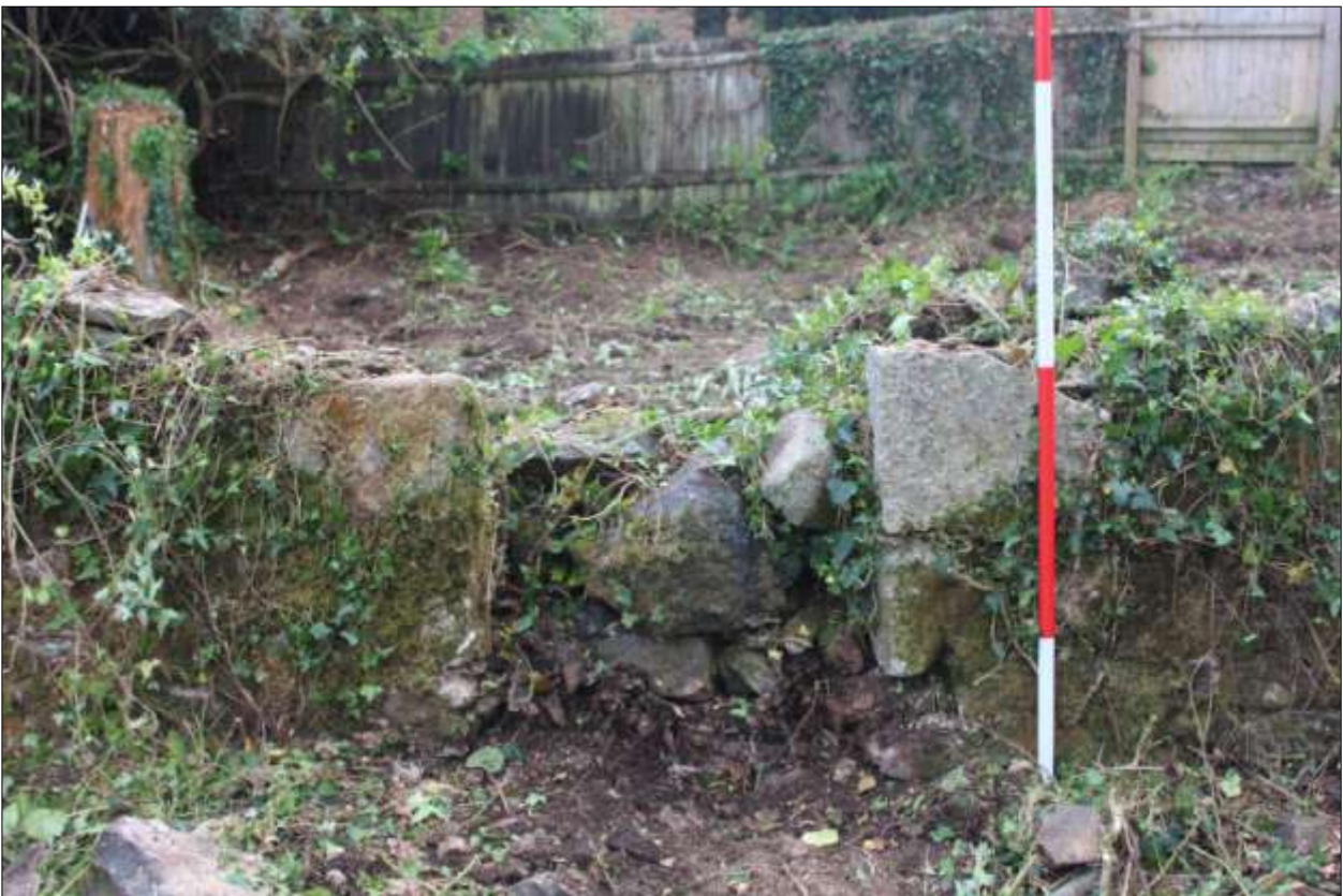
B2: the blocked door at the southern end of the west wall; viewed from the east (scale 2m).
