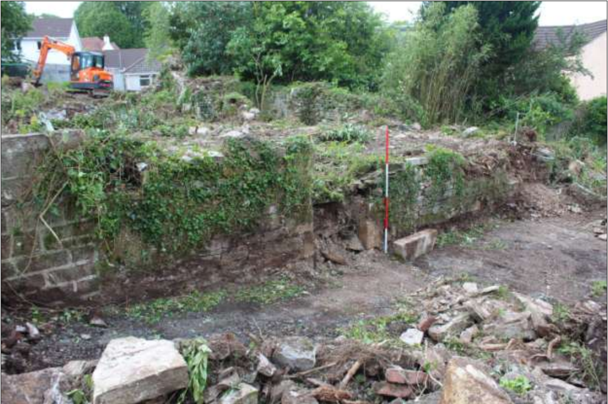
B4: the south wall of B4; viewed from the south-west (scale 2m).
