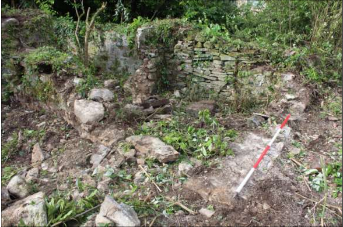
FIGURE 9: B3, VIEWED FROM THE SOUTH-WEST (SCALE 2M).
