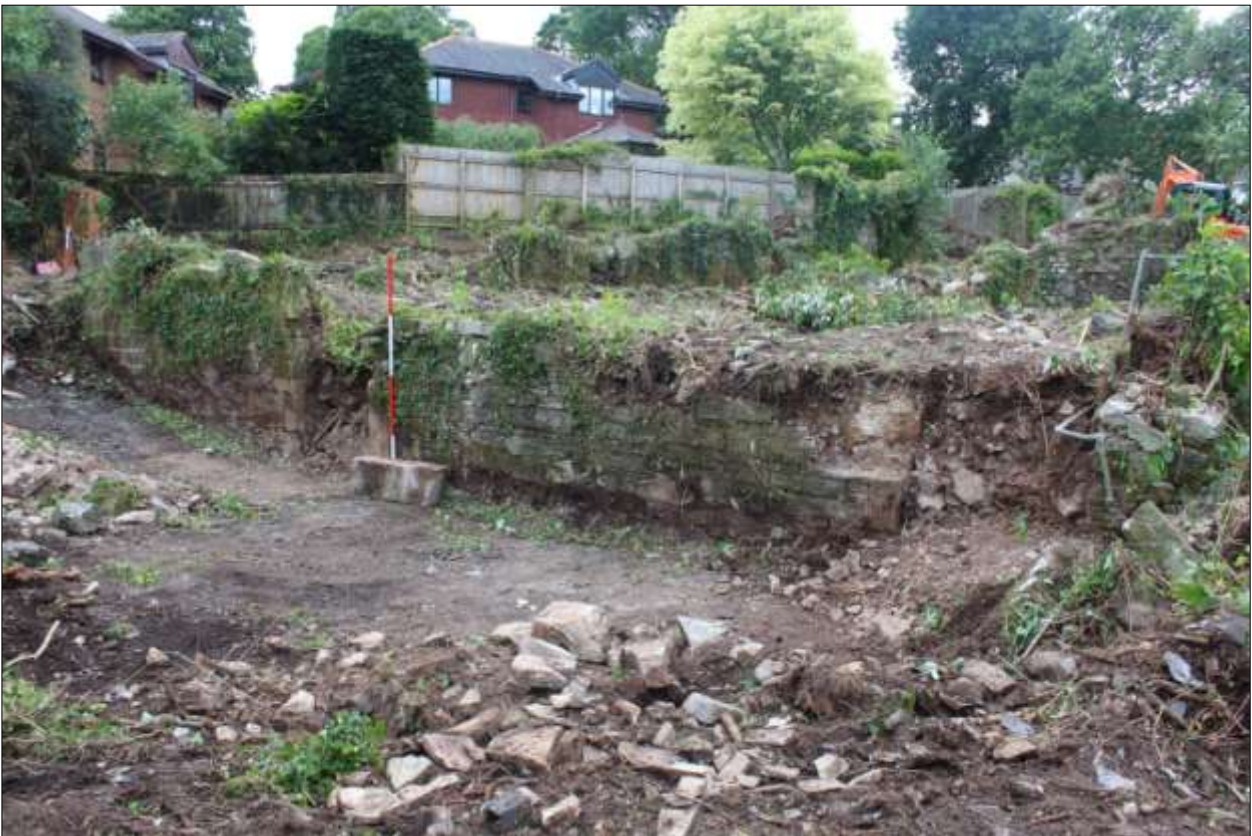
B4: the south wall of B4; viewed from the south-east (scale 2m).
