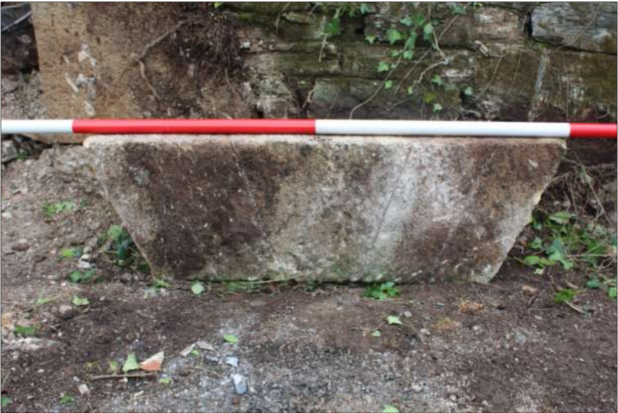
B4: detail of the granite lintel scored to imitate individual voussoirs (scale 2m).
