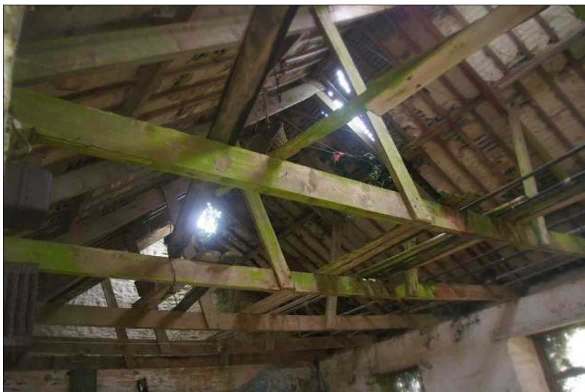
FIGURE 20: B1 ROOF STRUCTURE; VIEWED FROM THE NORTH-NORTH-WEST.
