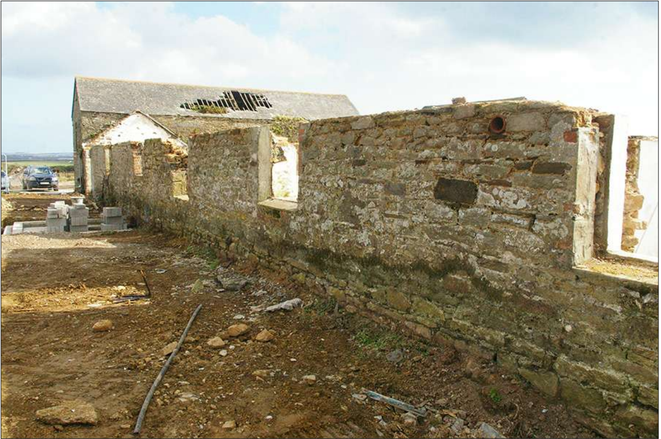
B3, NORTH-EAST ELEVATION; VIEWED FROM THE NORTH.
