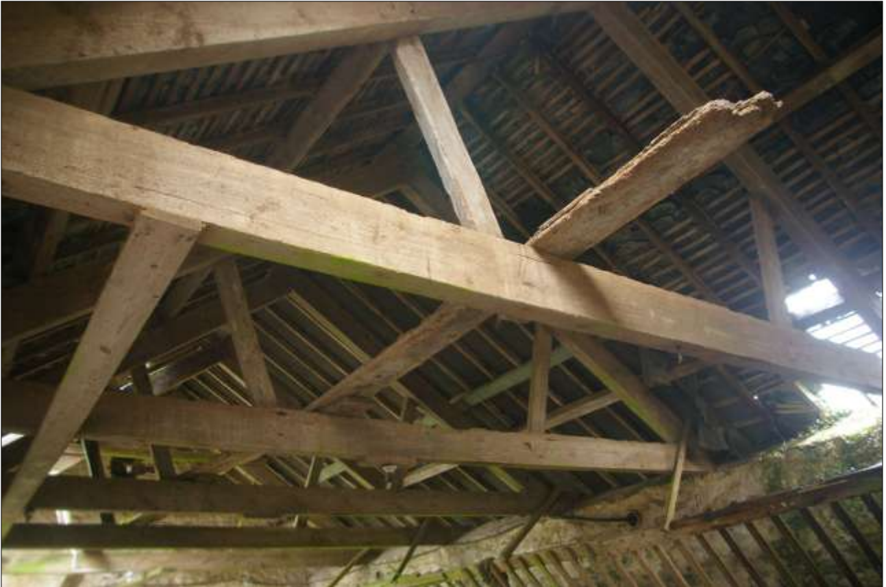
B4.2, SOUTH ROOM, ROOF STRUCTURE; VIEWED FROM THE NORTH-EAST.
