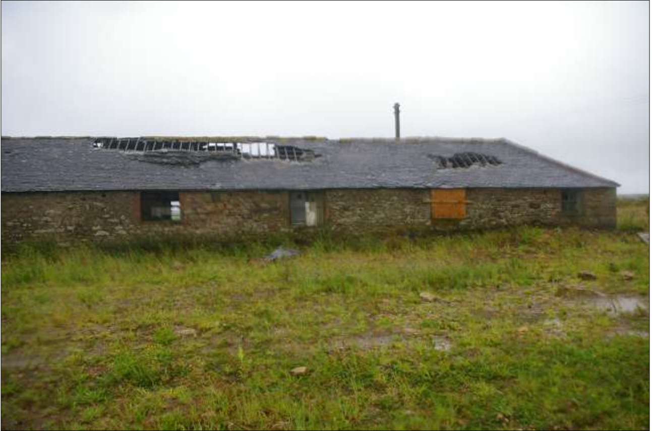
B3, NORTH-EAST ELEVATION; VIEWED FROM THE NORTH-EAST.
