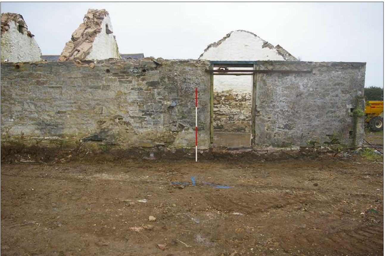
THE NORTH-WEST ELEVATION OF B5; VIEWED FROM THE NORTH-WEST (SCALE 2M).
