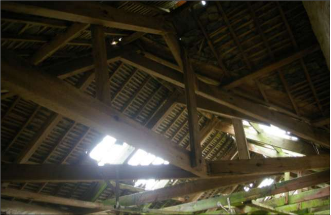
B3.2, ROOF STRUCTURE AT THE NORTHERN CORNER; VIEWED FROM THE WEST-SOUTH-WEST.
