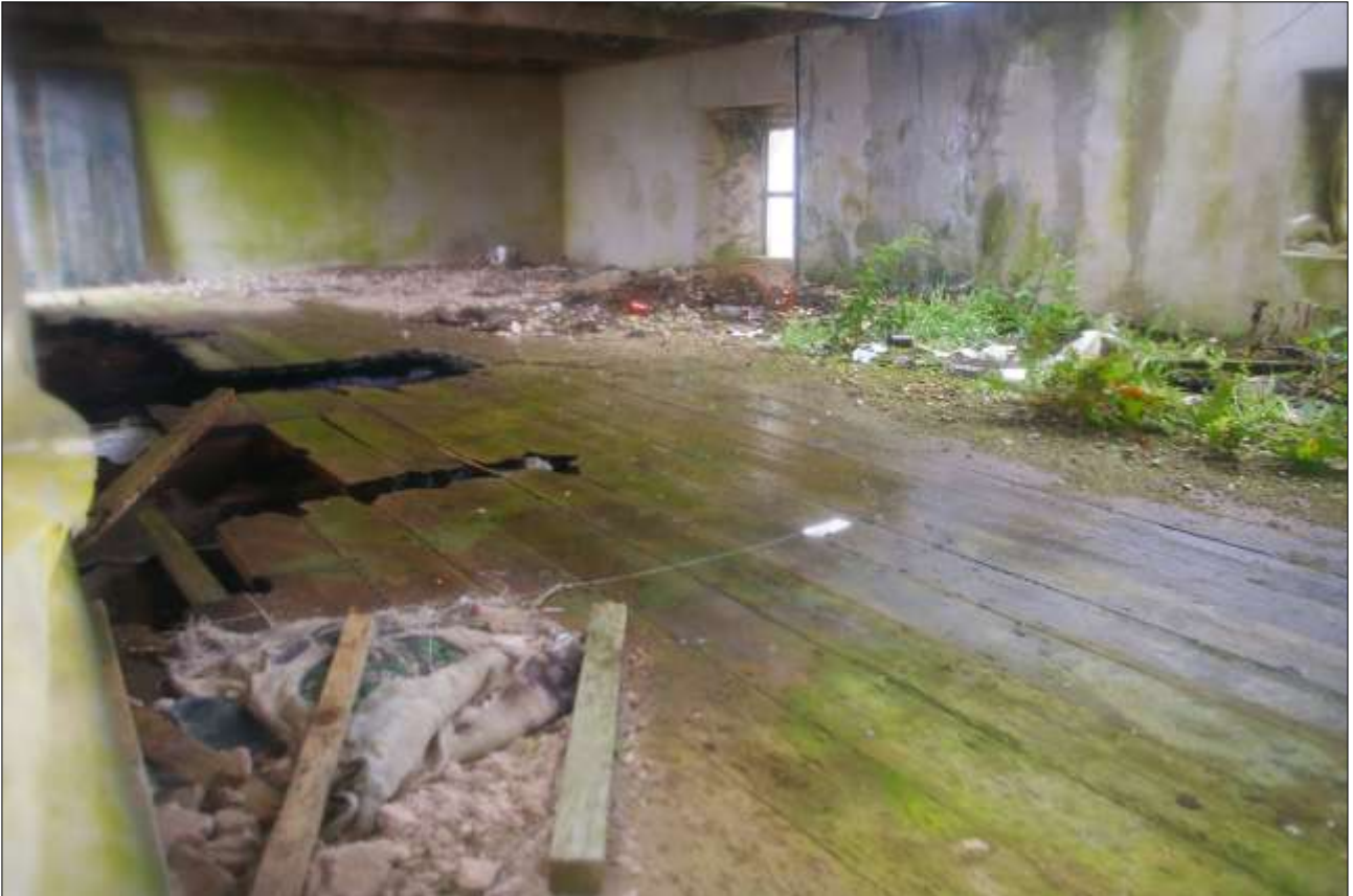
B2.3, FF ROOM, SHOWING THE 20 TH CENTURY BOARDED FLOOR; VIEWED FROM THE EAST.
