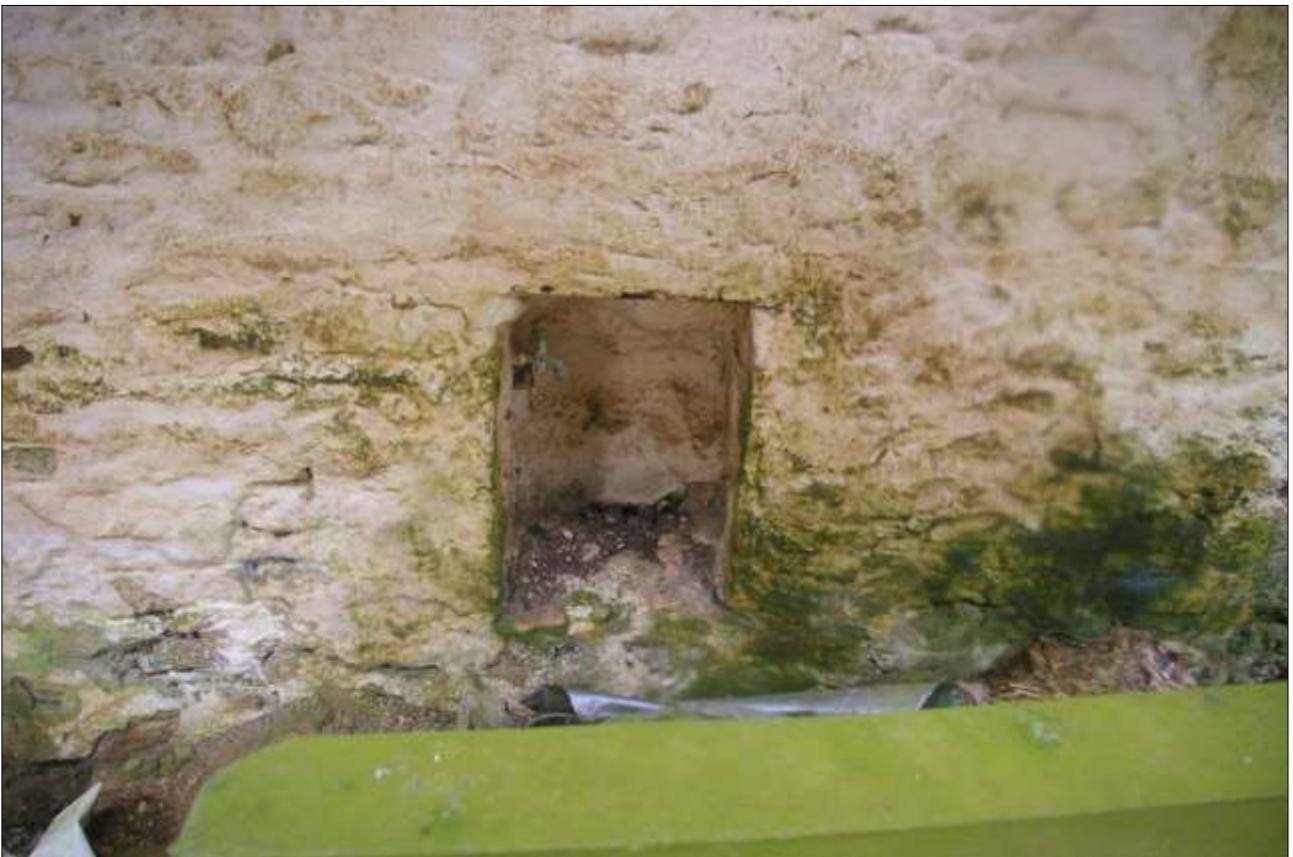
B3.2, WESTERN ROOM, A SMALL FORCED OPENING IN THE NORTH-EAST WALL WITH TAP FOR FLUSHING OUT THE TROUGHS; VIEWED FROM THE SOUTH-EAST.
