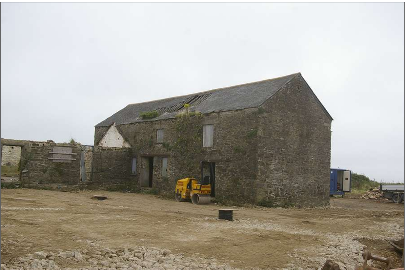
B2, DURING THE WORKS; VIEWED FROM THE SOUTH-WEST.
