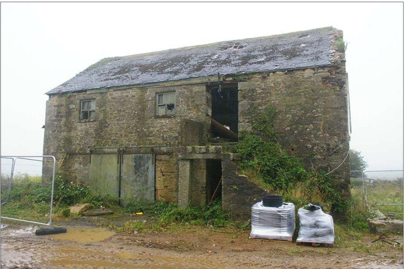
B1, NORTH-EAST ELEVATION; VIEWED FROM THE NORTH.
