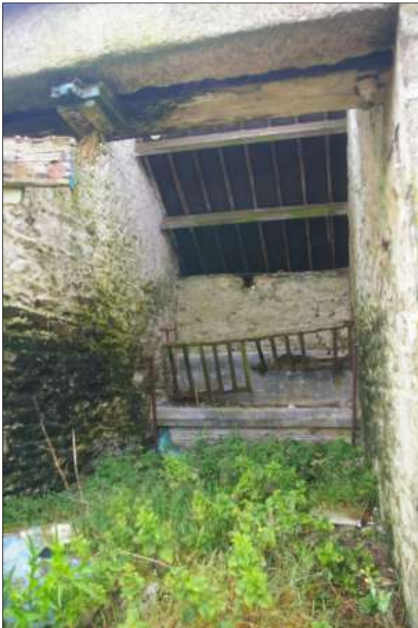
B5.1, NORTH ROOM; VIEWED FROM THE EAST-NORTH-EAST.
