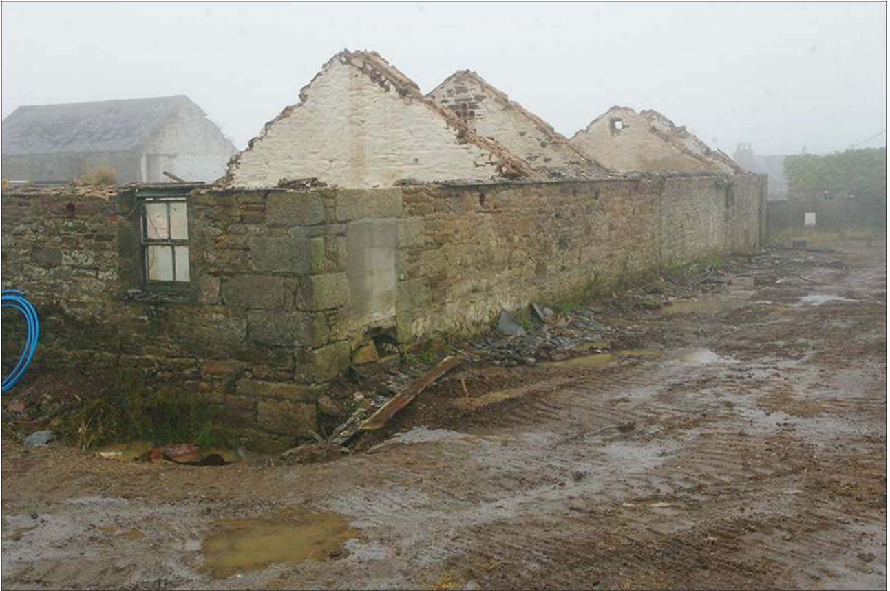
B4, DURING WORKS; VIEWED FROM THE WEST-NORTH-WEST.
