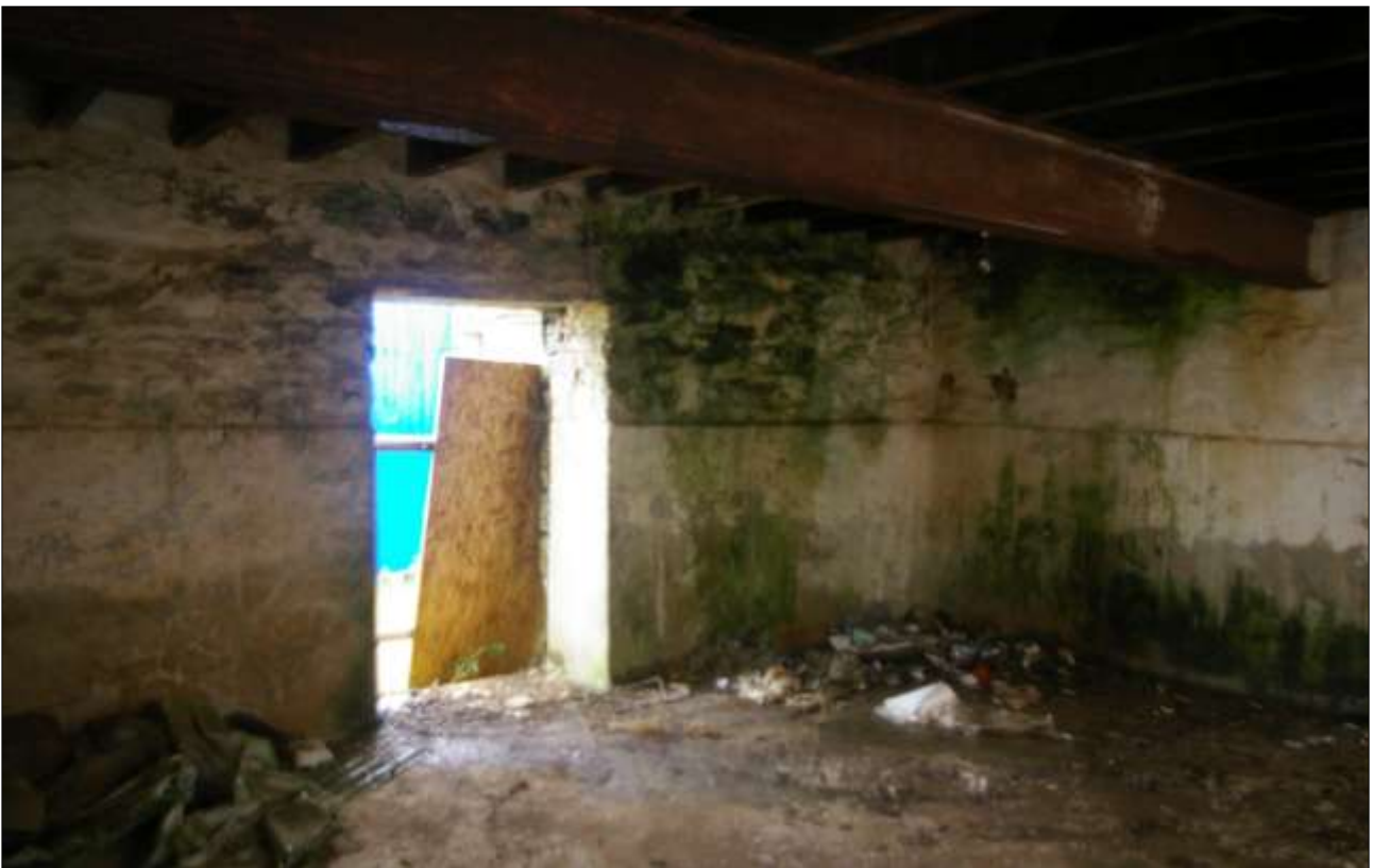
B2.1, SOUTHERN GF ROOM (D6); VIEWED FROM THE SOUTH, LOOKING NORTH.
