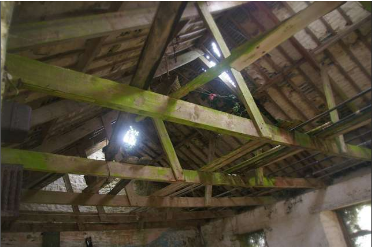
B1.3 ROOF STRUCTURE; VIEWED FROM THE NORTH-NORTH-WEST.
