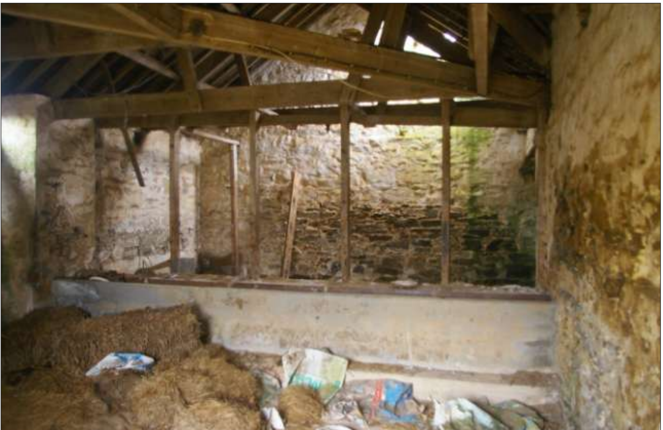
B5.2, SOUTH-WEST ROOM; VIEWED FROM THE SOUTH-WEST.
