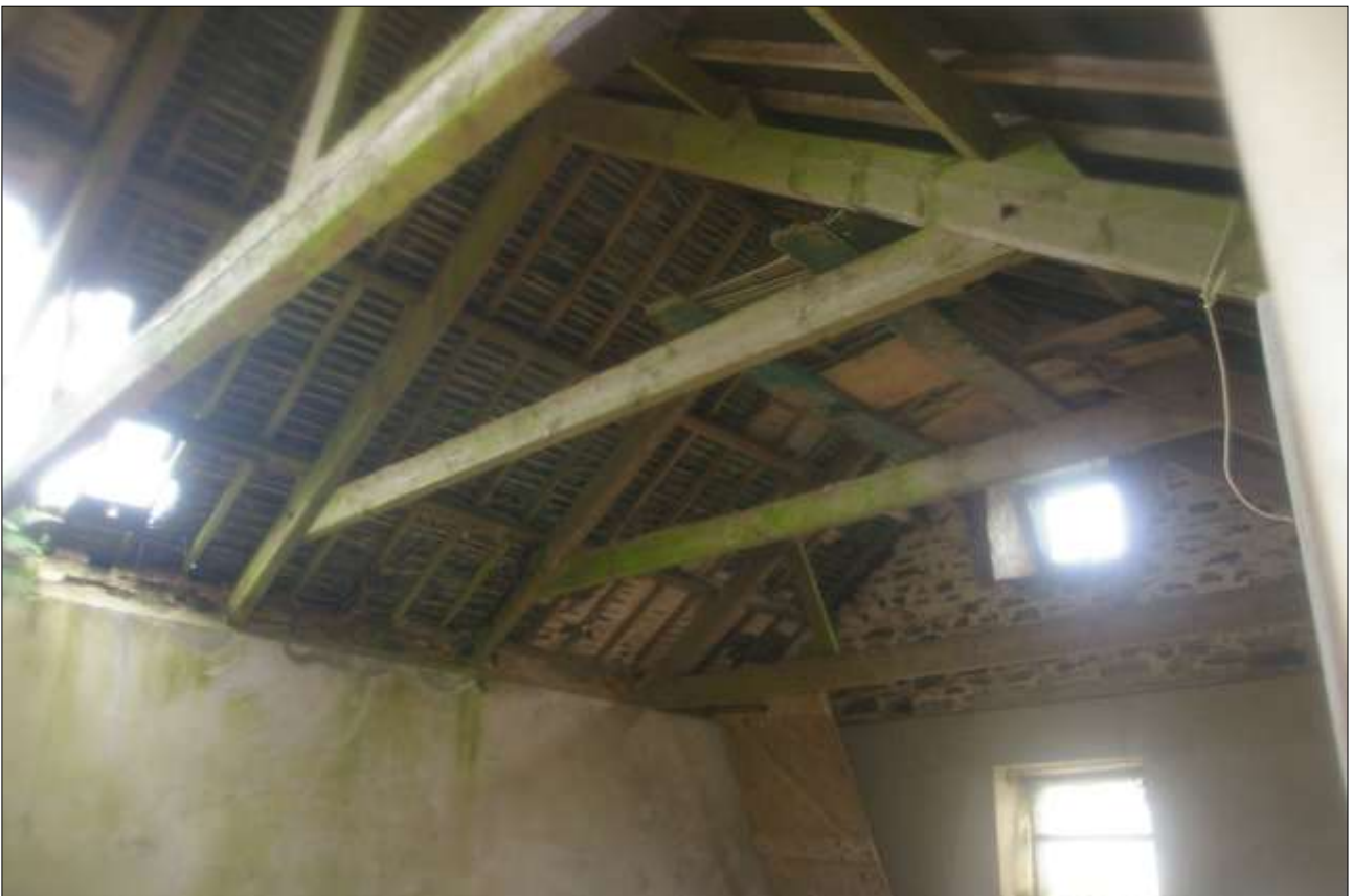
B2.3 ROOF STRUCTURE; VIEWED FROM THE SOUTH.
