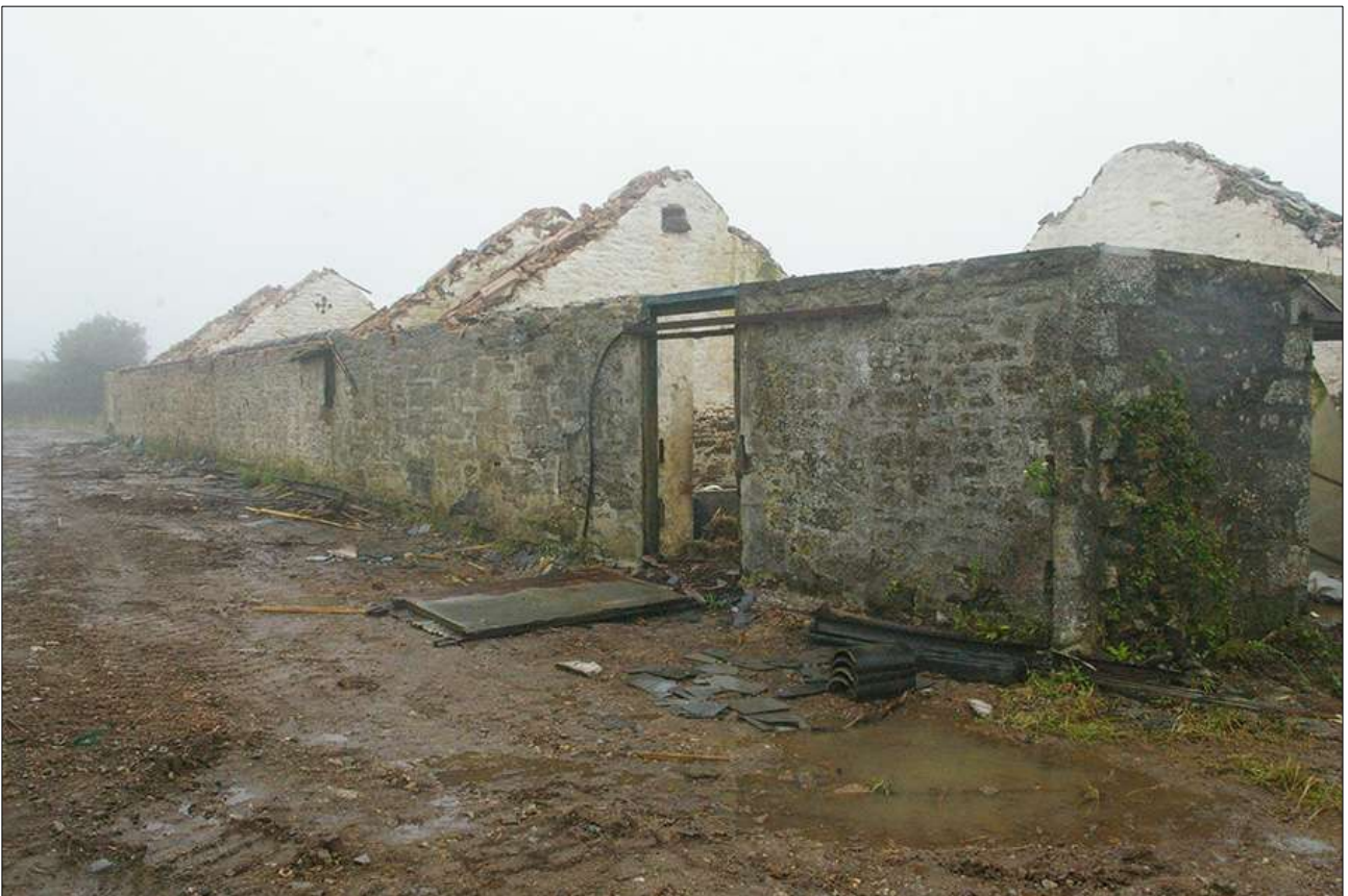
B5, NORTH-WEST ELEVATION, DURING WORKS; VIEWED FROM THE WEST.
