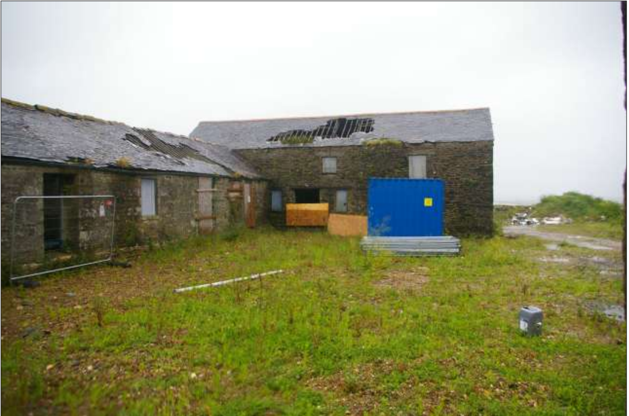
B2, FROM ACROSS THE CENTRAL YARD; VIEWED FROM THE WEST.
