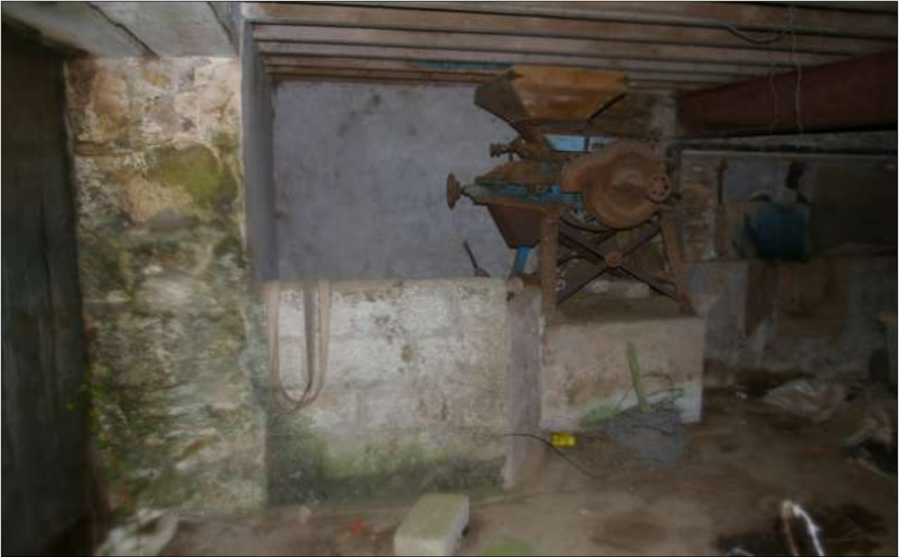
B1.1, EASTERN GF ROOM, SHOWING THE IN SITU MACHINERY (S2), AS VIEWED FROM THE DOORWAY (D3) INTO THE WEST ROOM; VIEWED FROM THE NORTH-WEST.
