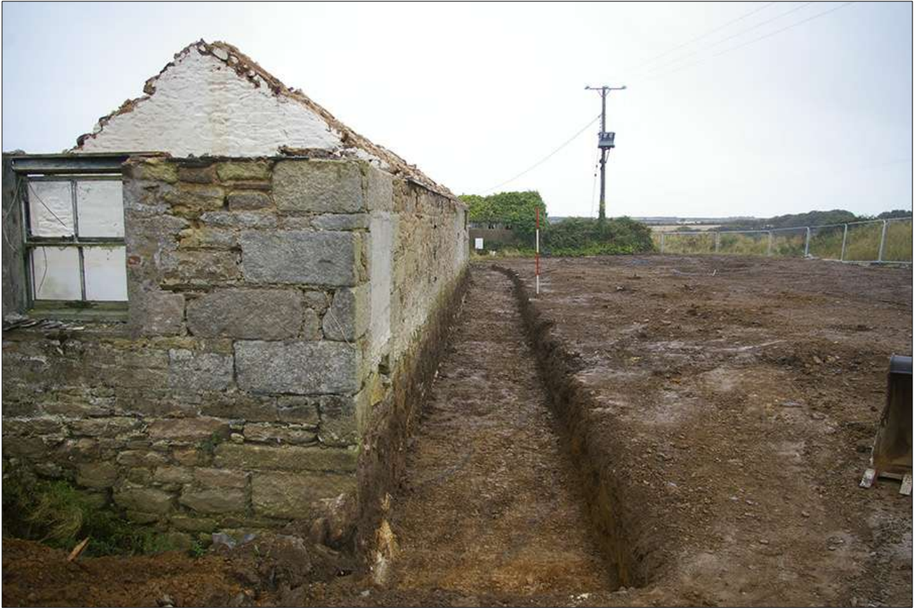
AREA EXCAVATED ALONG THE NORTH-WEST SIDE OF B4 AND B5; VIEWED FROM THE NORTH-EAST (SCALE 2M).
