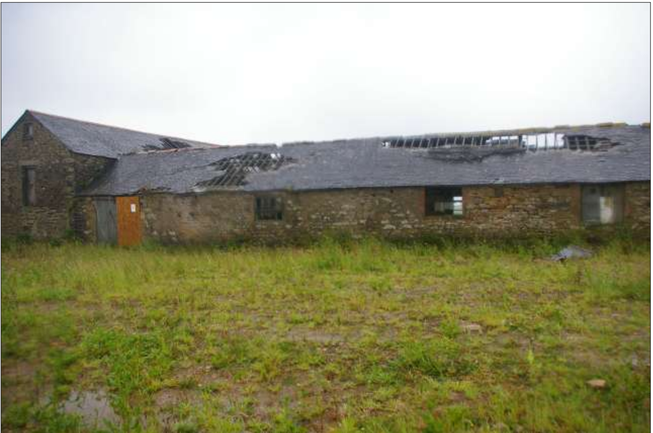
B3, NORTH-EAST ELEVATION, SHOWING THE CHANGE OF BUILD BETWEEN THE FIRST AND SECOND WINDOW FROM THE LEFT; VIEWED FROM THE NORTH-NORTH-EAST.
