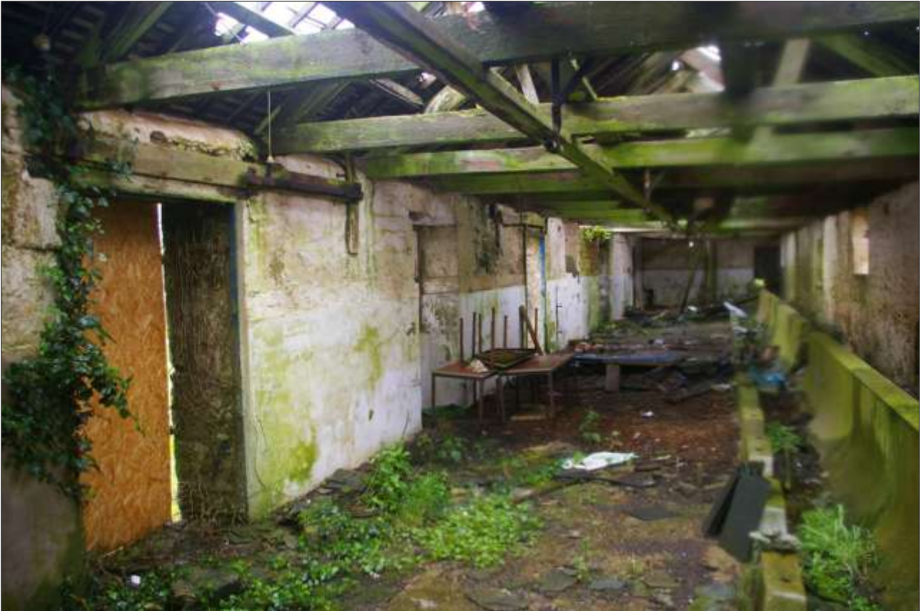
B3.2, WESTERN ROOM, VIEWED FROM THE NORTH-EAST CORNER.
