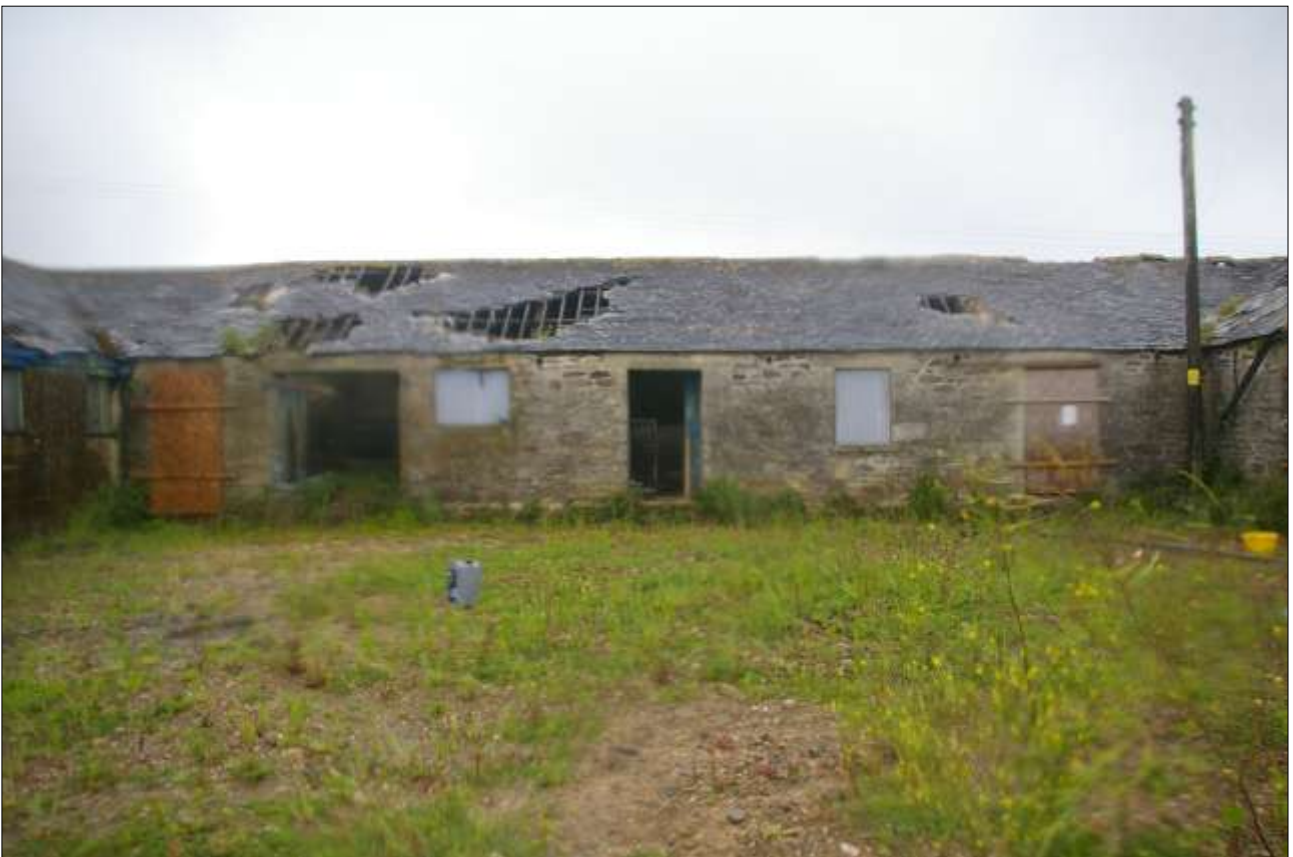
B4 (RIGHT) AND B5 (LEFT); VIEWED FROM THE SOUTH-EAST.
