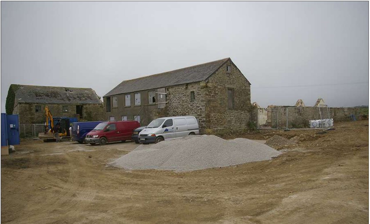
PENBRO FARM, DURING WORKS; VIEWED FROM THE NORTH-EAST.
