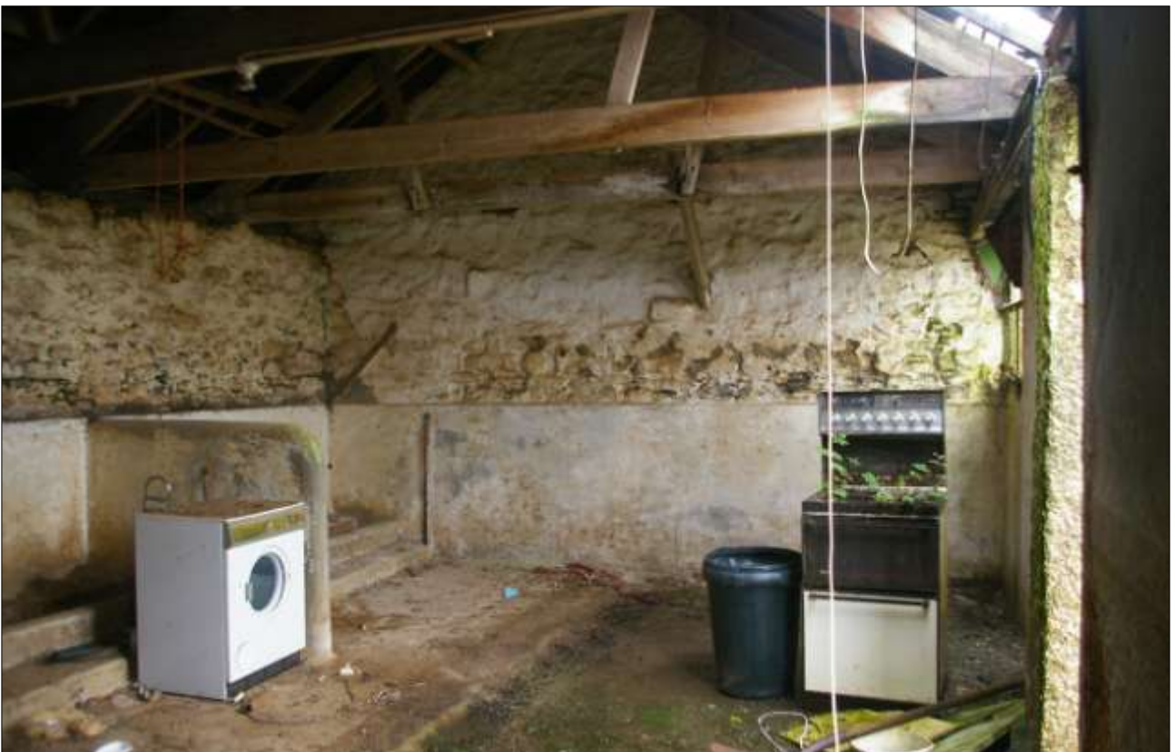
B5.3, EAST ROOM; VIEWED FROM THE EAST-SOUTH-EAST.
