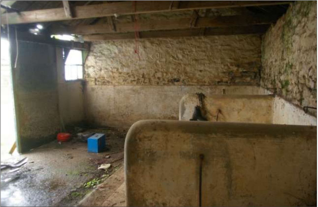
B5.3, EAST ROOM; VIEWED FROM THE WEST-SOUTH-WEST.
