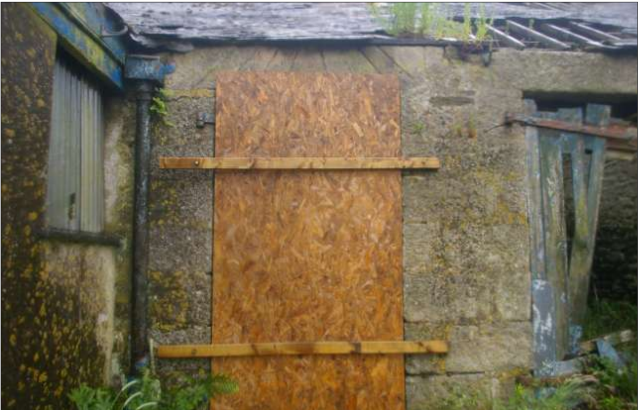
B5, SOUTH-EAST YARD ELEVATION, DOORWAY (D21) INTO THE SOUTH-WEST ROOM WITH INCISED UPSIDE-DOWN LINTEL; VIEWED FROM THE EAST-SOUTH-EAST.
