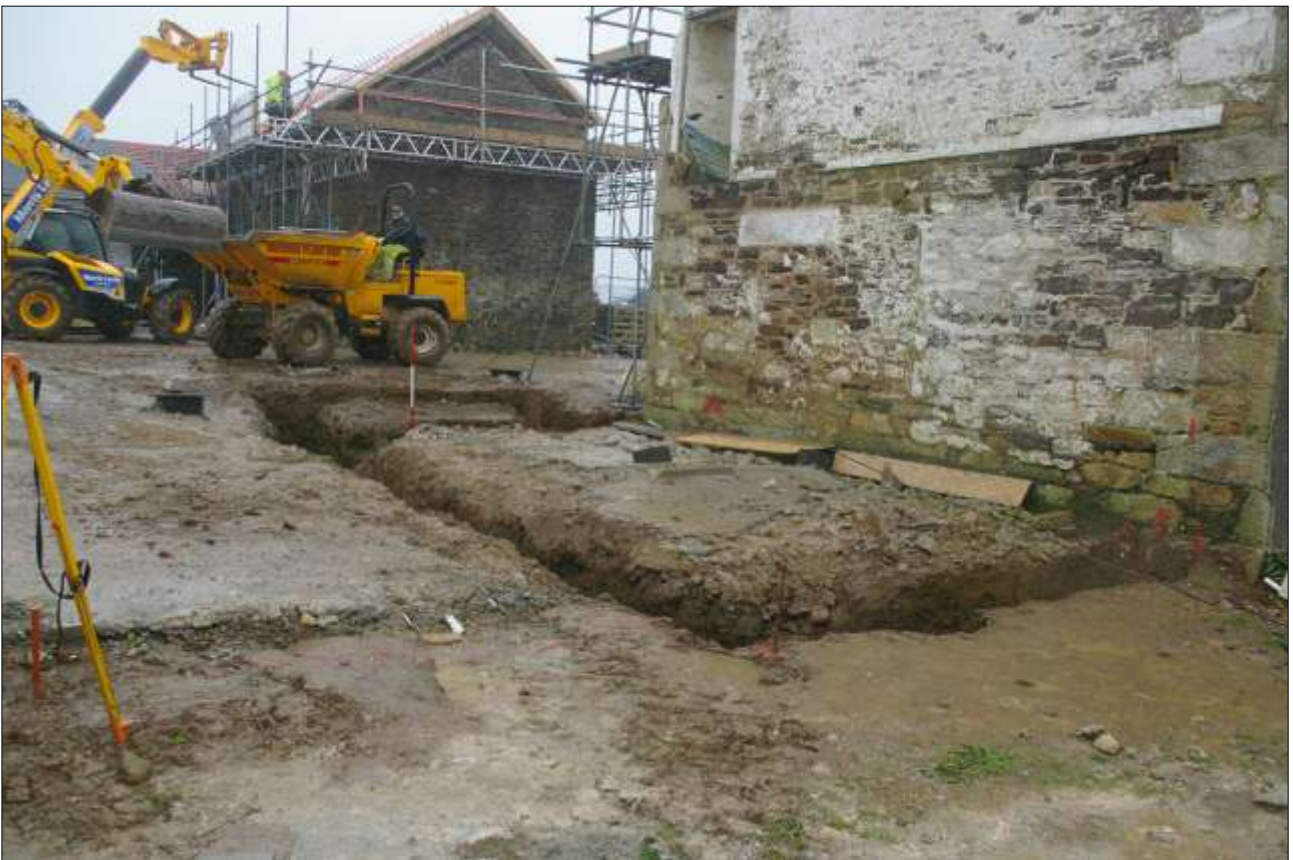
FOUNDATION TRENCH WEST OF B1; VIEWED FROM THE SOUTH-WEST (SCALE 2M).
