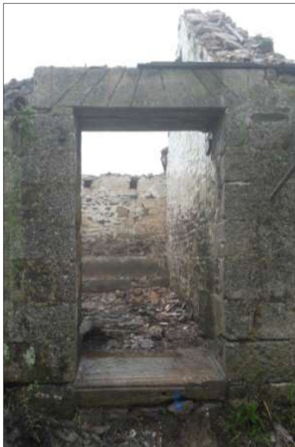
RIGHT: B5, DURING WORKS, DOORWAY (D21) INTO THE SOUTH-WEST ROOM FROM THE YARD, SHOWING INCISED LINTEL AND MOULDED GRANITE FIRE-SURROUND REUSED AS A THRESHOLD; VIEWED FROM THE SOUTH-EAST.
