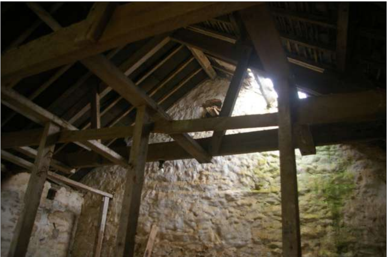
B5.2, SOUTH-WEST ROOM, ROOF STRUCTURE; VIEWED FROM THE SOUTH-SOUTH-WEST.
