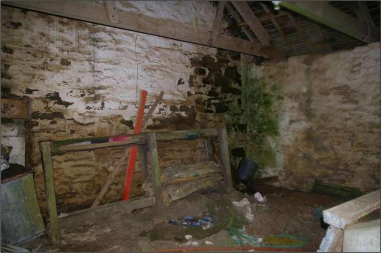
B3.1, EASTERN ROOM AND WALL OF B2; VIEWED FROM THE NORTH.
