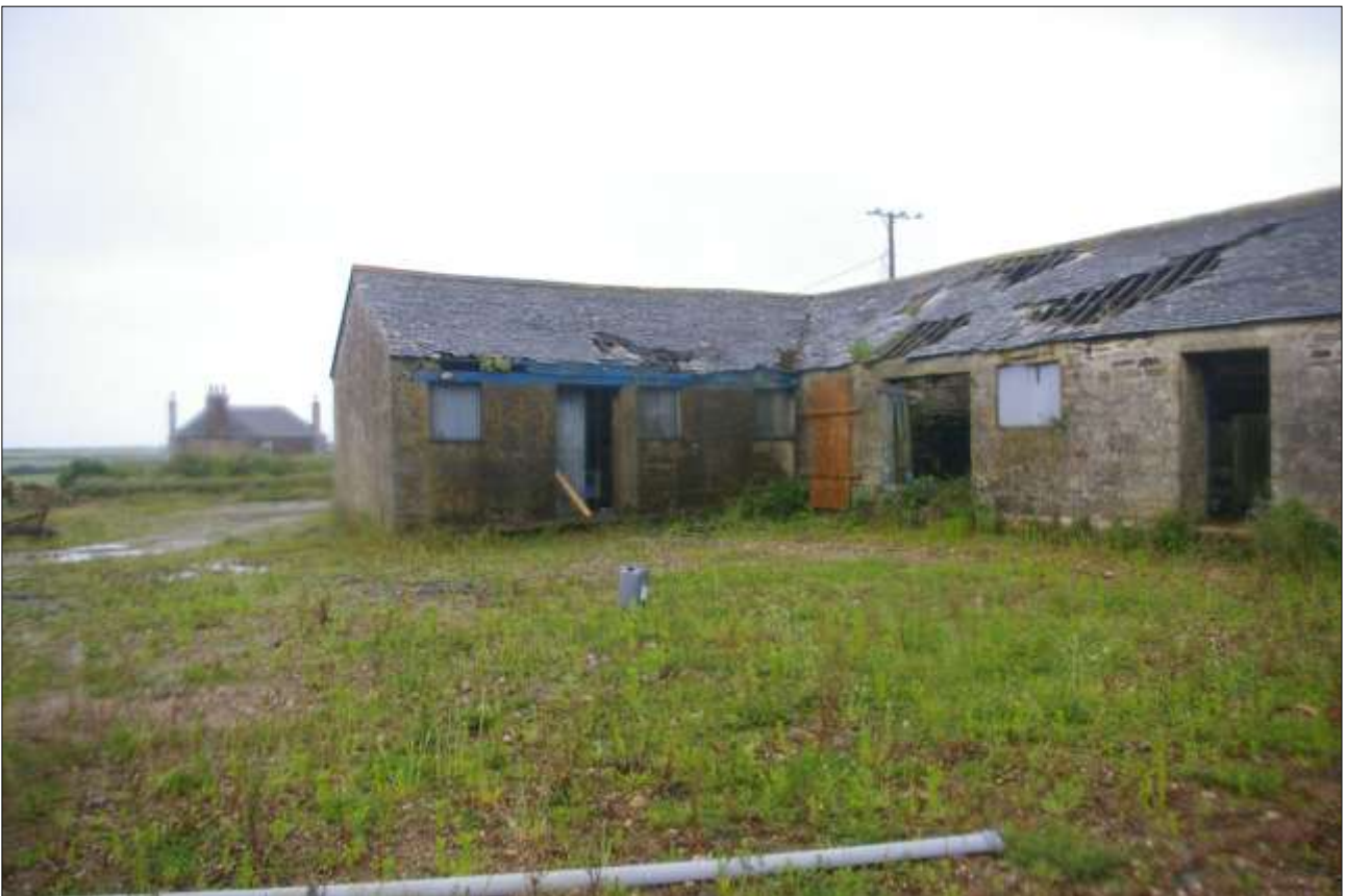
B5, YARD ELEVATIONS; VIEWED FROM THE NORTH-EAST.
