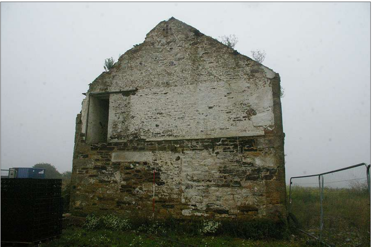
B1, NORTH-WEST ELEVATION; VIEWED FROM THE NORTH-WEST (SCALE 2M).
