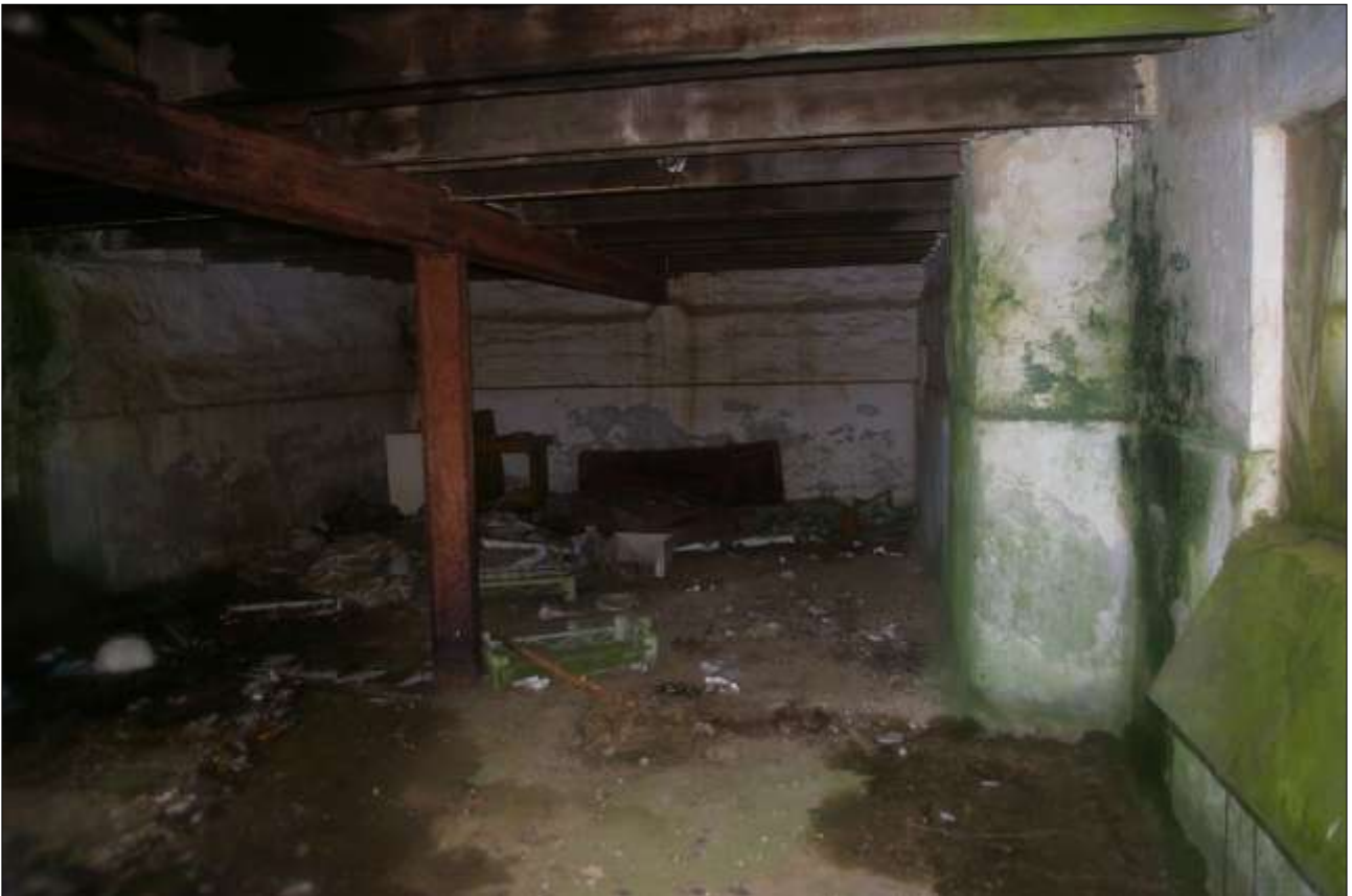
B2.2, NORTHERN GF ROOM; VIEWED FROM THE SOUTH.
