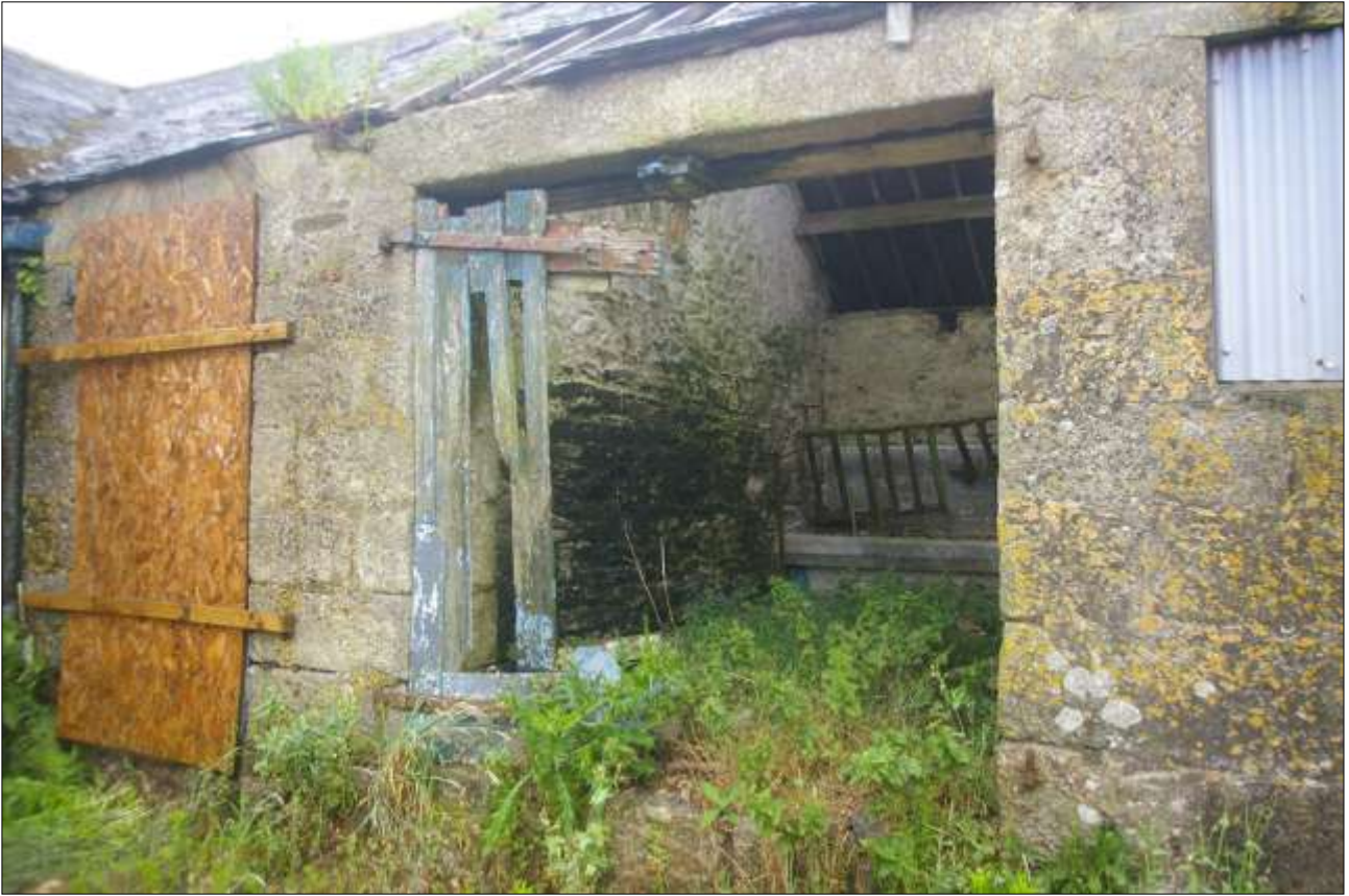
B5.1, NORTH ROOM; VIEWED FROM THE EAST.
