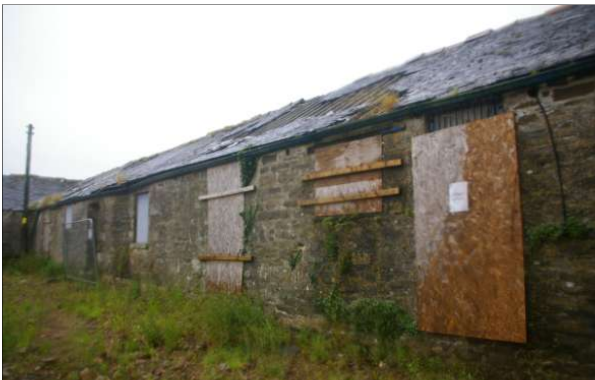
FIGURE 14: B3, THE SOUTH-WEST ELEVATION; VIEWED FROM THE SOUTH-SOUTH-EAST.
