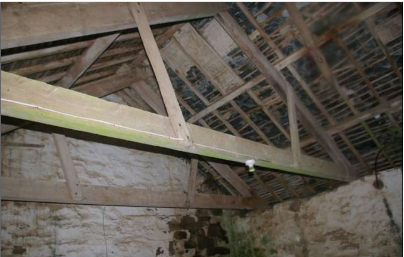
B3.1, EASTERN ROOM, ROOF STRUCTURE; VIEWED FROM THE NORTH.
