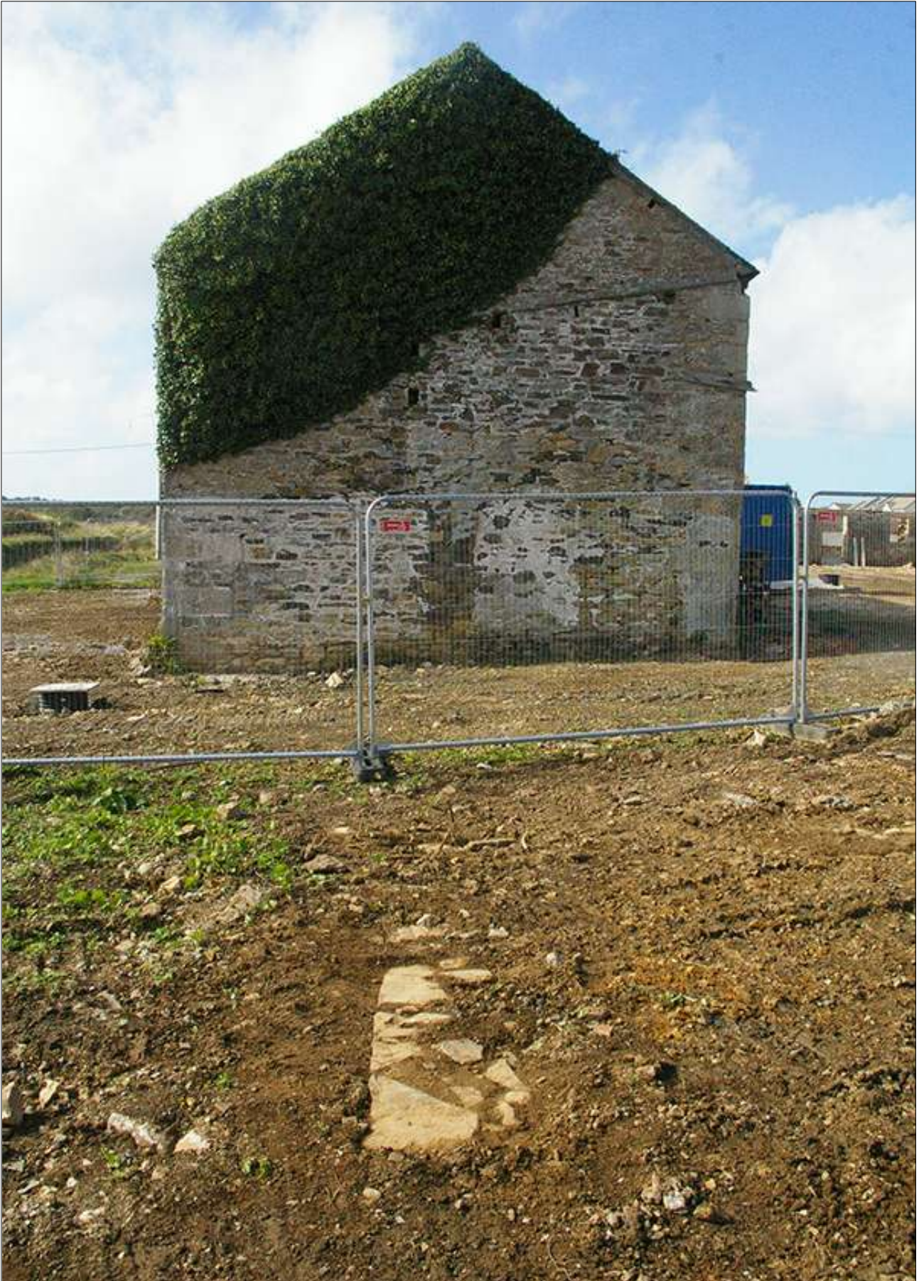
B1, SOUTH-EAST ELEVATION, WALL {302} IN THE FOREGROUND; VIEWED FROM THE SOUTH-EAST.
