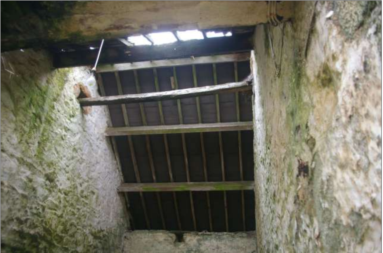
B5.1, NORTH ROOM, ROOF STRUCTURE; FROM THE EAST-NORTH-EAST.
