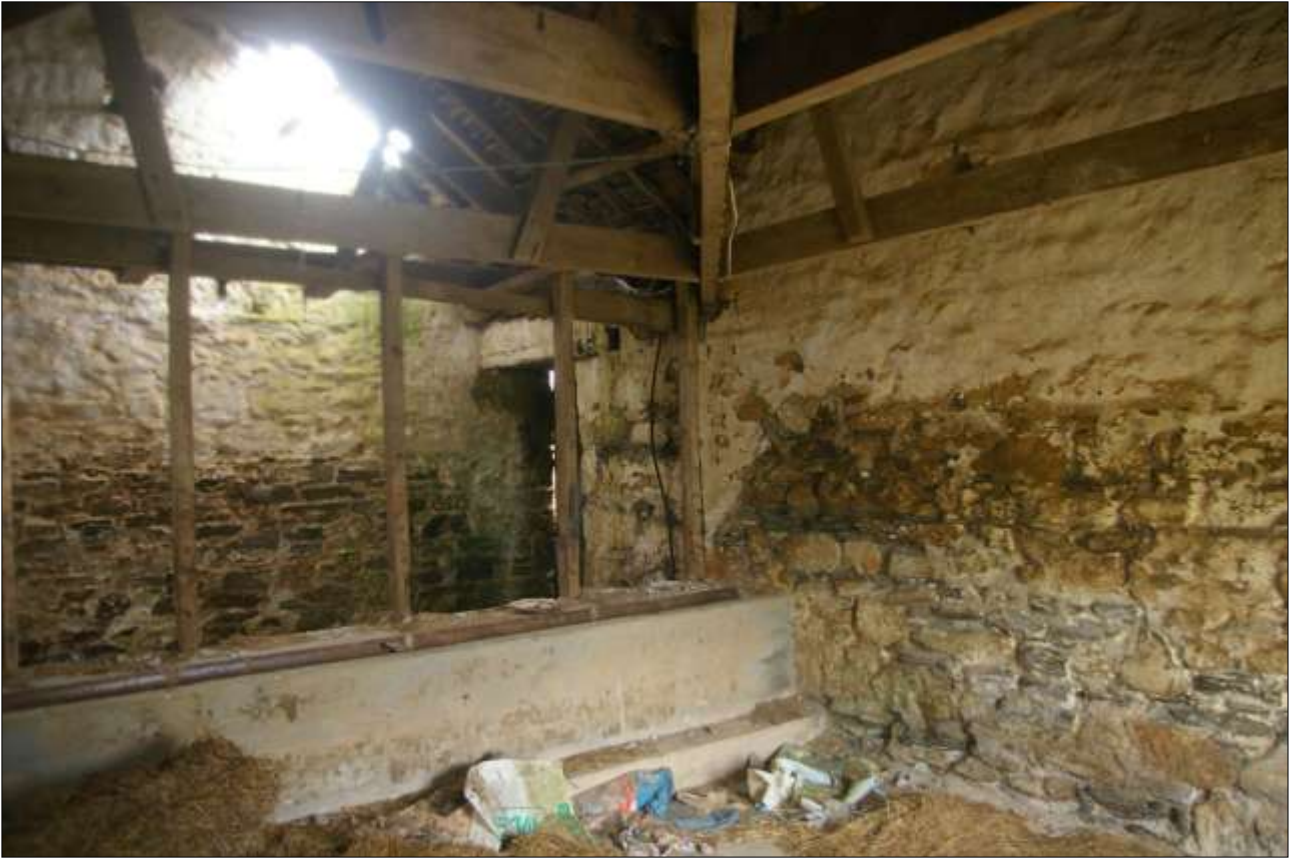
B5.2, SOUTH-WEST ROOM; VIEWED FROM THE WEST.
