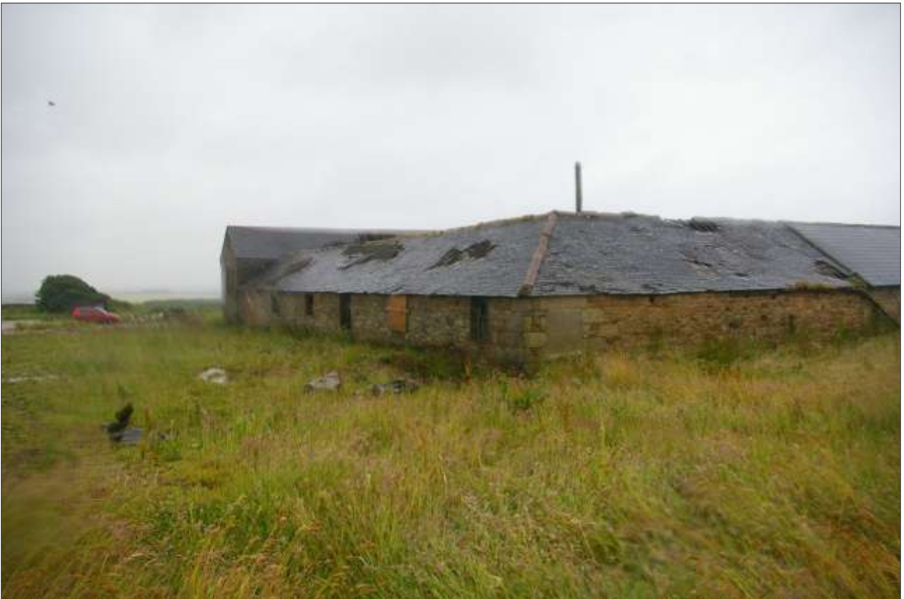
B3, NORTH-EAST ELEVATION; VIEWED FROM THE NORTH.
