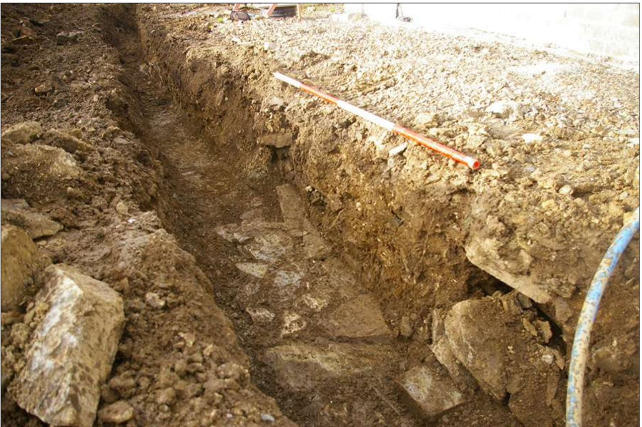
WALL {313}; VIEWED FROM THE EAST (SCALE 2M).
