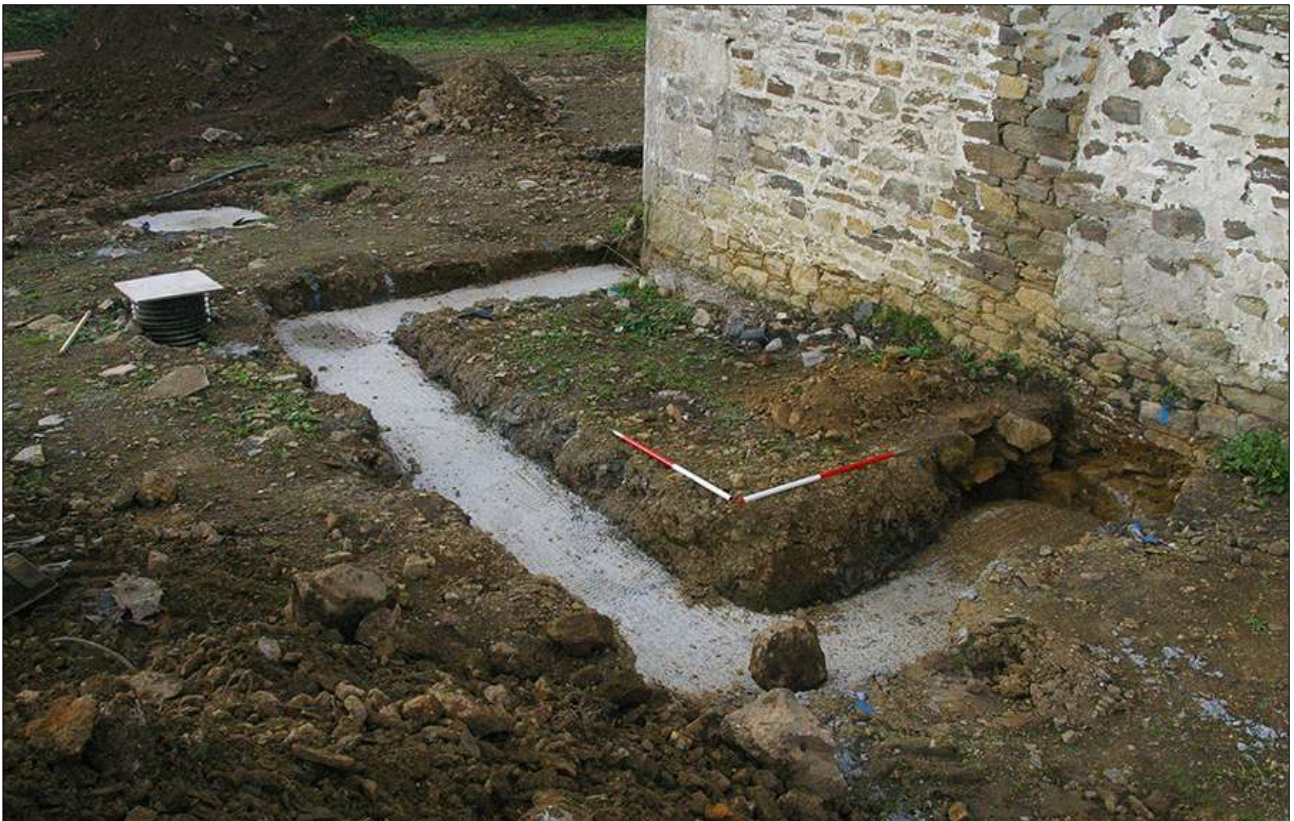
FOUNDATION TRENCH EAST OF B1; VIEWED FROM THE EAST (SCALE 1M).
