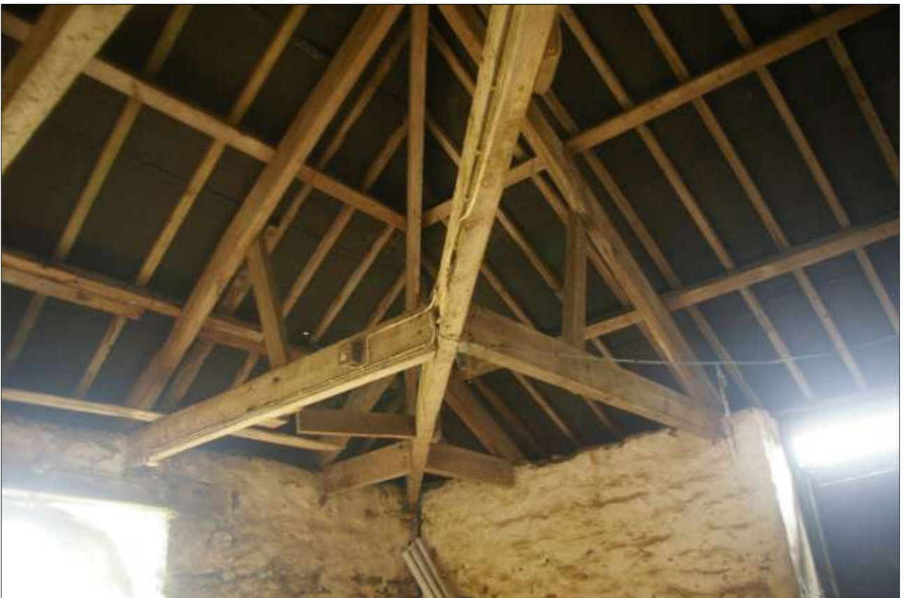
B5.2, SOUTH-WEST ROOM, ROOF STRUCTURE; VIEWED FROM THE EAST-NORTH-EAST.
