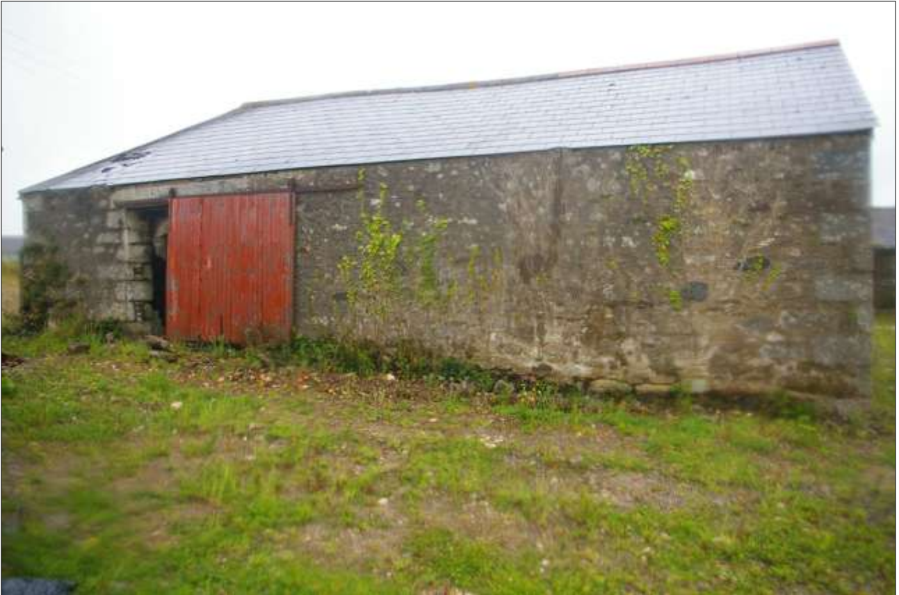
B5, SOUTH-WEST ELEVATION; VIEWED FROM THE SOUTH.
