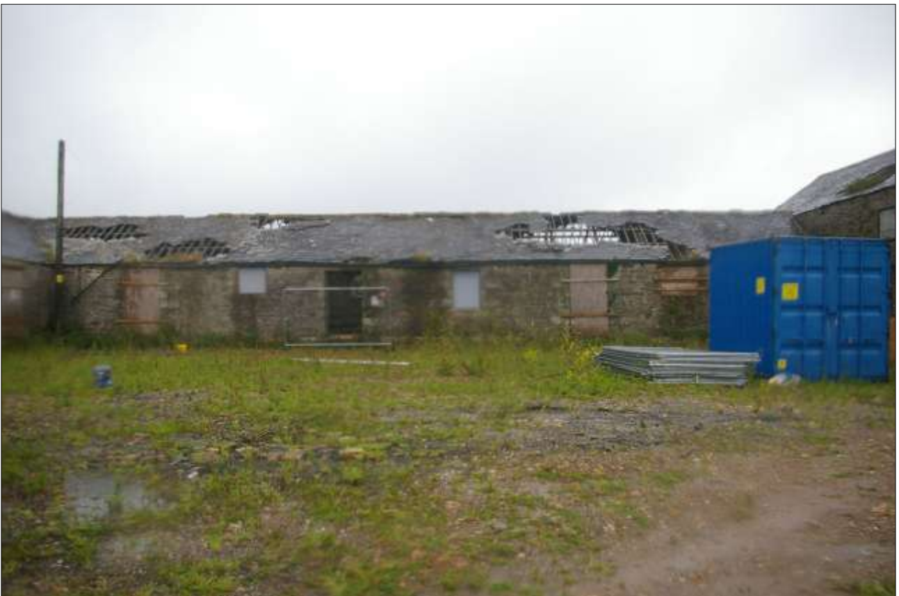
B3, THE SOUTH-WEST ELEVATION; VIEWED FROM THE SOUTH-WEST.
