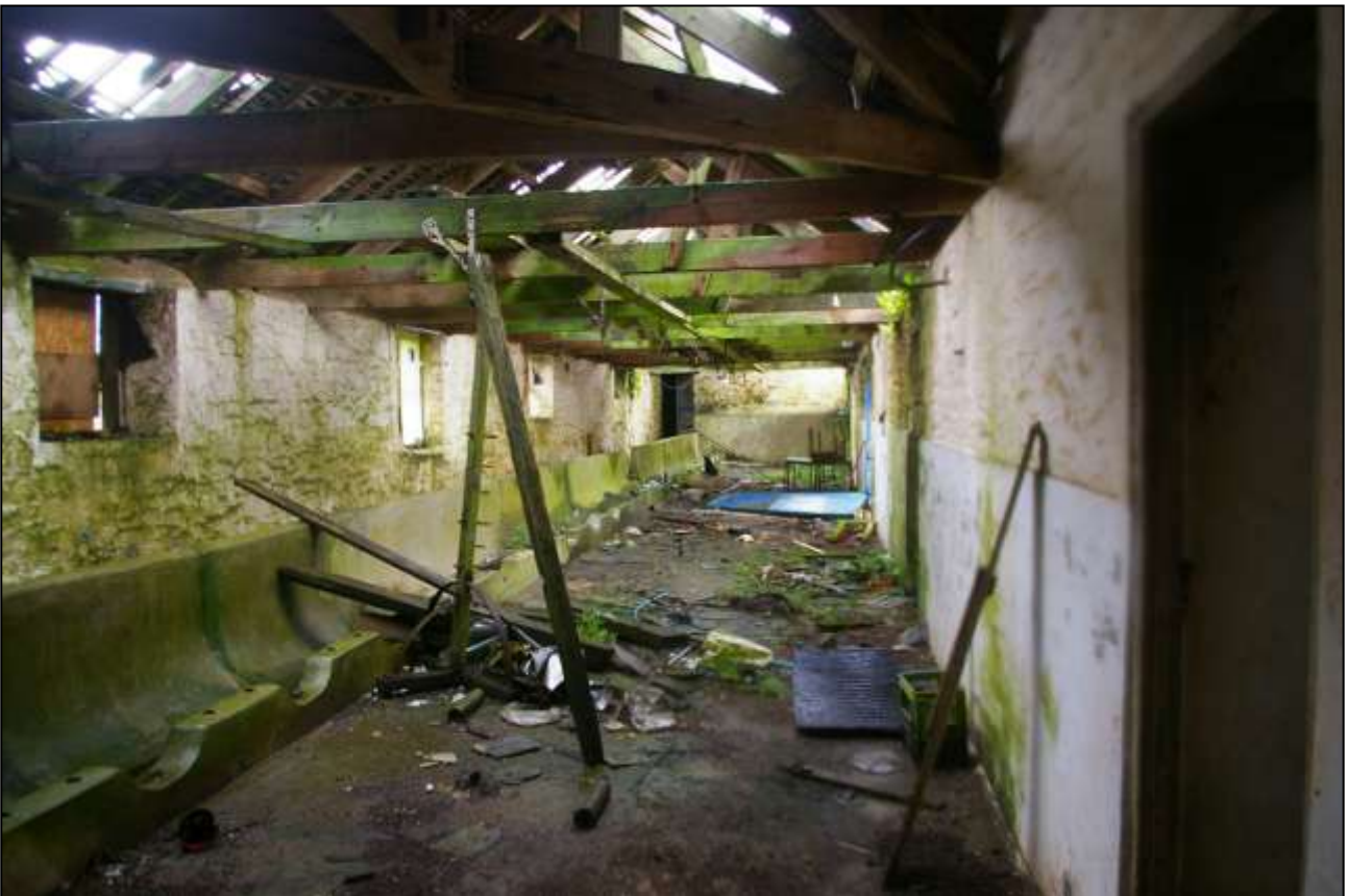
B3.2, WESTERN ROOM; VIEWED FROM SOUTH-WEST CORNER.
