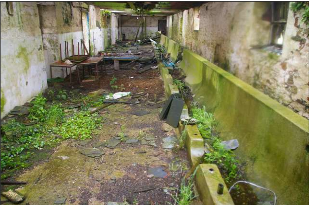
B3.2, WESTERN ROOM, SHOWING THE CONCRETE FLOORS AND CATTLE STALLS; VIEWED FROM THE SOUTH-EAST.
