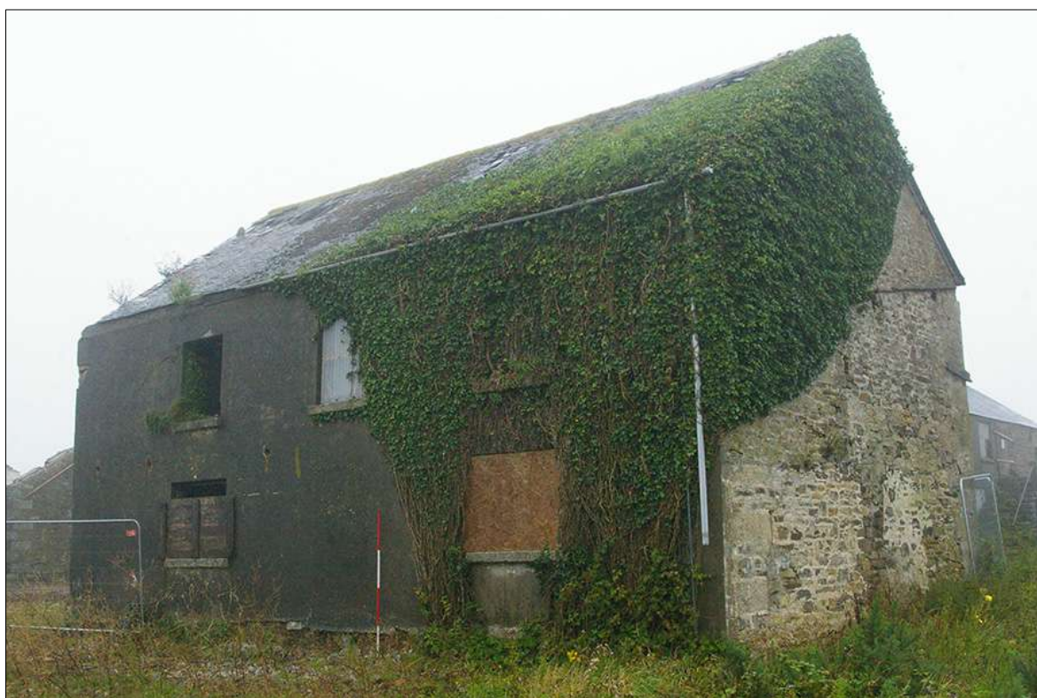
FIGURE 12: B1, SOUTH-WEST ELEVATION; VIEWED FROM THE SOUTH (SCALE 2M).
