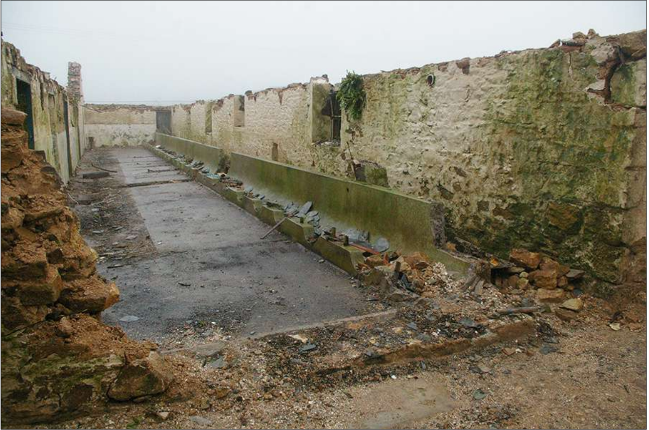
B3.2, DURING WORKS; VIEWED FROM THE SOUTH-EAST.
