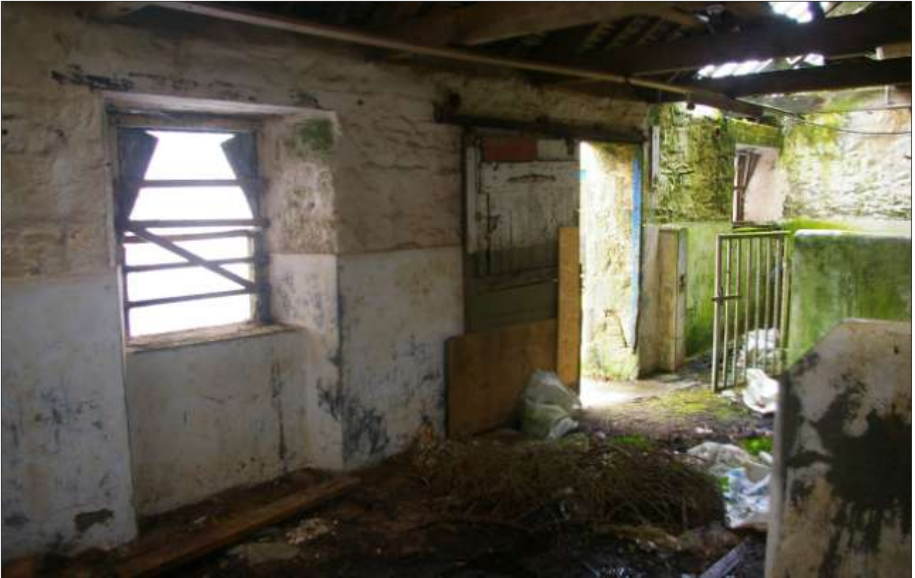
B4, SOUTH ROOM, SOUTH-EAST ELEVATION; VIEWED FROM THE NORTH.
