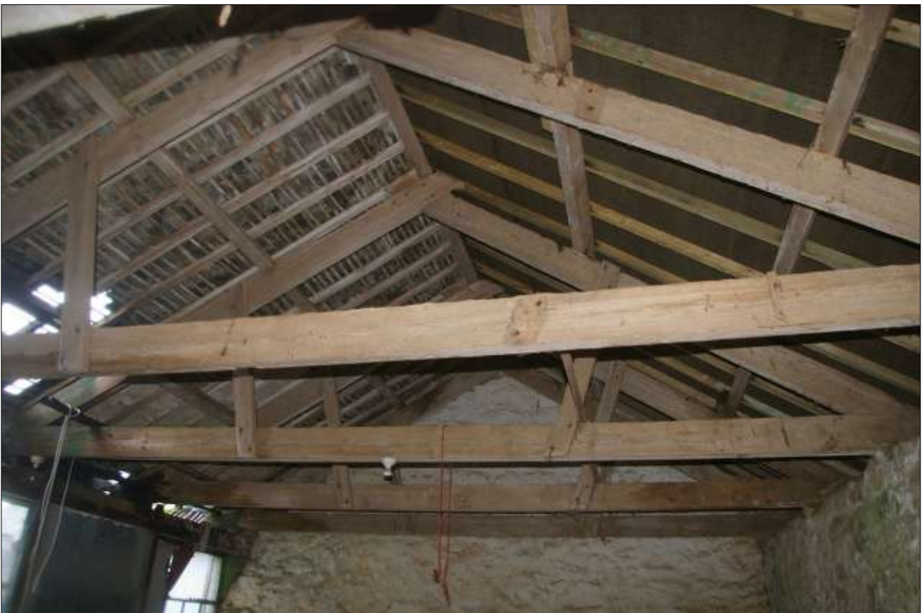
B5.3, EAST ROOM, ROOF STRUCTURE; VIEWED FROM THE WEST-SOUTH-WEST.
