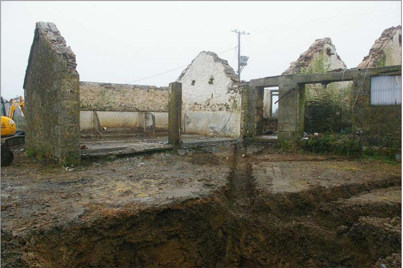
B5, AS ABOVE, DURING MONITORING WORKS; VIEWED FROM THE EAST.
