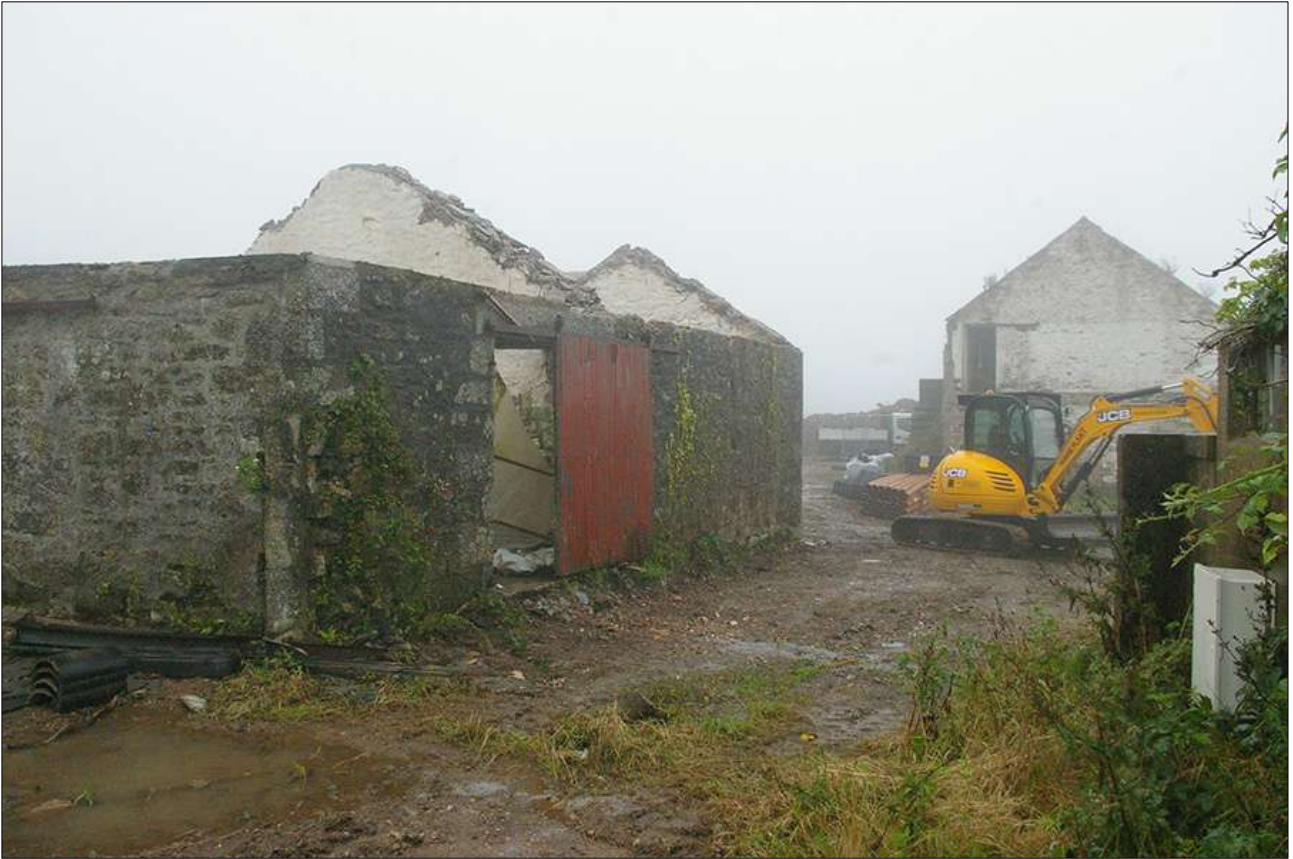
B5, DURING WORKS; VIEWED FROM THE WEST.
