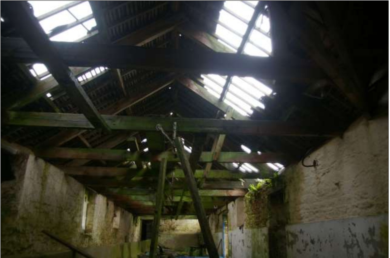
B3.2, ROOF STRUCTURE; VIEWED FROM THE WEST-NORTH-WEST.
