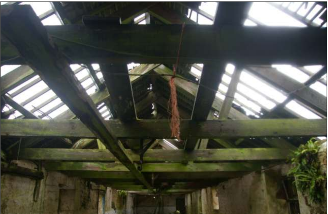
B3.2, ROOF STRUCTURE; VIEWED FROM THE SOUTH-EAST.
