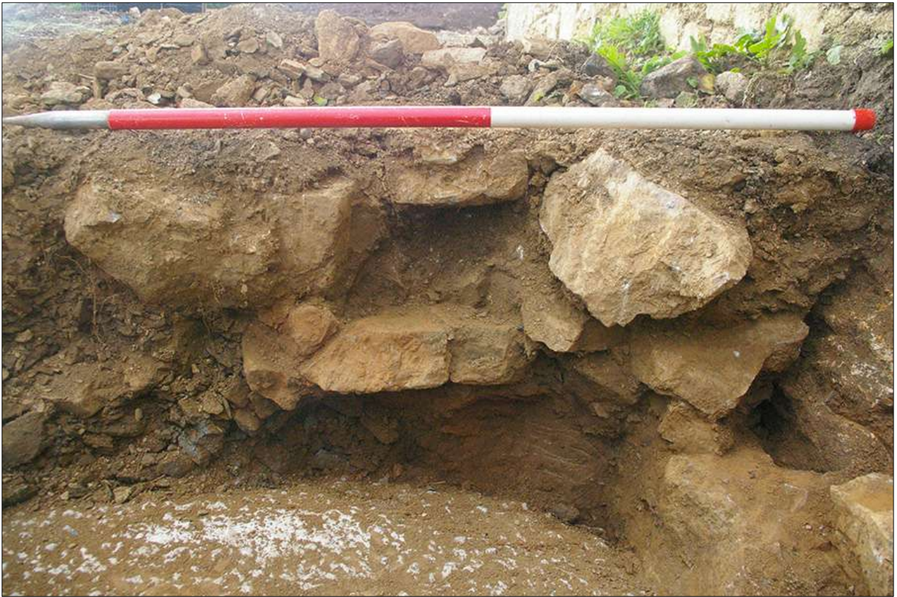
WALL {305}; VIEWED FROM THE NORTH-EAST (SCALE 1M).
