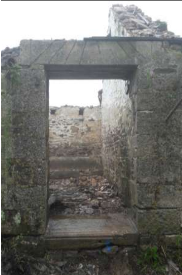
FIGURE 17: B5.2 (D21), NORTH-EAST ELEVATION, SHOWING THE REUSED GRANITE LINTEL (INCISED LINES TO MIMIC VOUSSOIRS, INSERTED UPSIDE-DOWN) AND REUSED MOULDED GRANITE FIREPLACE LINTEL; VIEWED FROM THE EAST.
