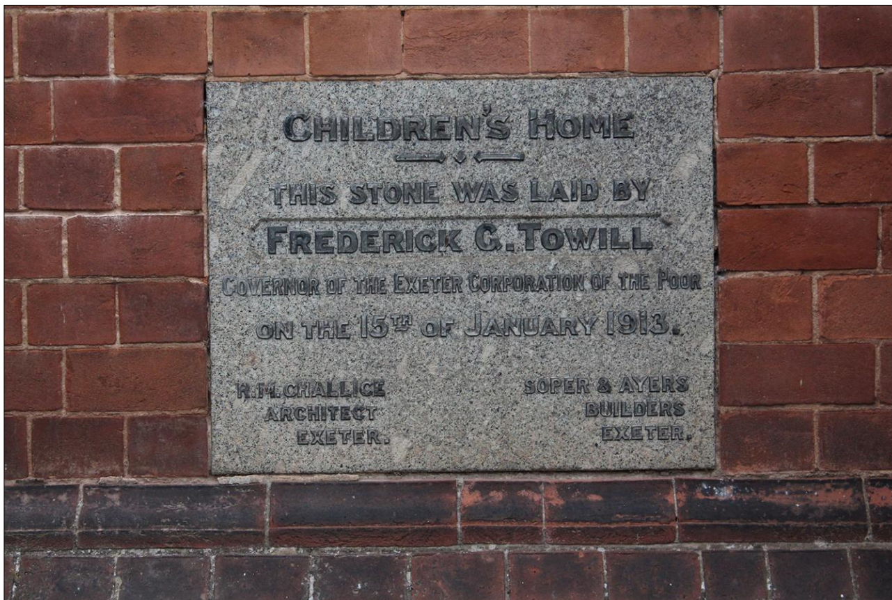
31. DETAIL OF PLAQUE/FOUNDATION STONE IN FRONT (SOUTH-WEST) EXTERNAL ELEVATION OF BUILDING; VIEWED FROM THE SOUTH-WEST.
