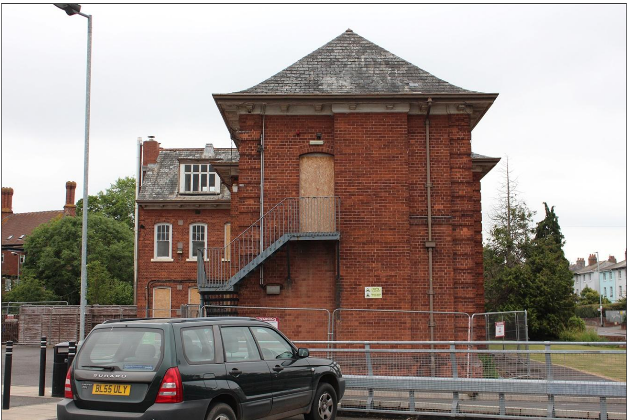
20. NORTH-WEST EXTERNAL ELEVATION OF BUILDING; VIEWED FROM THE NORTH-WEST.
