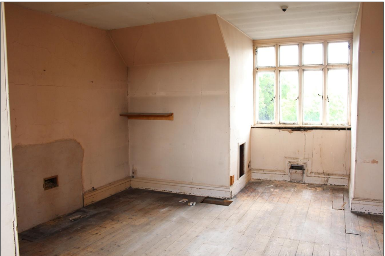
96. VIEW OF ROOM S7; VIEWED FROM THE NORTH-WEST.
