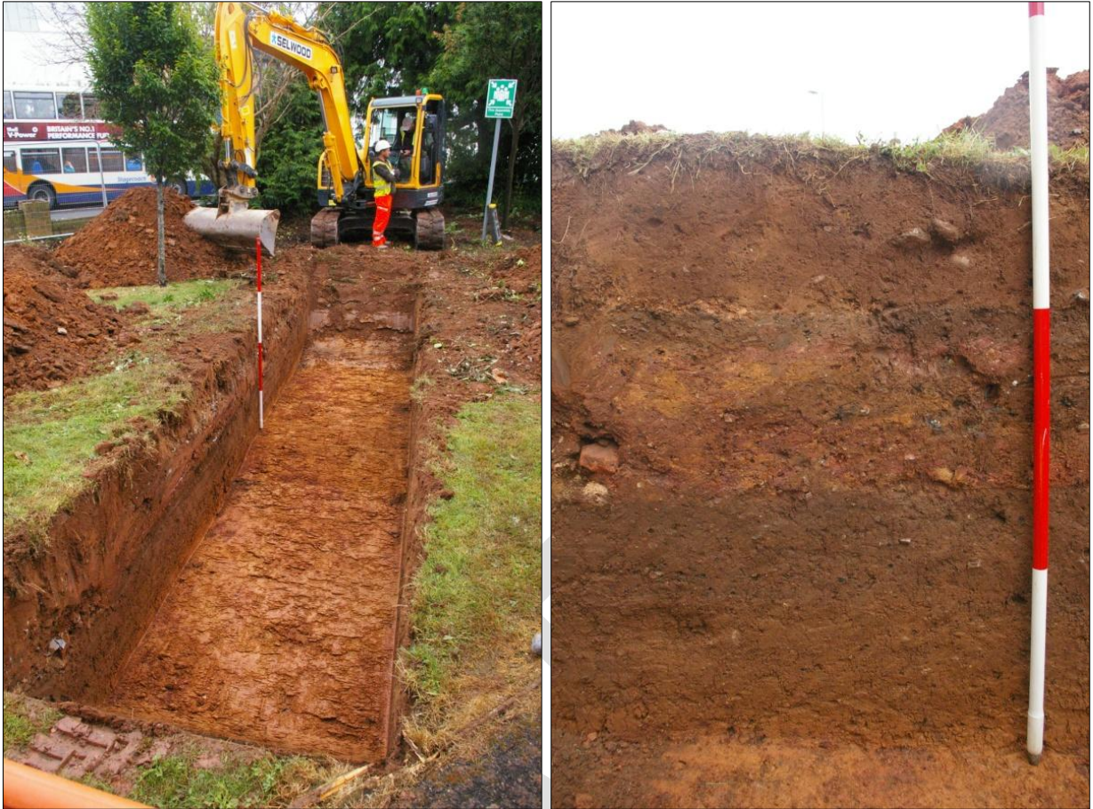
FIGURE 3: (LEFT) TRENCH 01 POST-EXCAVATION; VIEWED FROM THE EAST (2M SCALE).
