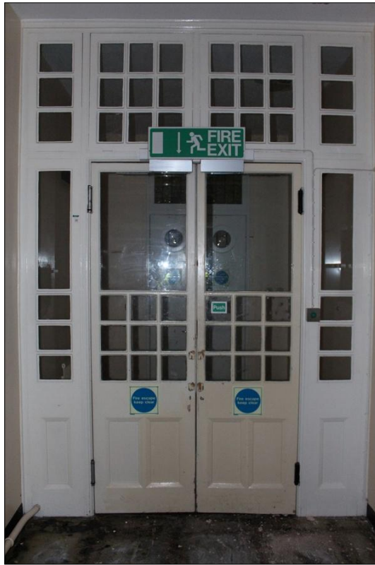
43. DETAIL OF SCREEN BETWEEN ROOM 21 AND ROOM 22; VIEWED FROM THE NORTH-EAST.
