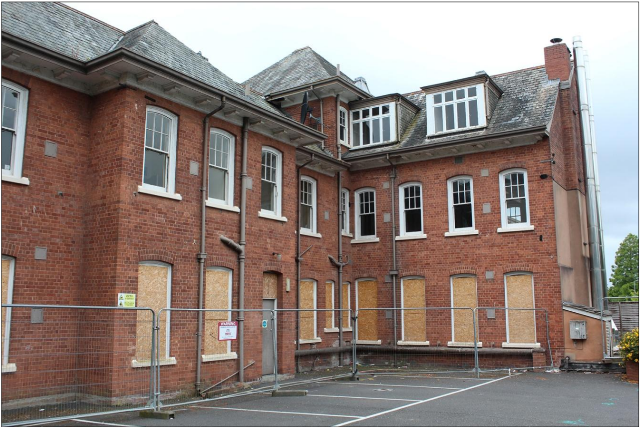
11. REAR (NORTH-EAST) EXTERNAL ELEVATION OF BUILDING; VIEWED FROM THE EAST.
