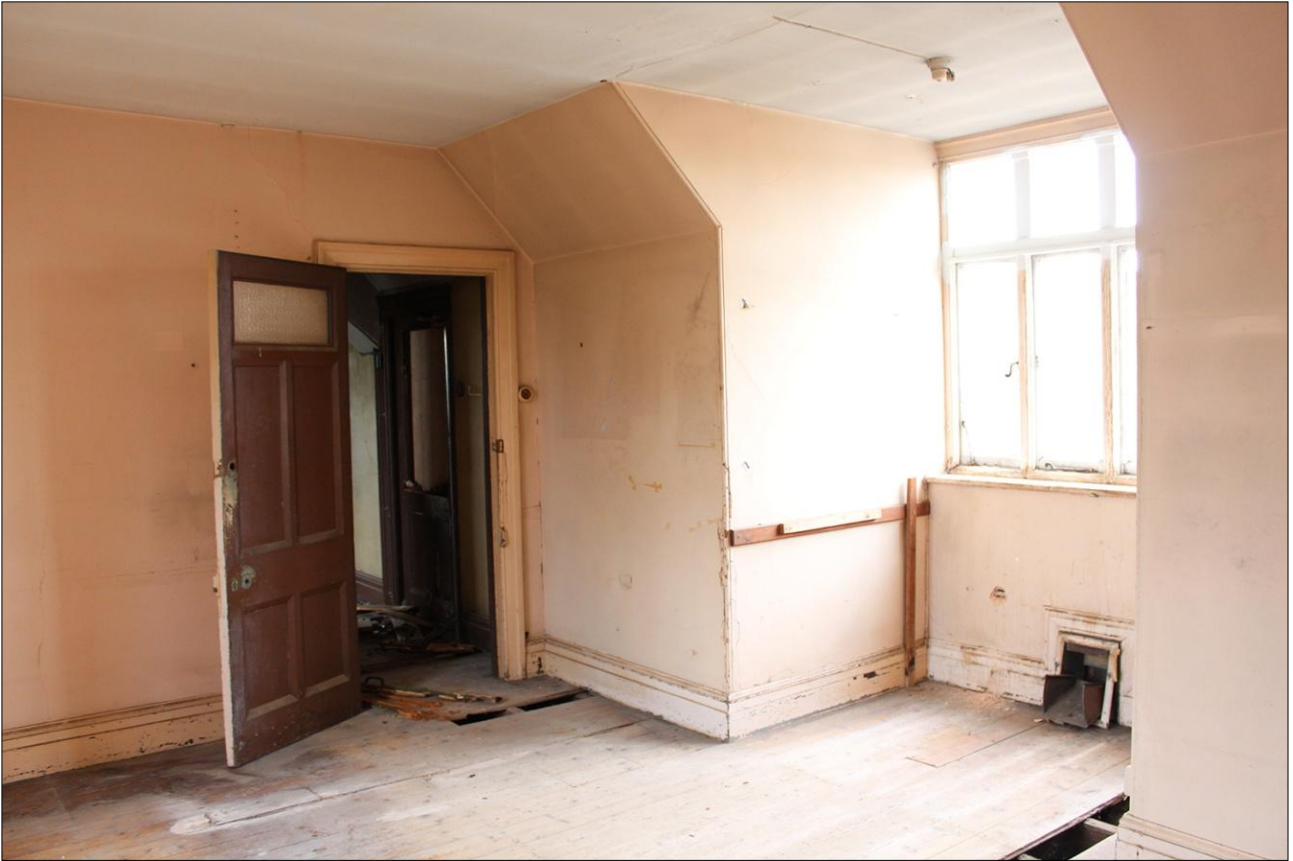
95. VIEW OF ROOM S7; VIEWED FROM THE NORTH-EAST.
