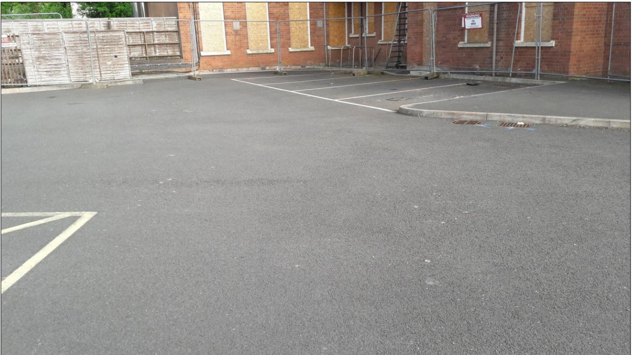
8. CAR PARK AREA TO REAR (NORTH) OF BUILDING, WEST END; VIEWED FROM THE NORTH-WEST (NO SCALE).
