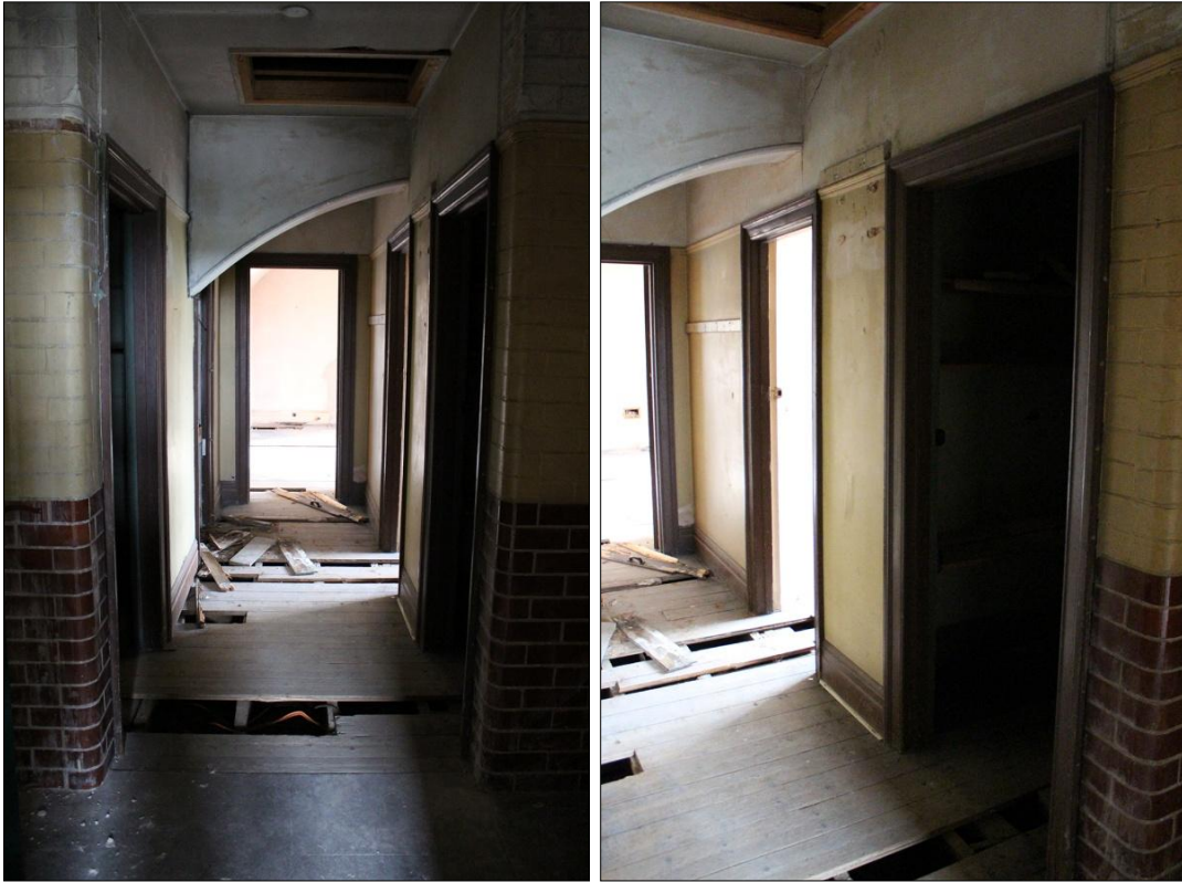
LEFT: 89. VIEW ALONG CORRIDOR S8; VIEWED FROM THE SOUTH-WEST.
