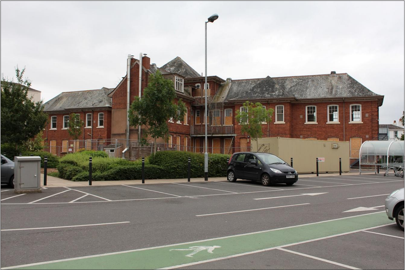
17. REAR (NORTH-EAST) EXTERNAL ELEVATION OF BUILDING; VIEWED FROM THE NORTH-WEST.
