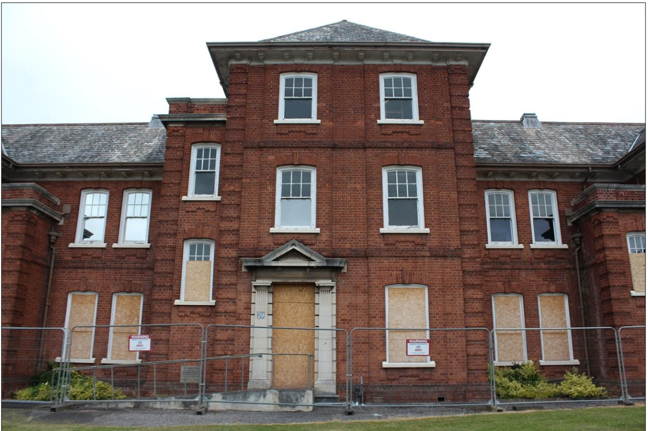
26. FRONT (SOUTH-WEST) EXTERNAL ELEVATION OF BUILDING, MID; VIEWED FROM THE SOUTH-WEST.
