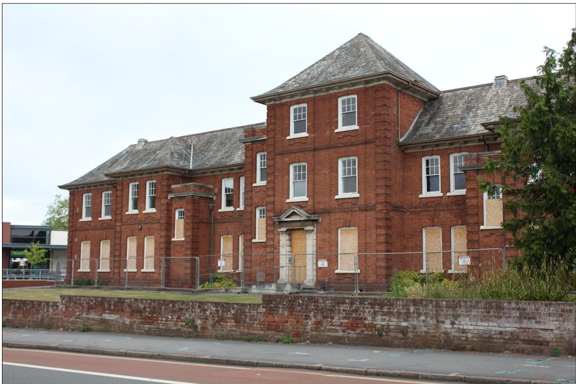
FIGURE 7: THE FRONT (SOUTH-WEST) ELEVATION OF THE BUILDING; VIEWED FROM THE SOUTH.
