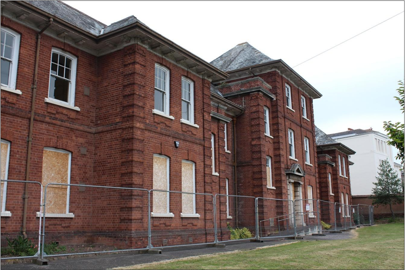
23. FRONT (SOUTH-WEST) EXTERNAL ELEVATION OF BUILDING; VIEWED FROM THE WEST.
