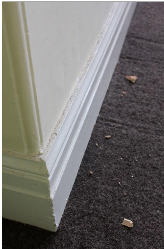
55. DETAIL OF SKIRTING, ROOM F4; VIEWED FROM THE NORTH-EAST.
