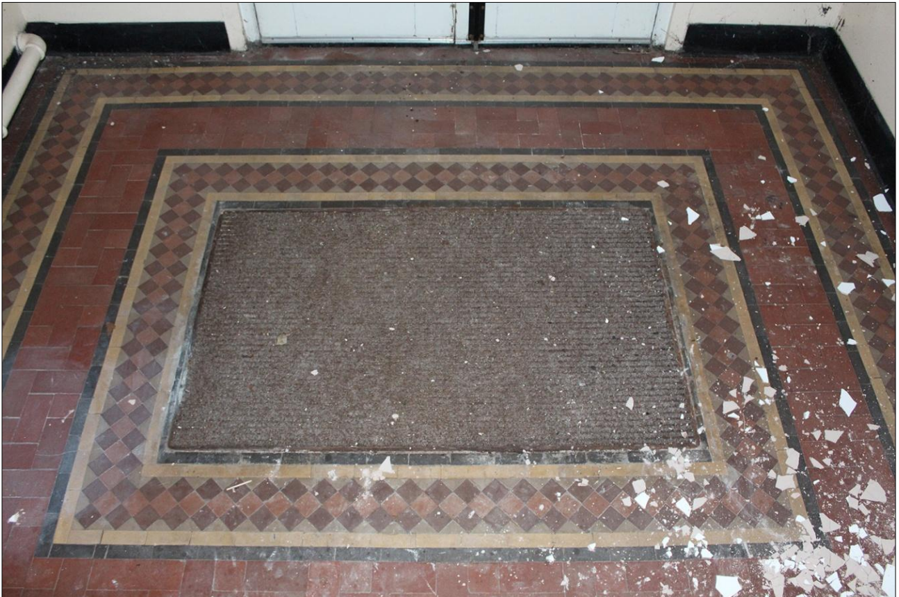
44. DETAIL OF FLOOR SURFACE WITHIN ROOM 22; VIEWED FROM THE NORTH-EAST.
