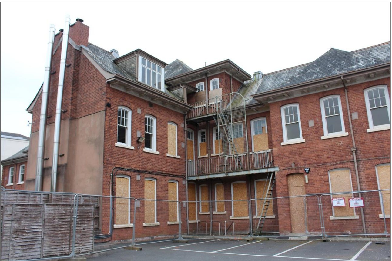
14. REAR (NORTH-EAST) EXTERNAL ELEVATION OF BUILDING, WEST END; VIEWED FROM THE NORTH-WEST.
