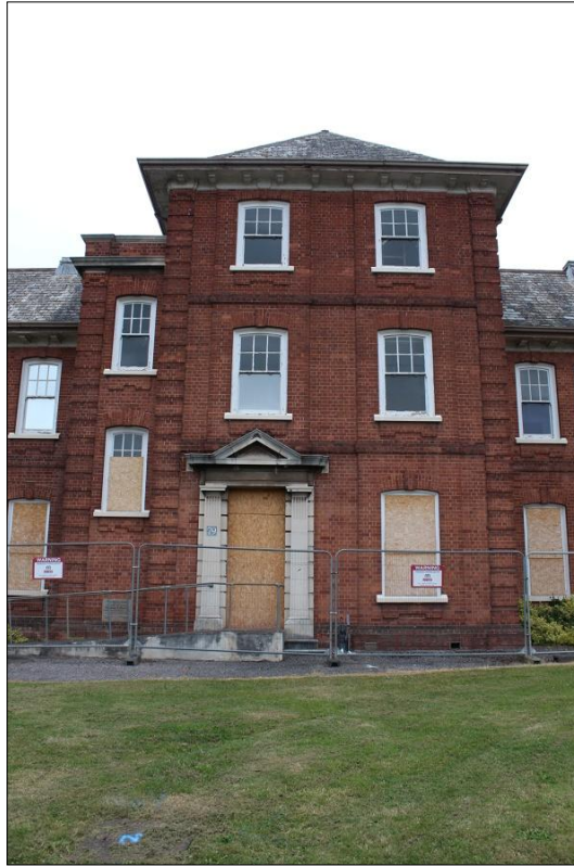
25. FRONT (SOUTH-WEST) EXTERNAL ELEVATION OF BUILDING, MID; VIEWED FROM THE SOUTH-WEST.
