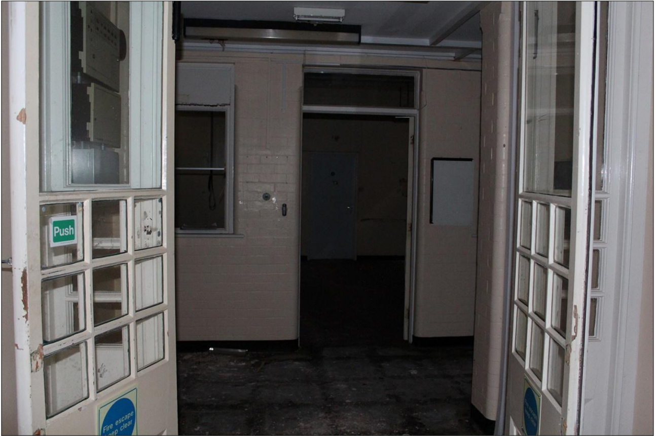
45. VIEW OF ROOM 21; VIEWED FROM THE SOUTH-WEST.
