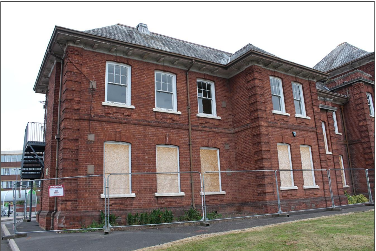
22. FRONT (SOUTH-WEST) EXTERNAL ELEVATION OF BUILDING, WEST END; VIEWED FROM THE SOUTH-WEST.
