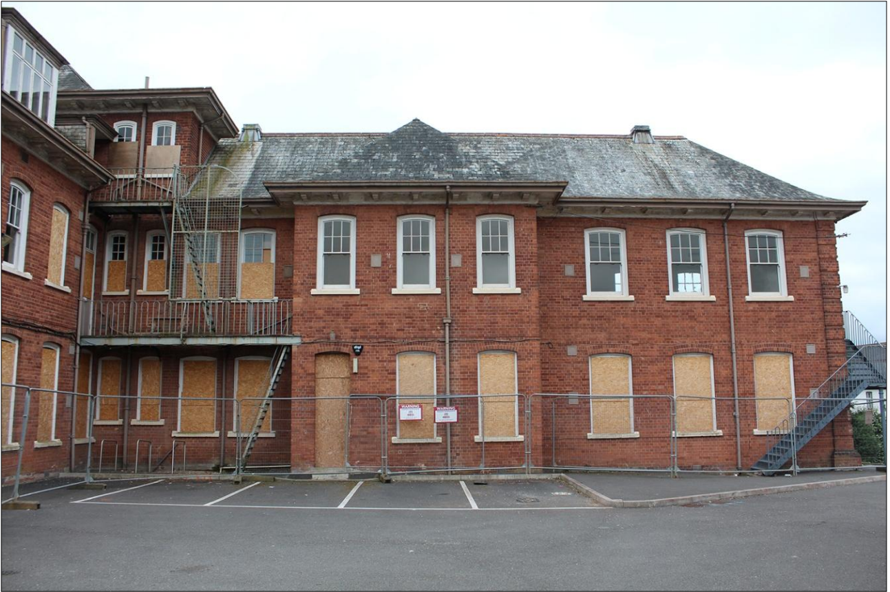
13. REAR (NORTH-EAST) EXTERNAL ELEVATION OF BUILDING, WEST END; VIEWED FROM THE NORTH-EAST.
