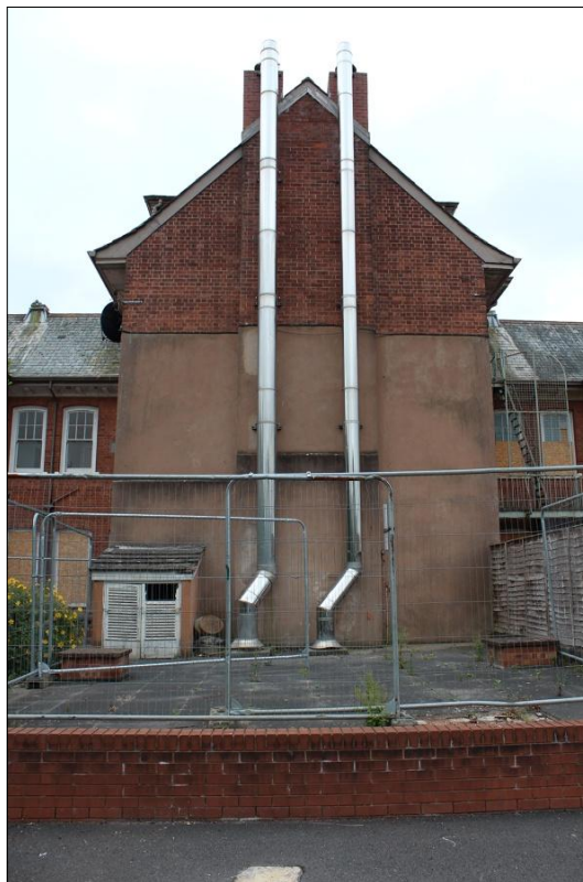
12. REAR (NORTH-EAST) EXTERNAL ELEVATION OF BUILDING, MID; VIEWED FROM THE NORTH-EAST.
