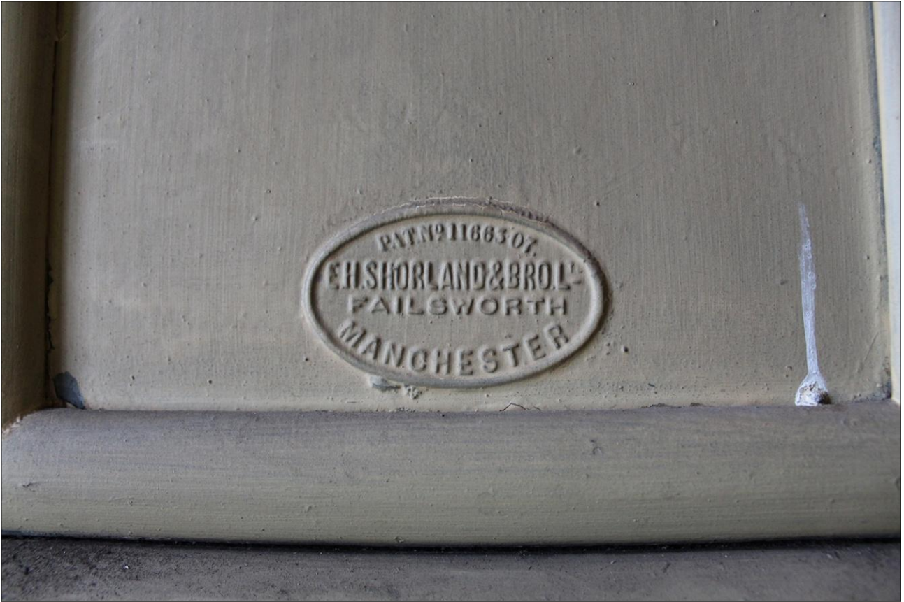
104. DETAIL OF THE NAMEPLATE ON THE VENT IN ROOM S11; VIEWED FROM THE NORTH-WEST.
