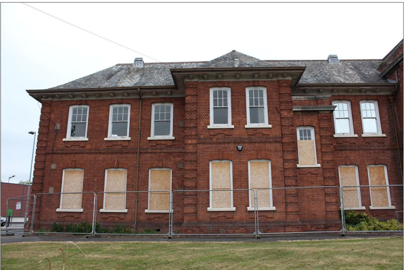
24. FRONT (SOUTH-WEST) EXTERNAL ELEVATION OF BUILDING, WEST END; VIEWED FROM THE SOUTH-WEST.
