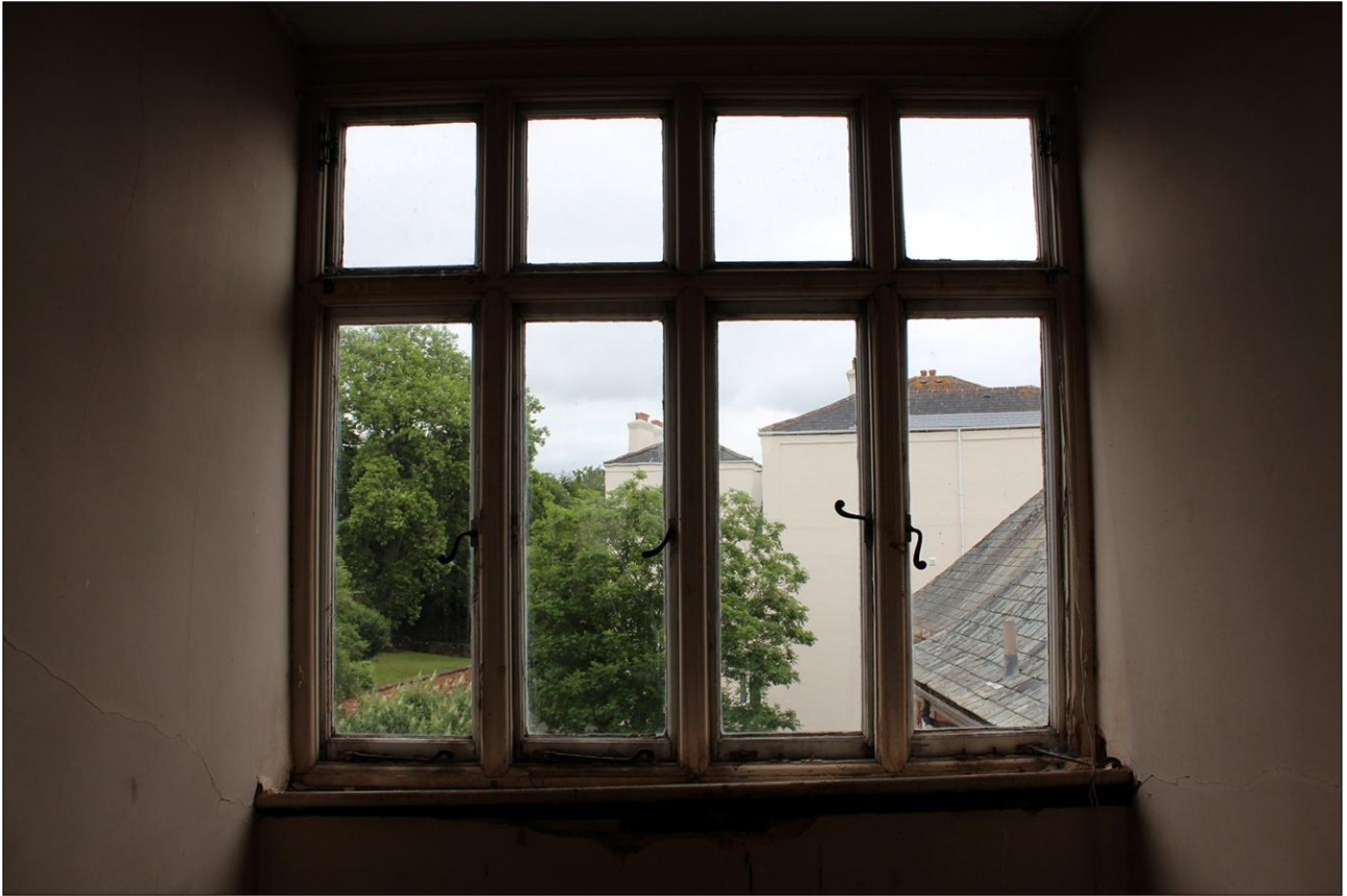
97. DETAIL OF THE WINDOW OPENING IN THE SOUTH-EAST WALL OF ROOM S7; VIEWED FROM THE NORTH-WEST.
