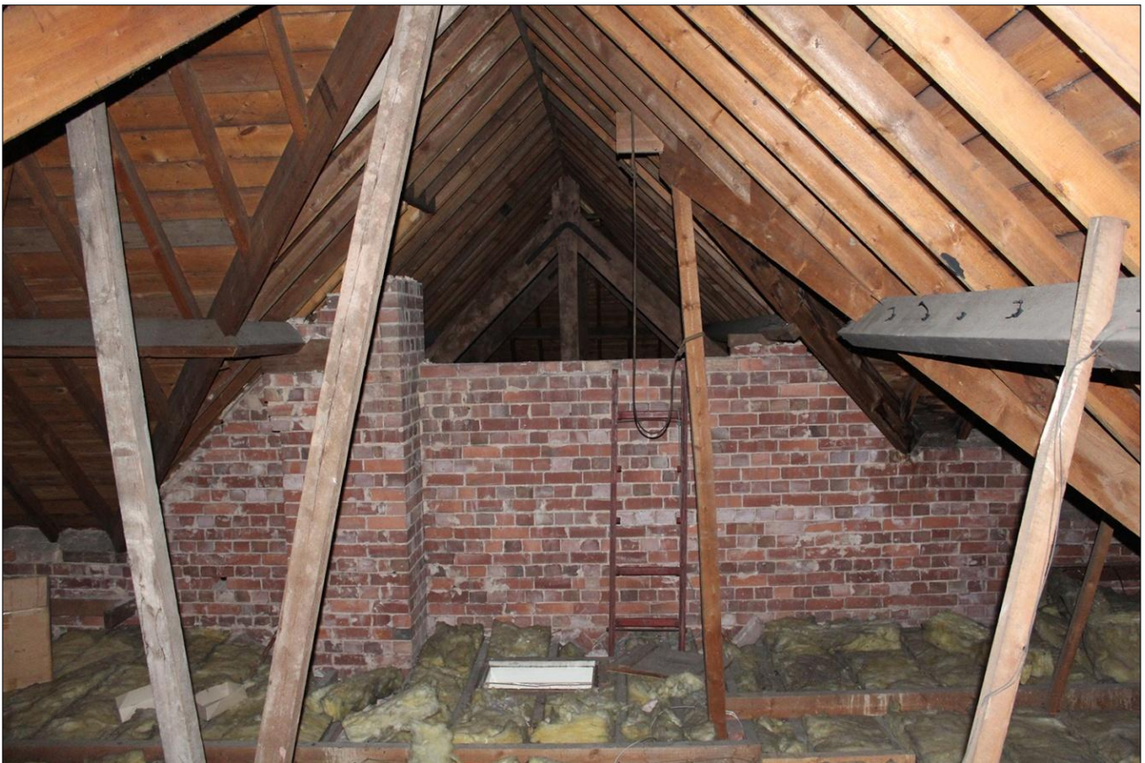
88. DETAIL OF THE ROOF STRUCTURE WITHIN ROOM S13 WITH DIVIDING BRICKWORK; VIEWED FROM THE NORTH-WEST.
