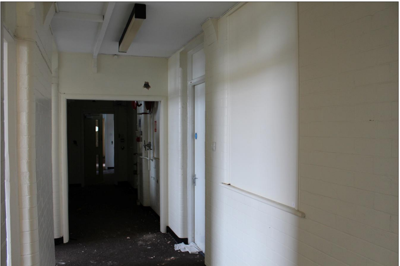
62. VIEW ALONG CORRIDOR F10; VIEWED FROM THE SOUTH-EAST.
