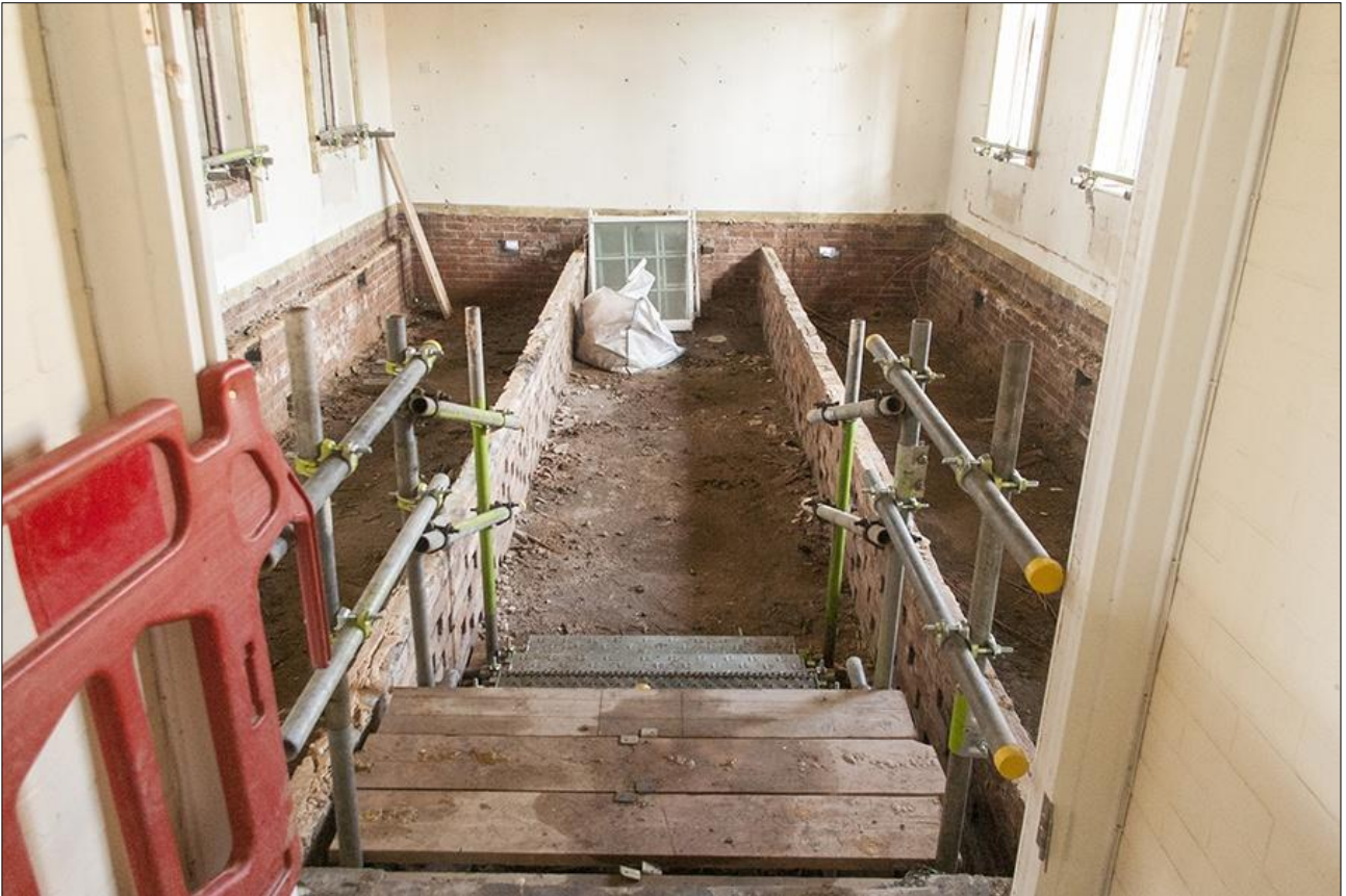
106. ROOM G1, SHOWING THE UNDER-FLOOR CAVITY; VIEWED FROM THE SOUTH-EAST.
