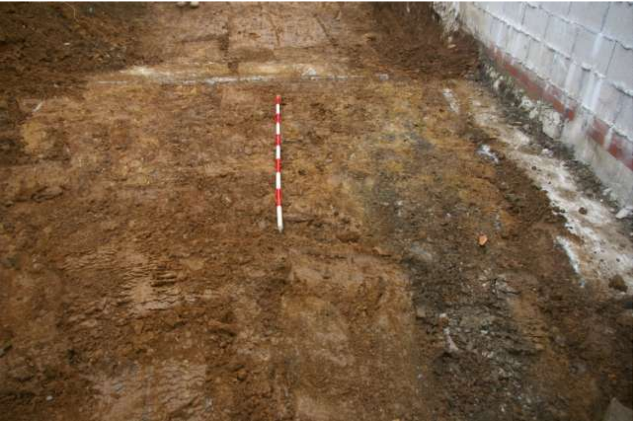
Figure 3: Concrete foundation trenching for garage; from the north (2m scale).
