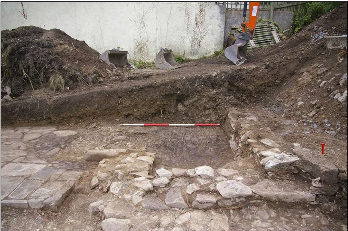
SECTION ALONG WESTERN LIMIT OF EXCAVATION; VIEWED FROM THE SOUTH-EAST (2M SCALE).
