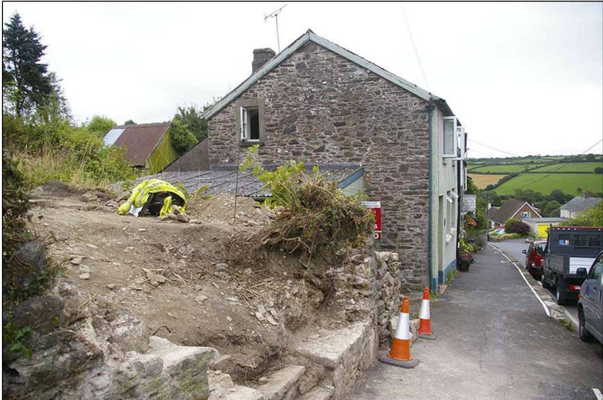
ENTRANCE TO SITE DURING EXCAVATION; VIEWED FROM THE WEST (1M SCALE).
