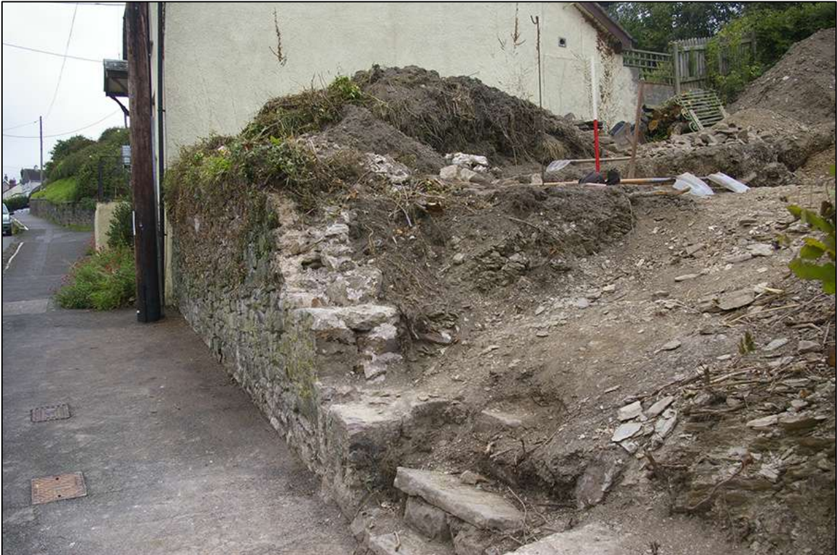
ENTRANCE TO SITE DURING EXCAVATION; VIEWED FROM THE SOUTHSOUTH-EAST (1M SCALE).
