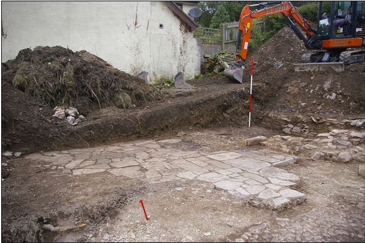
WESTERN HALF OF SITE, MID-EXCAVATION; VIEWED FROM THE SOUTH (2M SCALE).
