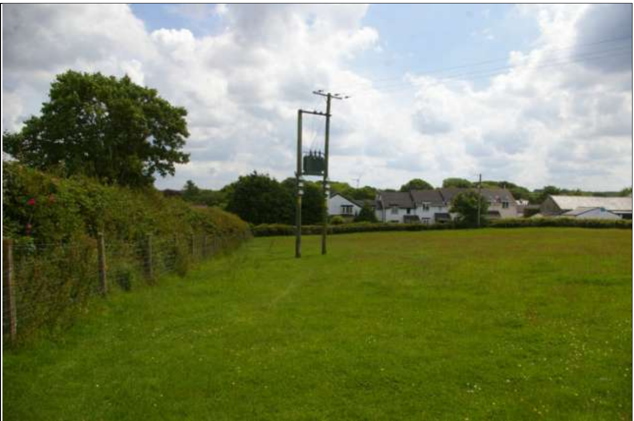
TELEGRAPH POLES IN THE SOUTH-EAST OF THE SITE; VIEWED FROM THE NORTH.
