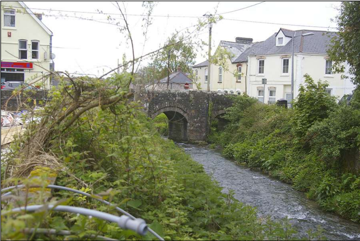
FIGURE 17: THE 'OLD BRIDGE' TO THE SOUTH OF THE SITE; VIEWED FROM THE NORTH-WEST.
