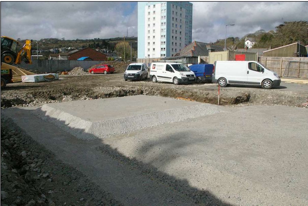
FIGURE 10: LARGE EXCAVATED AREA; VIEWED FROM THE SOUTH (1M SCALE).
