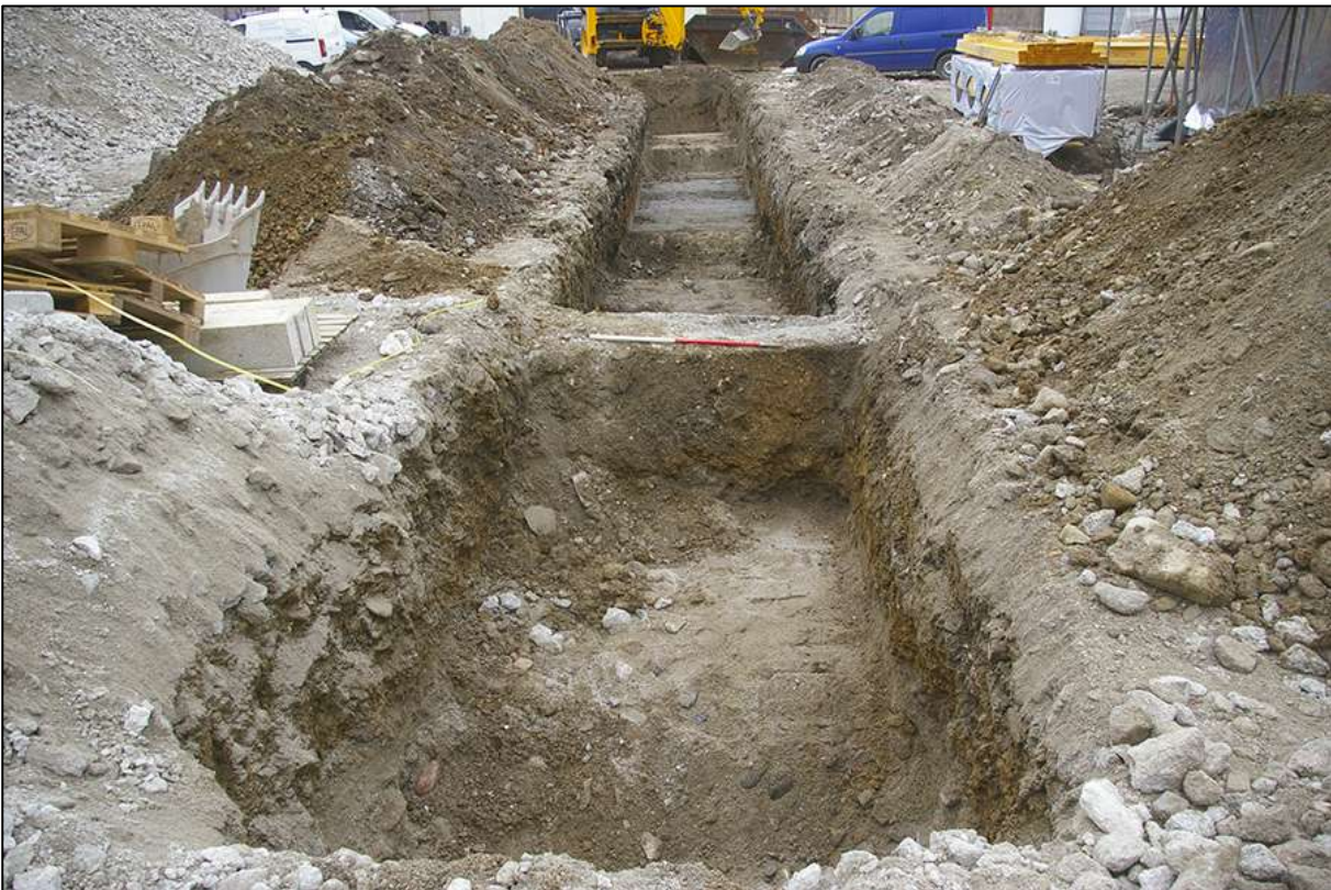
FIGURE 16: 24M LONG TRENCH, POST-EXCAVATION; VIEWED FROM THE SOUTH-WEST (1M SCALE).
