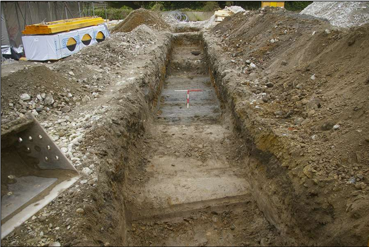
FIGURE 19: 24M LONG TRENCH, POST-EXCAVATION; VIEWED FROM THE NORTH-EAST (1M AND 2 M SCALES).
