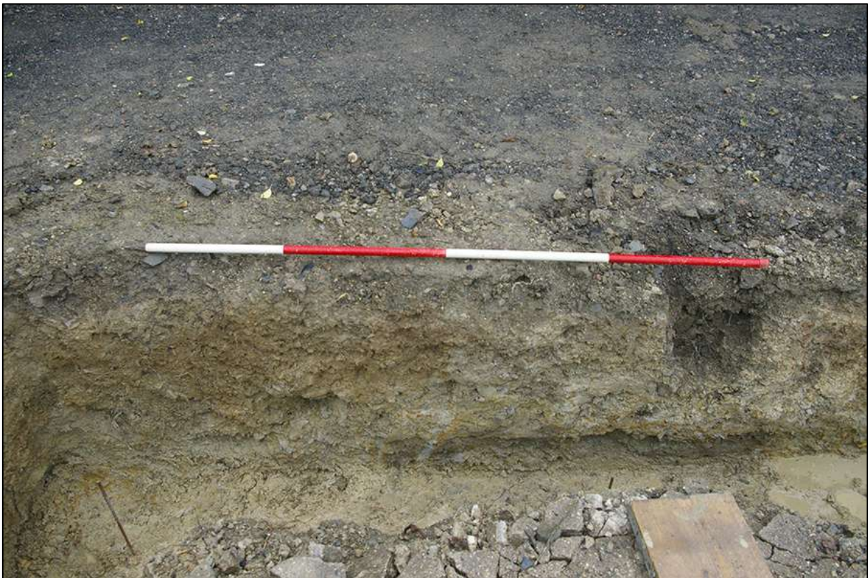
AREA 01 NORTHERN FOUNDATION TRENCH, SOUTH-WEST FACING SECTION, WEST END; VIEWED FROM THE SOUTH-WEST (2M SCALE).
