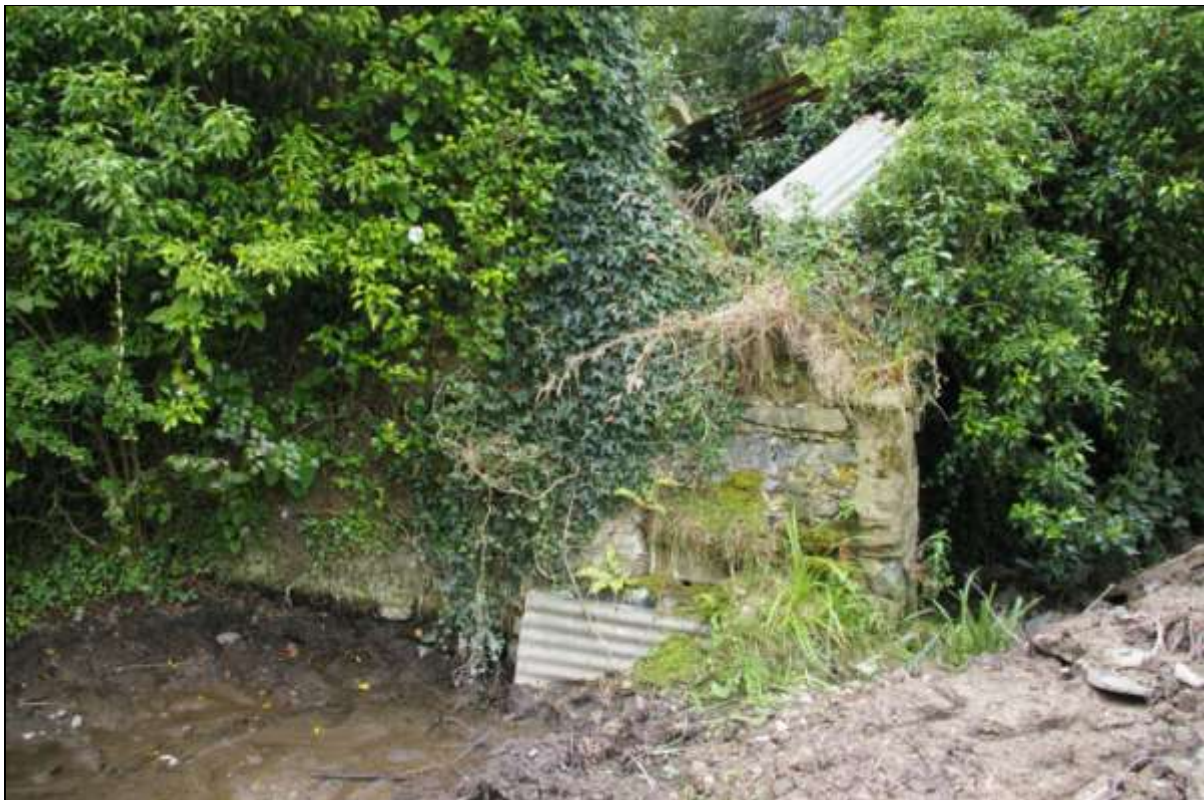
FIGURE 6: BUILDING 6 NORTH-EAST ELEVATION; VIEWED FROM THE NORTH (NO SCALE).
