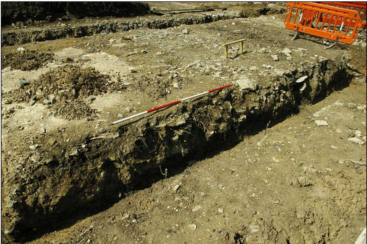
AREA 01 MIDDLE FOUNDATION TRENCH, NORTH-EAST FACING SECTION EAST END, OBLIQUE; VIEWED FROM THE EAST-NORTH-EAST (2M SCALE).
