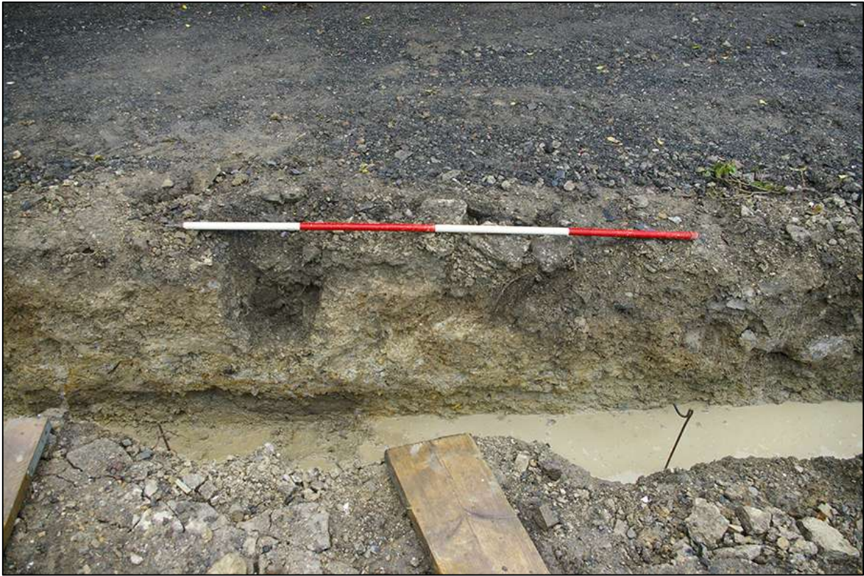
AREA 01 NORTHERN FOUNDATION TRENCH, WALL CUT [145] SOUTH-EAST FACING SECTION; VIEWED FROM THE SOUTH-WEST (2M SCALE).
