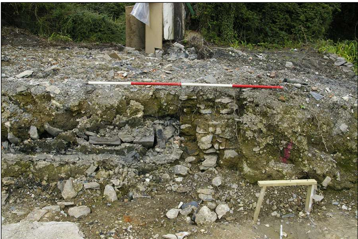
BUILDING 1, DETAIL OF WALL CONSTRUCTION WITH ABUTTING BURNT RUBBLE BACKFILL; VIEWED FROM THE SOUTH-EAST (2M SCALE).
