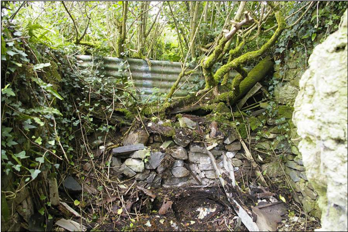
BUILDING 3 INTERNAL NORTH-WEST ELEVATION (EAST WALL); VIEWED FROM THE NORTH-WEST (NO SCALE).
