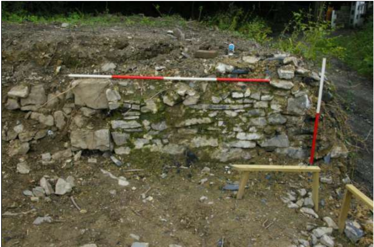
FIGURE 7: WALL 2 SOUTH-EAST ELEVATION, NORTHERN END, SHOWING TWO ABUTTING PHASES OF WALL CONSTRUCTION; VIEWED FROM THE SOUTH-EAST (1M & 2M SCALES).
