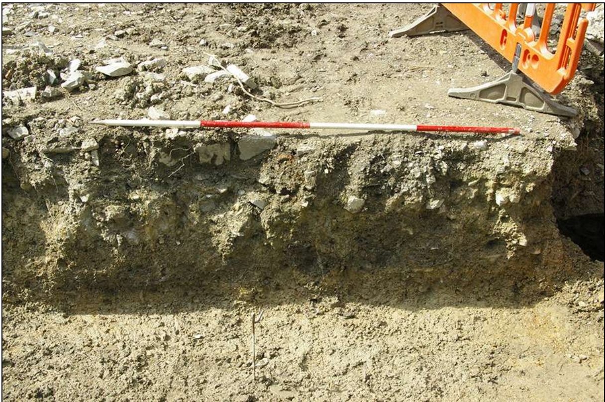
AREA 01 MIDDLE FOUNDATION TRENCH, NORTH-EAST FACING SECTION, MID; VIEWED FROM THE NORTH-EAST (2M SCALE).
