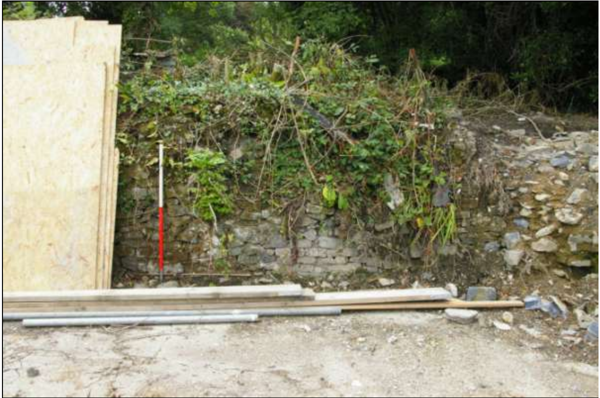
FIGURE 8: WALL 3 NORTH-EAST ELEVATION, WESTERN END; VIEWED FROM THE NORTH-EAST (1M SCALE).
