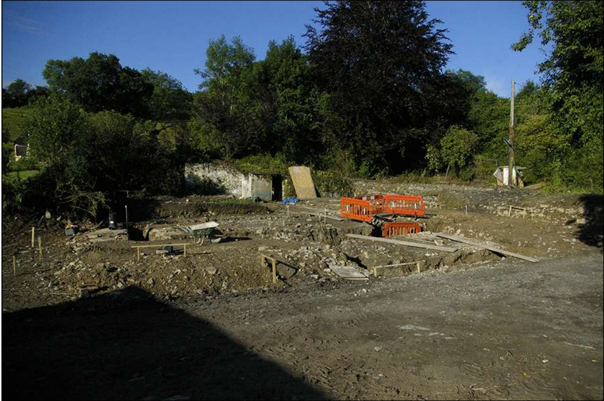
GENERAL SITE SHOT, AREA 01; VIEWED FROM THE NORTH-EAST (NO SCALE).
