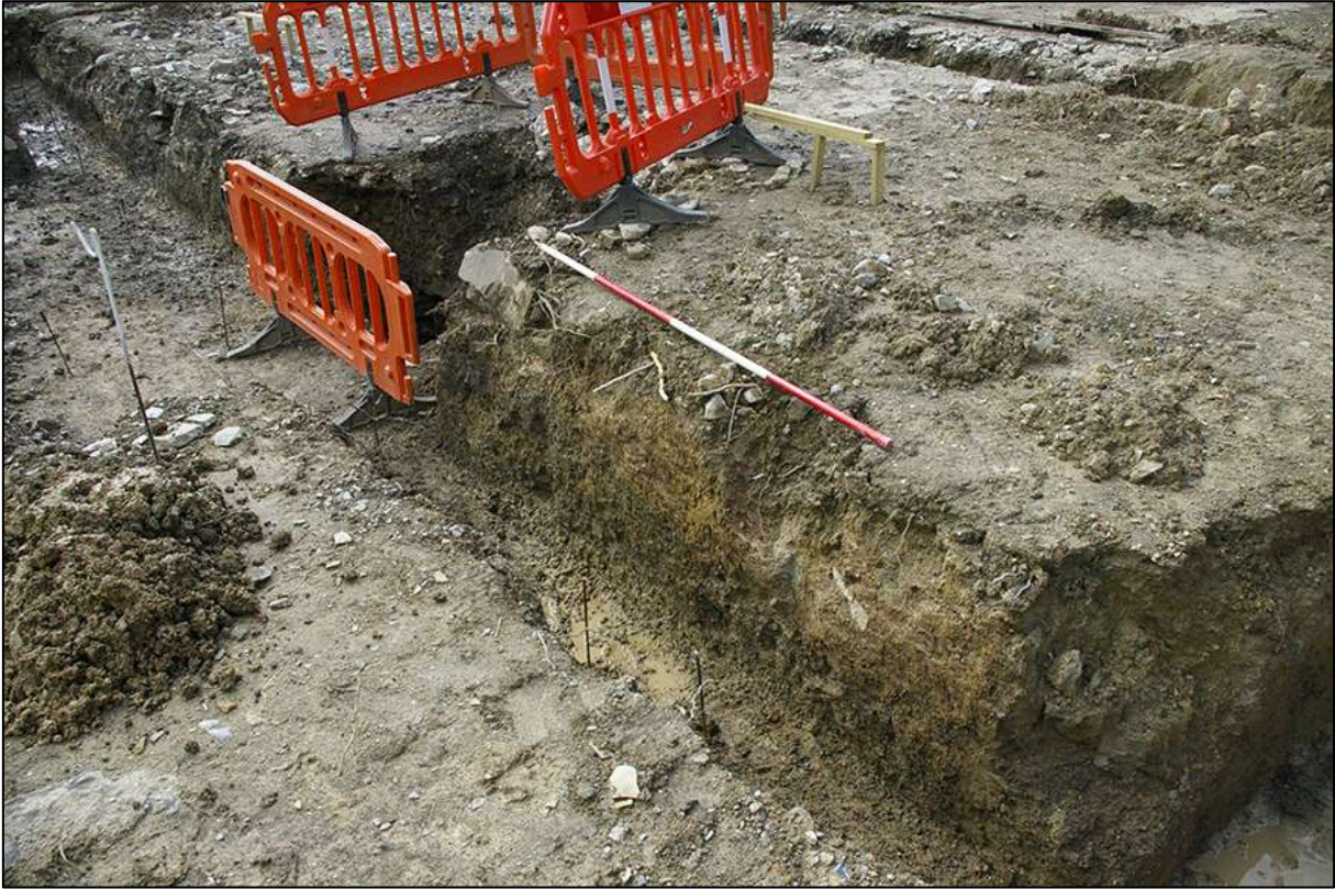
AREA 01 MIDDLE FOUNDATION TRENCH, NORTH-EAST FACING SECTION, WEST END, OBLIQUE; VIEWED FROM THE NORTH-WEST (2M SCALE).
