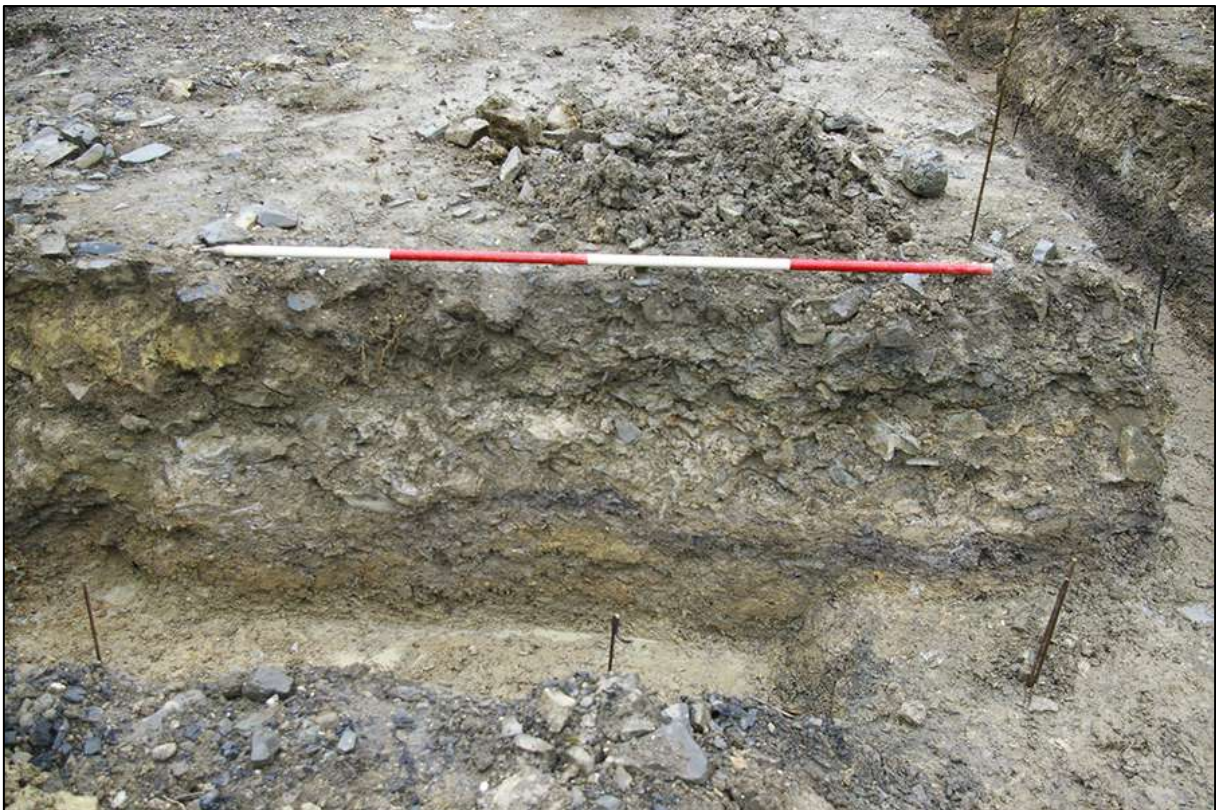
AREA 01 NORTH-EASTERN FOUNDATION TRENCH, NORTH-WEST FACING SECTION, SOUTH END; VIEWED FROM THE NORTH-WEST (2M SCALE).
