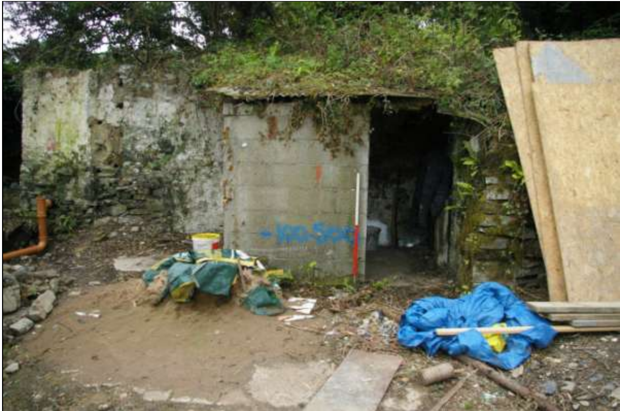
FIGURE 3: BUILDING 2 NORTH-EAST ELEVATION; VIEWED FROM THE NORTH-EAST (1M SCALE).
