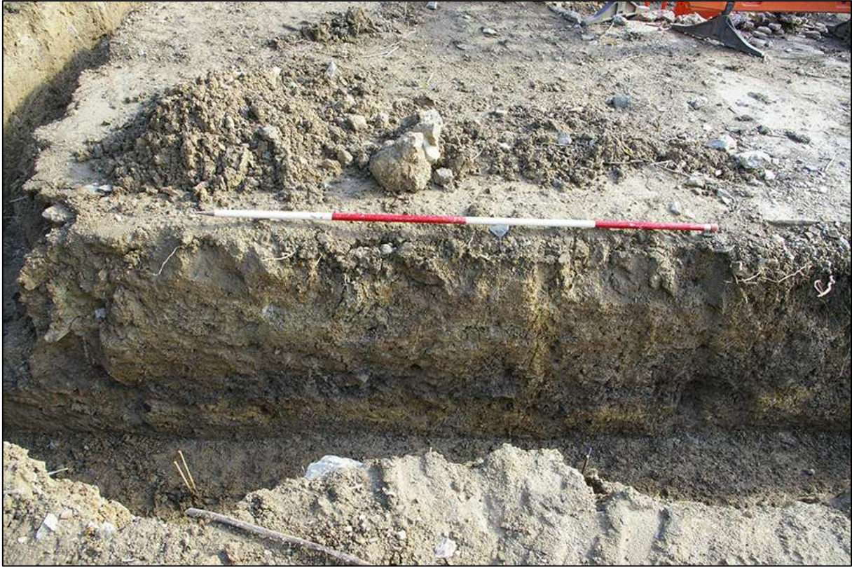
AREA 01, SOUTHERN FOUNDATION TRENCH SOUTH-WEST FACING SECTION, WEST END; VIEWED FROM THE SOUTH-WEST (2M SCALE).
