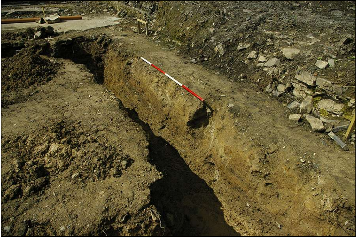
AREA 01 SOUTH-WESTERN FOUNDATION TRENCH, SOUTH-EAST FACING SECTION, OBLIQUE; VIEWED FROM THE NORTH-EAST (2M SCALE).
