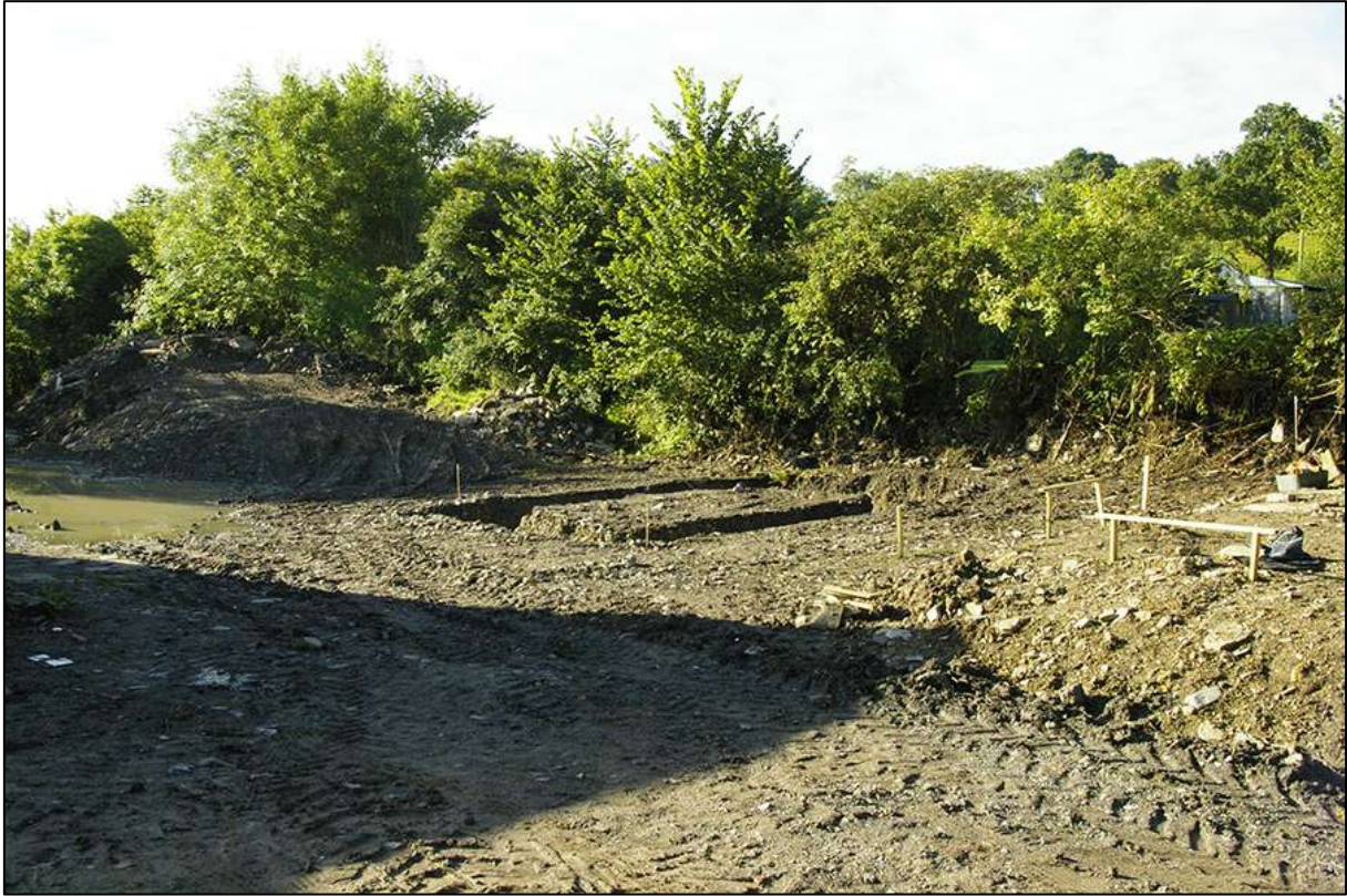
GENERAL SITE SHOT, AREA 02; VIEWED FROM THE NORTH (NO SCALE).
