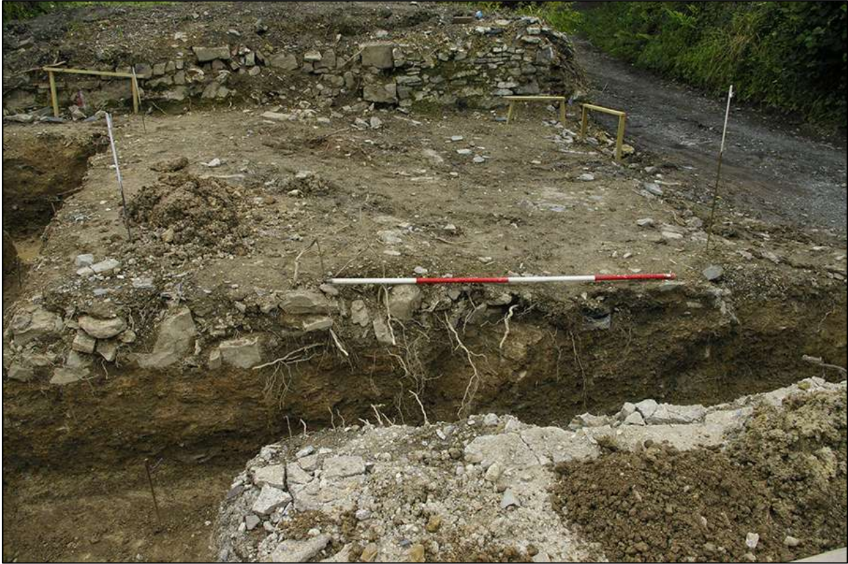
AREA 01 SOUTH-WESTERN FOUNDATION TRENCH, SOUTH-EAST FACING SECTION, NORTH END; VIEWED FROM THE SOUTH-EAST (2M SCALE).
