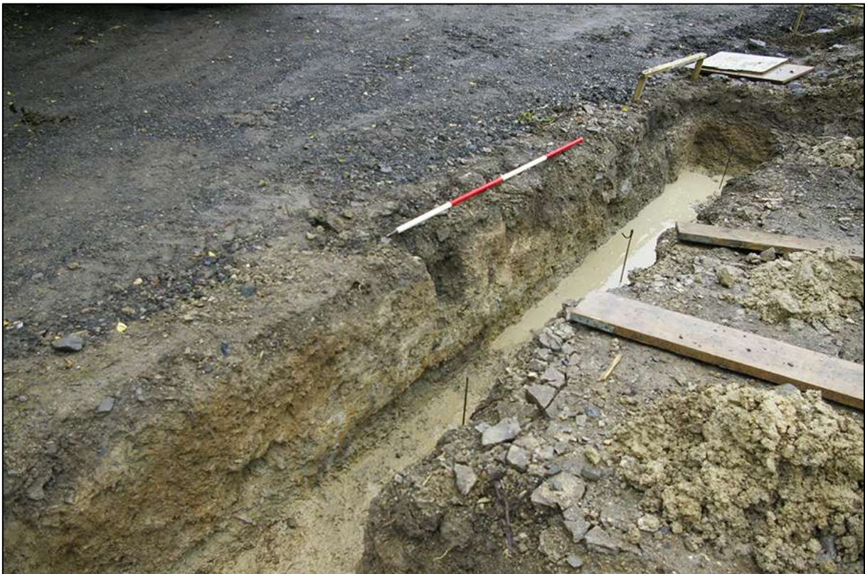
AREA 01 NORTHERN FOUNDATION TRENCH, SOUTH-WEST FACING SECTION, OBLIQUE; VIEWED FROM THE SOUTH-WEST (2M SCALE).
