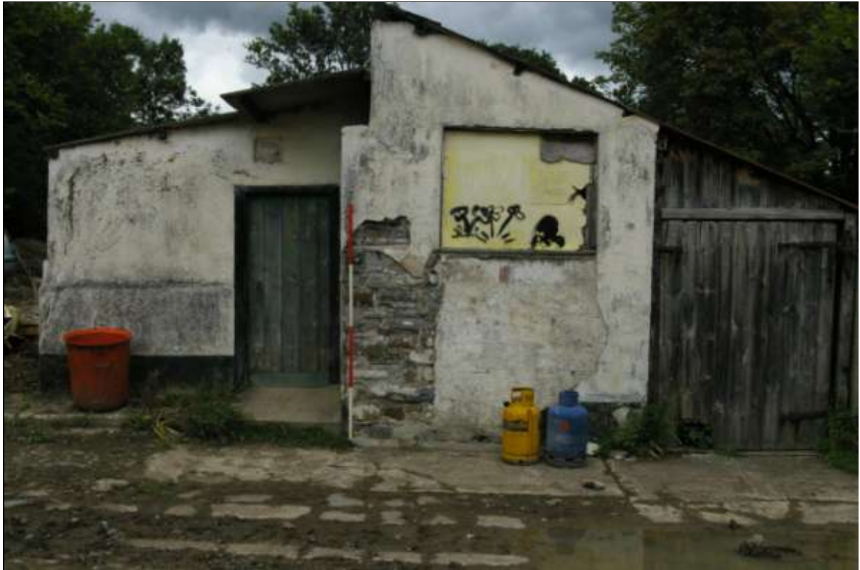
FIGURE 5: BUILDING 5 SOUTH-EAST ELEVATION; VIEWED FROM THE SOUTH-EAST (2M SCALE).
