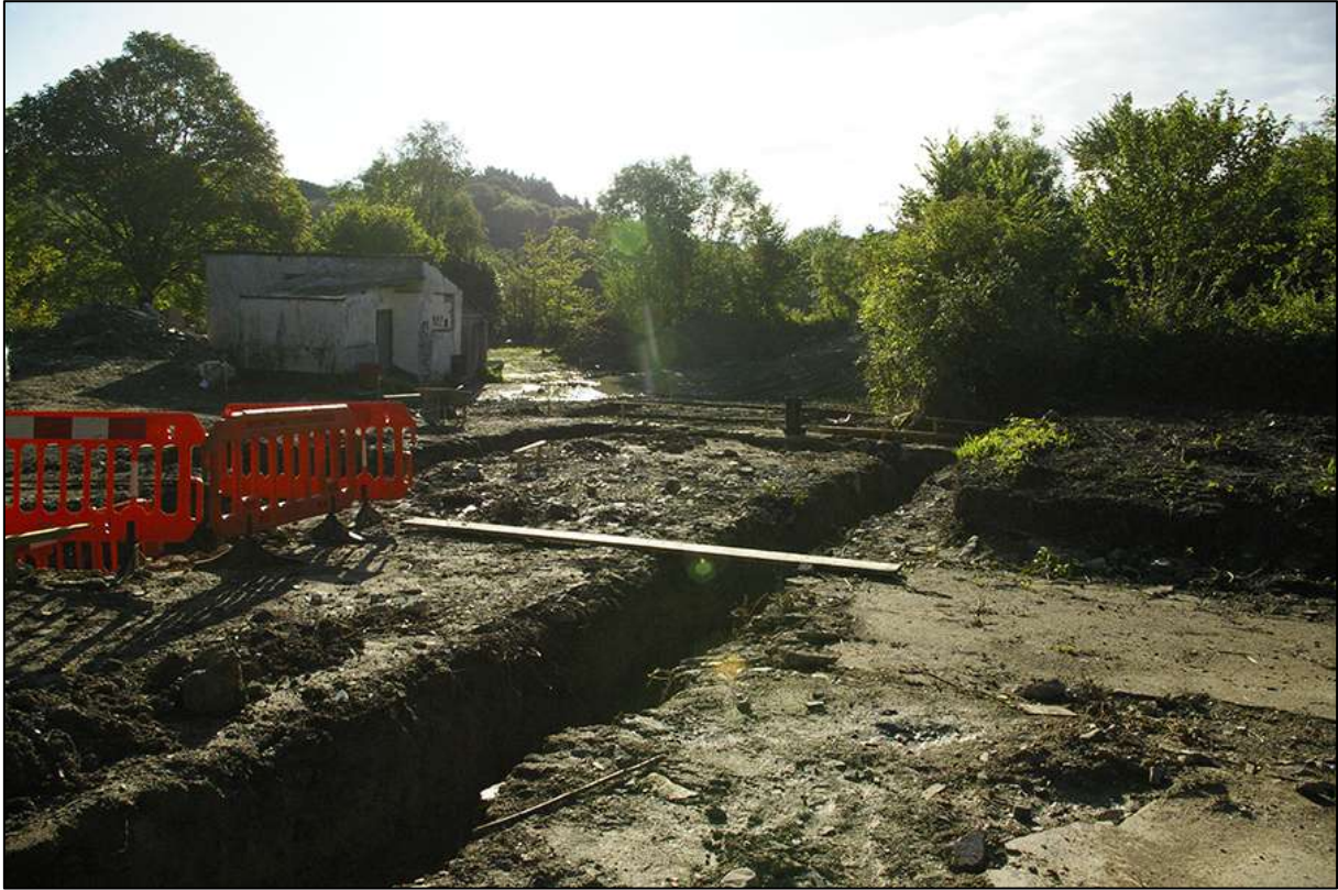
GENERAL SITE SHOT, AREA 01; VIEWED FROM THE SOUTH-WEST (NO SCALE).
