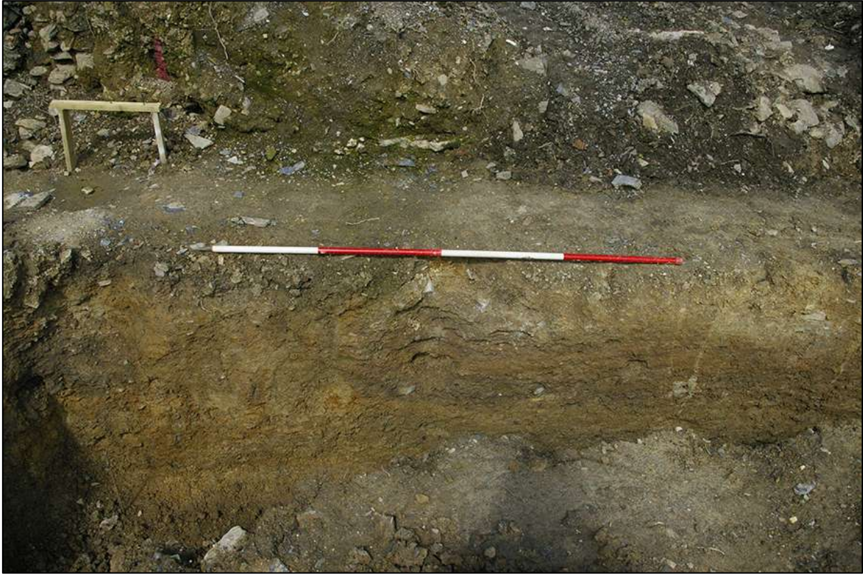
AREA 01 SOUTH-WESTERN FOUNDATION TRENCH, SOUTH-EAST FACING SECTION, SOUTH END; VIEWED FROM THE SOUTH-EAST (2M SCALE).
