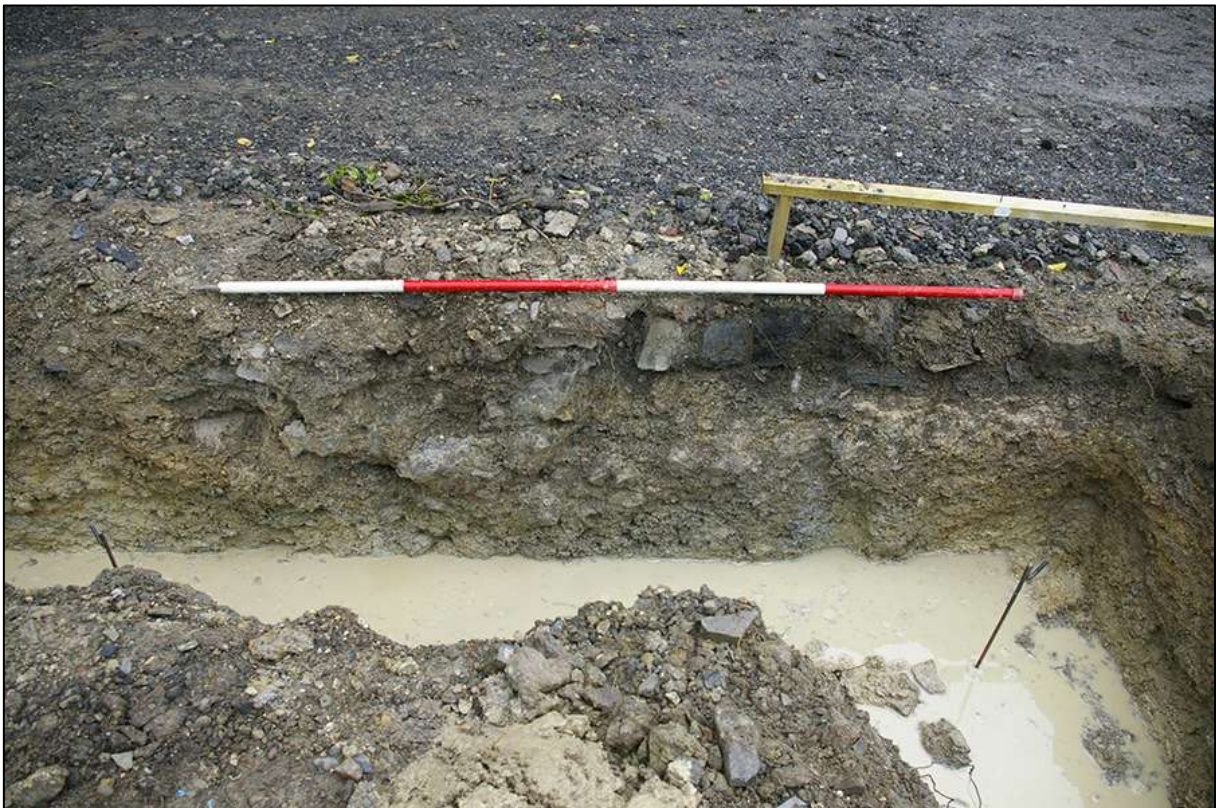
AREA 01 NORTHERN FOUNDATION TRENCH, SOUTH-WEST FACING SECTION, EAST END; VIEWED FROM THE SOUTH-WEST (2M SCALE).
