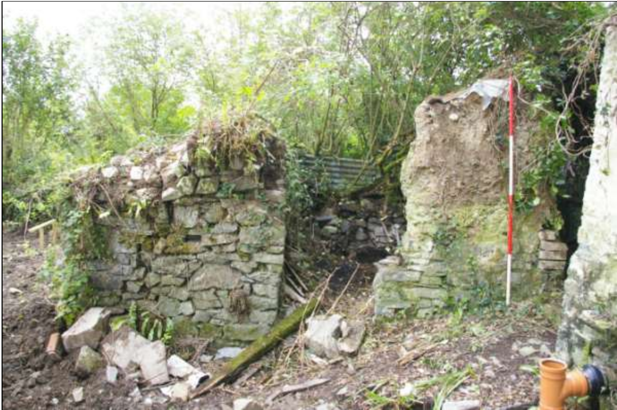
FIGURE 4: BUILDING 3 NORTH-WEST ELEVATION; VIEWED FROM THE NORTH-WEST (2M SCALE).
