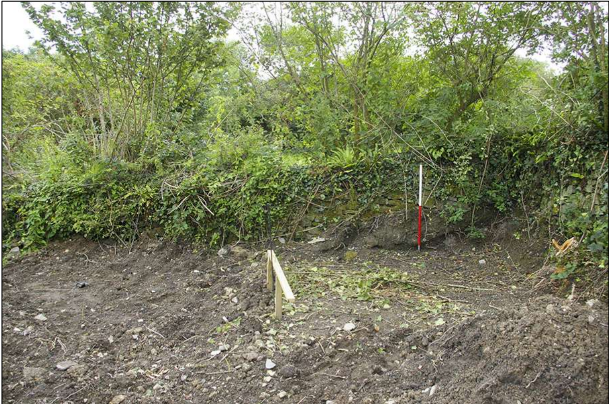
WALL 5 NORTH-WEST ELEVATION OF NORTH RETURN AT EAST END; VIEWED FROM THE NORTH-WEST (1M SCALE).
