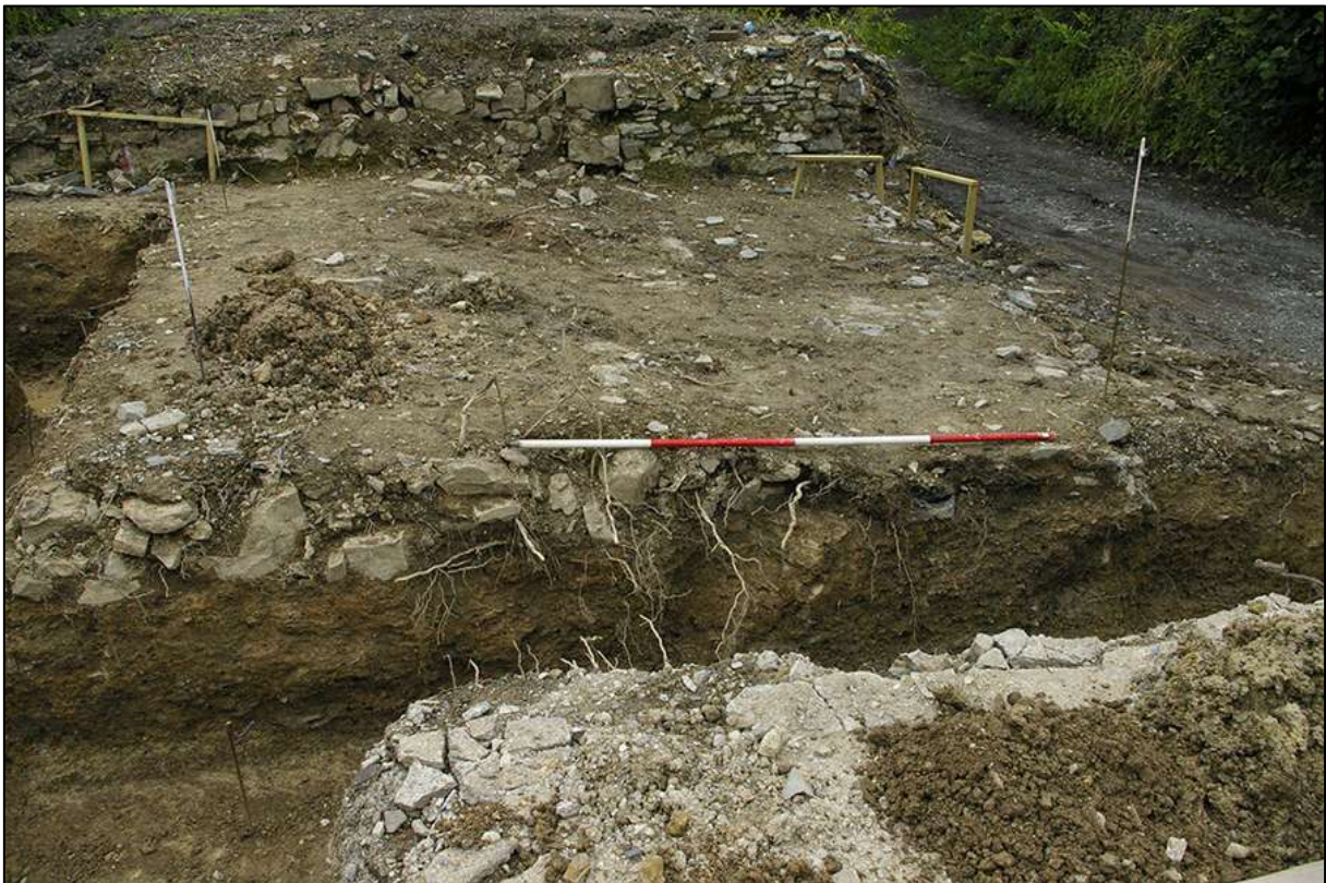
AREA 01 NORTH-WESTERN FOUNDATION TRENCH, SOUTH-EAST FACING SECTION, OBLIQUE; VIEWED FROM THE SOUTH-SOUTH-EAST (2M SCALE).
