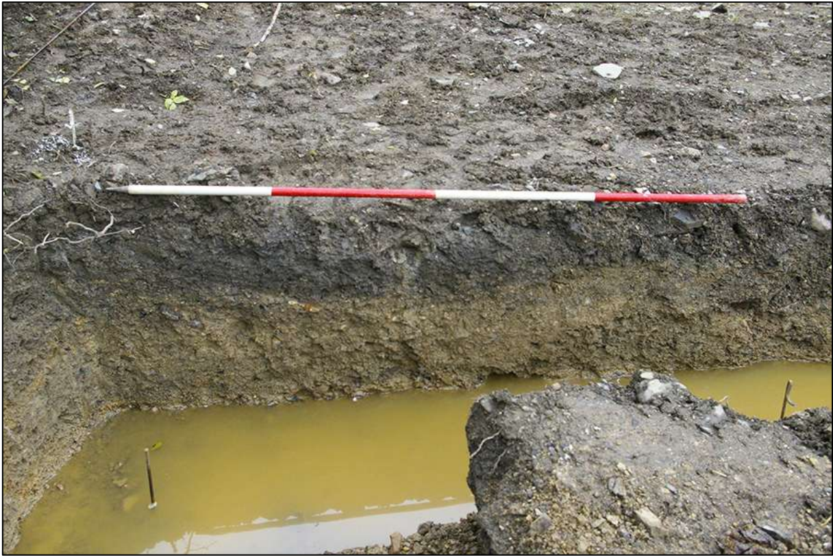
AREA 02 WESTERN FOUNDATION TRENCH, SOUTH-EAST FACING SECTION, SOUTH END; VIEWED FROM THE SOUTH-EAST (2M SCALE).
