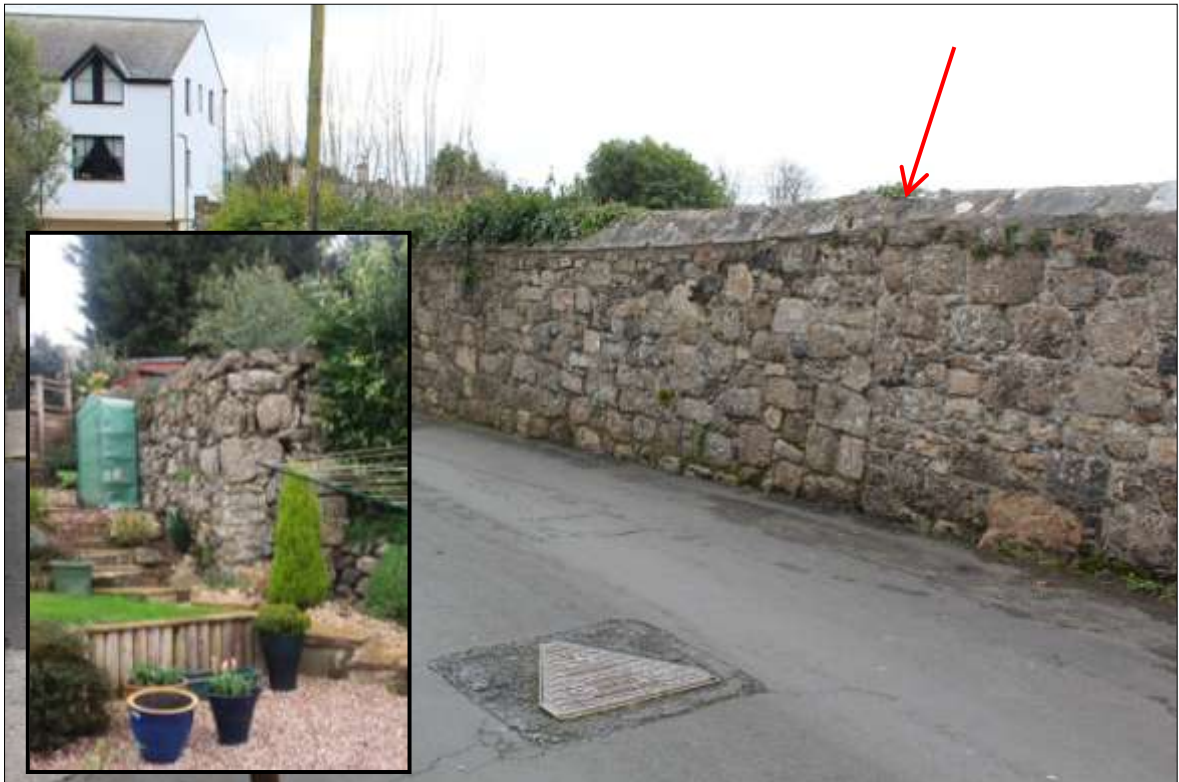
FIGURE 11: THE EAST WALL OF THE GRAVEYARD SHOWING A BREAK IN BUILD (INDICATED), VIEWED FROM THE NORTH , WITH AN INSET SHOWING THE WALL IN THE BACK GARDEN OF A PROPERTY ON ABBEY ROAD (COURTESY OF F BILLINGE).
