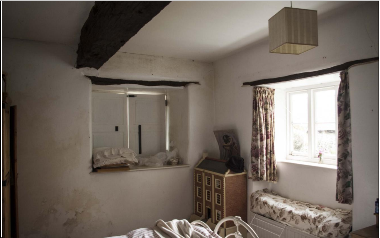
View of the forced window to the east and a further window to the south set within larger blocked opening, in the south-east corner of the east range, within the small bedroom; from the west-north-west.
