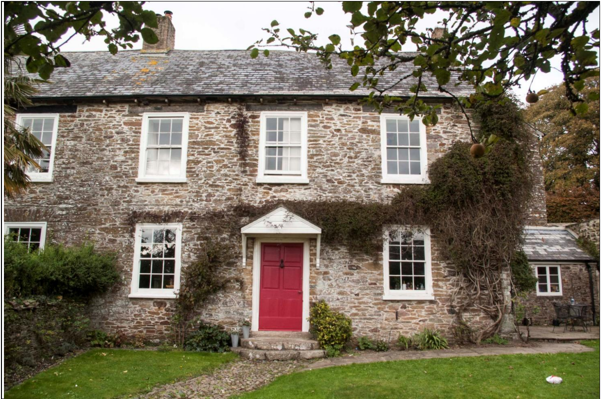
Figure 6: The south front elevation of Old Traine, the eastern of the two dwellings formed from the former hall range in c.1800; from the south.
