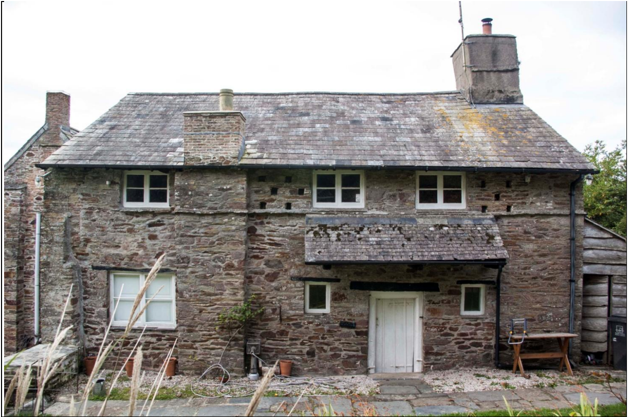
Figure 7: The east elevation of the east range; from the east.
