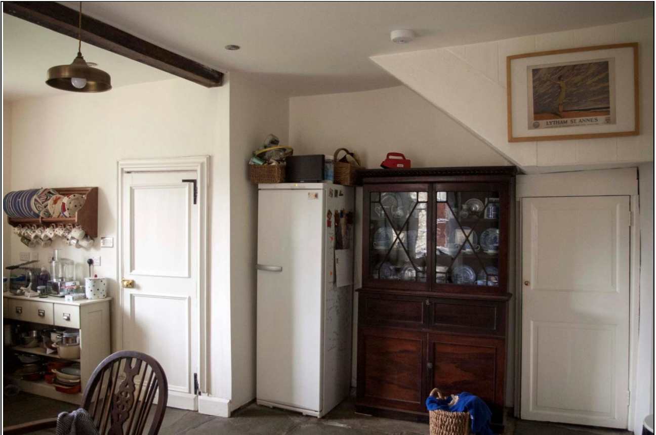
View of the kitchen in the south range, with reused two panel 17 th century door to under stair cupboard and a reset bolection moulded door and frame to the hallway; from the north-east.
