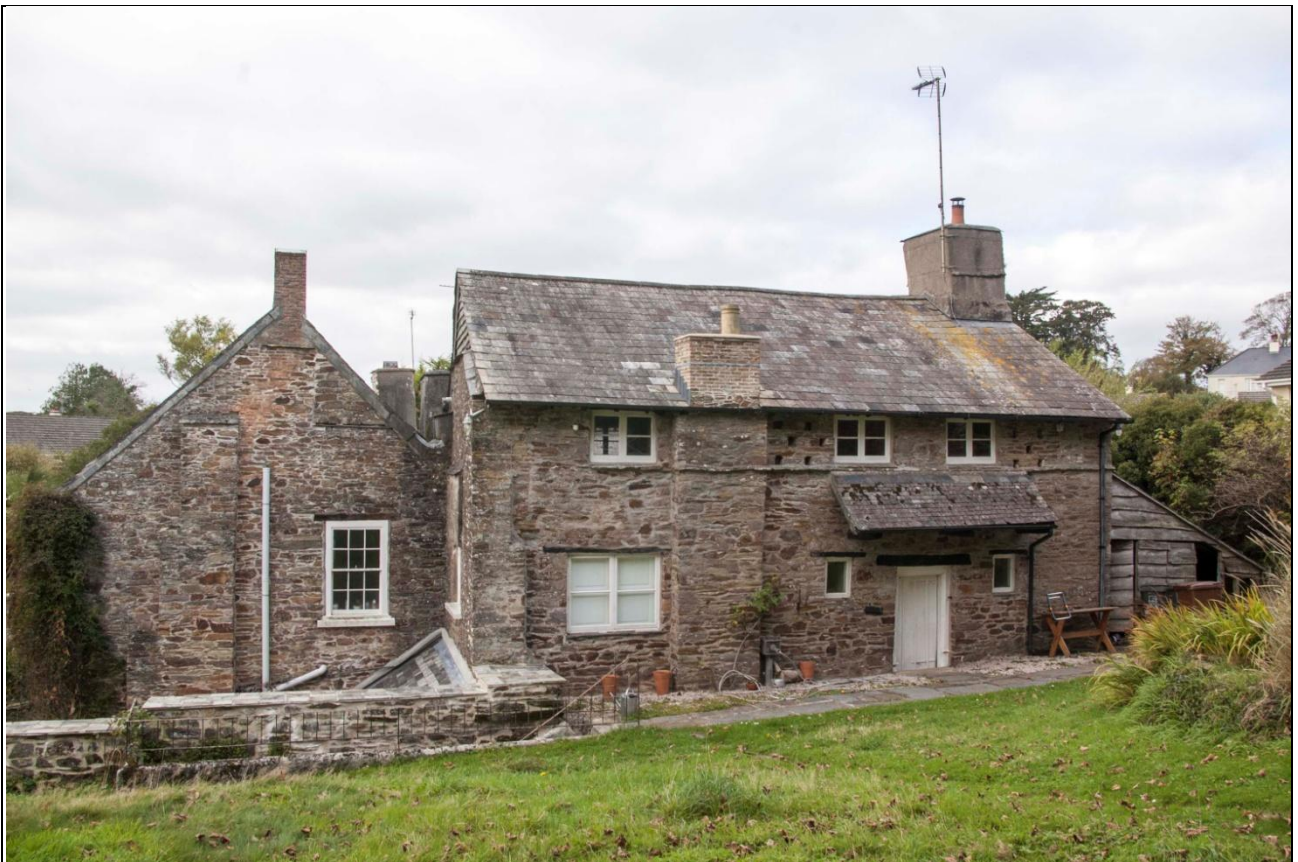
View of the relationship between the east elevation of the east range that of the south range; from the east-south-east.
