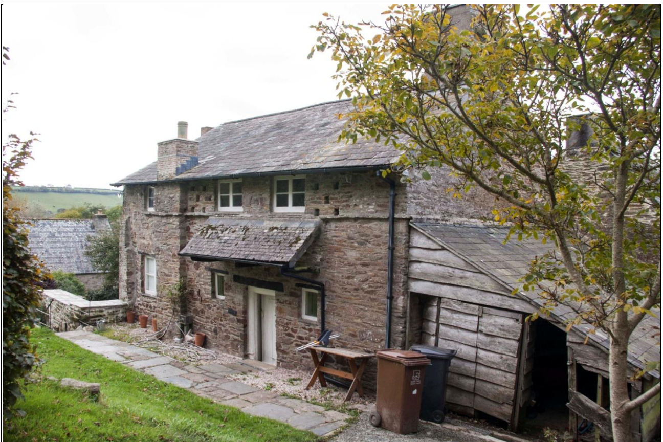
The east elevation of the east range, showing porch, which incorporates surviving sections of pentice, with drip course above, showing it formally ran almost the entire length of the elevation; from the north-east.
