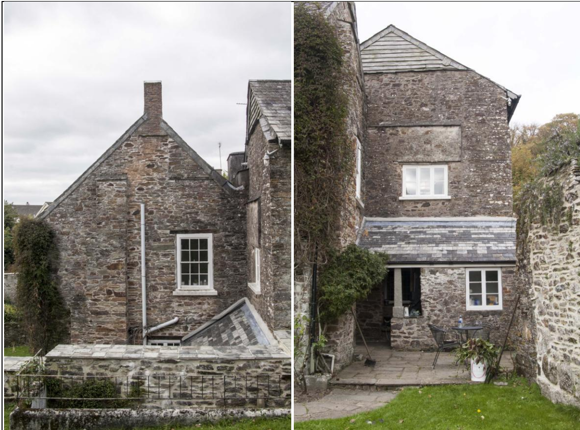
Left: View of the east end of the south range, viewed over the former east wall, now within the garden, showing the truncation of this range in the c.1800 rebuild; from the east.
