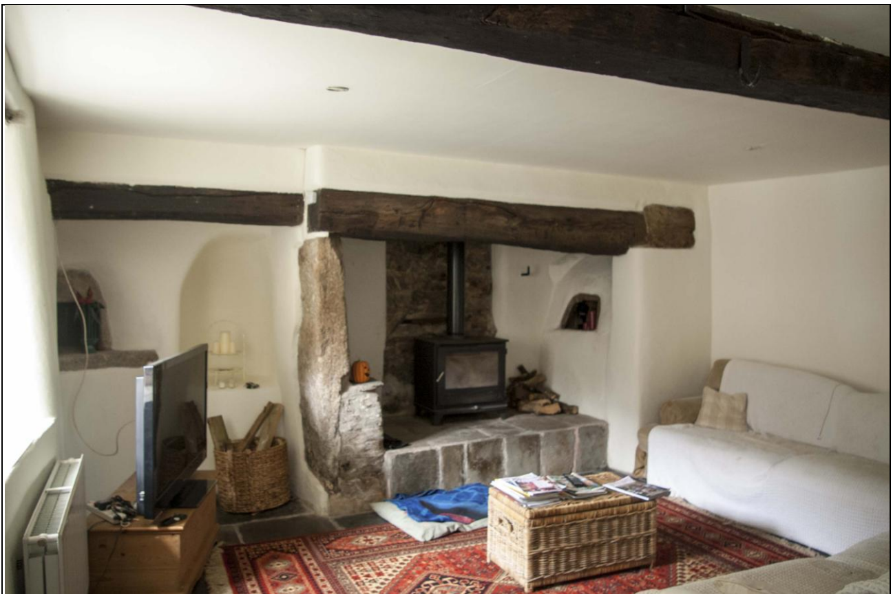
The hearth, ovens and smoke chamber, of 17 th century date, in the north wall of the east range, note the massive cut off beam to the east side, suggestive of an earlier (medieval) open smoke bay.
