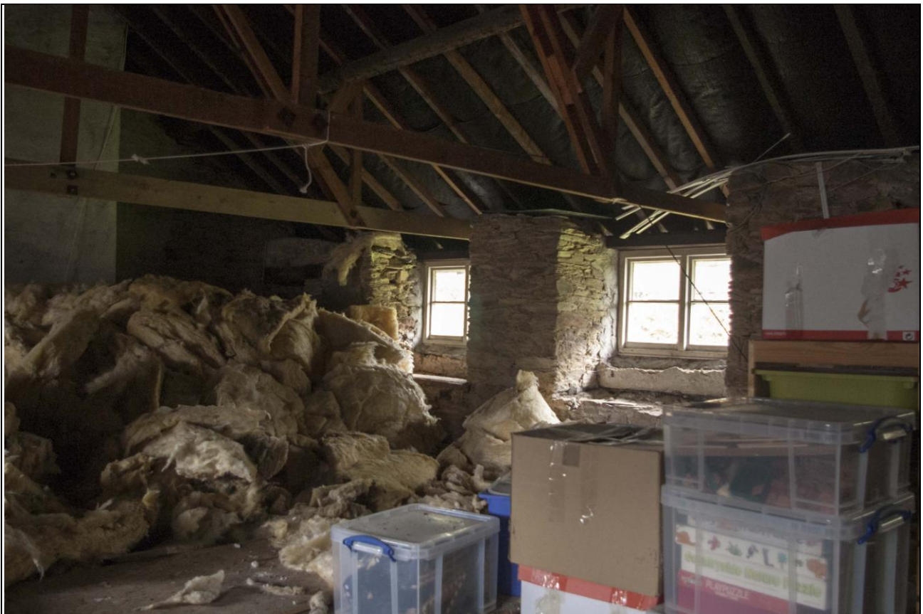
View of the inserted later casements, on the second floor of the east range, showing the conversion from storage to servant accommodation, probably in c.1800; from the south-west.
