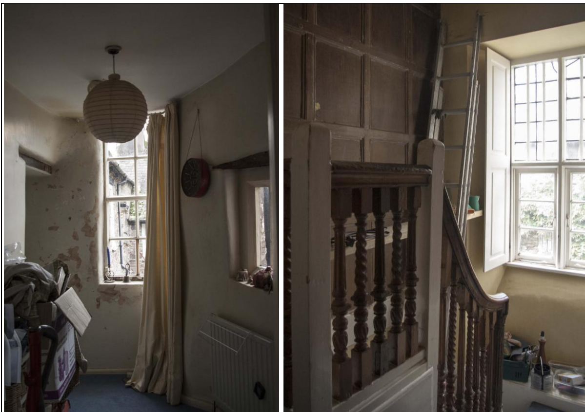
Left: View of the east stair turret at first floor level, opened up, with stair removed; from the east. Right: View of the first floor landing in the south range, with sections of fine moulded handrail and turned balusters of 18 th century date, set within a later plain frame of c.1800, with basic chamfered block newel posts. Once belonging to a grand stair, now removed or reset, possibly not even original to the house; from the south-east.
