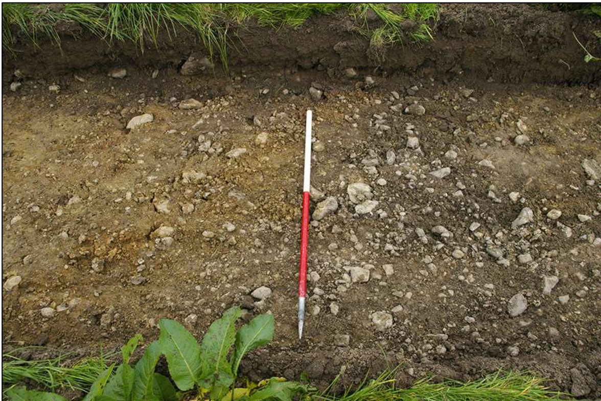
DRAINS [315], [317]; VIEWED FROM THE SOUTH-EAST (1M SCALE).
