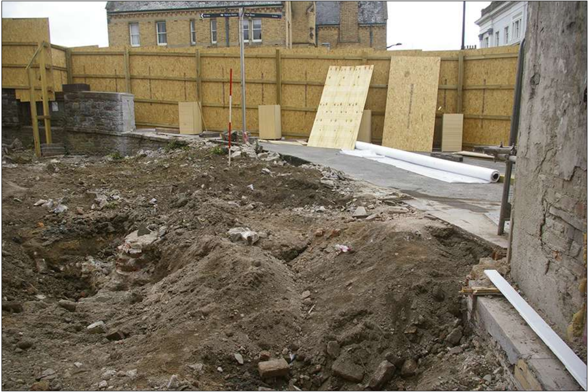
29. AREA 06, PRE-EXCAVATION, NORTH END; FROM THE SOUTH-EAST (2M SCALE).
