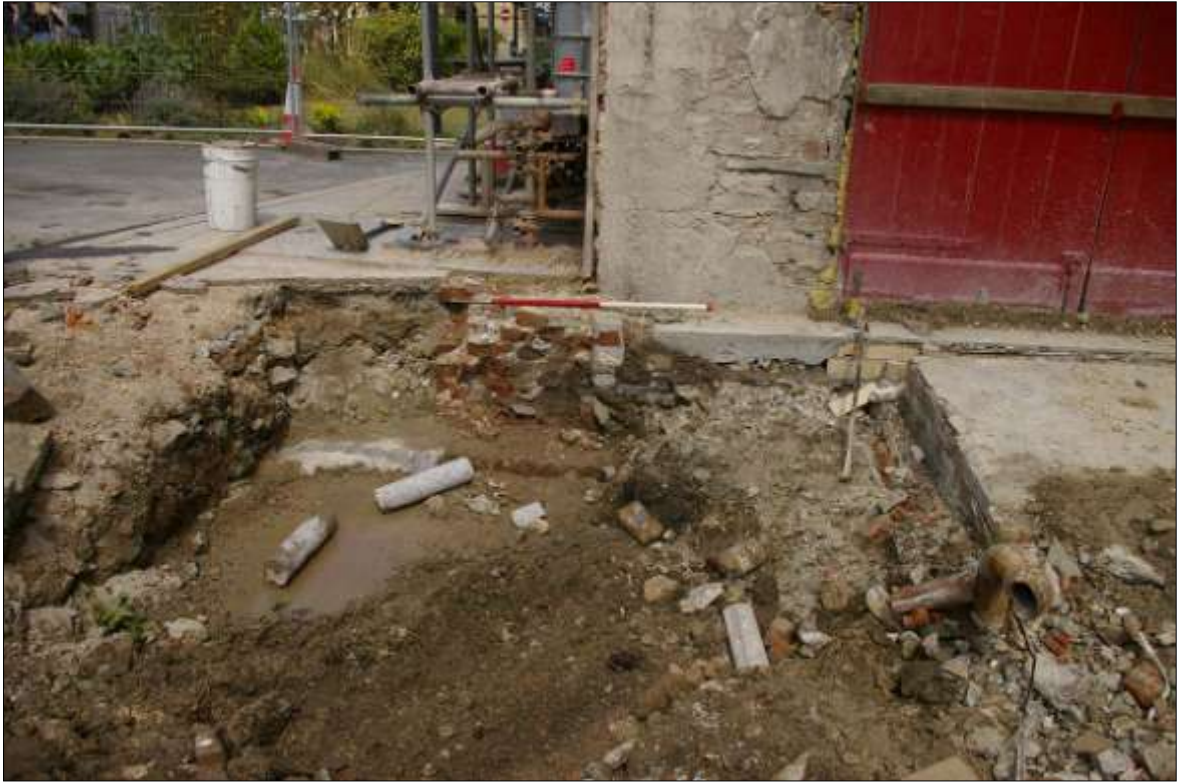
17. AREA 04B, WALL {521}, SOUTH-WEST FACING PROFILE; FROM THE SOUTH-WEST (1M SCALE).
