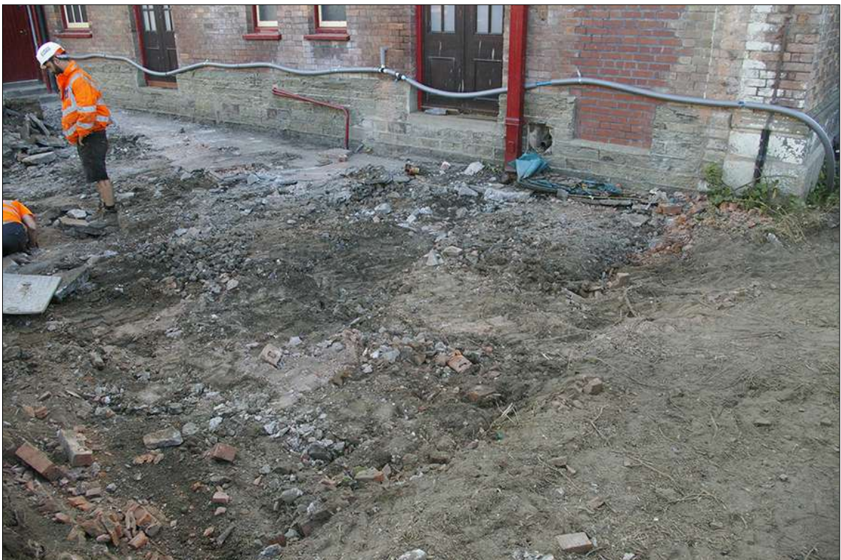
2. GENERAL SITE VIEW SHOWING DEMOLITION WORKS; FROM THE SOUTH-WEST (NO SCALE).
