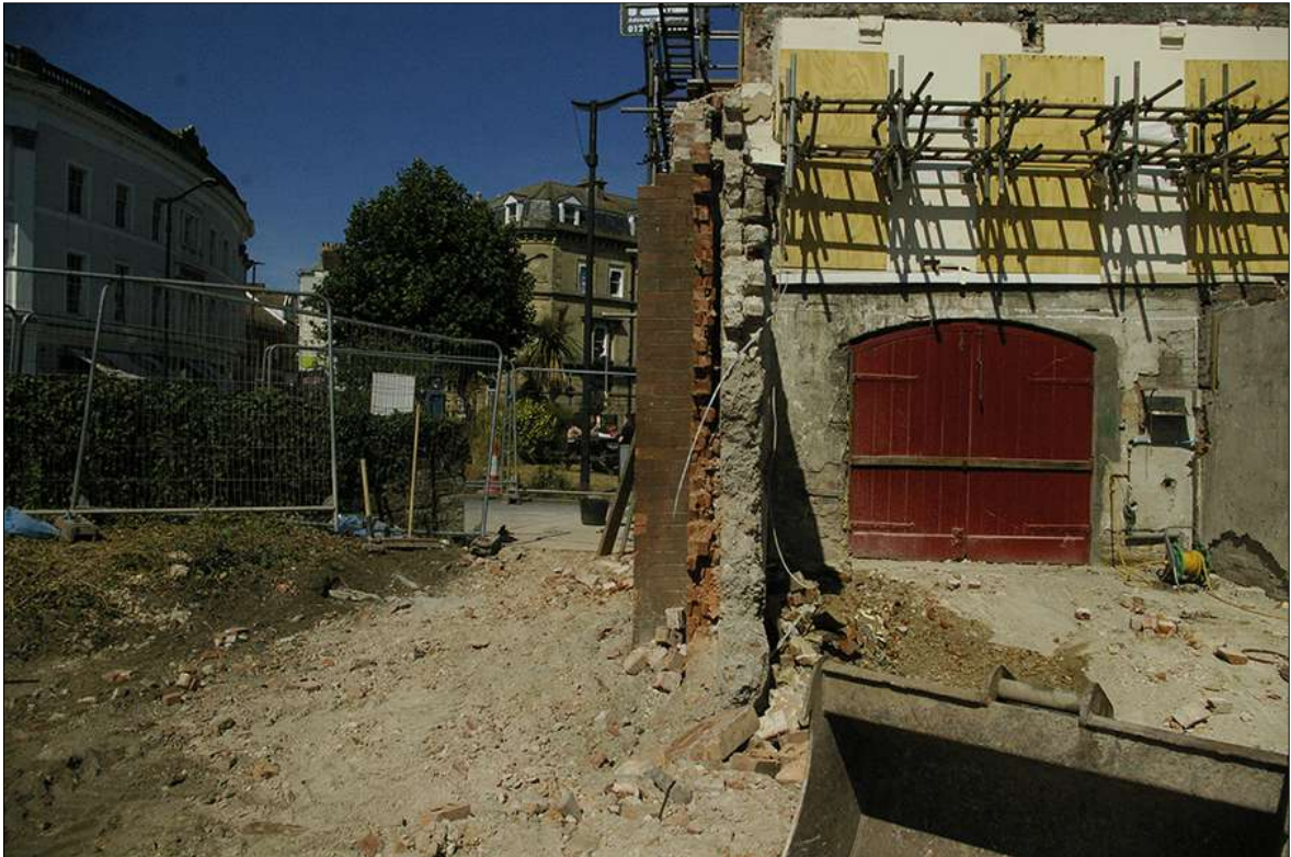
12. AREA 04B, WALL {521} SHOWING BRICK SKIN {457}; FROM THE SOUTH-WEST (NO SCALE).
