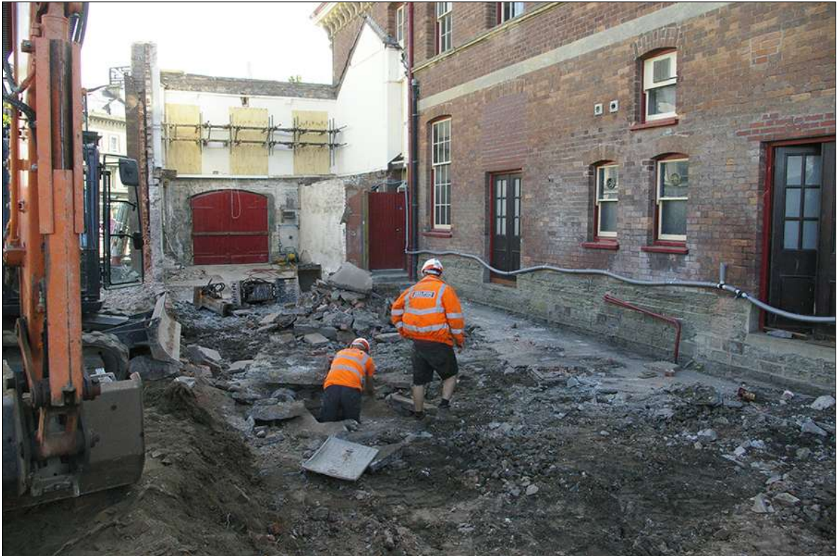
1. GENERAL SITE VIEW SHOWING DEMOLITION WORKS; FROM THE SOUTH-WEST (NO SCALE).
