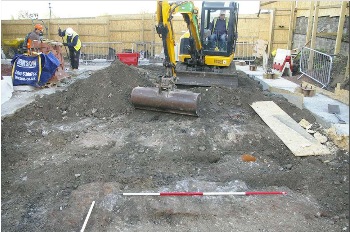
42. AREA 06, WORKING SHOT, SHOWING WALL {490}; FROM THE NORTH-EAST (2M SCALE).
