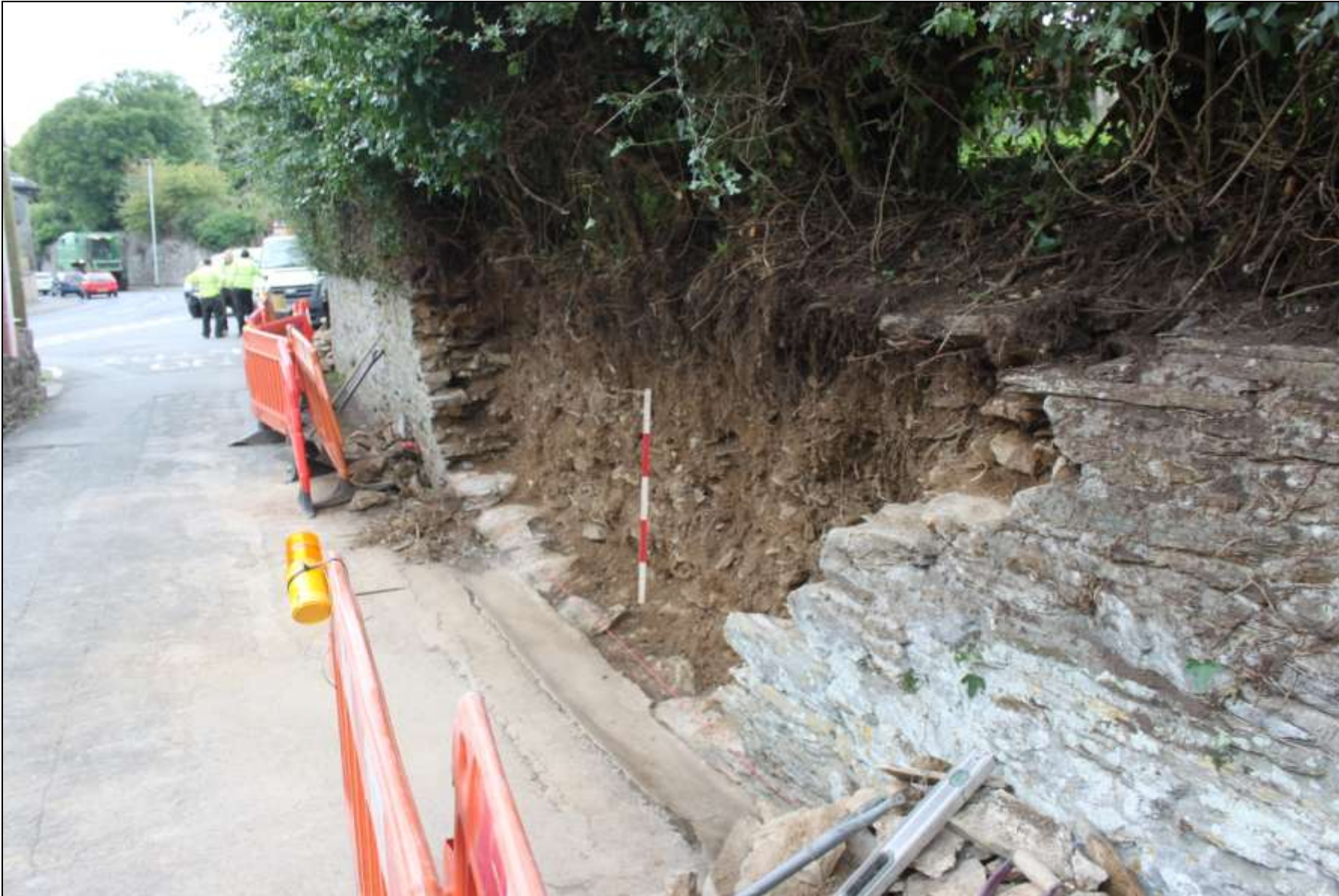
Figure 3: Full extent of wall removal, viewed from the south-east (1m scale).
