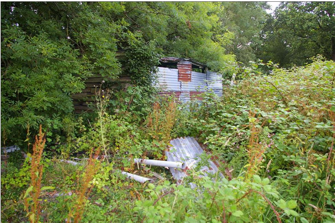
24. DETAIL OF THE SURVIVING SHED STRUCTURE AT THE EASTERN EDGE OF F5; VIEWED FROM THE NORTH-WEST.
