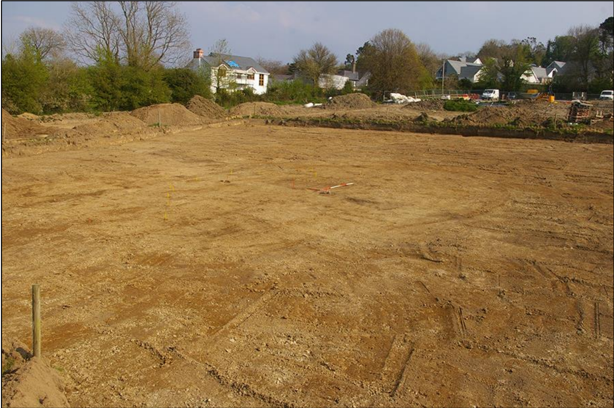
2. AREA 18, PRE-EXCAVATION; VIEWED FROM THE NORTH-WEST (1M & 2M SCALES).
