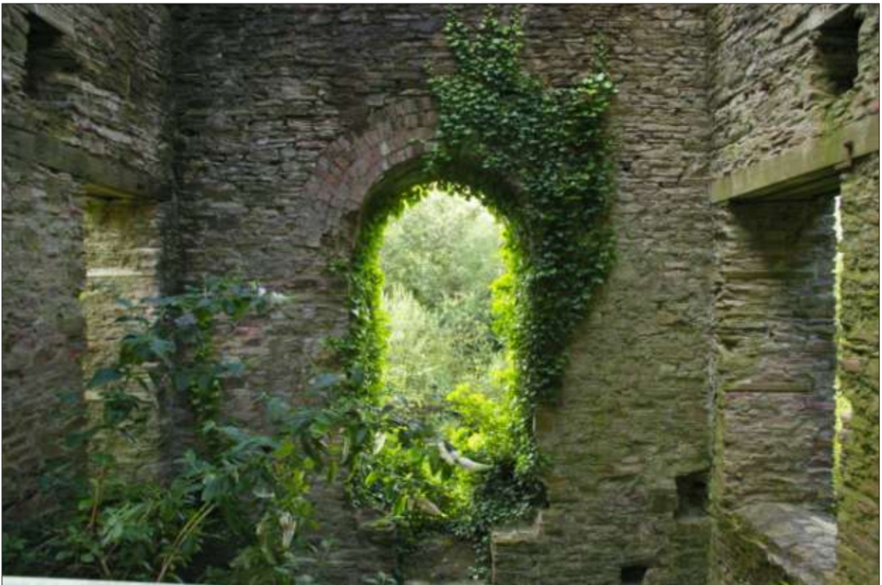
View towards the site from the inside of the pumping engine house, showing screening from trees; viewed from the north.
