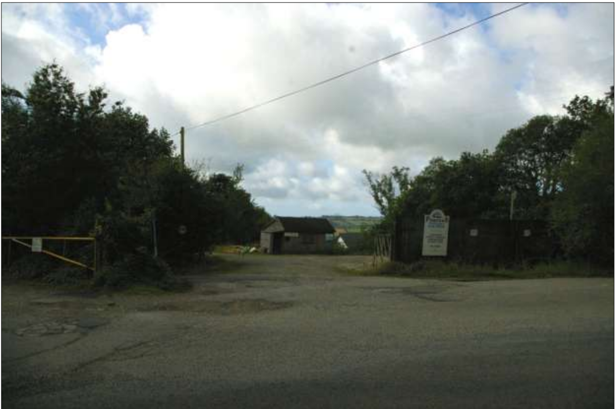
Some of the light industrial units on the developed part of The Prince of Wales Mine; viewed from the north.
