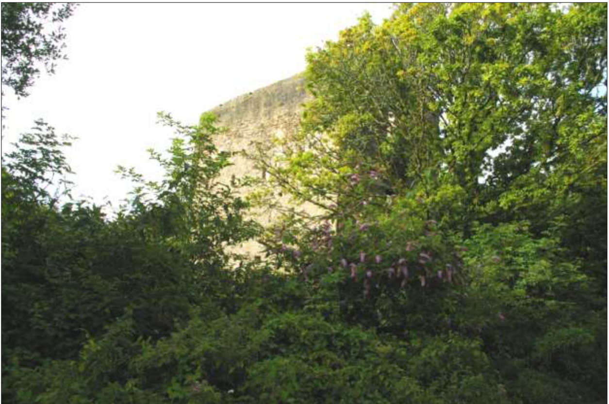
Detail of the pumping engine house, showing the trees and undergrowth; viewed from the north-east.
