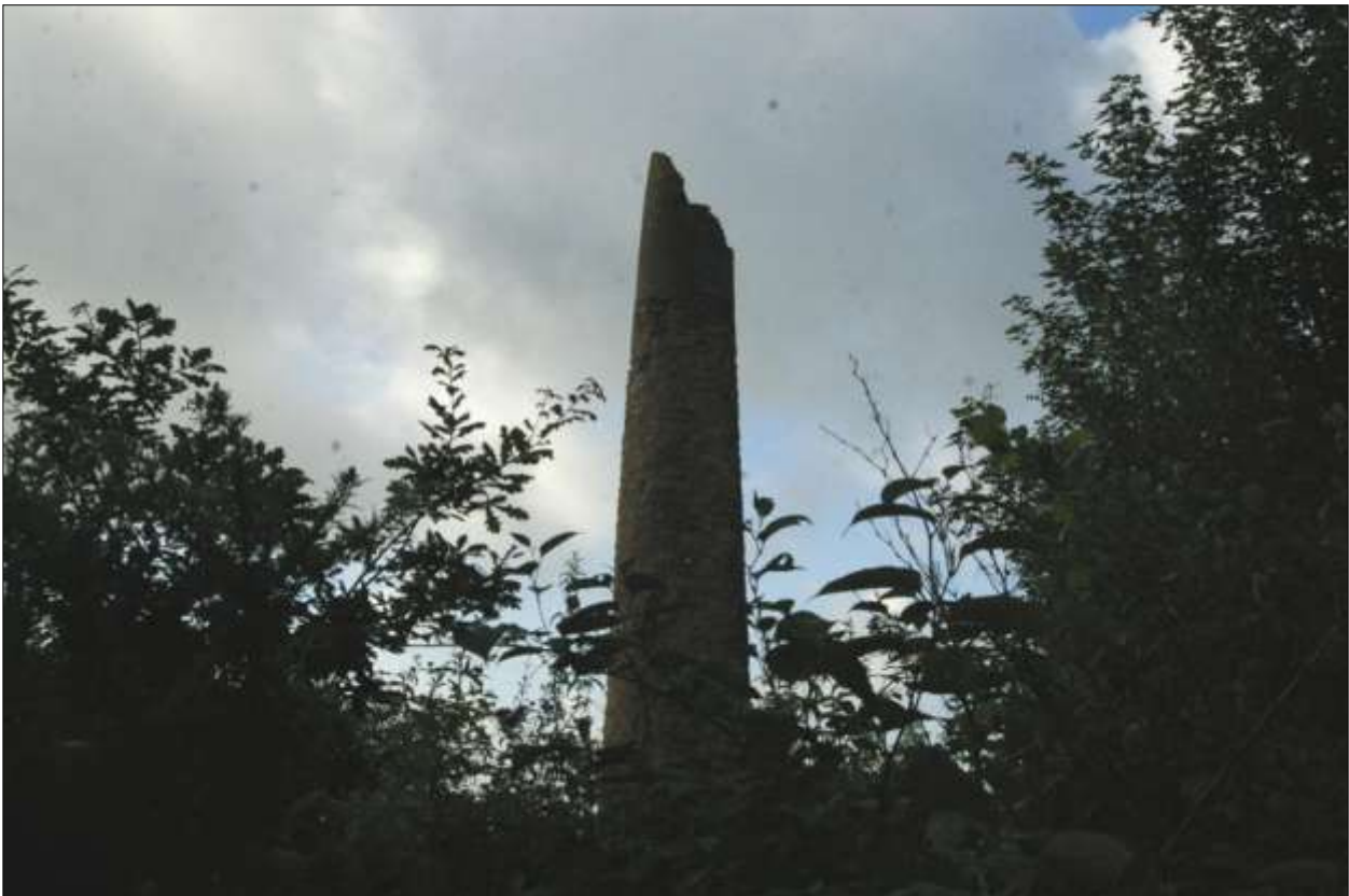
View of the stamps engine house chimney; viewed from the north-north-west.
