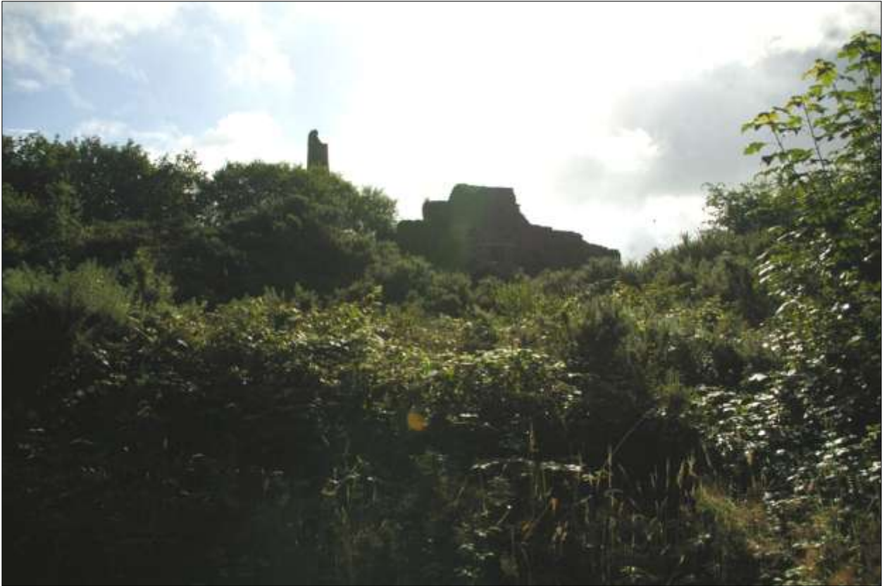
View of the stamps engine house and chimney, showing the trees and undergrowth; viewed from the north-west.
