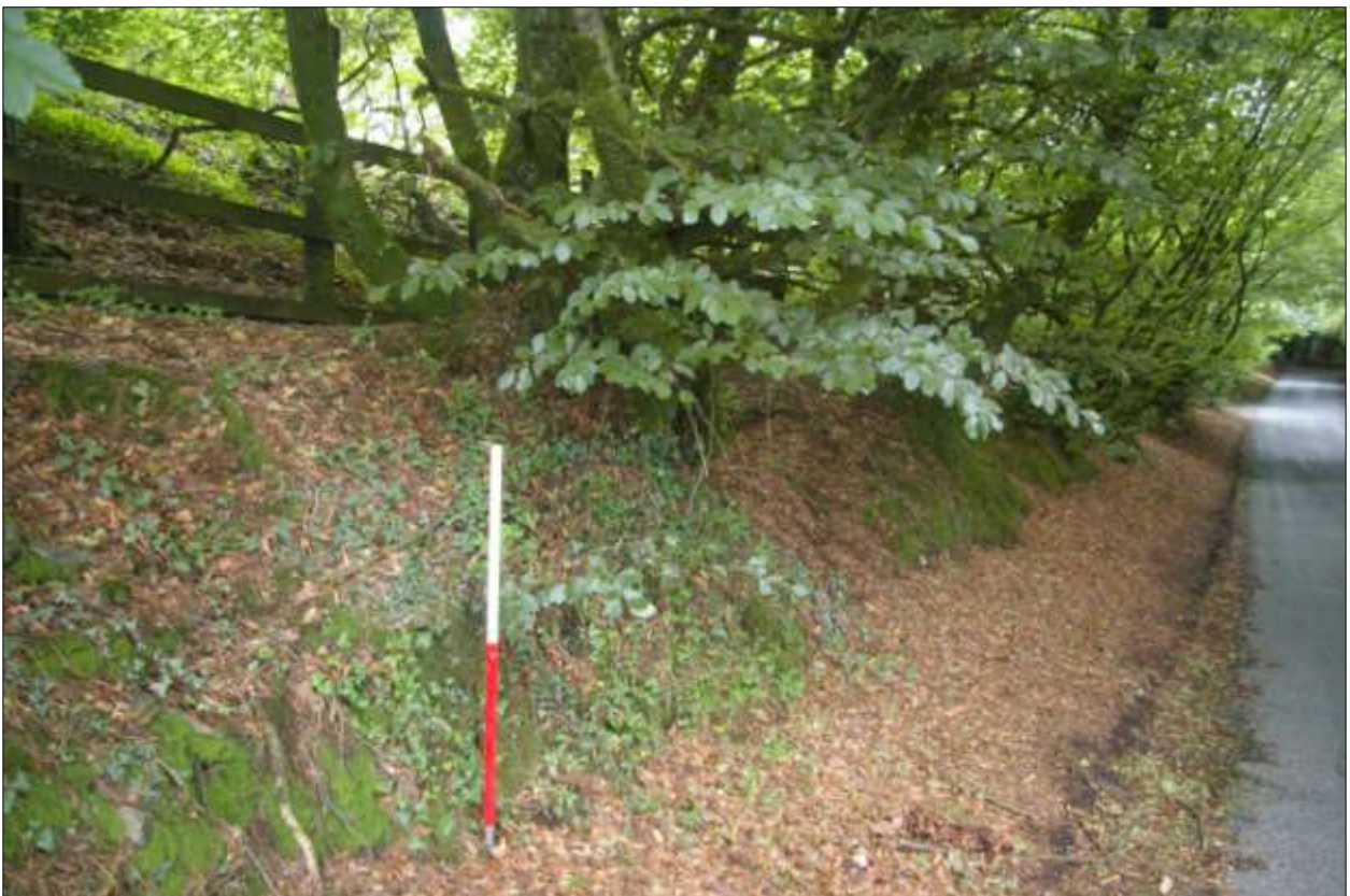
The roadside bank at the southern boundary of The Prince of Wales Mine SAM; viewed from the south-west (1m scale).
