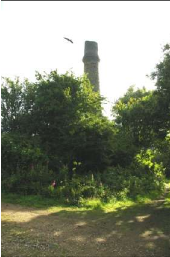
Views of the pumping engine house chimney; viewed from the south-west.
