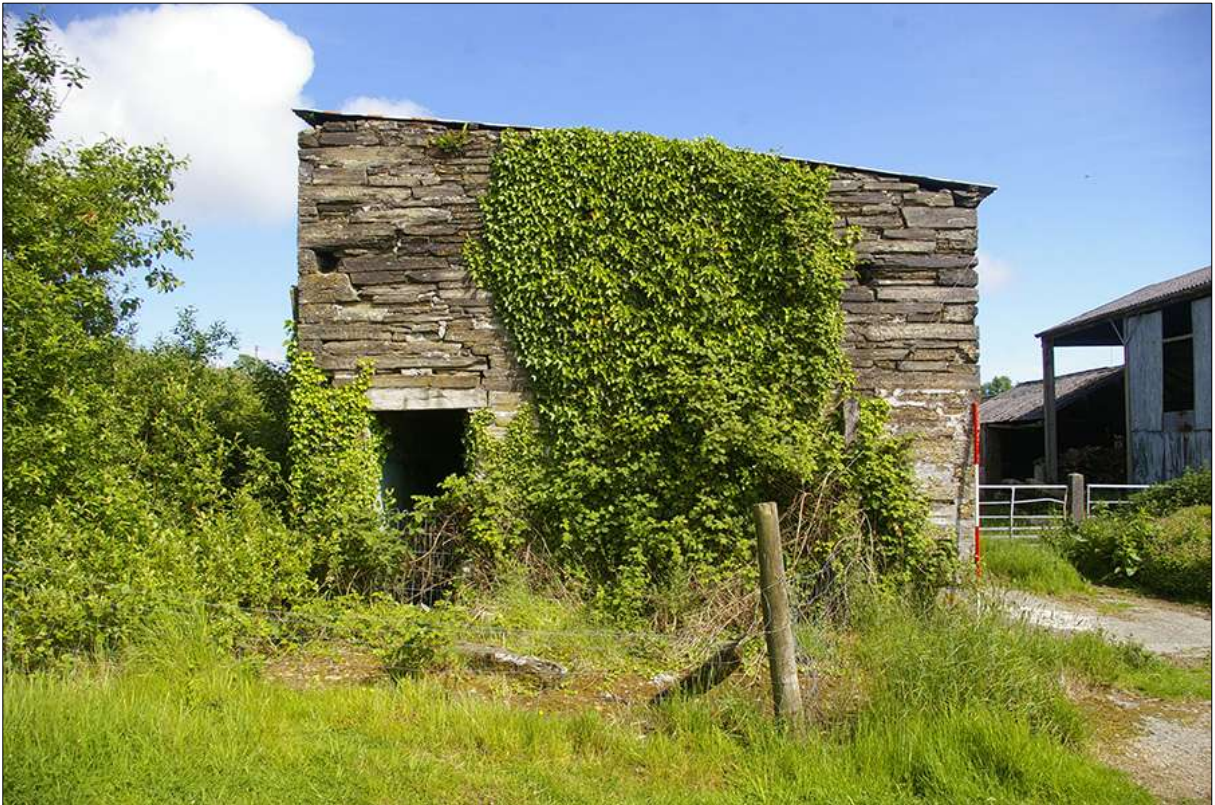
As above; viewed from the north-west, looking south-east (scale 2m).
