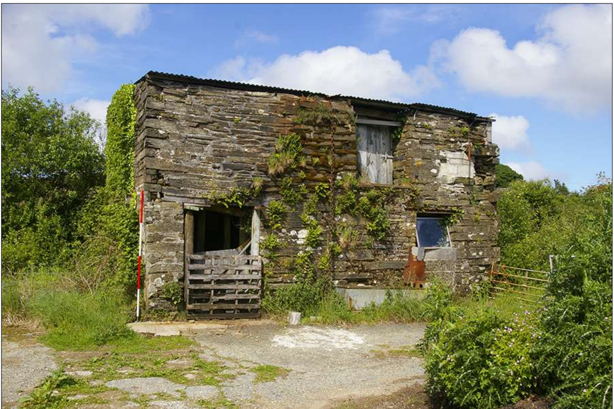
The late 19 th century historic stone-rubble barn beyond the eastern edge of the site; viewed from the south-west, looking north-east (scale 2m).
