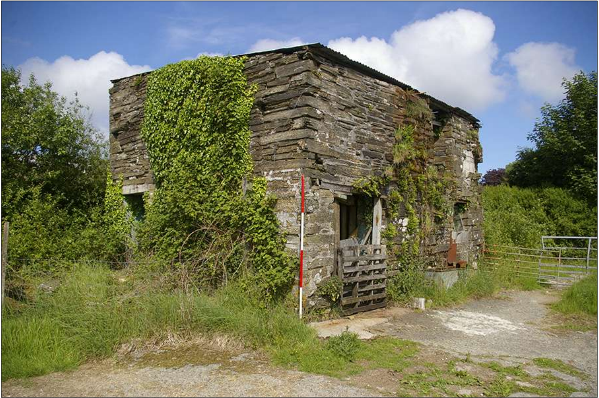
As above; viewed from the west, looking east (scale 2m).
