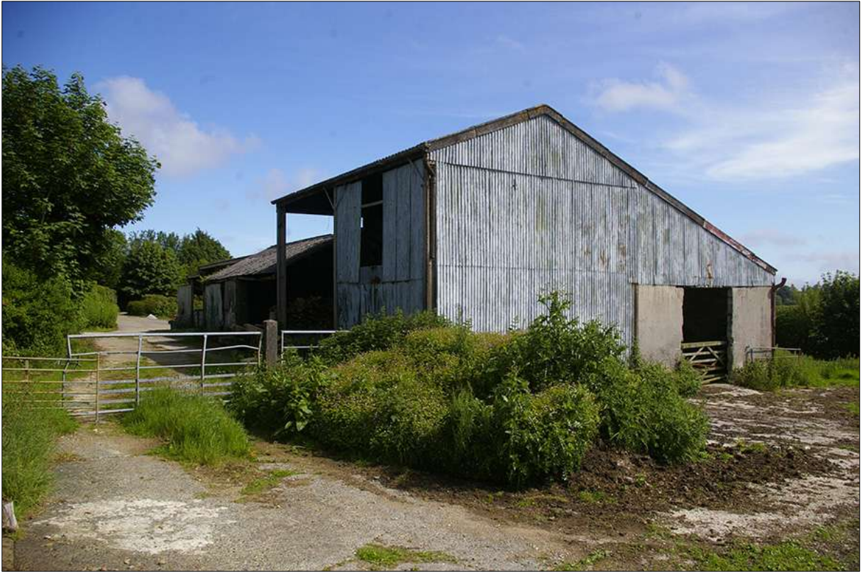
The recent pole barn with lean-to at the western end of Beneathway Farm; viewed from the north-west, looking south-east.
