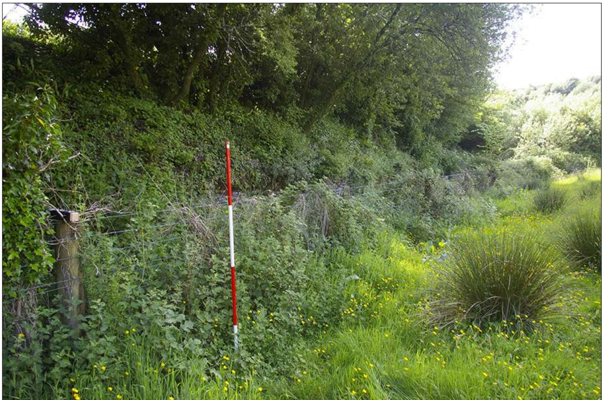
The southern end of the western field, showing part of walled railway embankment; viewed from the north-east, looking south-west (scale 2m).
