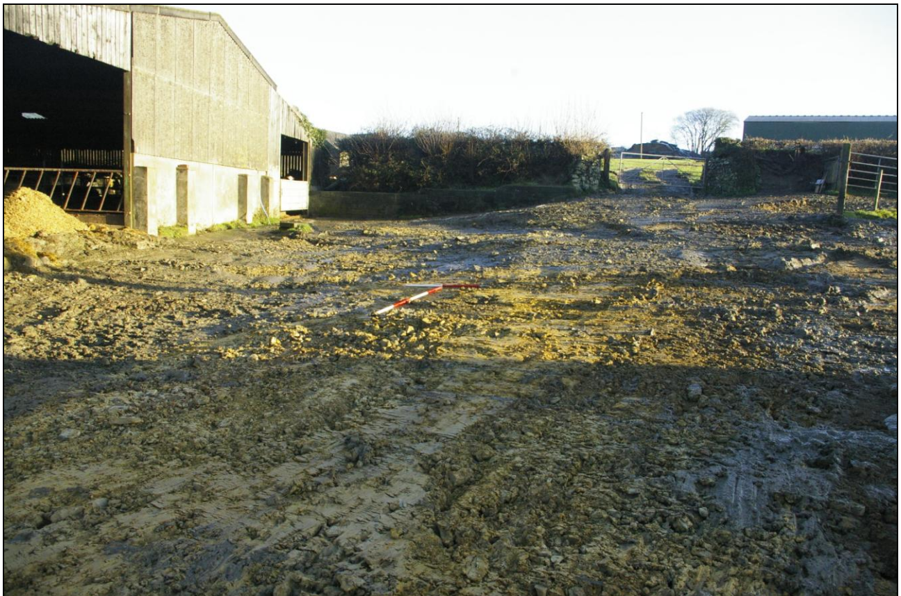
Figure 3: Area 01 viewed from the south-west (1m & 2m scale).
