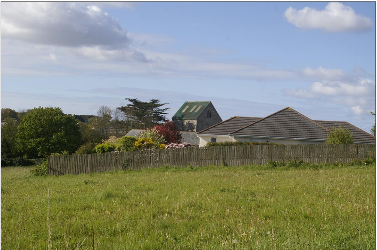
As above, with the roof of Loggans Mill rising above the roofs of the adjacent houses.
