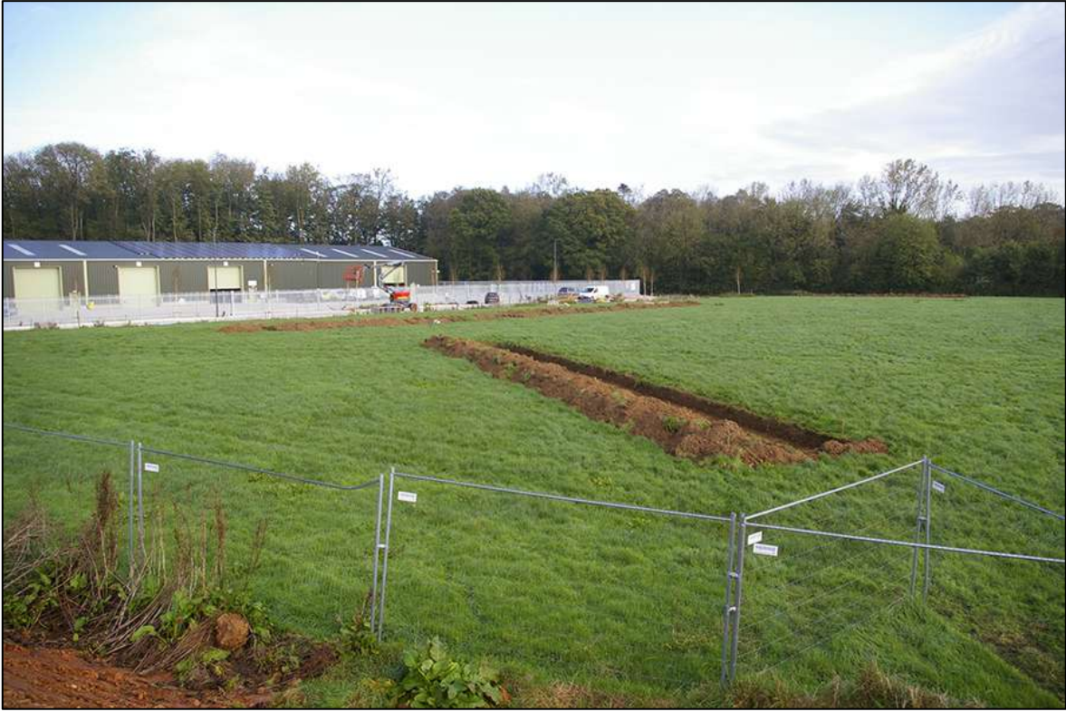
GENERAL SITE VIEW SHOWING TRENCHES #1 AND #7; VIEWED FROM THE WEST (NO SCALE).
