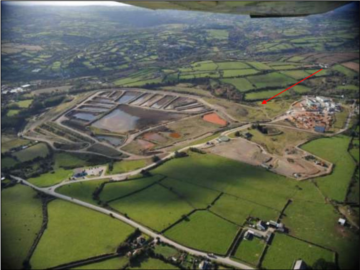
FIGURE 7: AERIAL PHOTOGRAPH FROM 2006 FOLLOWING THE REMOVAL OF THE PROCESSING PLANT AND A GREENING OF THE WHEAL JANE SITE. THE APPROXIMATE LOCATION OF THE SITE IS INDICATED (WHEAL JANE GROUP).
