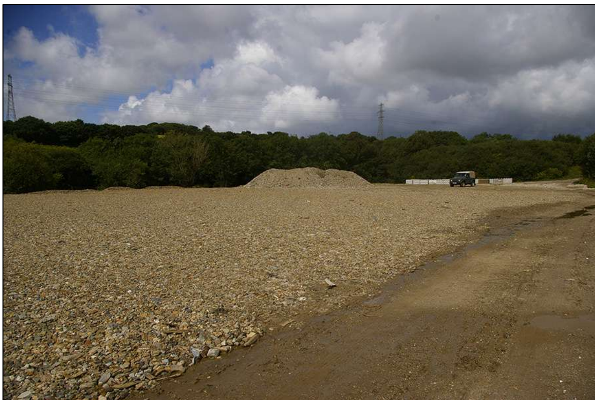
FIGURE 9: THE SITE VIEWED FROM THE EAST CORNER; LOOKING WEST (NO SCALE).
