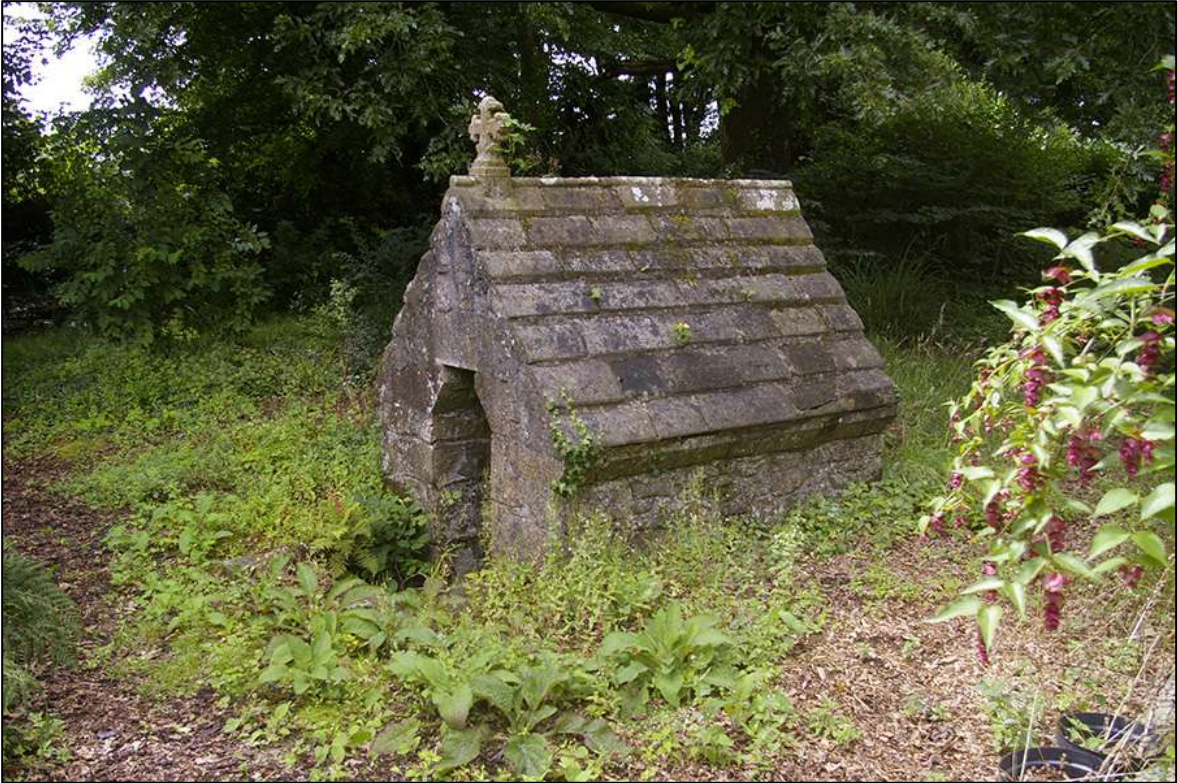
THE WELL-HEAD IN ST MICHAEL’S CHURCH YARD; LOOKING SOUTH-WEST (NO SCALE).
