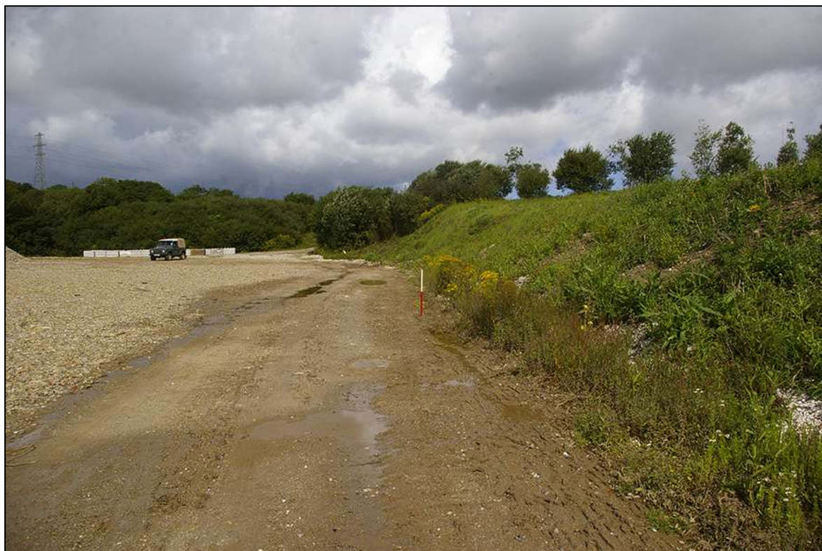
VIEW FROM THE EAST CORNER OF THE SITE; LOOKING NORTH-WEST (1M SCALE).
