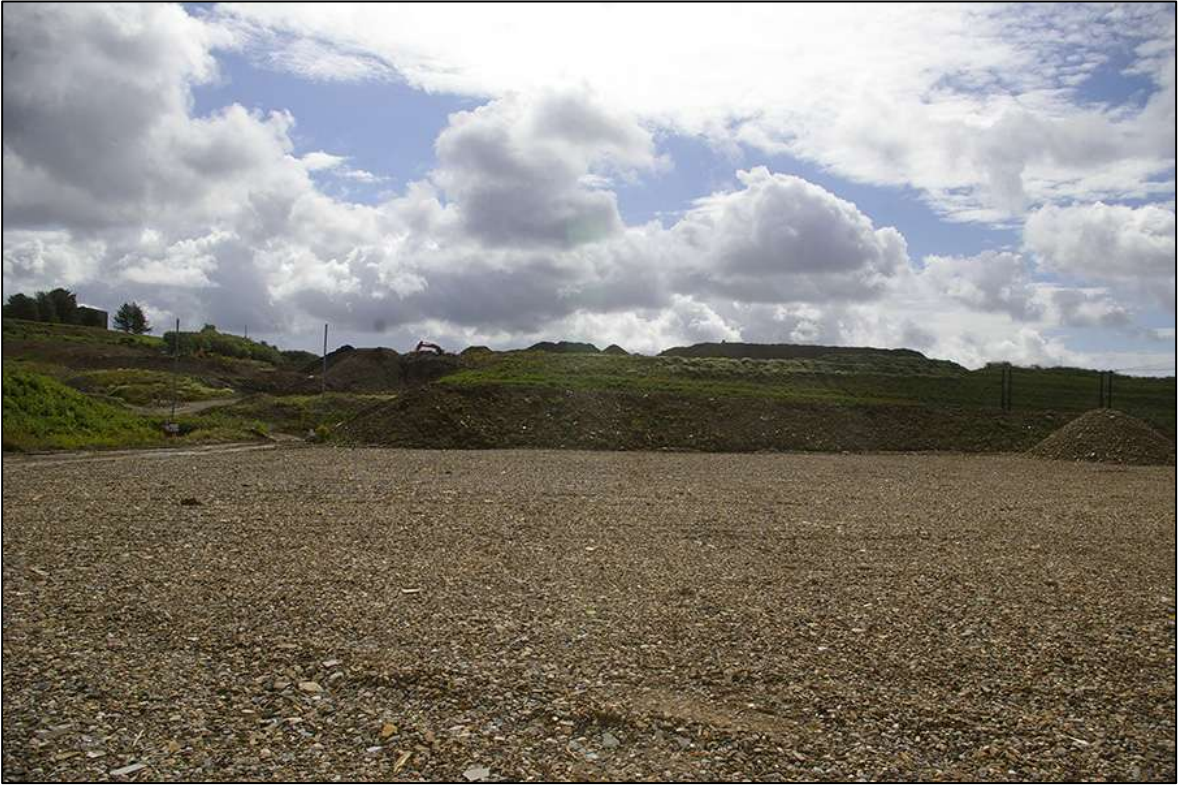
VIEW FROM THE MIDDLE OF THE SITE; LOOKING SOUTH-EAST (NO SCALE).
