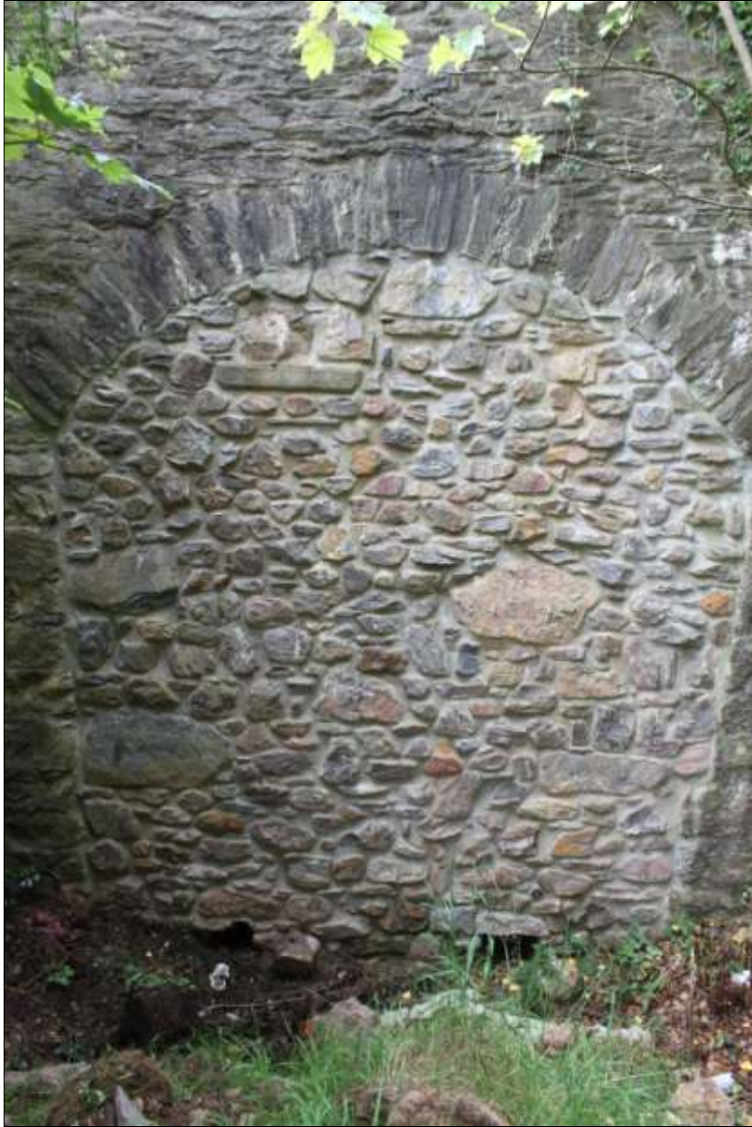
DETAILED SHOT OF THE BLOCKED TUNNEL, VIEWED FROM THE NORTH.
