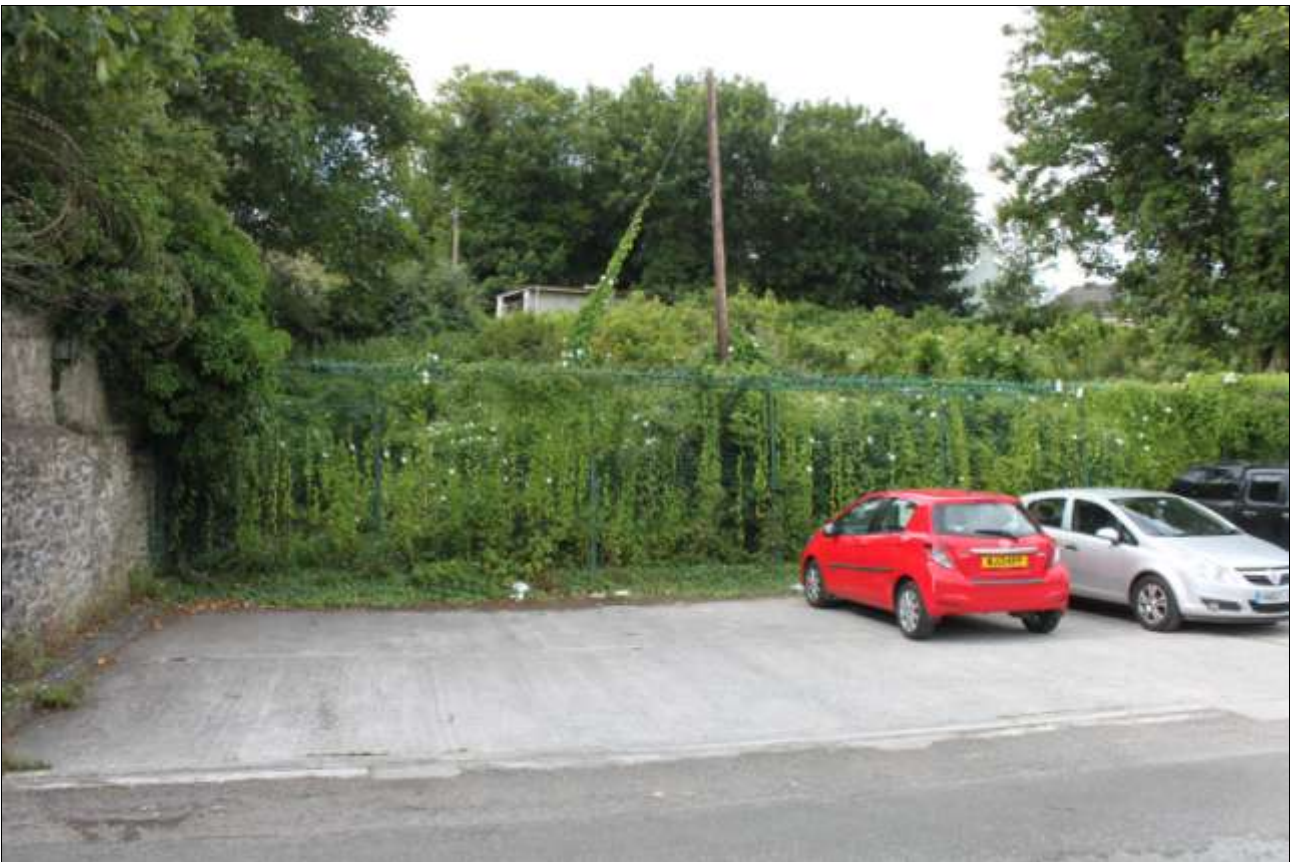
THE WESTERN PARKING AREA, WITH HISTORIC WALL TO THE LEFT, AND OVERGROWN GARDENS. THE MODERN GARAGE ON THE SOUTHERN BOUNDARY IS VISIBLE ABOVE THE OVERGROWN SCRUB.
