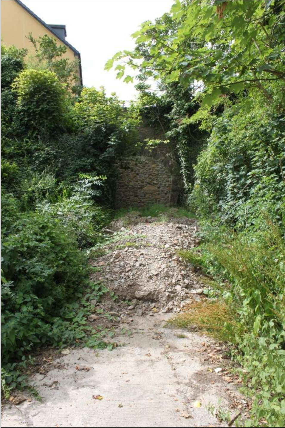
SHOT OF LOCATION OF FORMER RAILWAY AND BLOCKED TUNNEL, VIEWED FROM THE NORTH.
