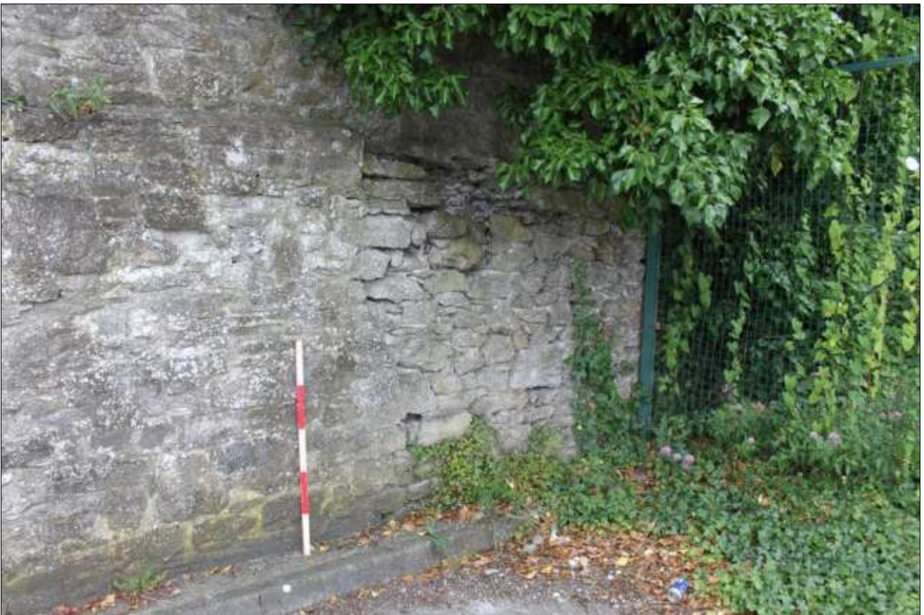
AS ABOVE, DETAIL, VIEWED FROM THE NORTH-WEST (1M SCALE).
