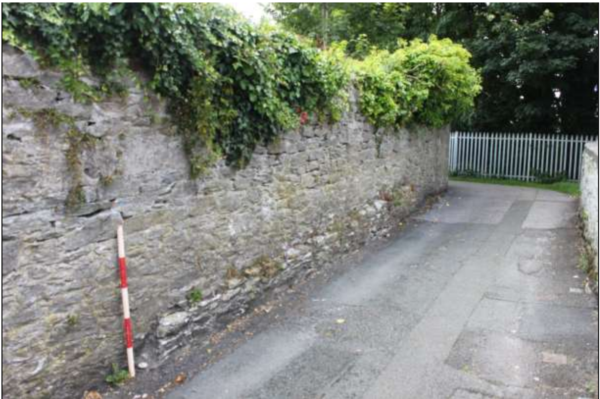
FIGURE 16: SOUTHERN END OF THE WESTERN SITE BOUNDARY (OPPOSITE KELLY COTTAGES), VIEWED FROM THE NORTH-WEST (1M SCALE). NOTE THE WALL IS BUILT OVER AND INCORPORATING PART OF AN EARLIER WALL.
