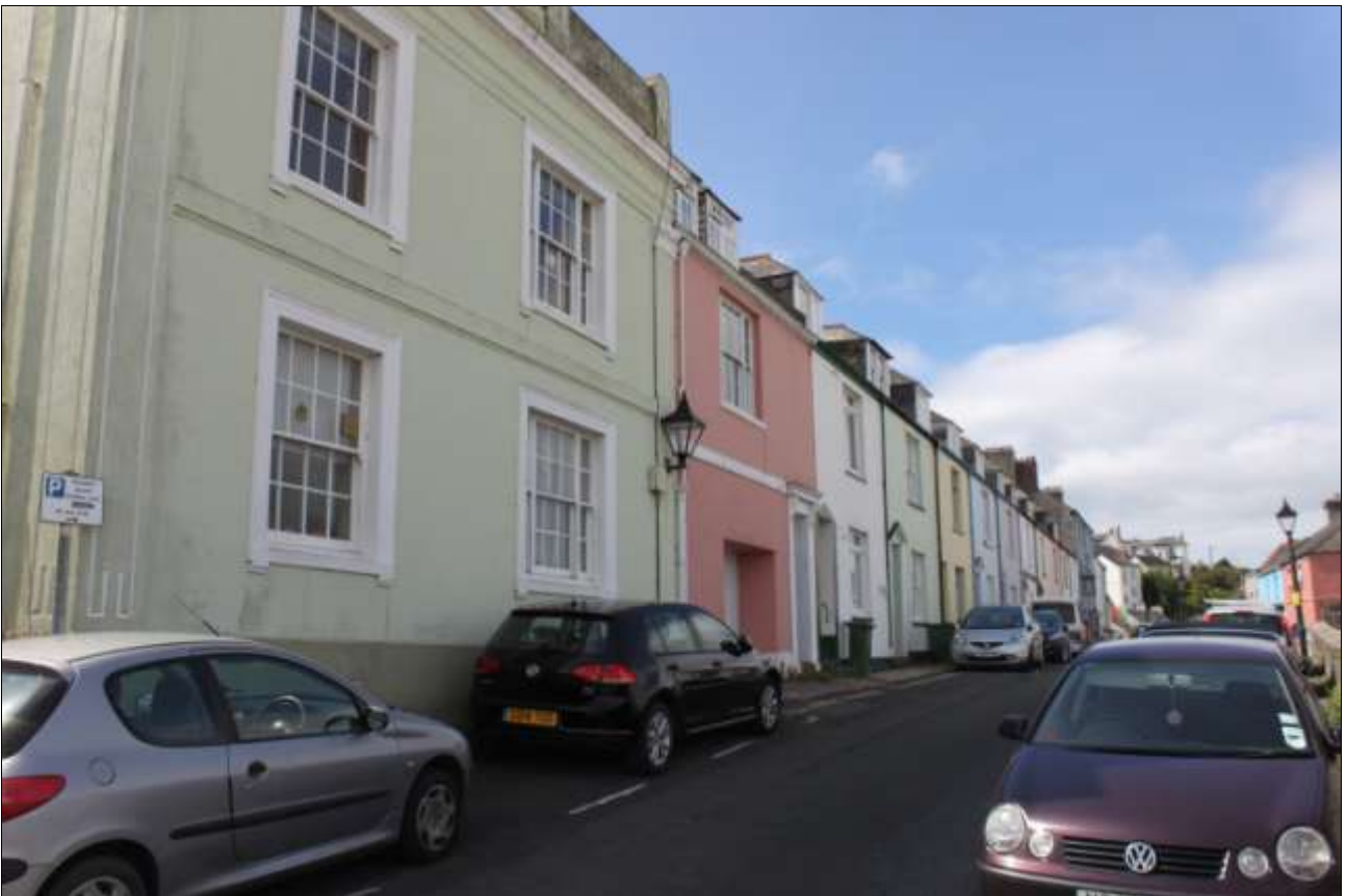
THE LISTED BUILDINGS ALONG BORINGDON ROAD, THE MANSION HOUSE IS TO THE LEFT OF SHOT, VIEWED FROM THE NORTH-EAST.
