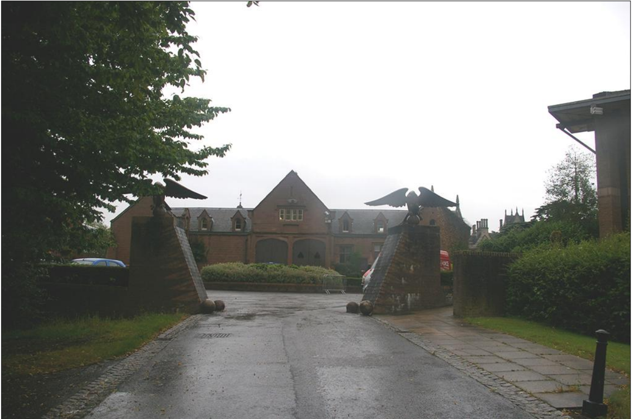
View of the Stableblock courtyard; viewed from the north.
