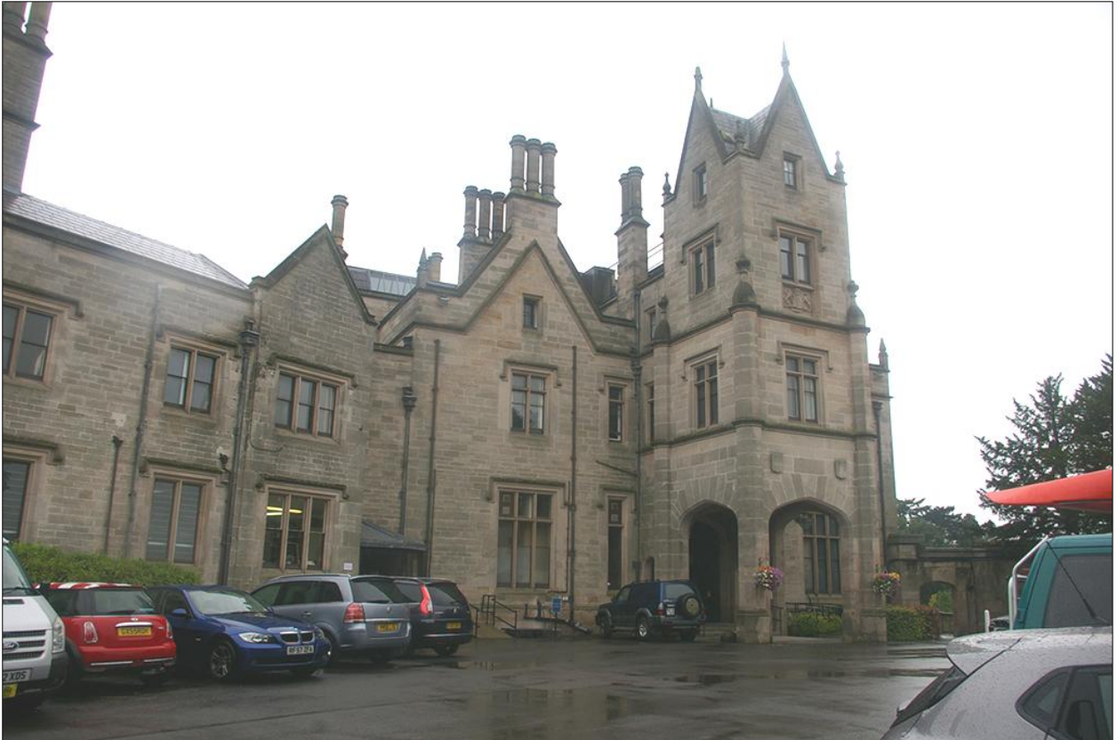
The north elevation of the Grade II* Listed Lilleshall Hall with its entrance tower; viewed from the north-north-east.
