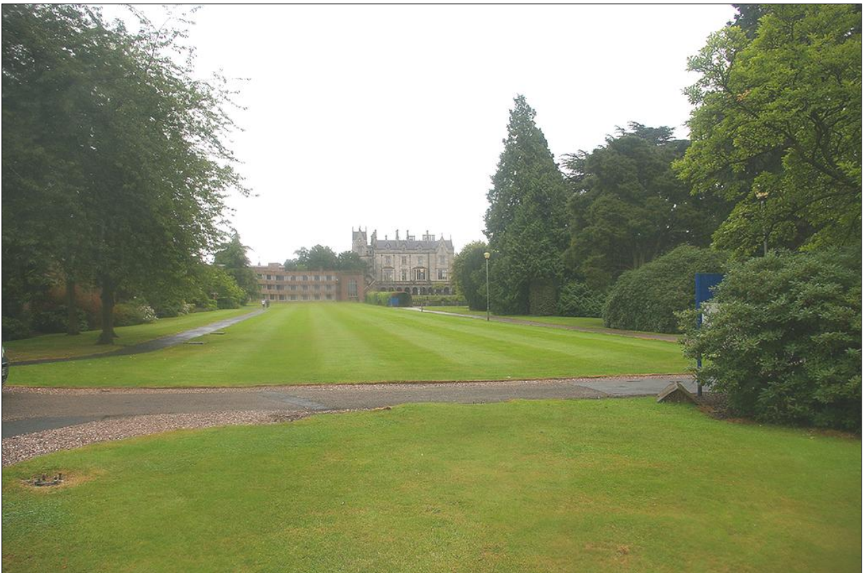
View to the Hall from the Grade II Screen; viewed from the west.
