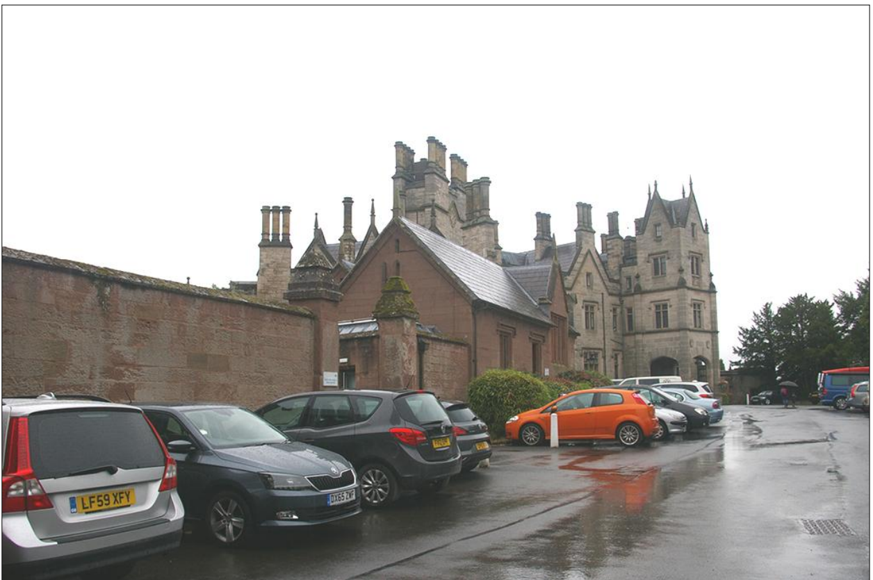
View of the Hall from the Gatehouse, showing the former courtyard now used for staff parking; viewed from the north-east.
