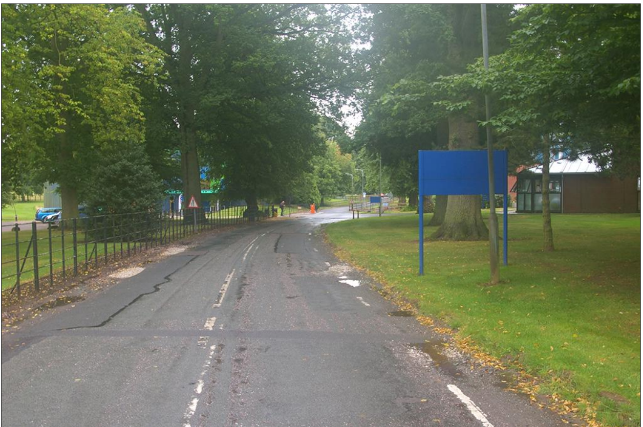
View down along the north drive from the entrance to the visitor's car park and looking towards Wenlock Hall (left of centre). The signage, fencing, bins, safety bollards and large modern buildings confer a distinctive modern institutional or campus-style character to the setting; viewed from the north-north-west.
