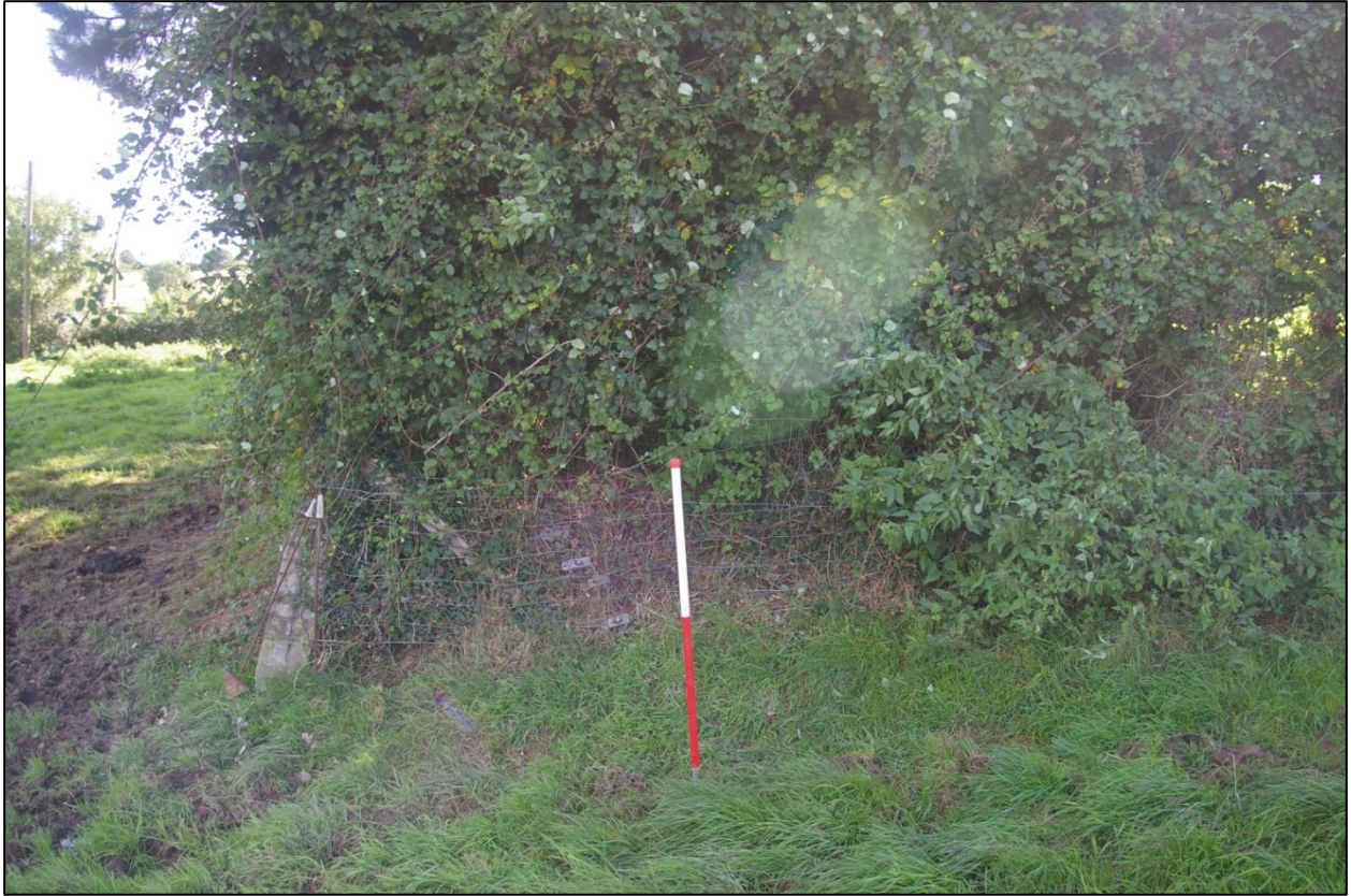
PHOTOGRAPH 11: VIEW OF BOUNDARY SURROUNDING VICARAGE PLOT; TAKEN FACING SOUTH (1M SCALE).
