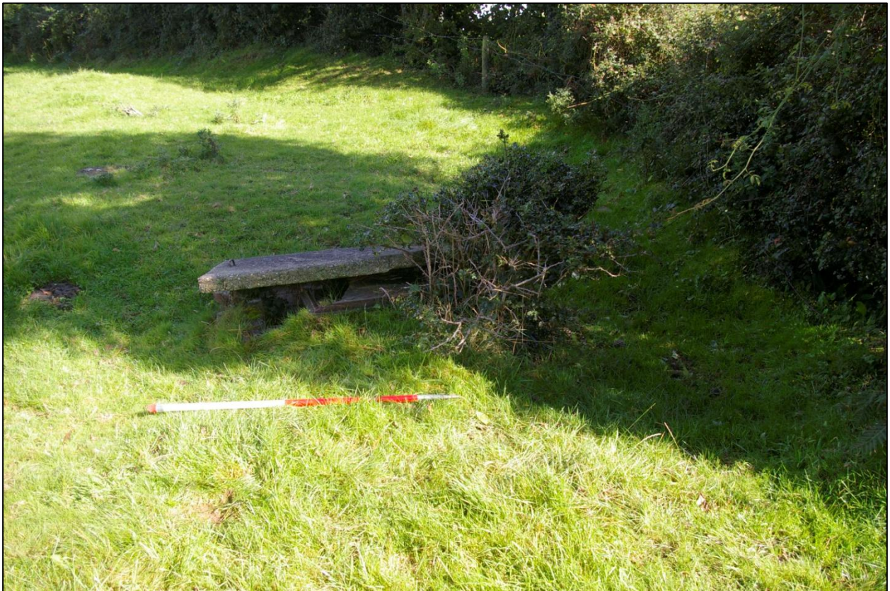
PHOTOGRAPH 12: VIEW OF MANHOLE COVER ALONG SOUTHERN BOUNDARY OF FIELD 2; TAKEN FACING EAST (1M SCALE).
