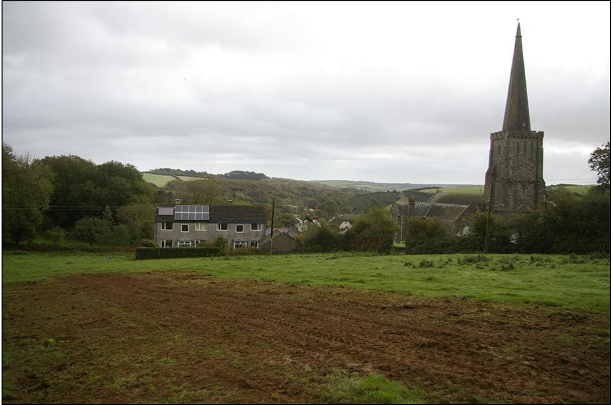
SITE SHOT, POST BACK-FILLING OF TRENCH 6; VIEWED FROM THE NORTH-WEST (NO SCALE).
