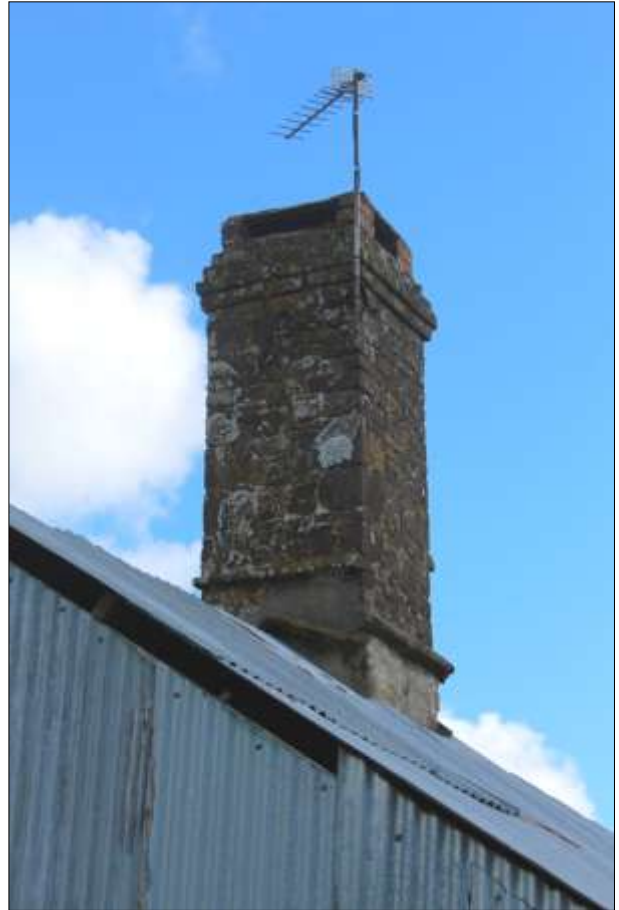
GOOD QUALITY CHIMNEY STONE STACK WITH CHAMFERED DRIP MOULDS; VIEWED FROM THE SOUTH WEST [LEFT] AND SSW [RIGHT].
