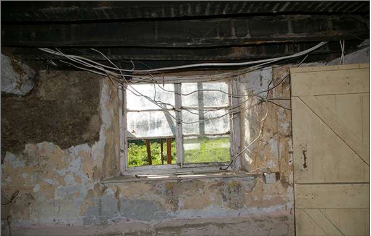
R1 SOUTH-WEST WALL, WEST WINDOW; VIEWED FROM THE NORTH-EAST.
