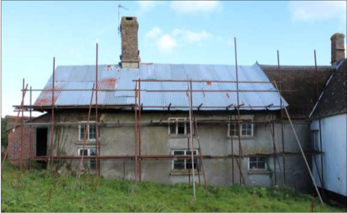
FIGURE 8: SOUTH ELEVATION, VIEWED FROM THE SOUTH.
