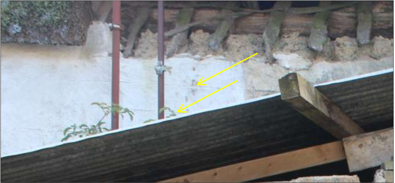
ASHLAR DETAILING ON THE NORTH-EAST WALL (INDICATED).
