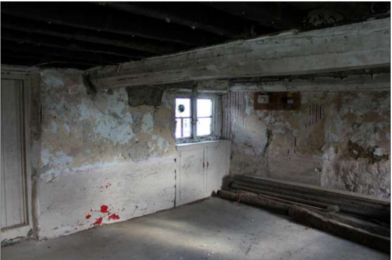
R1, NORTH-EAST WALL; VIEWED FROM THE WEST.
