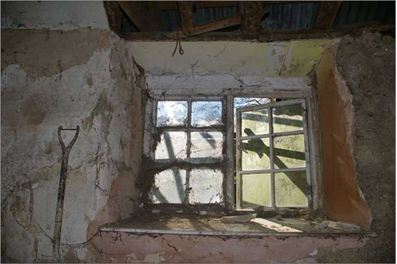
R4 SOUTH-WEST WALL, EAST WINDOW. VIEWED FROM THE NORTH-EAST.
