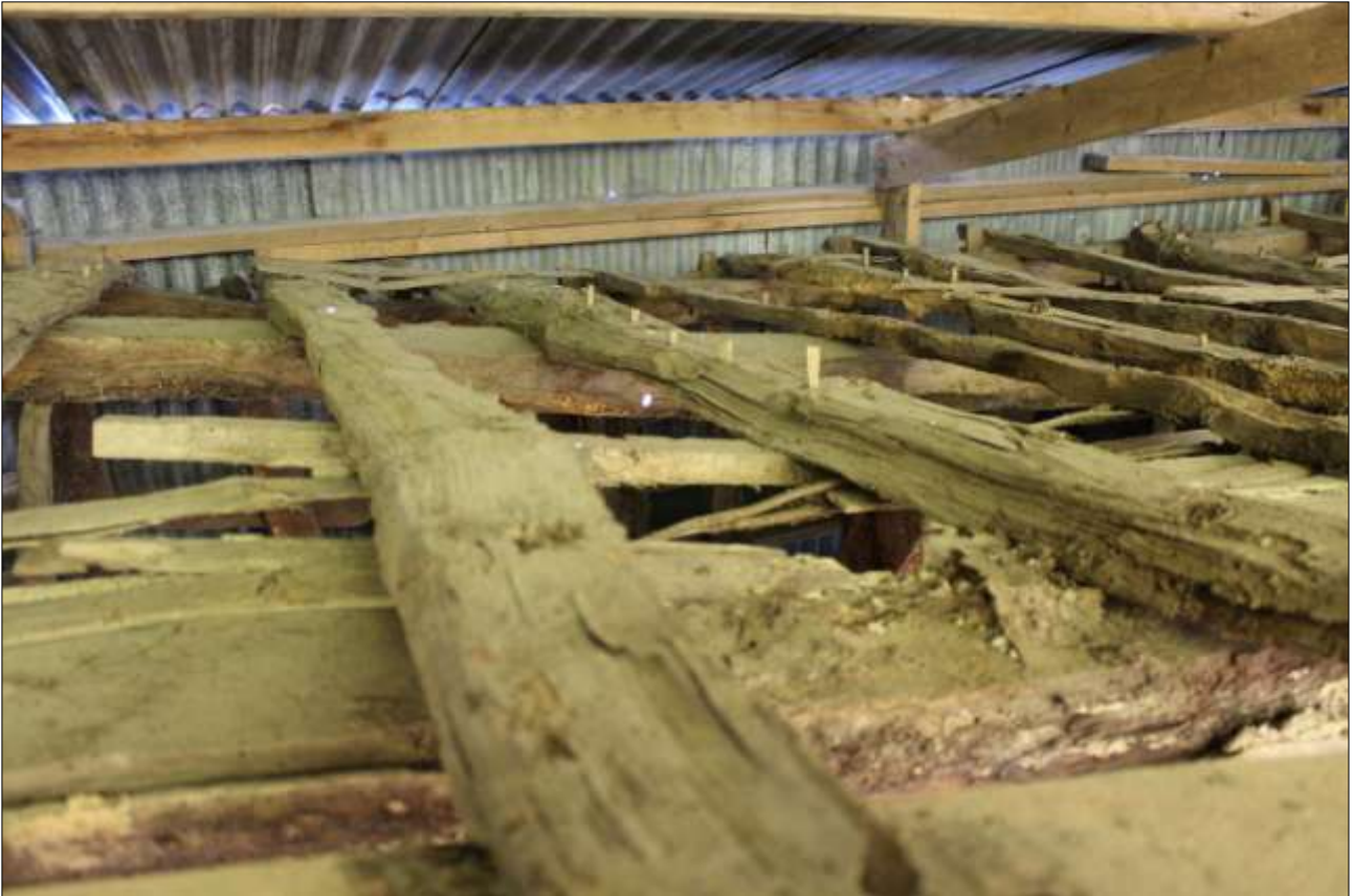
R4, DETAIL OF THE PEGGED RAFTERS; VIEWED FROM THE SOUTH.
