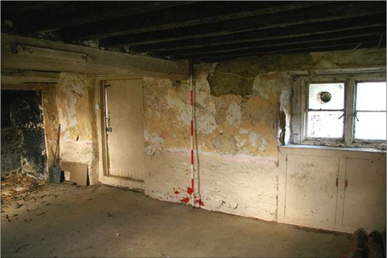
R1, NORTH-EAST WALL; VIEWED FROM THE SOUTH (SCALE 2M).
