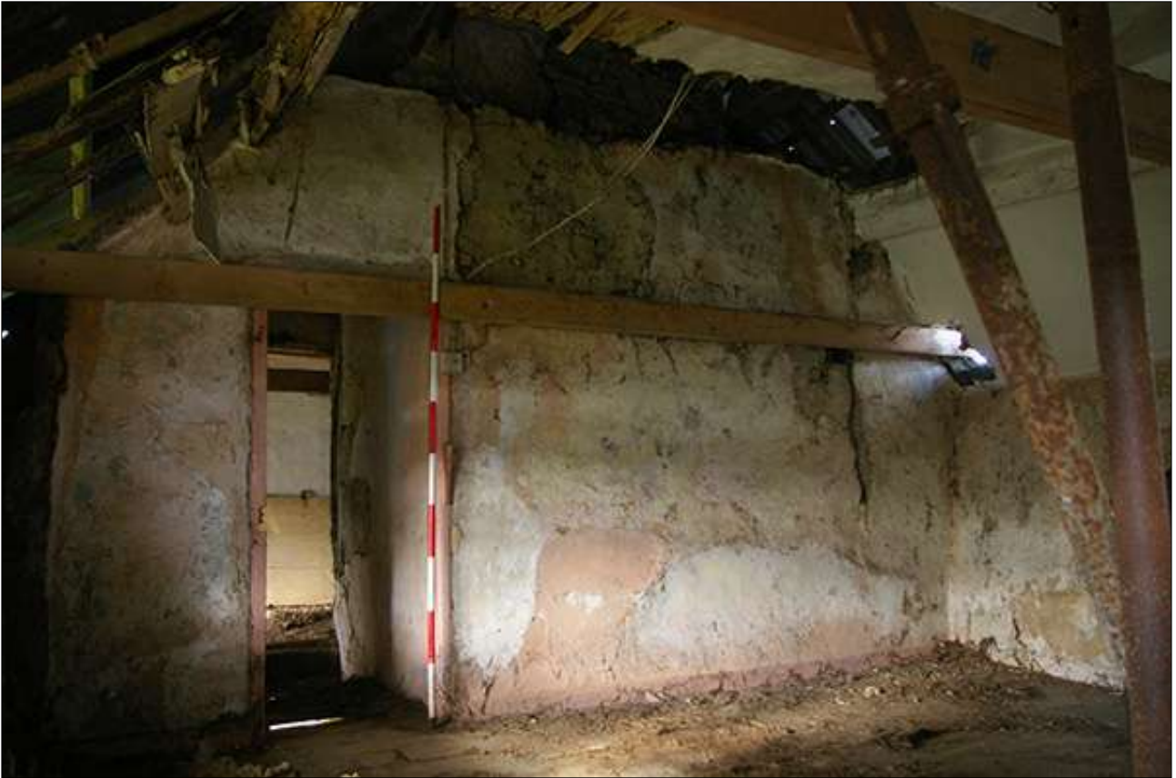
R4, SHOWING THE STACK; VIEWED FROM THE SOUTH-EAST (SCALE 2M).
