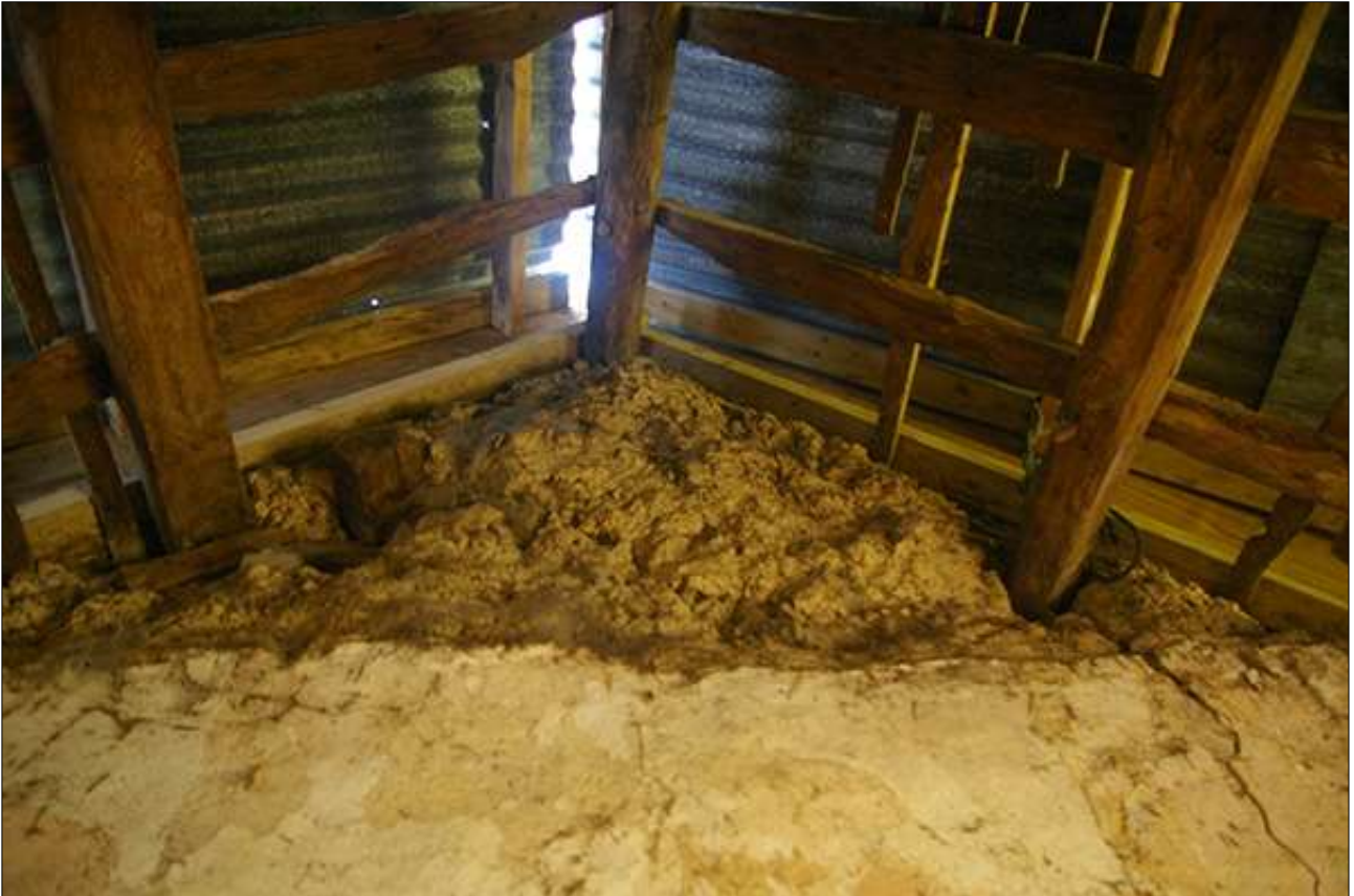
R4, THE APEX OF THE SOUTH-EAST GABLE; VIEWED FROM THE NORTH-WEST.
