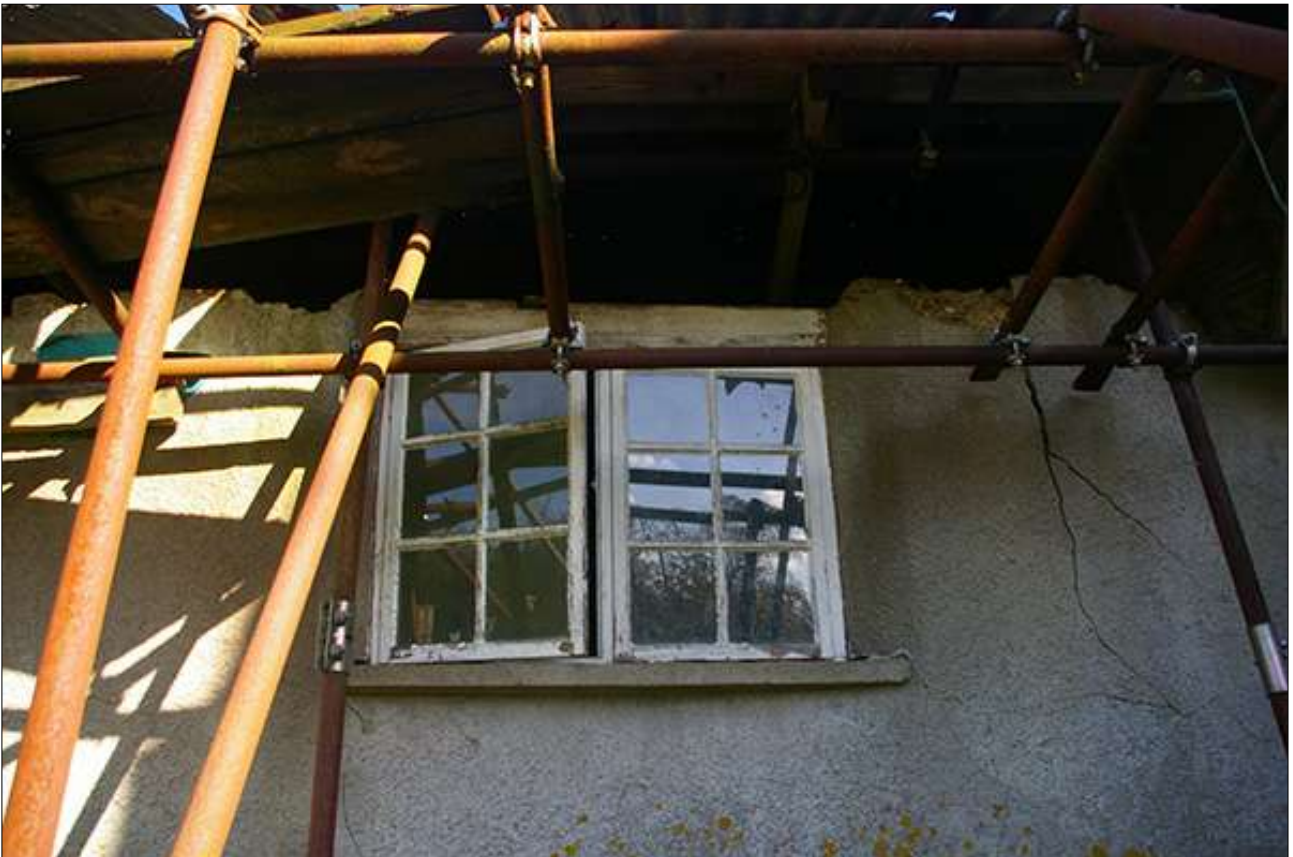
SOUTH-WEST ELEVATION, FF R4 EAST WINDOW, VIEWED FROM THE SOUTH-WEST.
