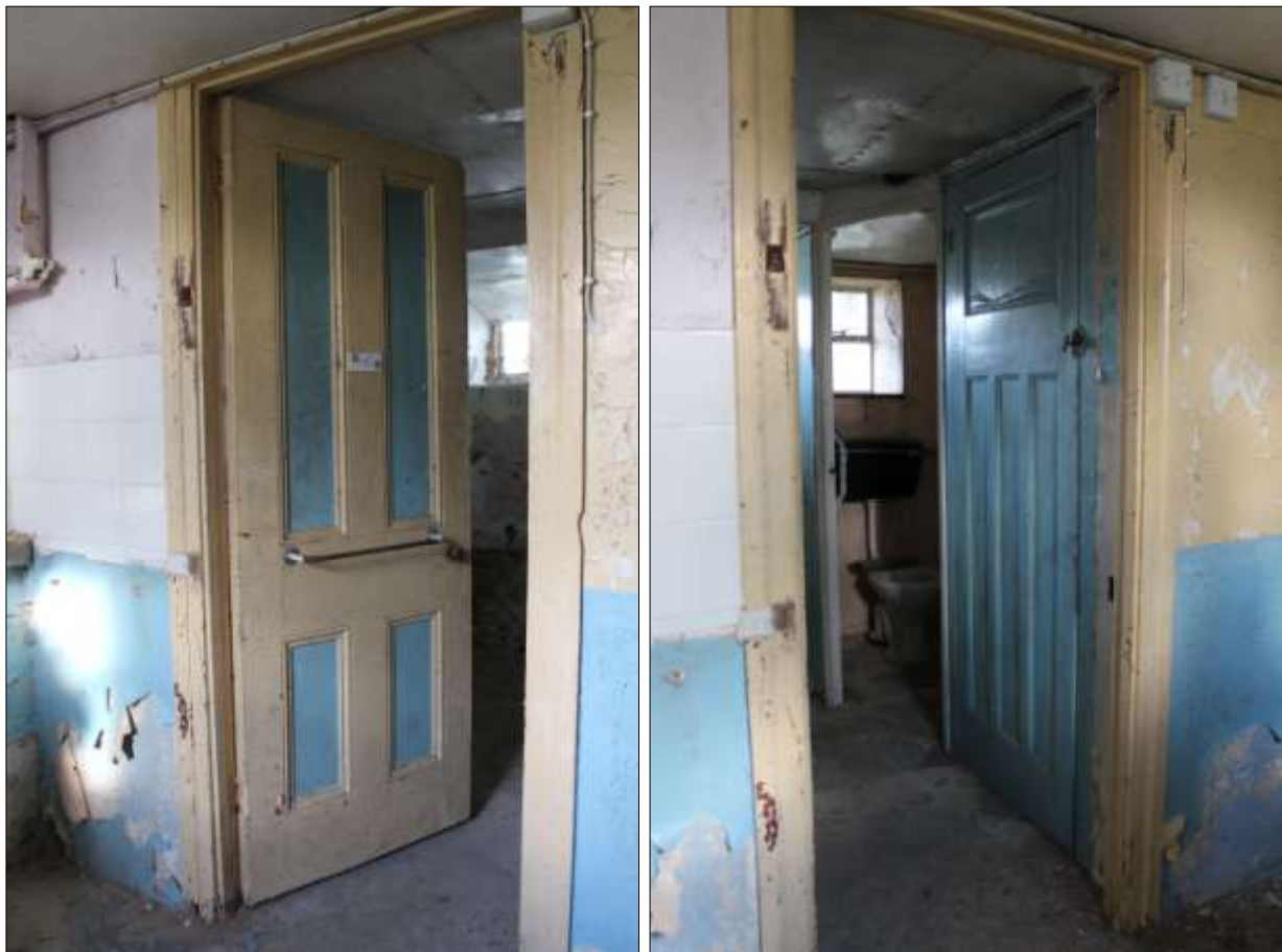
R2, THE INTERNAL PARTITIONS AND DOORS; VIEWED FROM THE SOUTH.
