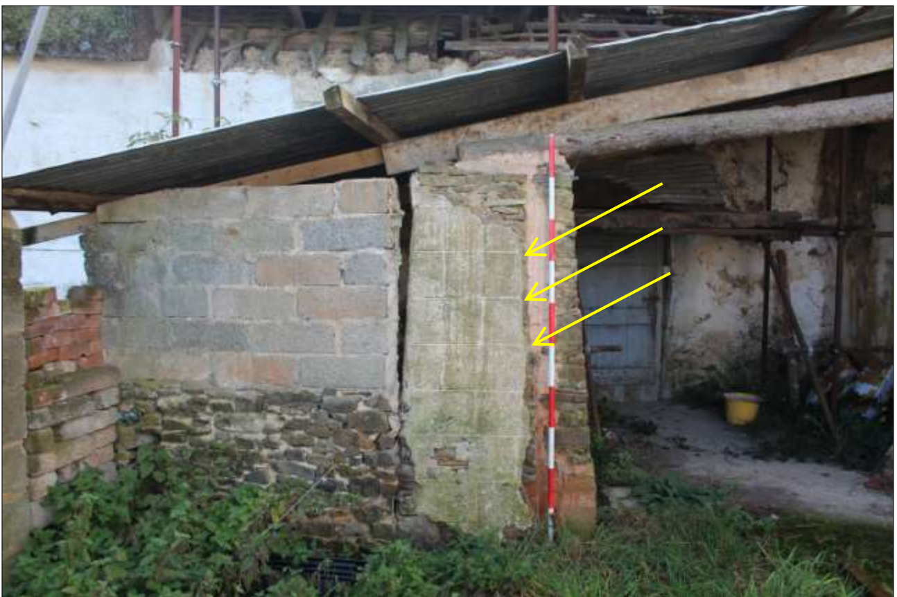
PART OF THE WALL OF THE FORMER LINHAY; VIEWED FROM THE NORTH-EAST (SCALE 2M). NOTE THE ASHLAR DETAILING ON THE PIER (INDICATED)
