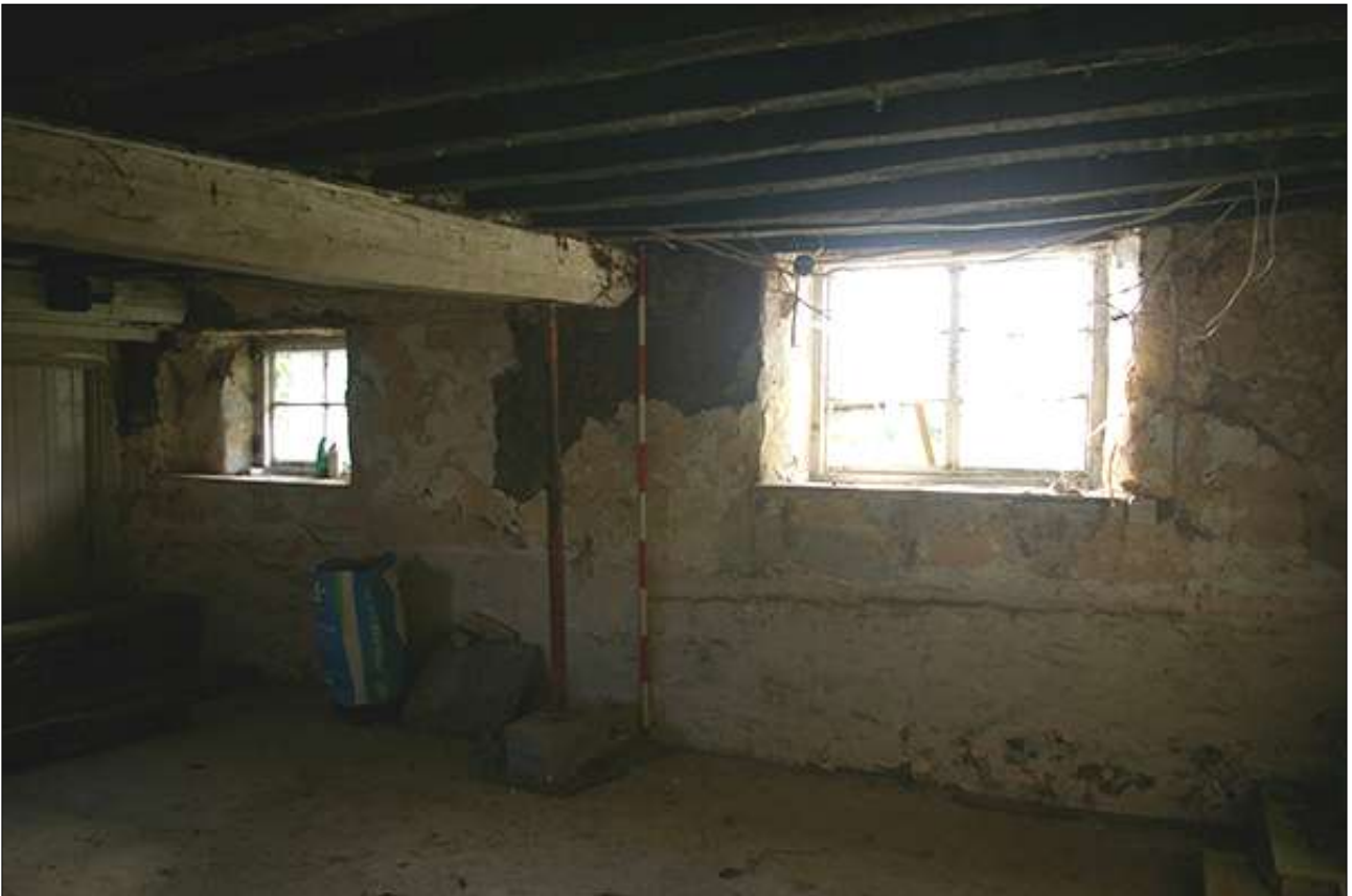
R1, SOUTH-WEST WALL; VIEWED FROM THE NORTH (SCALE 2M).
