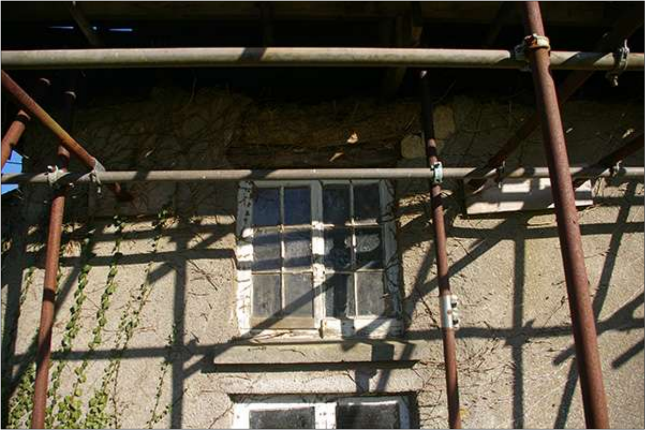
SOUTH-WEST ELEVATION, FF R5 WINDOW, VIEWED FROM THE SOUTH-WEST.
