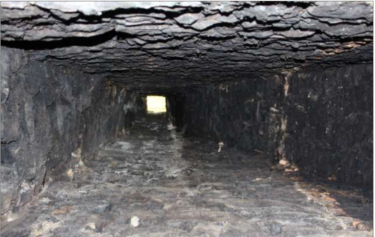
R1, VIEW UP THE CHIMNEY.
