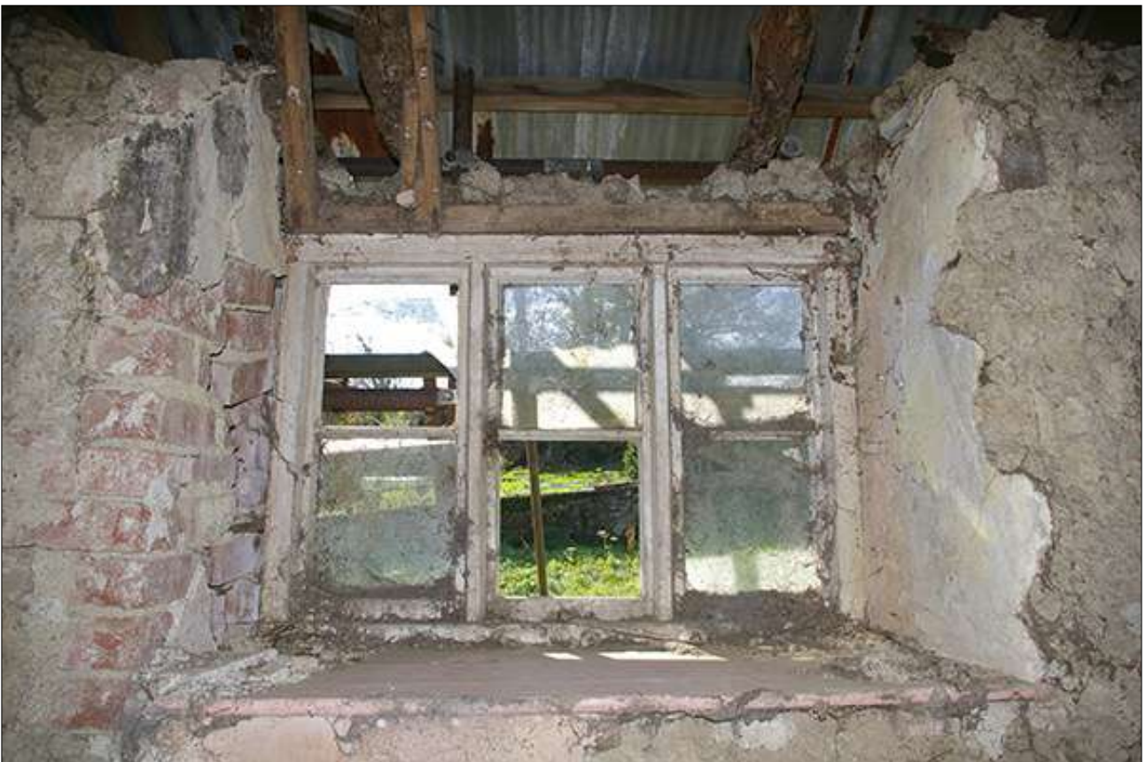
R4 SOUTH-WEST WALL, WEST WINDOW. VIEWED FROM THE NORTH-EAST.
