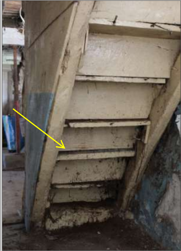
RIGHT: AS ABOVE, SHOWING DETAIL OF THE REUSED BEADED PLANKS (INDICATED); VIEWED FROM THE WEST.
