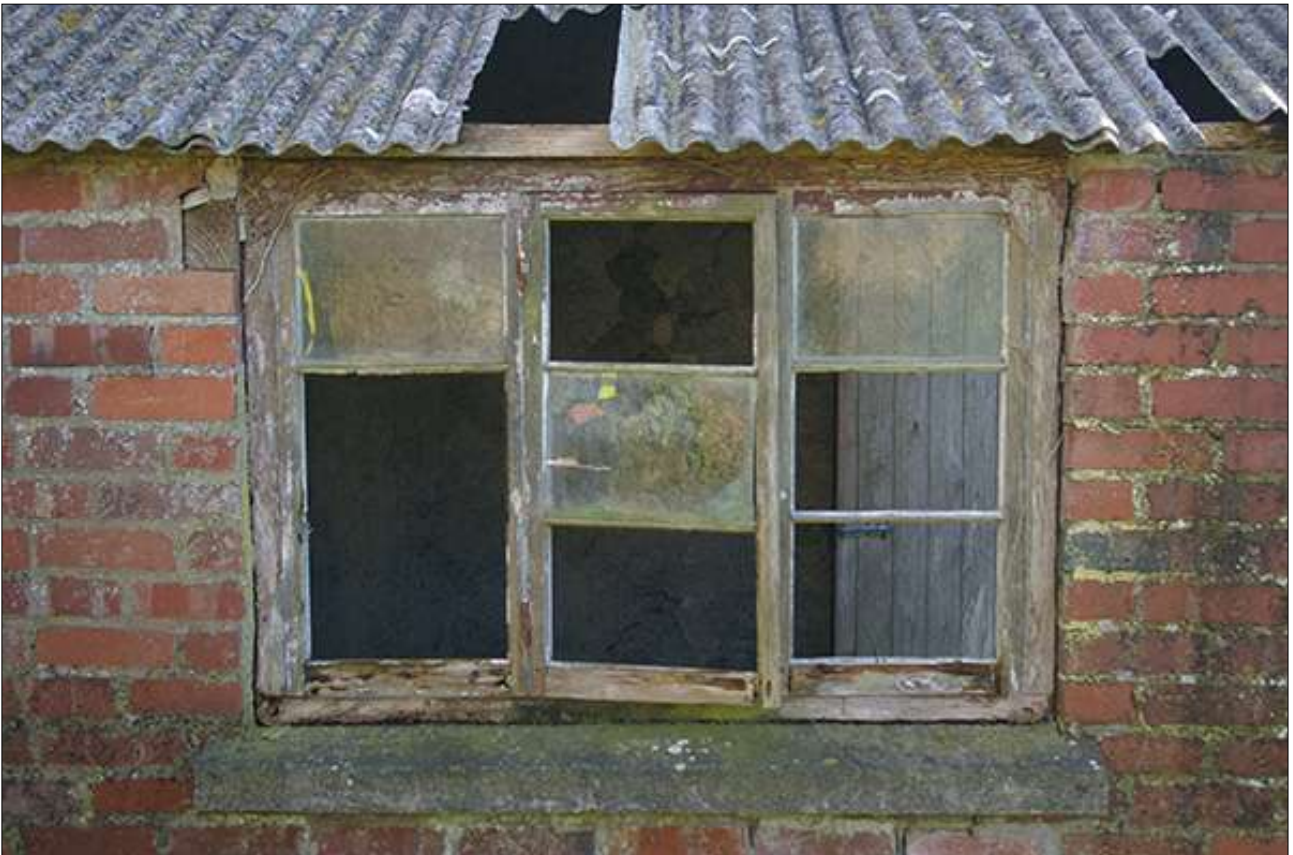
REUSED 19 TH CENTURY CASEMENT WINDOW IN R6; VIEWED FROM THE NORTH-WEST.
