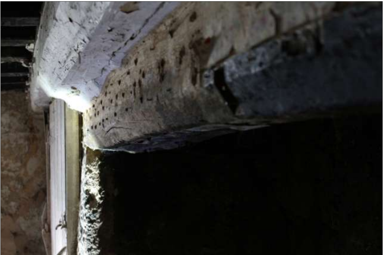
R1, DETAIL OF THE CHAMFER ON THE LINTEL AND GRANITE ORTHOSTAT; VIEWED FROM THE NORTH-EAST.
