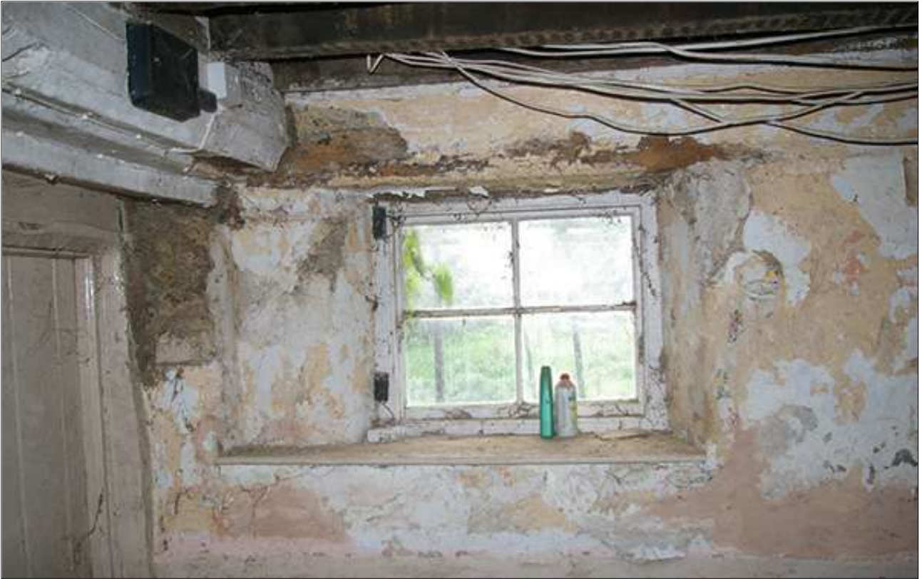
R1 SOUTH-WEST WALL, EAST WINDOW. VIEWED FROM THE NORTH-EAST.
