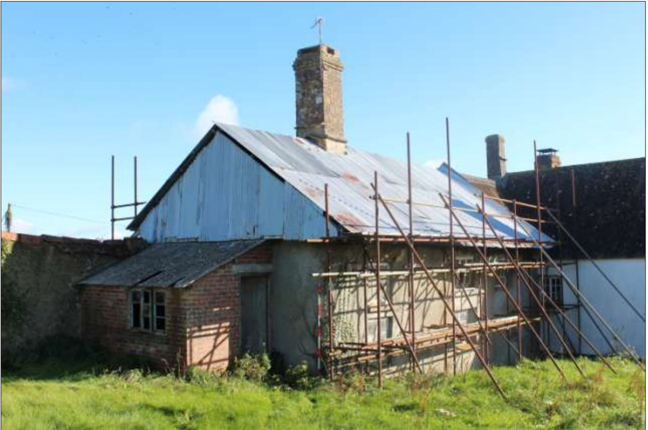
NORTH-WEST AND SOUTH-WEST ELEVATIONS; VIEWED FROM THE WEST (SCALE 2M).
