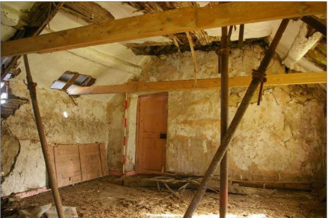
R4, SOUTH-EAST AND NORTH-EAST WALLS; VIEWED FROM THE WEST (SCALE 2M).
