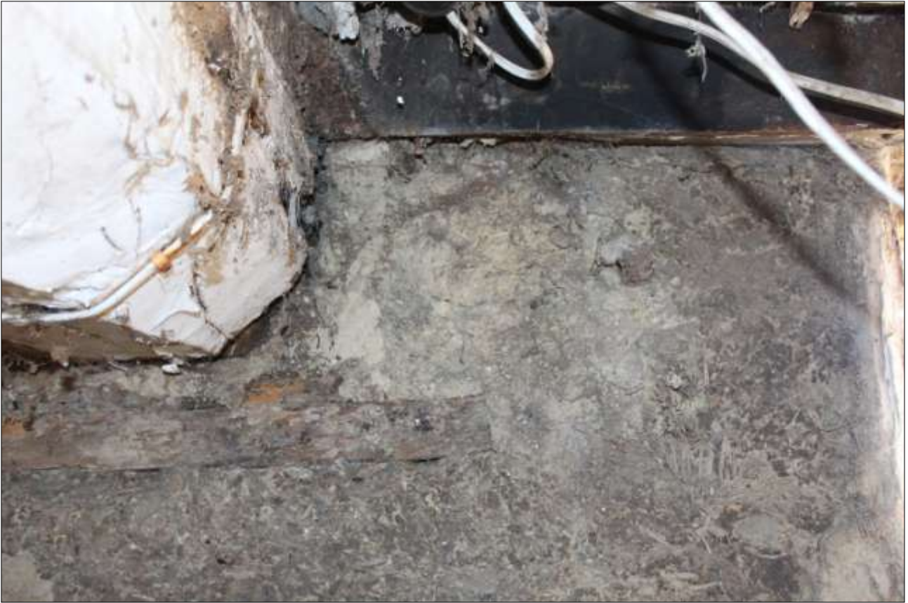
R1, DETAIL OF THE COB WHERE THE CENTRAL BEAM ENTERS THE SOUTH-WEST WALL; VIEWED FROM THE NORTH.
