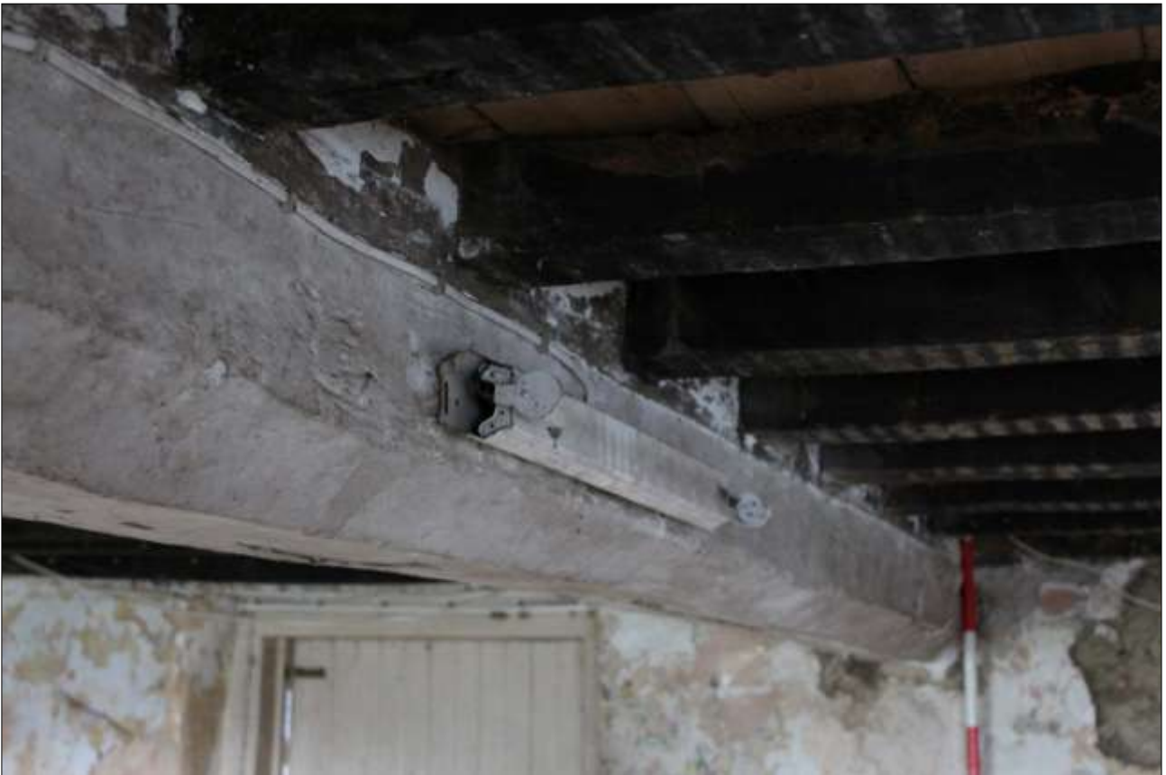
R1, DETAIL OF THE CENTRAL BEAM; VIEWED FROM THE SOUTH.
