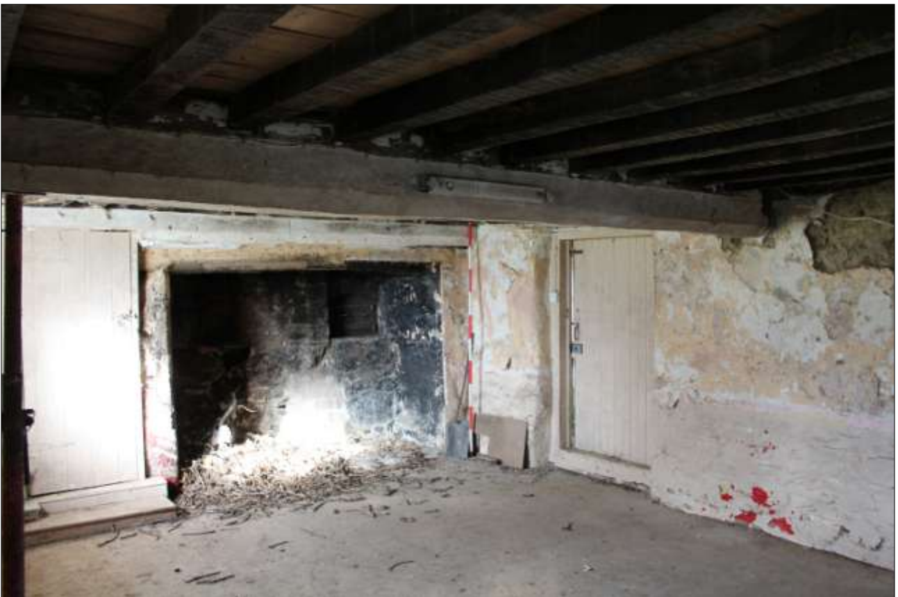
R1, NORTH-EAST AND NORTH-WEST WALLS; VIEWED FROM THE SOUTH-EAST (SCALE 2M).
