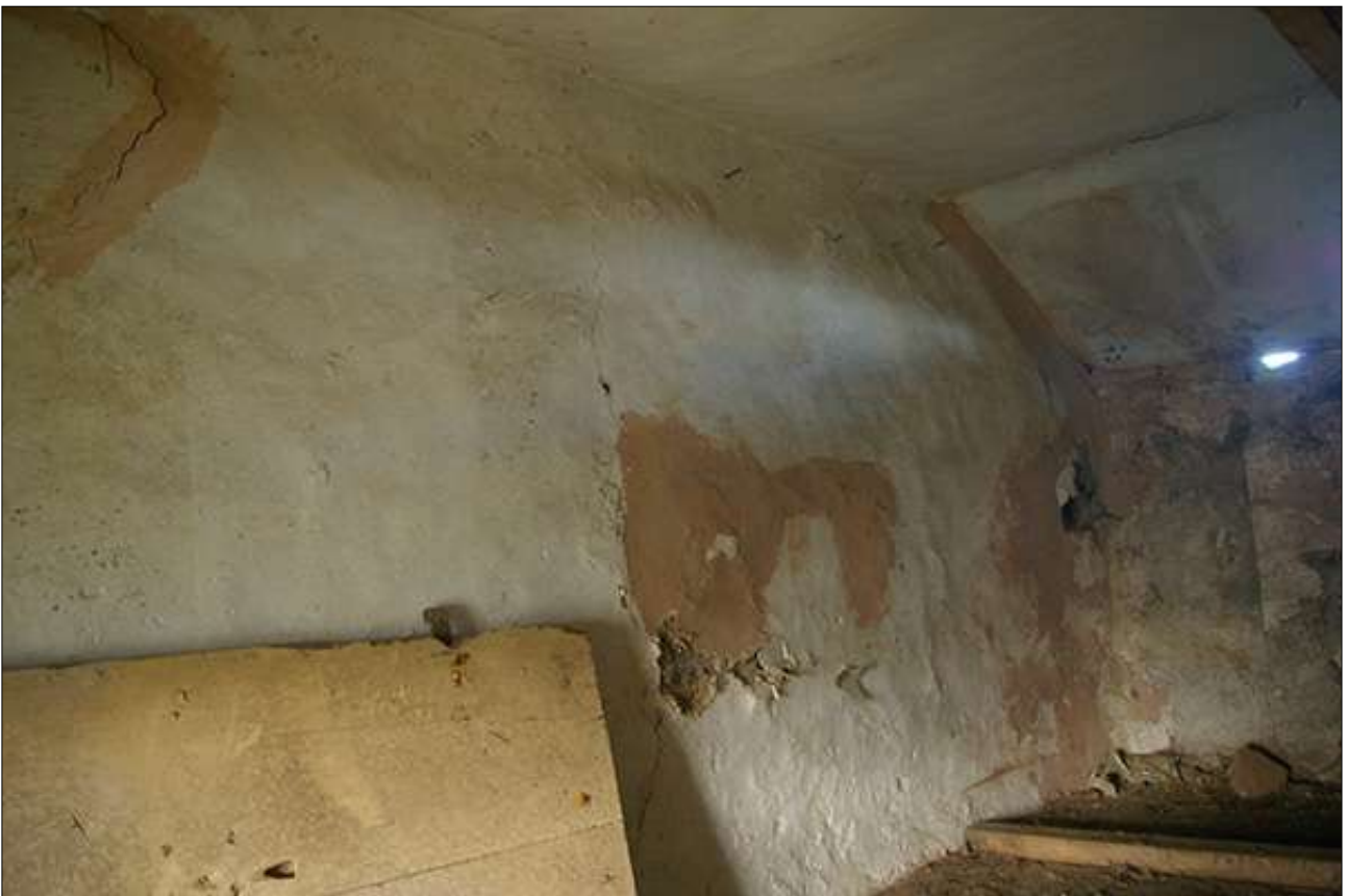
R5, THE NORTH-WEST GABLE; VIEWED FROM THE SOUTH.
