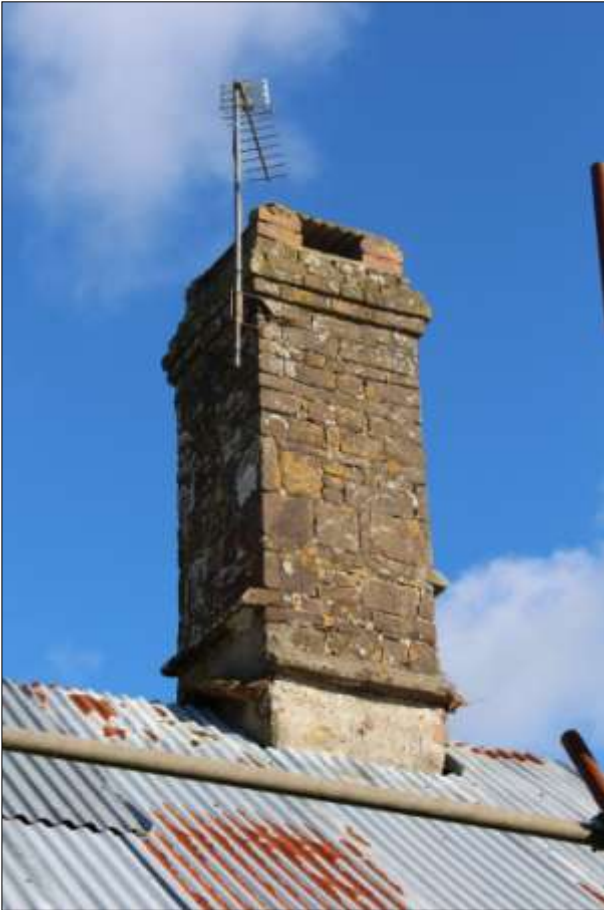
GOOD QUALITY CHIMNEY STONE STACK WITH CHAMFERED DRIP MOULDS; VIEWED FROM THE SOUTH WEST [LEFT] AND SSW [RIGHT].
