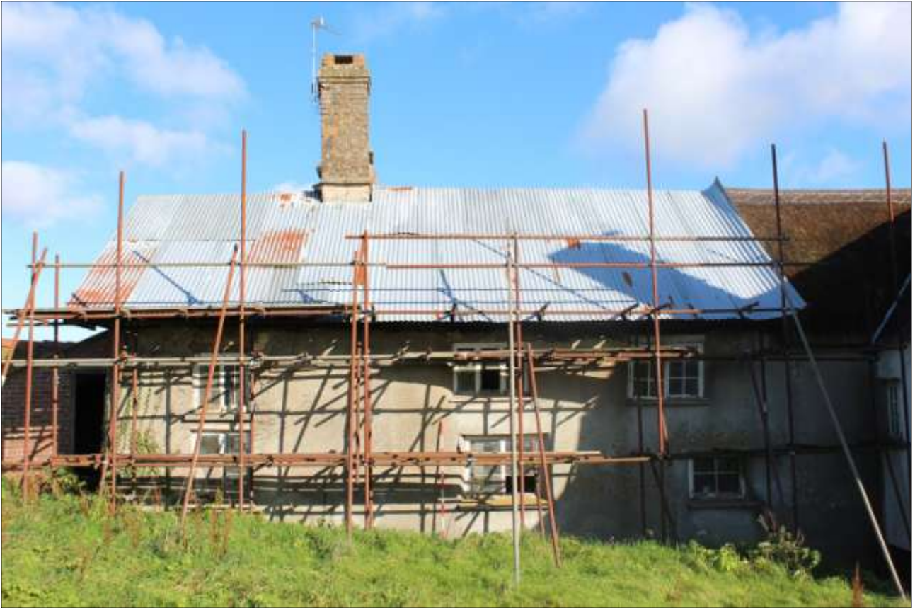
SOUTH-WEST ELEVATION; VIEWED FROM THE SOUTH-WEST (SCALE 2M).
