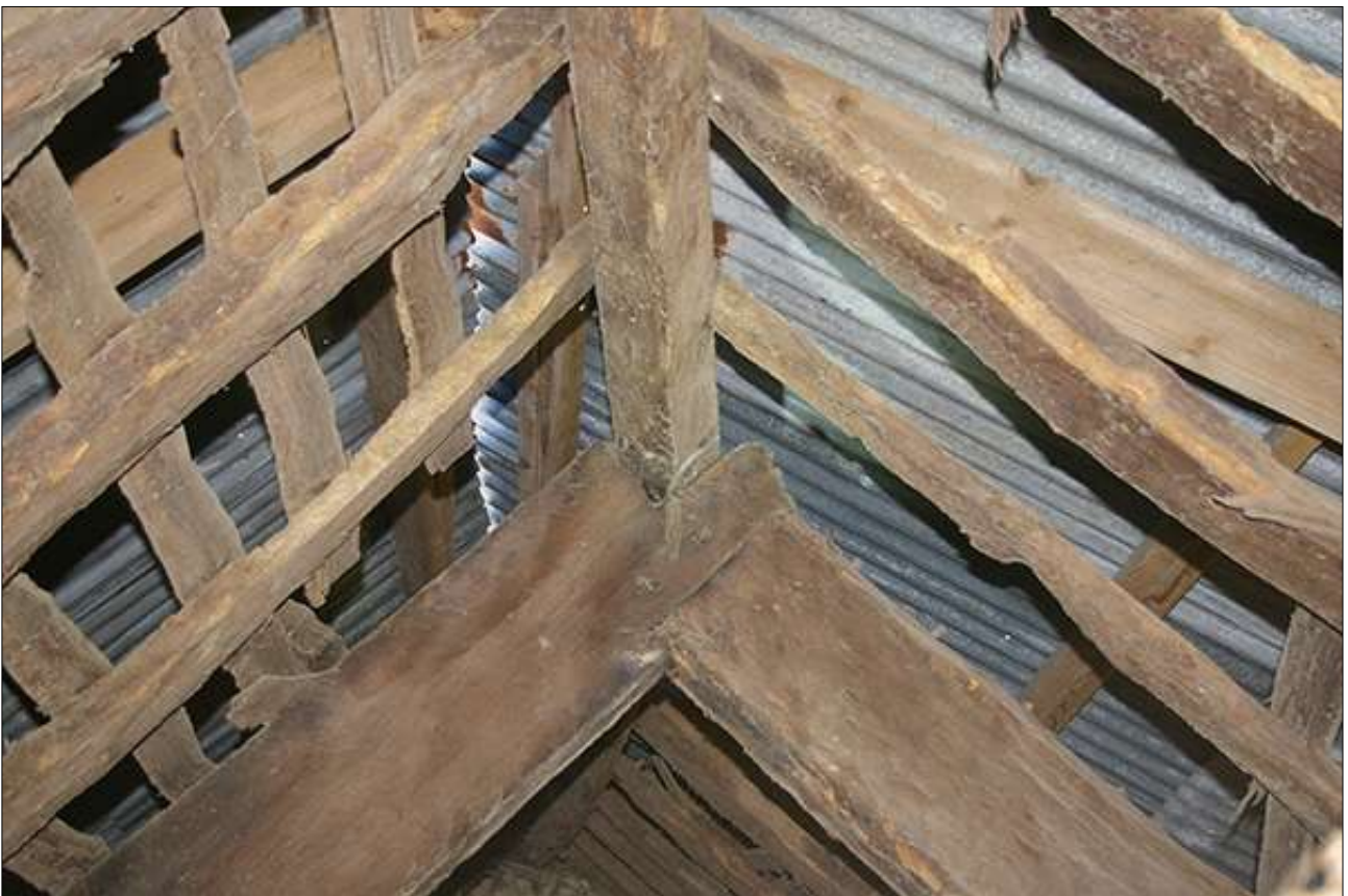
R4, DETAIL OF THE APEX OF TRUSS #1; VIEWED FROM THE NORTH-WEST.
