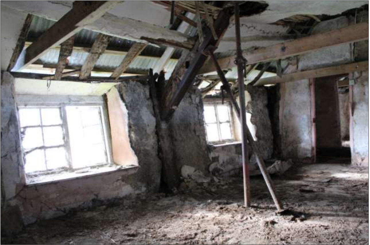
R4, SOUTH-WEST WALL; VIEWED FROM THE EAST.
