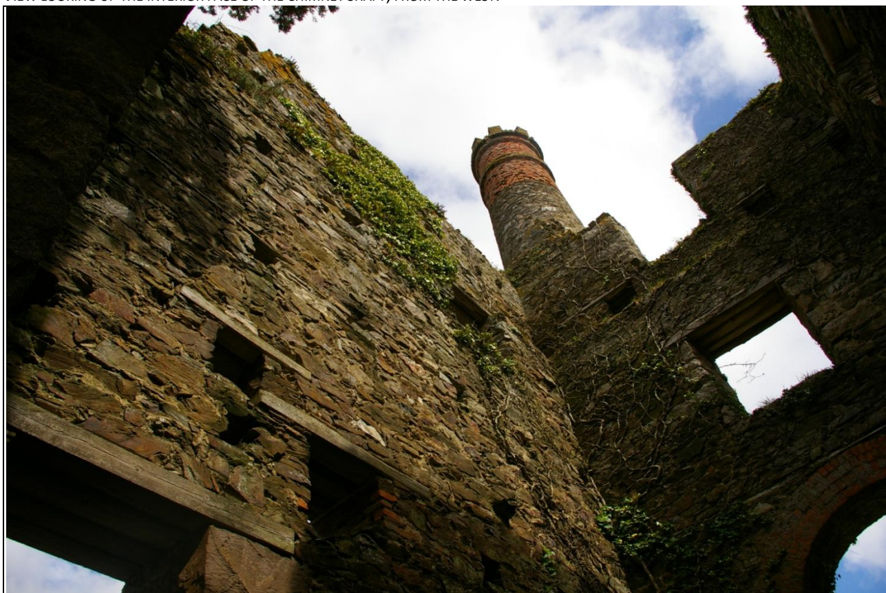
VIEW OF THE PARTICULARLY HEAVY BASE OF THE WALL TO THE LONG NORTH-EAST ELEVATION; FROM THE EAST.
