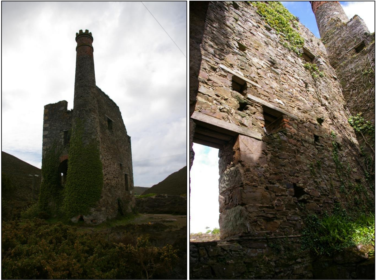
FIGURE 3 (LEFT): THE CHIMNEY WHICH CLASPS THE CORNER OF THE ENGINE HOUSE, FROM THE SOUTH, SOUTH-EAST.
