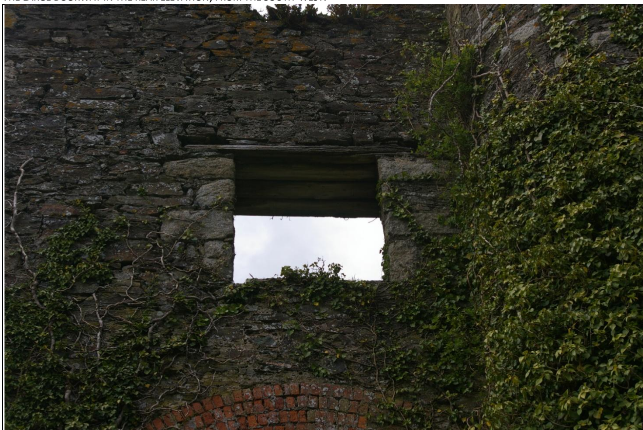
DETAIL OF OPENING WITH A WEATHERED ORIGINAL TIMBER LINTEL, IN THE REAR WALL OF THE ENGINE HOUSE; FROM THE SOUTH-WEST.
