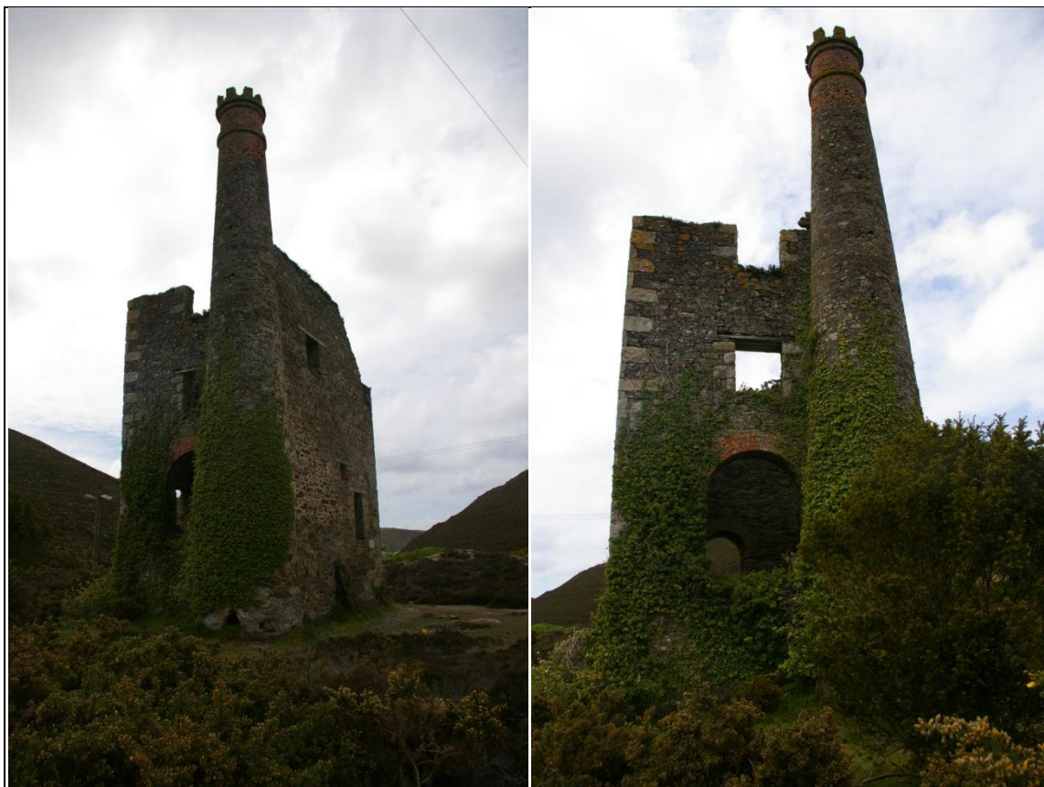
LEFT: THE CHIMNEY WHICH CLASPS THE CORNER OF THE ENGINE HOUSE, FROM THE SOUTH, SOUTH-EAST.
