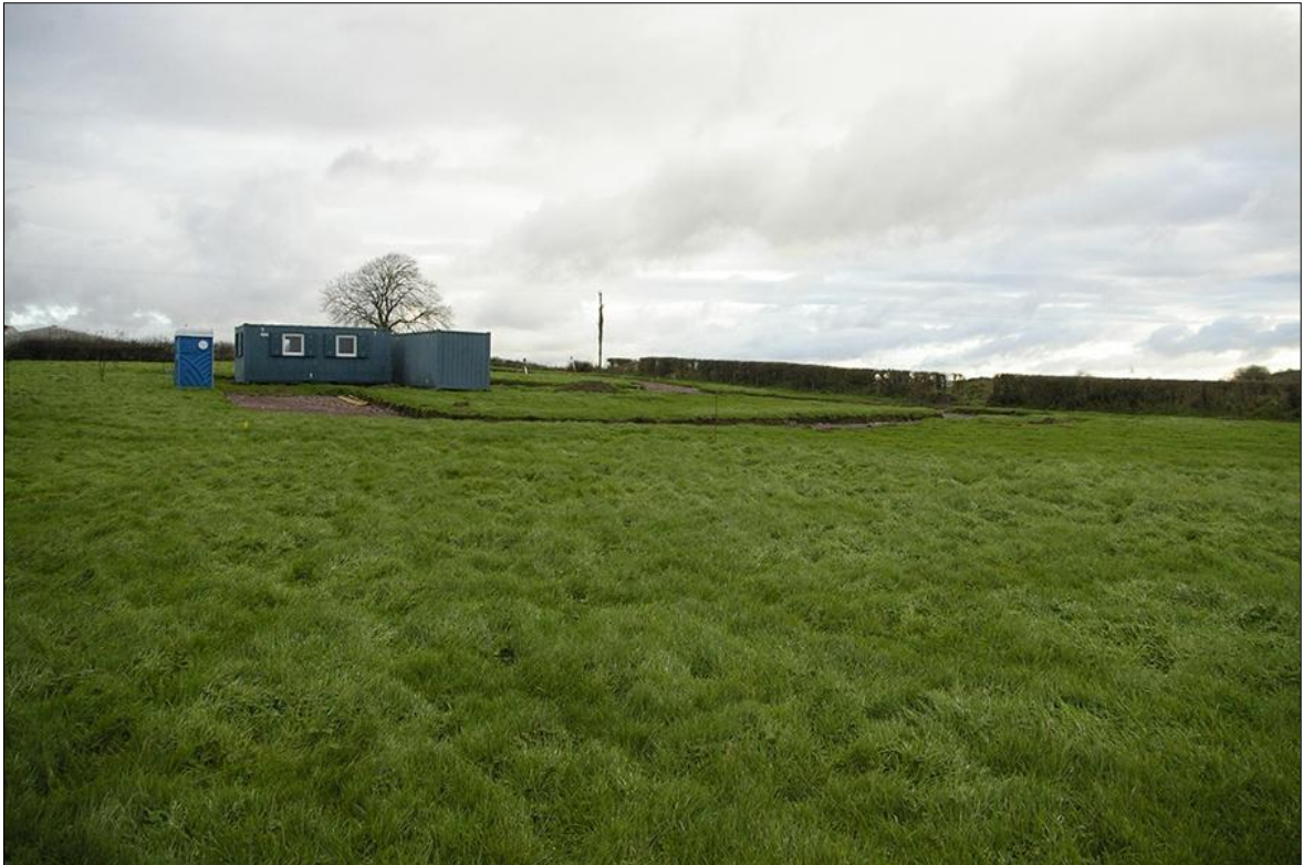
1. VIEW ACROSS SITE FROM SOUTH-WEST CORNER; VIEWED FROM THE SOUTH-WEST (NO SCALE).
