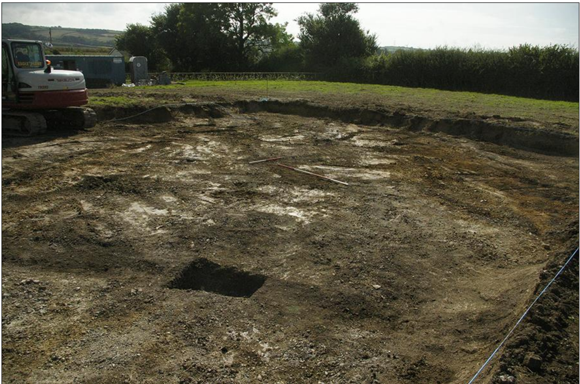
30. AREA 10, POST-EXCAVATION FOLLOWING MAIN SOIL STRIP; VIEWED FROM THE NORTH-EAST (1M & 2M SCALES).
