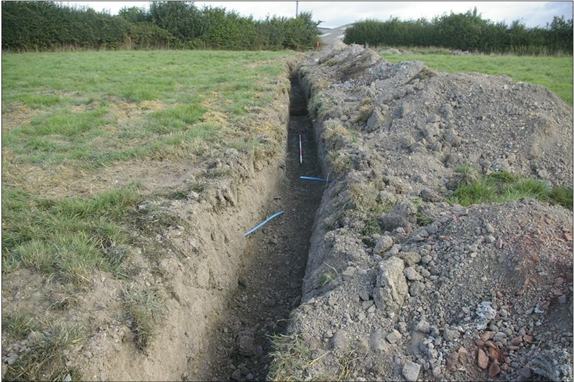
25. AREA 09, POST-EXCAVATION, SOUTH END; VIEWED FROM THE SOUTH-EAST (2M SCALE).
