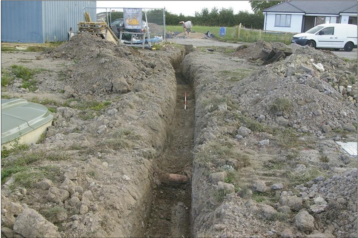
59. AREA 13, POST-EXCAVATION, CENTRAL SECTION; VIEWED FROM THE SOUTH-SOUTH-WEST (2M SCALE).
