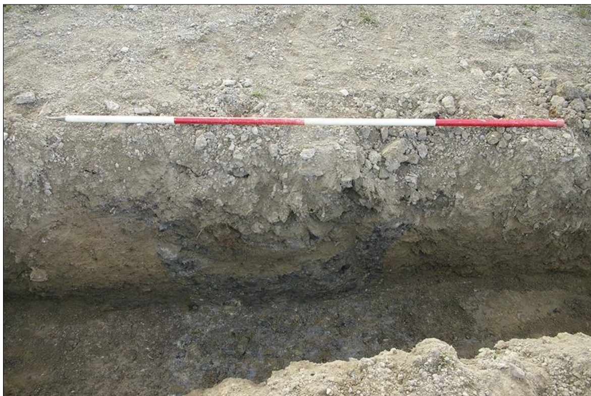
63. MODERN DRAIN CUT [1304], WEST FACING SECTION; VIEWED FROM THE WEST (2M SCALE).
