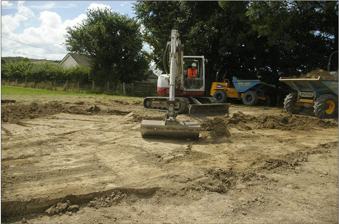
47. WORKING SHOT, AREA 12 MID-EXCAVATION; VIEWED FROM THE NORTH-WEST (NO SCALE).
