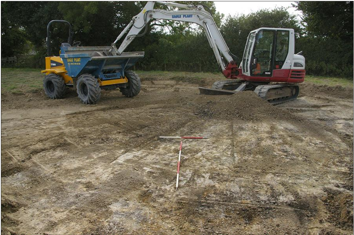
39. WORKING SHOT, AREA 11 MID-EXCAVATION; VIEWED FROM THE NORTH-EAST (1M & 2M SCALES).
