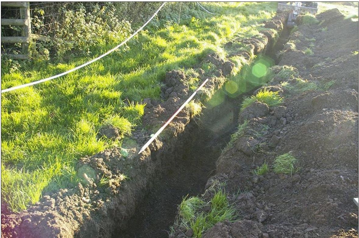
18. AREA 07, SOUTH-WEST FACING SECTION, OBLIQUE; VIEWED FROM THE WEST (2M SCALE).
