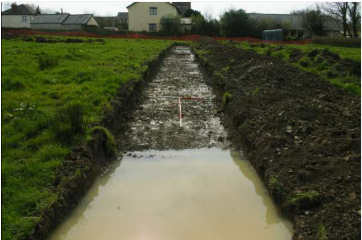
Trench #4; post-excitation; viewed from the north (1m & 2m scales).
