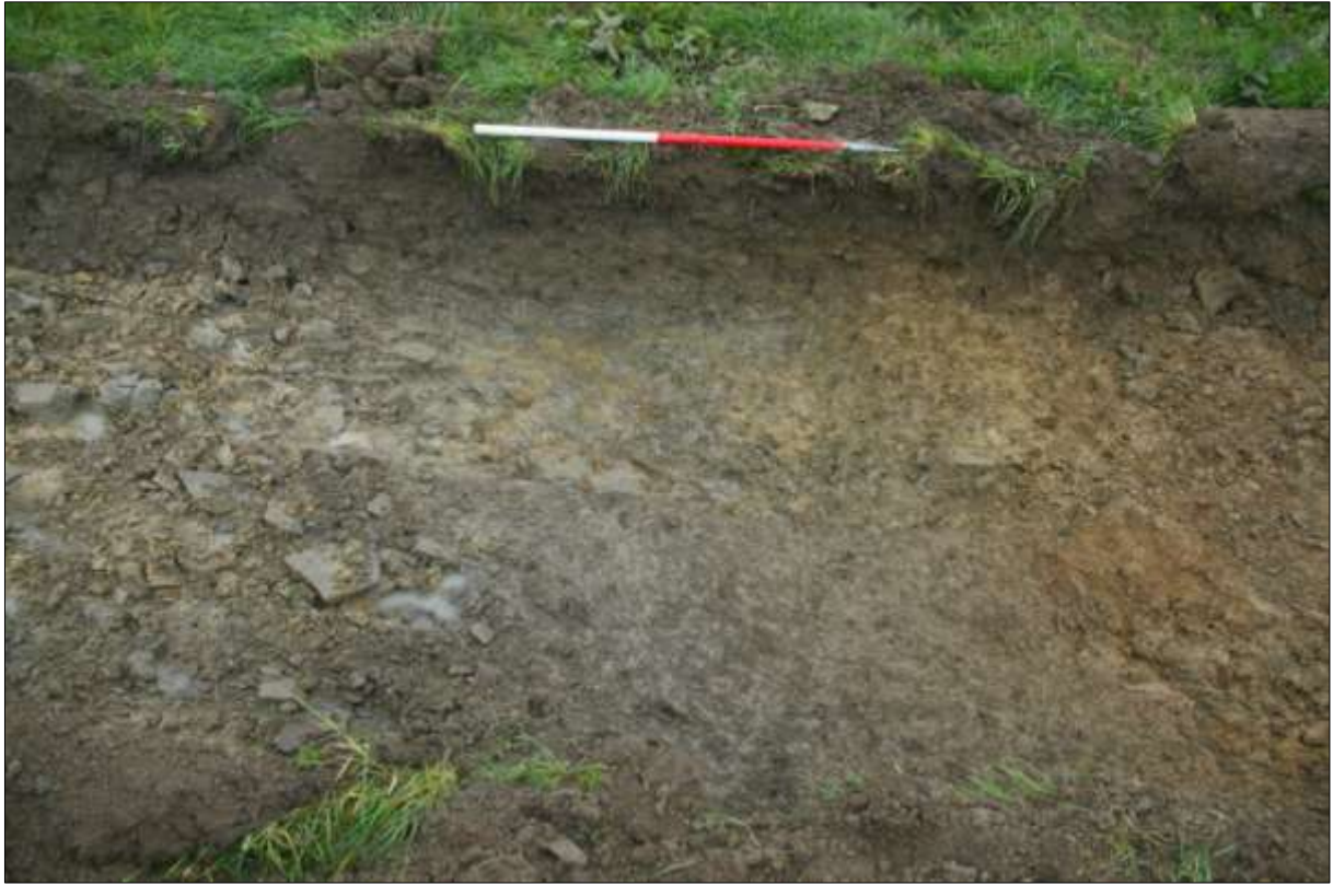
Ditch [308]; post-excavation; viewed from the west (1m scale).
