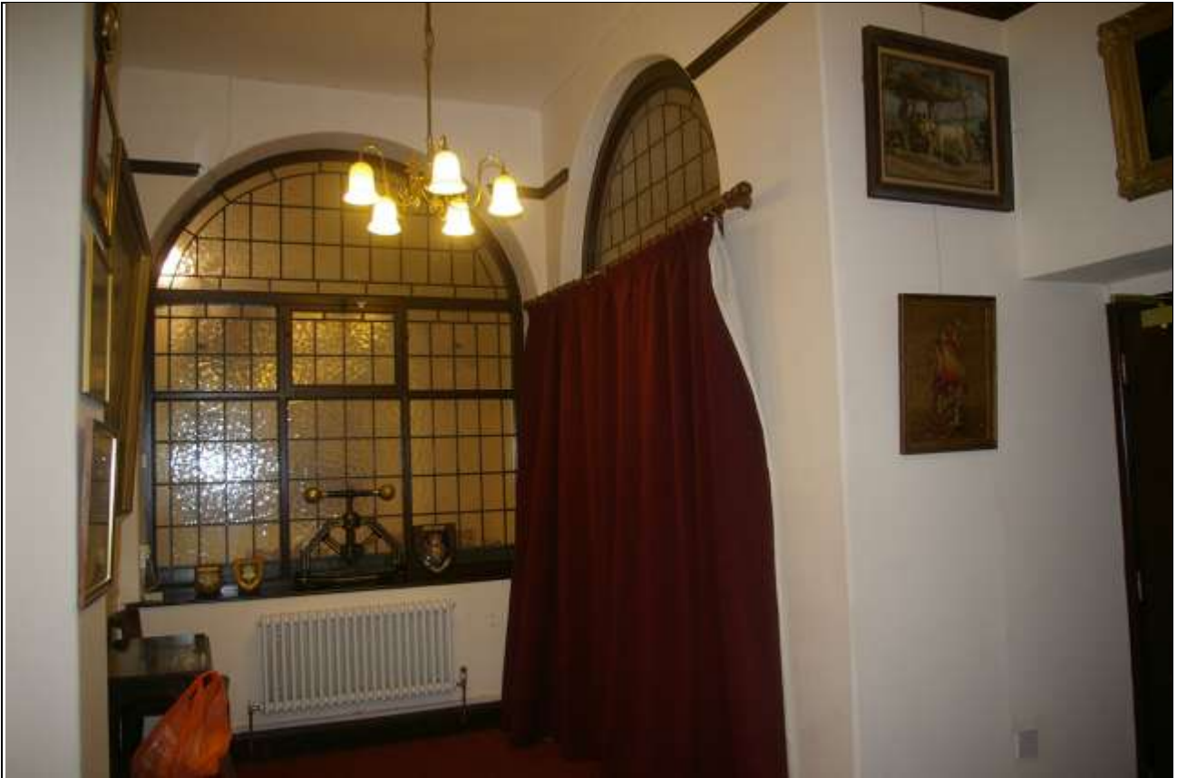
THE LOBBY/WAITING ROOM (ROOM 17) TO THE MAYOR'S PARLOUR, WITH LEADED GLAZED SCREEN IN THE BLOCKED ARCHED OPENING TO THE REST OF THE GROUND FLOOR AND SMALLER GLAZED LEADED FANLIGHT ABOVE A BLOCKED DOORWAY LEADING EAST; FROM THE SOUTH.
