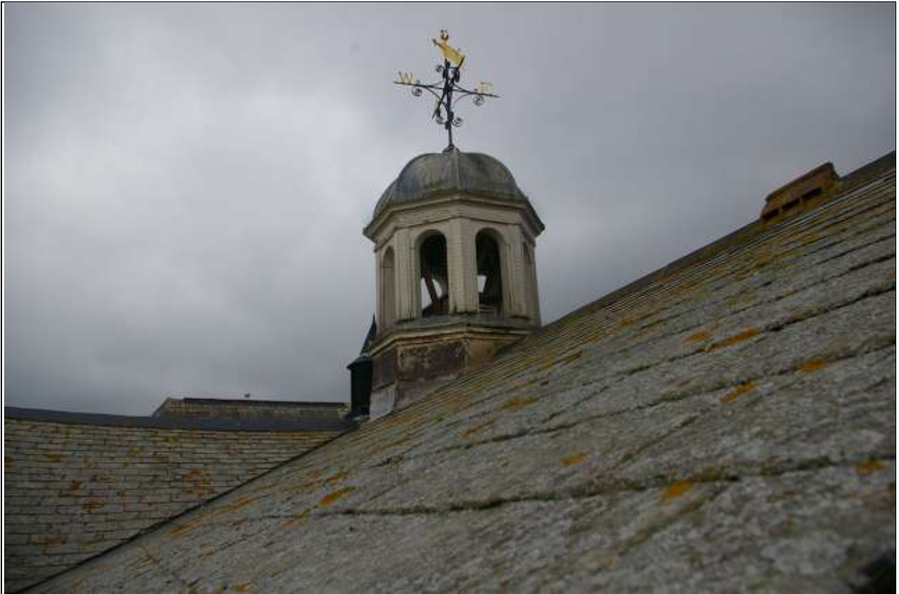
THE OCTAGONAL TIMBER BELL CUPOLA ON THE ROOF OF THE GUILDHALL WITH 1714 FORMER BUTCHERS' YARD BELL; FROM THE SOUTH, SOUTH-WEST.
