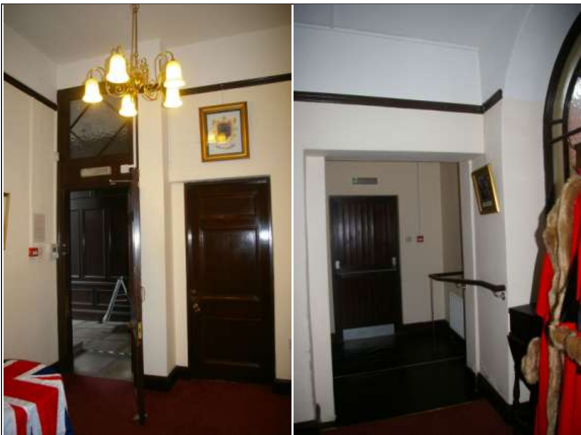
LEFT: THE 17 TH CENTURY STYLE DOORWAY WITH GLAZED FANLIGHT TO THE OPEN VESTIBULE (ROOM 15) AND PANELLED DOOR TO MAYOR'S PARLOUR (ROOM 16); FROM THE EAST-NORTH-EAST. RIGHT: ROOM 18, LOOKING THROUGH THE FORCED WALL OPENING TO FIRE ESCAPE AND DISABLED TOILETS; FROM THE SOUTH-SOUTH-WEST.
