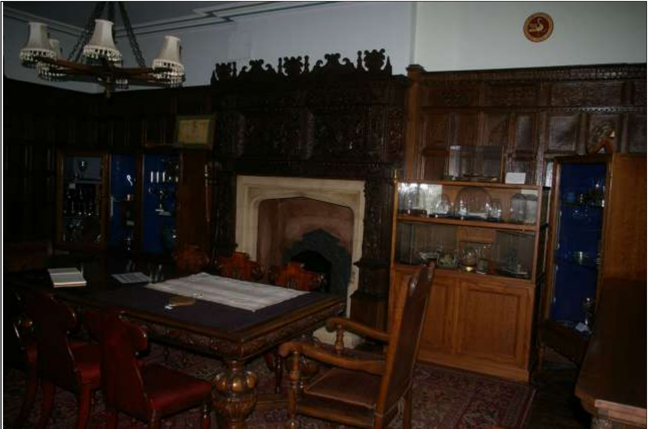
ROOM 5; THE SOUTH WALL OF THE MEETING ROOM, WITH SALVAGED RESET 17 TH CENTURY PANELLING, CAVETTO SIMPLE PLASTER CORNICE, 19 TH CENTURY AND FINE 16 TH CENTURY SALVAGED CARVED OVERMANTEL; FROM THE NORTH-WEST.
