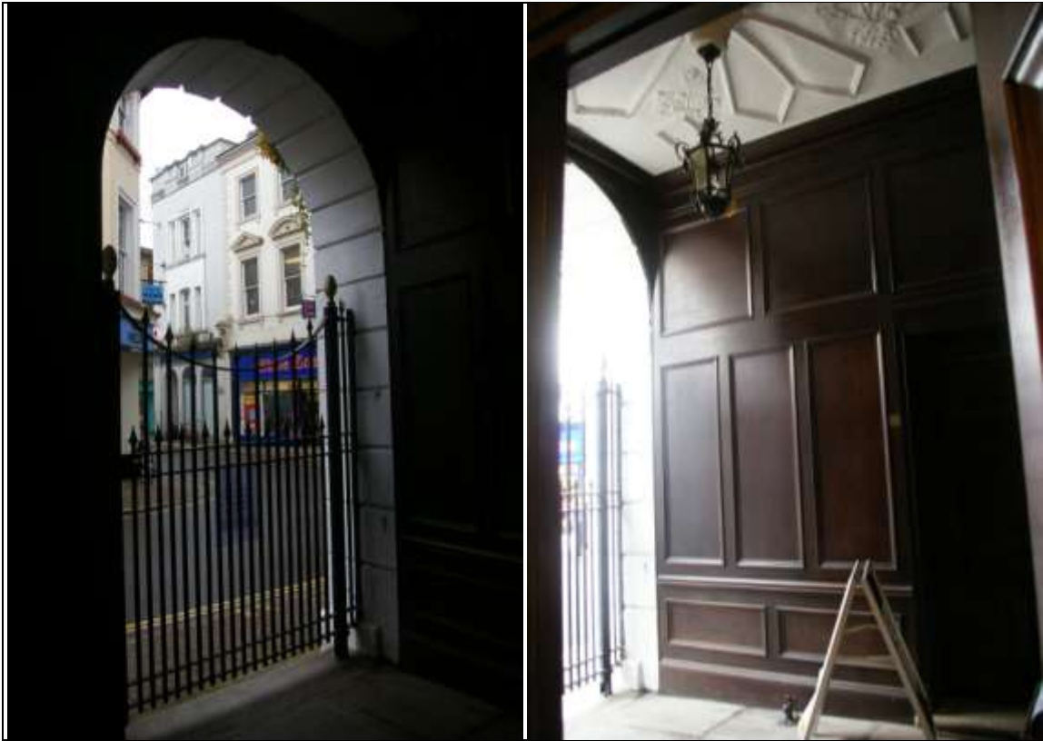
LEFT: ROOM 15; THE ROUND ARCHED BUTCHER'S ROW ENTRANCE IN THE SOUTH ELEVATION; FROM THE NORTH-EAST. RIGHT: 1920S PANELLING INSTALLED IN THE VESTIBULE, WITH A FRAGMENT OF A PENDANT 17 TH CENTURY PLASTER CEILING FITTED ABOVE.
