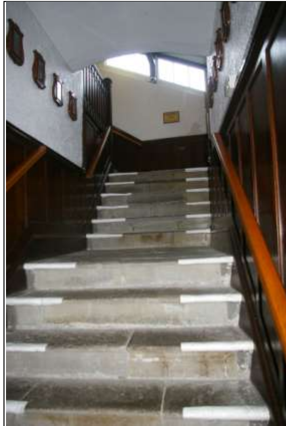
THE GRAND STONE STAIR WHICH RISES FROM THE BUTCHER'S ROW ENTRANCE OF THE BUILDING, BUT MAY HAVE BEEN RESET, WITH 1920S PANELLING TO SIDES; FROM THE WEST.
