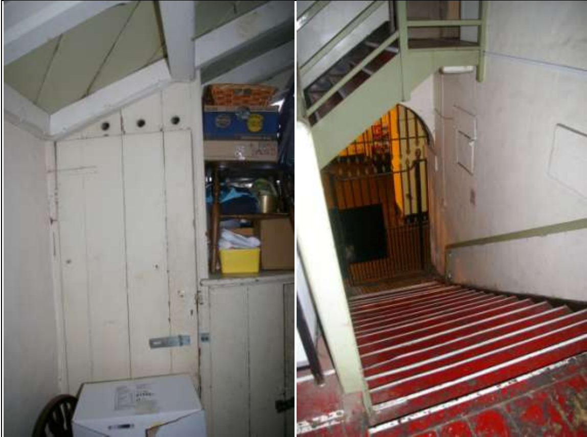
LEFT: THE PUBLIC GALLERY STEPS (ROOM 13) DROPPING TO THE GROUND FLOOR OF THE GUILDHALL; FROM THE NORTH-NORTH-EAST. RIGHT: THE BEADED PLANK BOARDED CUPBOARDS ON THE LANDING OF THE PUBLIC GALLERY STEPS (ROOM 13); FROM THE WEST.
