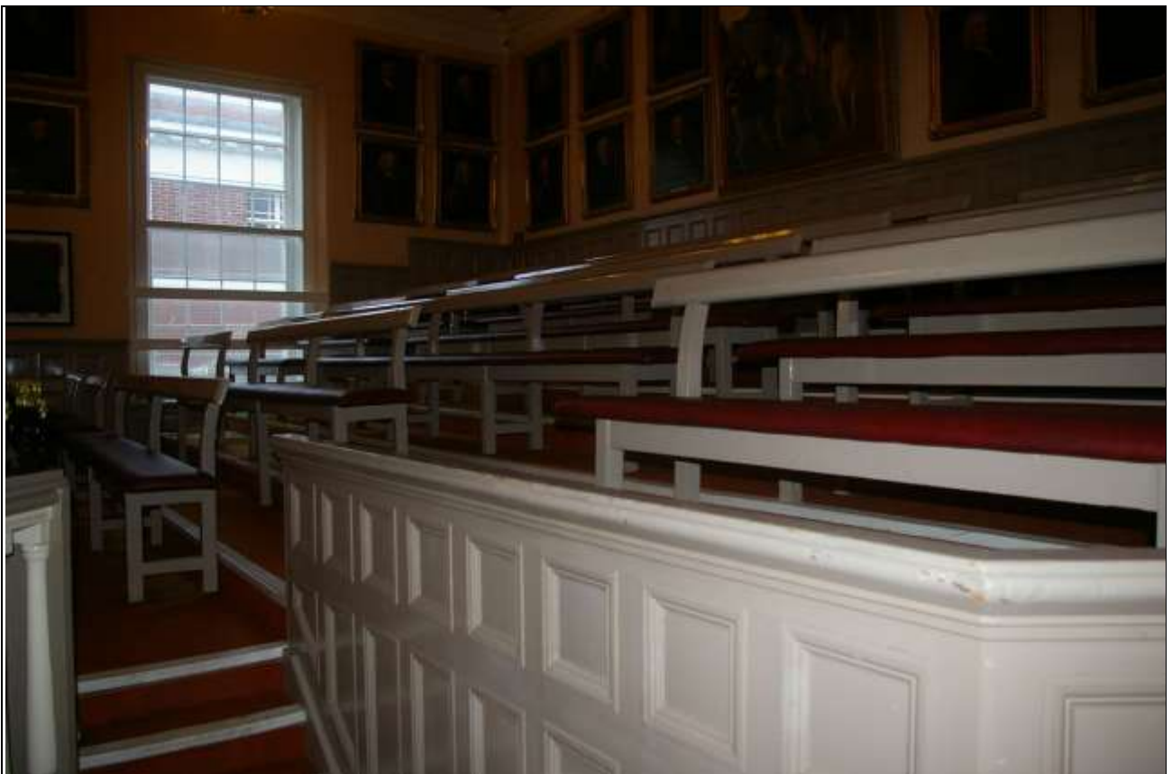
THE TIERED PUBLIC GALLERY AREA OF THE MAIN CHAMBER (ROOM 6), WITH REFITTED 20 TH CENTURY BENCHES; FROM THE EAST, SOUTH-EAST.
