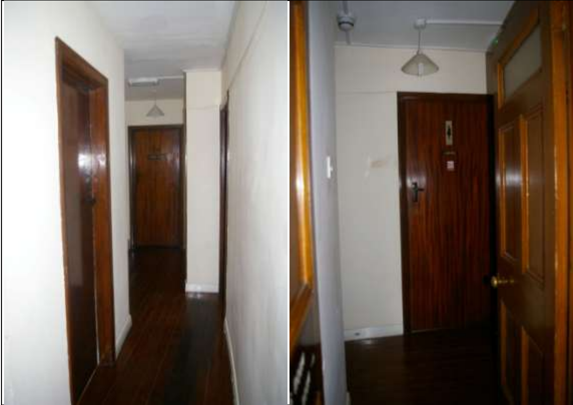
LEFT: ROOM 8; VIEW TO THE ROBING ROOM (ROOM 7) AND KITCHEN (ROOM 10); FROM THE SOUTH. RIGHT: THE DOORWAY FORCED IN THE EAST WALL ACCESSING ROOMS 7-12, RESET WITH PANELLED DOOR CASEMENT; FROM THE WEST.
