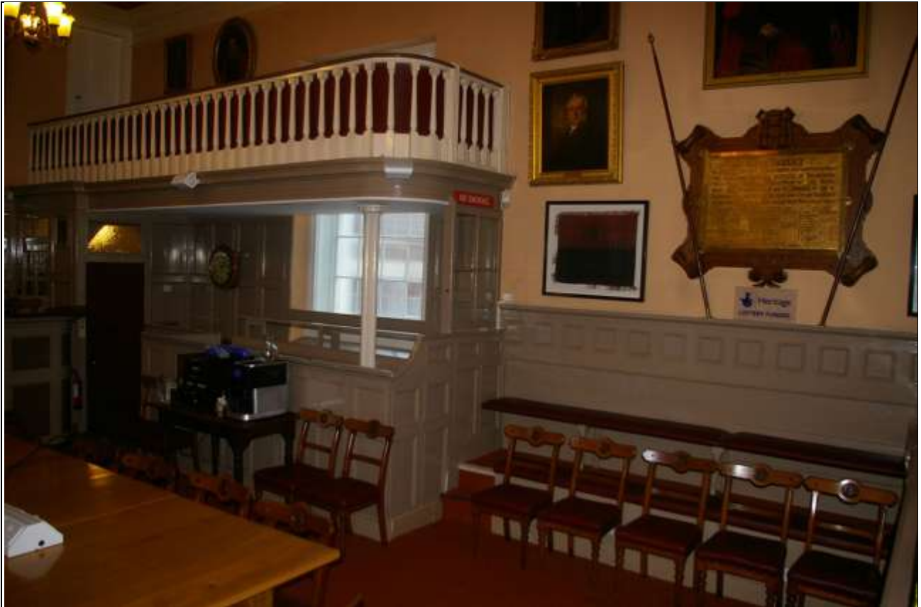
ROOM 6; THE WEST SECOND FLOOR GALLERY, SUPPORTED ON SLENDER COLUMN AND PANELLED SEATING BELOW, WITH OPEN BENCHES TO THE NORTH; FROM THE NORTH-EAST.
