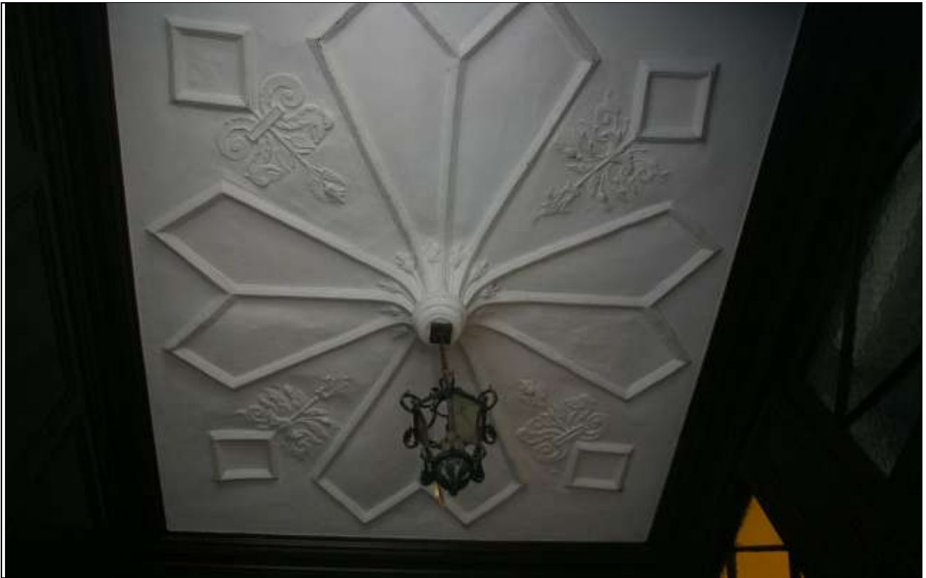
ROOM 15; FRAGMENT OF 17 TH CENTURY PENDANT PLASTER ROOF, RESET AND REWORKED INTO A COPY CEILING; FROM THE SOUTH (BELOW).
