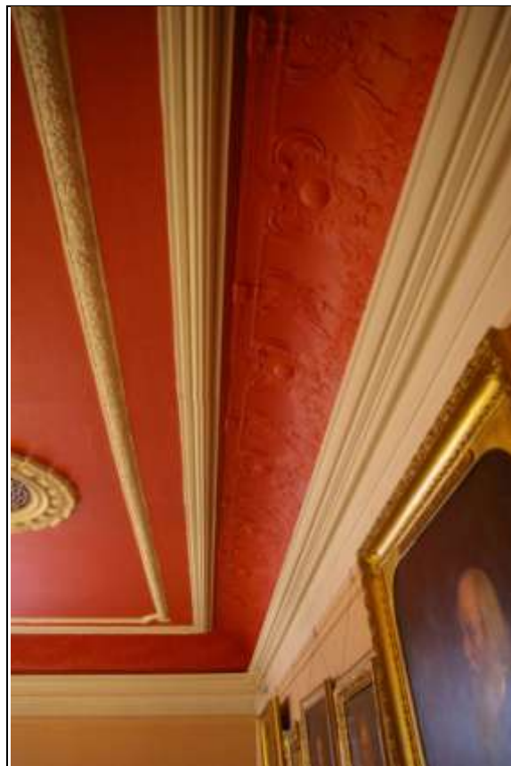
DETAIL OF THE ANAGLYPTA WALLPAPER APPLIED IN THE LATER 19 TH CENTURY TO THE SIMPLE CAVETTO SIDES OF THE MOULDED PLASTER CEILING OF ROOM 6; FROM THE WEST.
