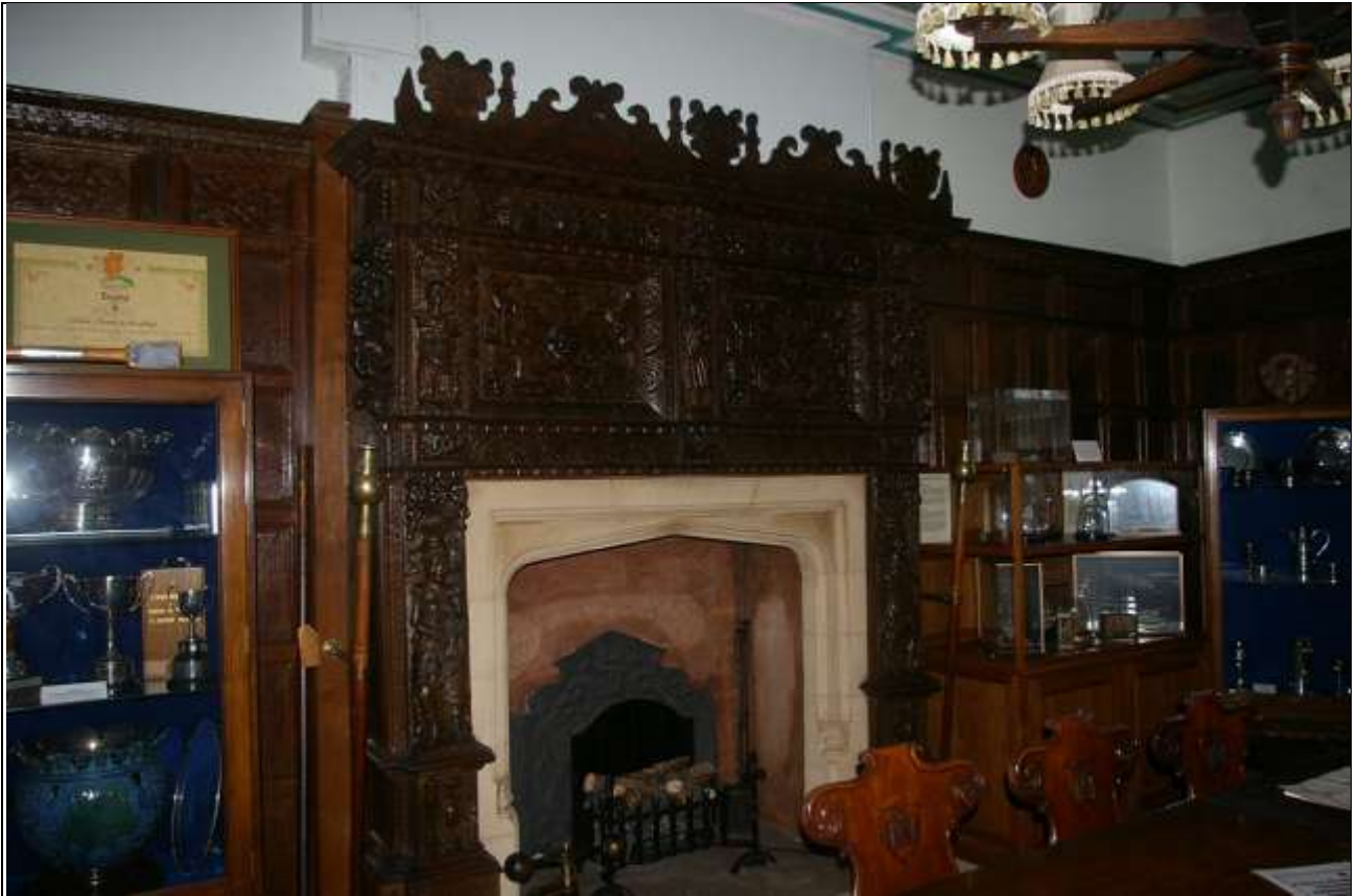
ROOM 5; THE ELABORATELY CARVED OVERMANTEL, FITTED TO A TYPICAL SHALLOW 19 TH CENTURY STACK, WITH LATE 19 TH OR EARLY 20 TH CENTURY NEO-GOTHIC STONE COMPOSITE FIREPLACE; FROM THE NORTH-EAST.
