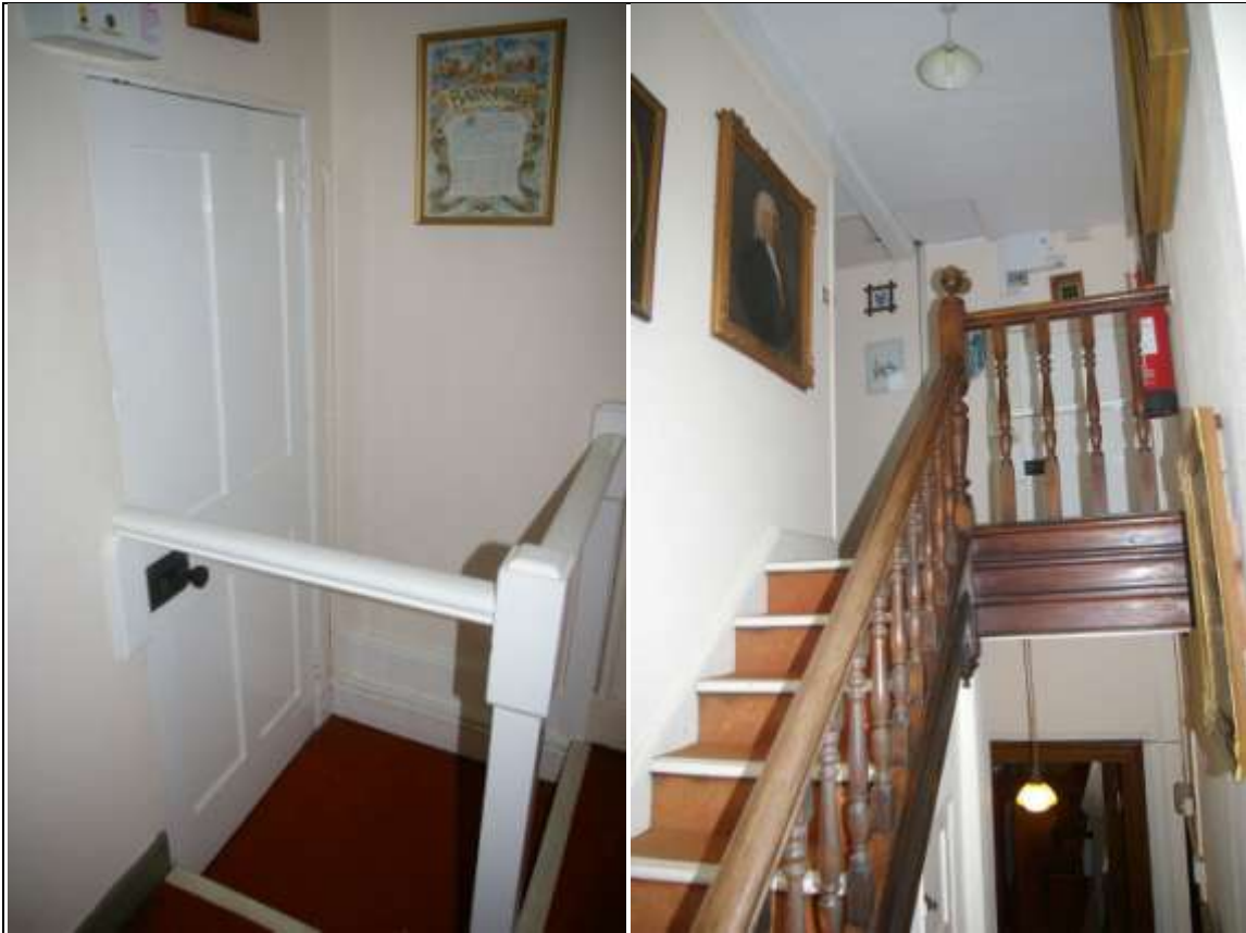
LEFT: ROOM 2; THE SMALL 19 TH CENTURY PANELLED DOOR LEADING TO THE EAST SECOND FLOOR BALCONY; FROM THE SOUTH-WEST. RIGHT: ROOM 4/ROOM 2; THE STAIRS TO THE SECOND FLOOR, A 20 TH CENTURY STAIR, A HISTORIC COPY; FROM THE SOUTH.
