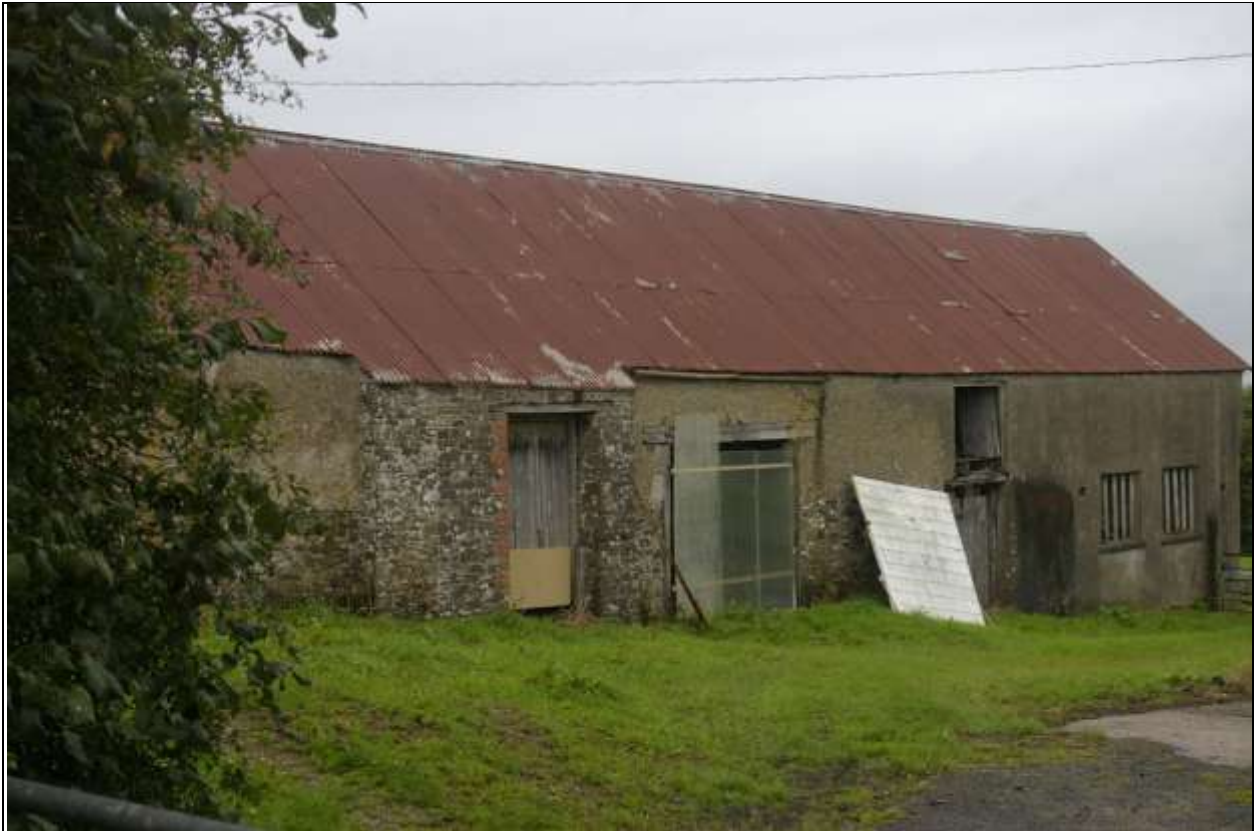
The Listed barn at Great Gorwood; from the south-west.
