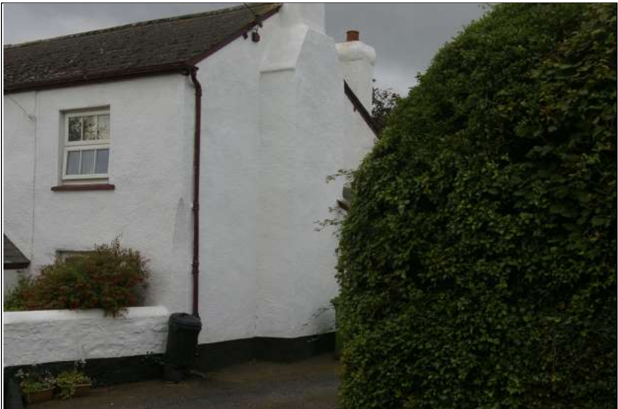
View towards the site from the Coach & Horses Inn, locally blocked; from the east-north-east.
