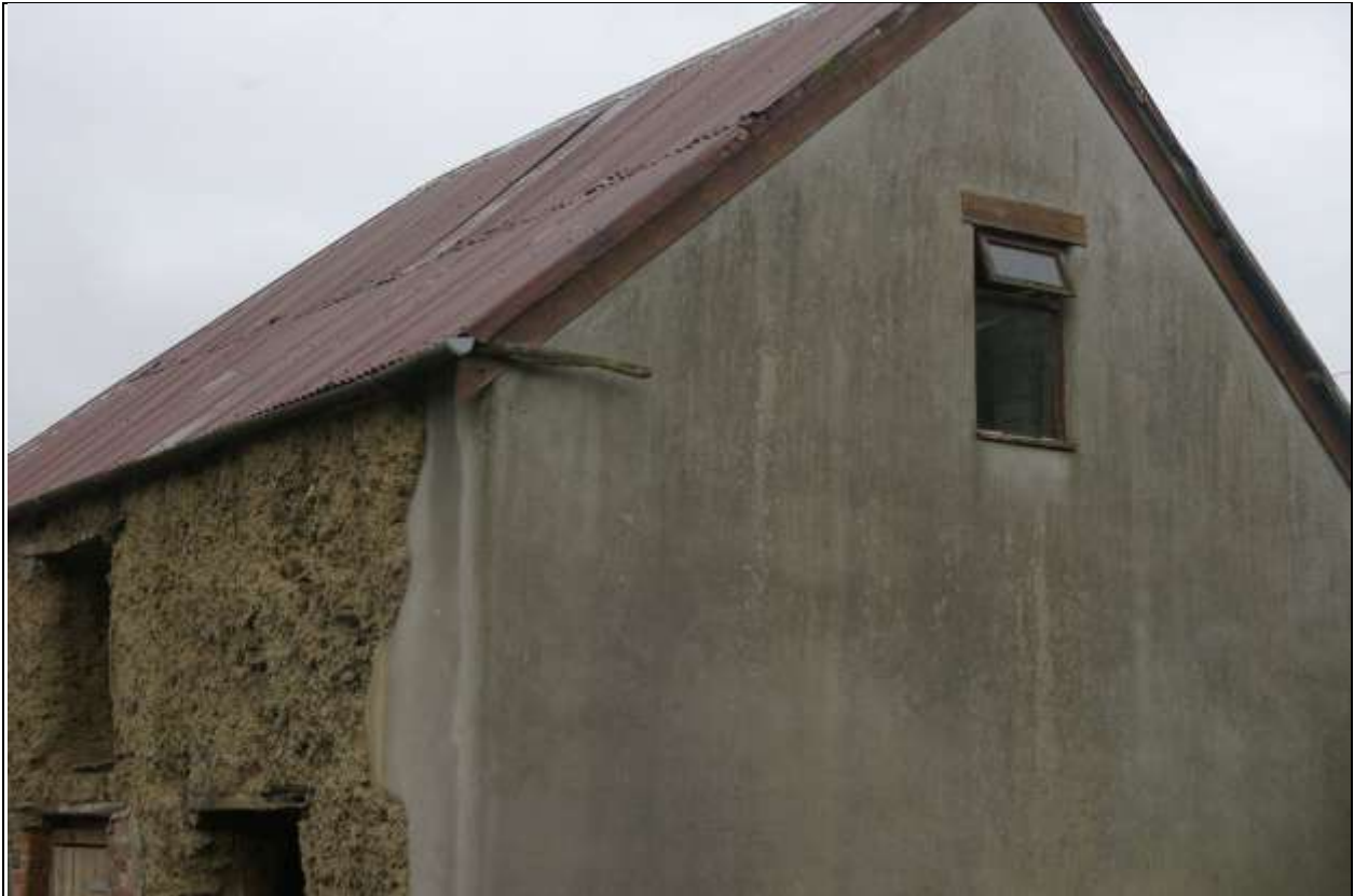
As above, showing modern repairs.
