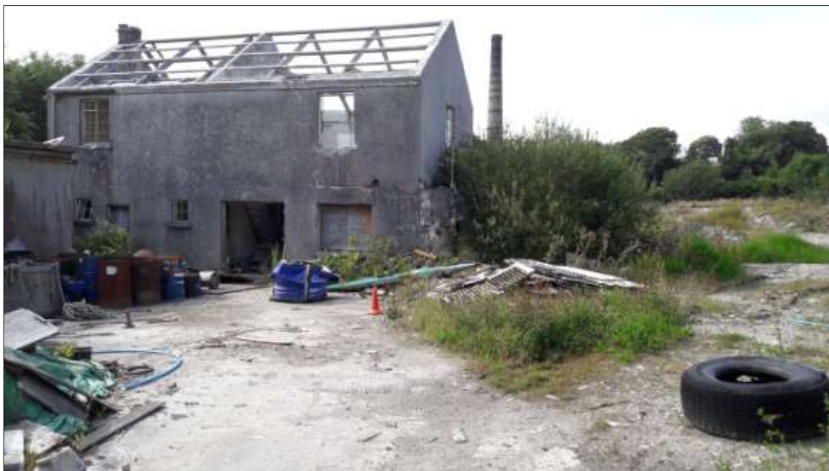
FIGURE 24: B2, VIEWED FROM THE SOUTH-EAST.
