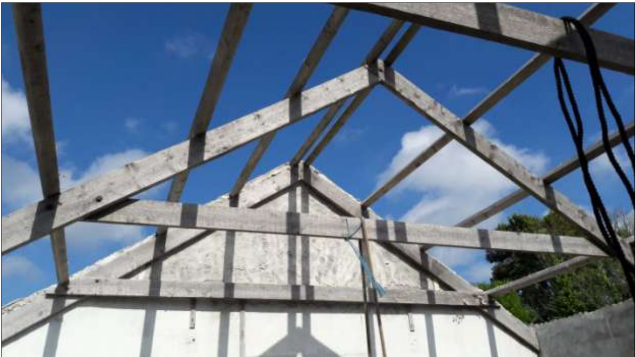
The exposed roof structure in B2, viewed from the west.
