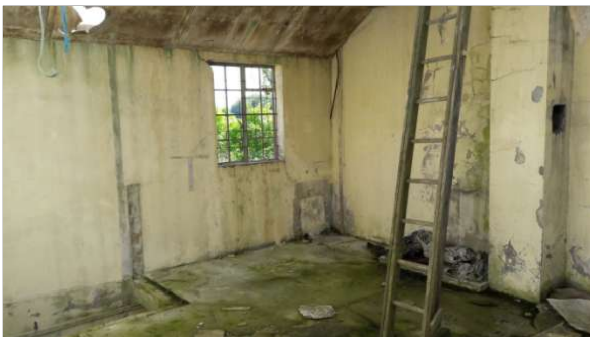
FIGURE 25: THE FIRST-FLOOR INTERIOR OF THE STAFF WELFARE, VIEWED FROM THE NORTH-EAST.
