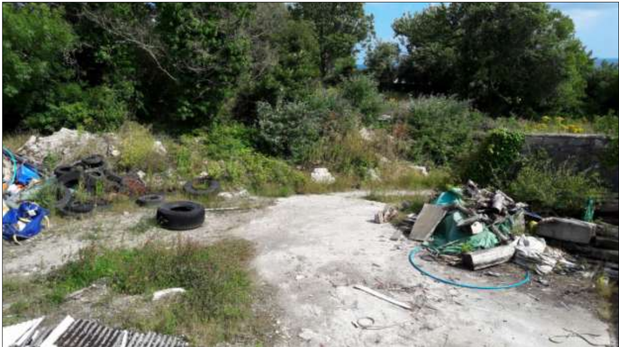
The lower part of T8, showing the breach in the wall; viewed from the north-west.
