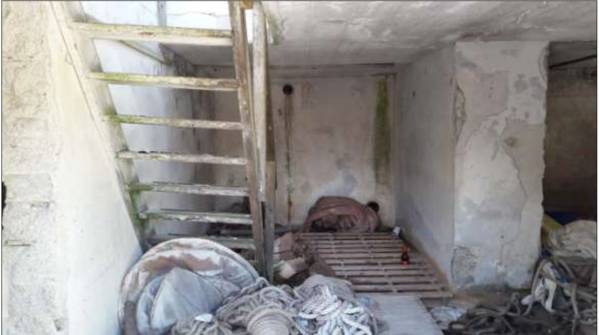
FIGURE 28: THE GROUND-FLOOR INTERIOR OF THE PUMP HOUSE, VIEWED FROM THE SOUTH.
