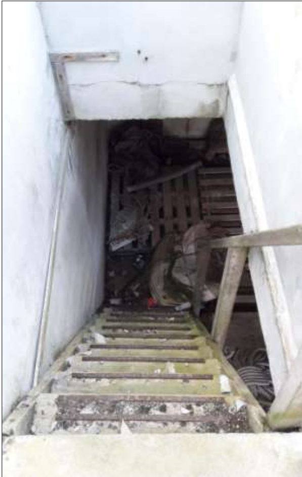
B2, the surviving stairs in the pump house.
