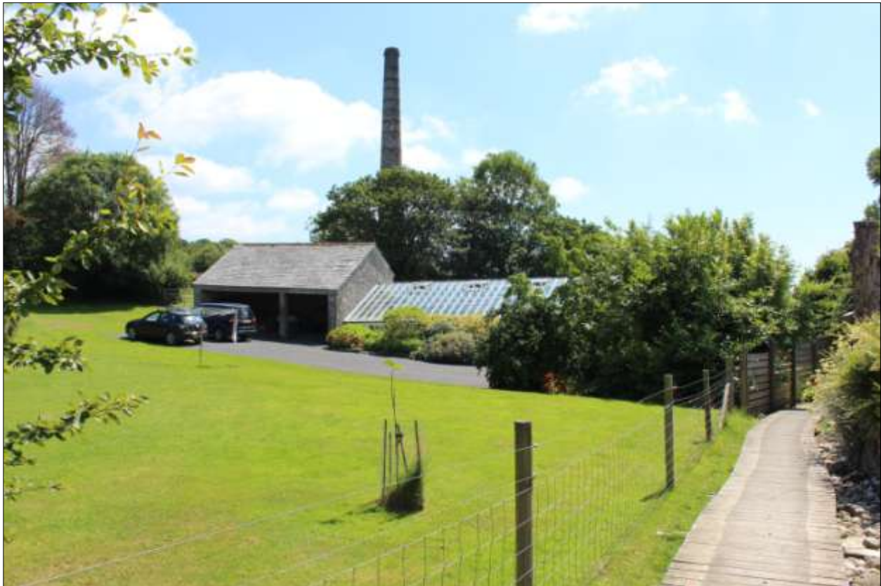
The converted farm buildings to the north of Polmear Farm; viewed from the north-west.
