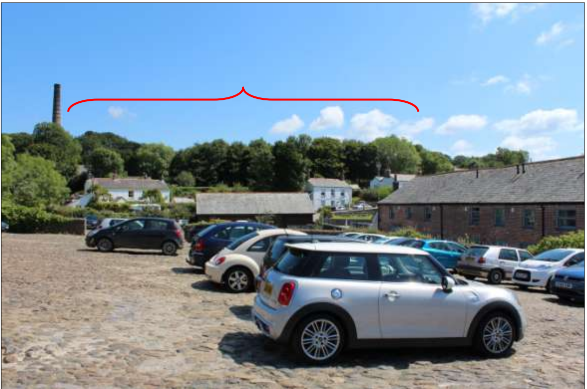
FIGURE 33: VIEW FROM THE CAR PARK (FORMER ORE FLOORS) AT THE RASHLEIGH ARMS HOTEL; VIEWED FROM THE WSW. THE SITE LIES BEHIND THE BANK OF TREES ON THE SKYLINE (INDICATED).
