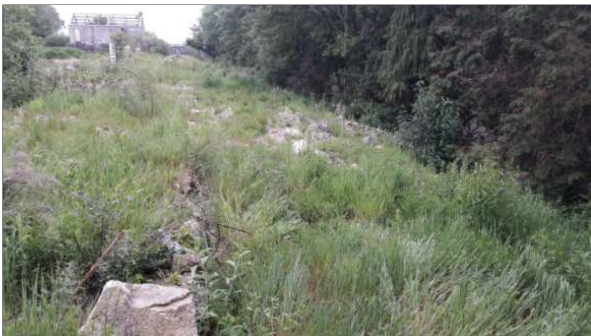
FIGURE 19: THE INFILLED COMPARTMENTS OF THE LINHAY, VIEWED FROM THE NNW.
