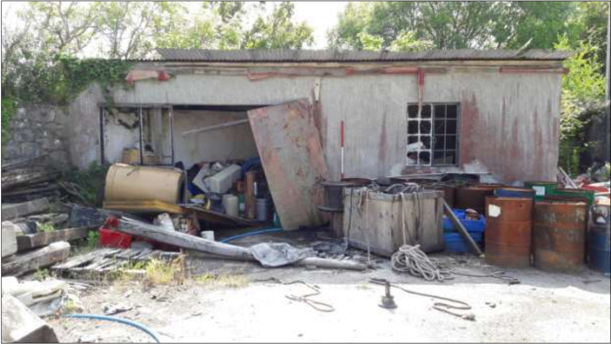
The east elevation of B3, viewed from the east (2m).
