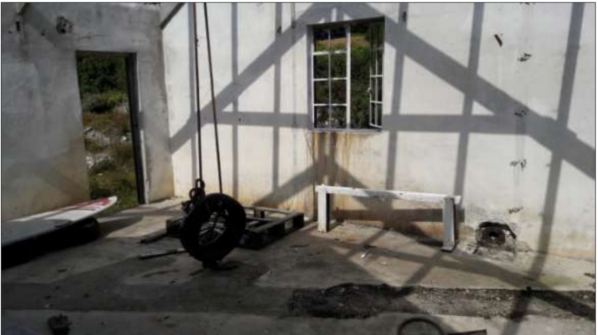
FIGURE 29: THE FIRST-FLOOR INTERIOR OF THE PUMP HOUSE, VIEWED FROM THE SOUTH-WEST.
