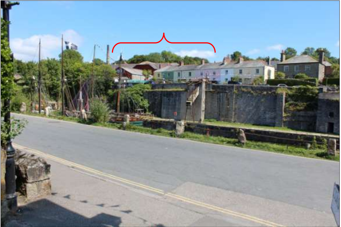
FIGURE 34: VIEW FROM THE HARBOUR OUTSIDE THE HARBOURSIDE INN; VIEWED FROM THE SSW. VIEWS TO THE SITE ARE BLOCKED BY THE HERITAGE CENTRE BUILDING (INDICATED).
