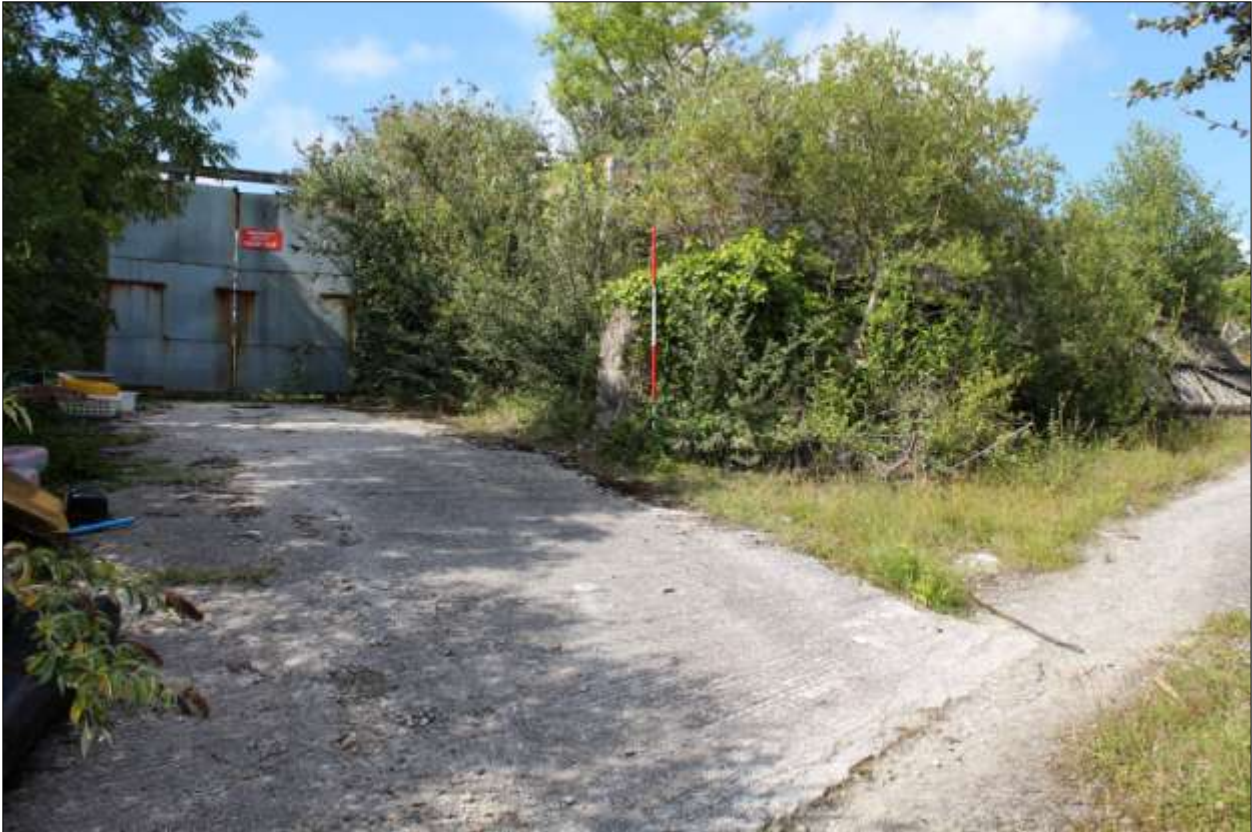
The concrete ramp leading up to the steel doors; viewed from the south (scale 2m).
