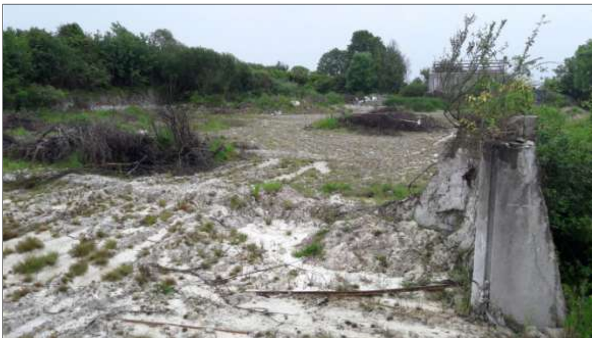
FIGURE 10: THE SETTLING TANKS, VIEWED FROM THE NNW.
