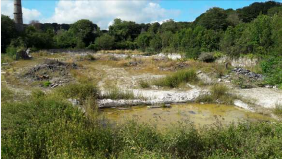
FIGURE 11: THE SETTLING TANKS, VIEWED FROM THE SSE.
