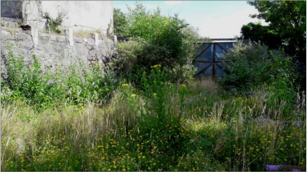
The southern end of the drying floor, viewed from the NNW.
