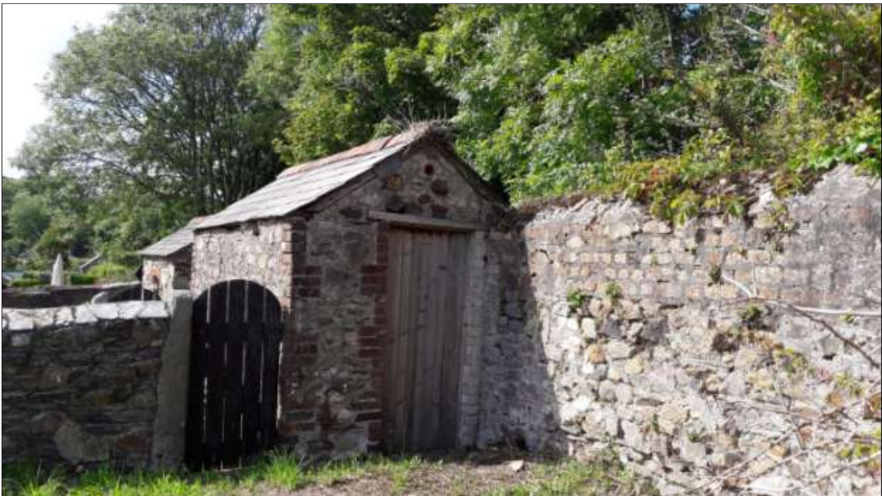
One of the small buildings (privies) to the rear of the properties on Quay Road, viewed from the south. This building is to the rear of nos. 23-24. Note the use of brick in the wall to the left (the property boundary with the Lower Dry), perhaps derived from the flues.
