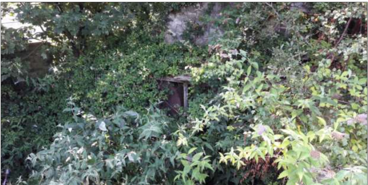
The structure next to the north wall of C1 in the linhay; viewed from the south.
