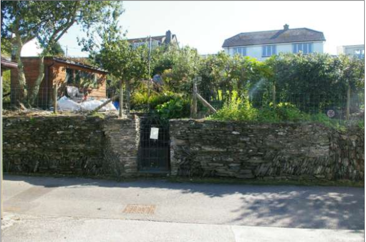
FIGURE 7: VIEW OF THE WALL FROM THE NORTH.
