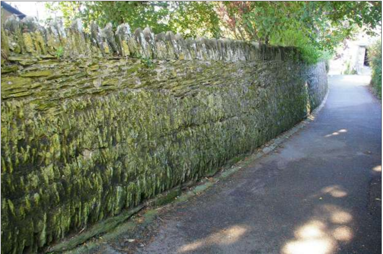
DETAIL OF THE WALL FLANKING BATTERY LANE; VIEWED FROM THE SOUTH.
