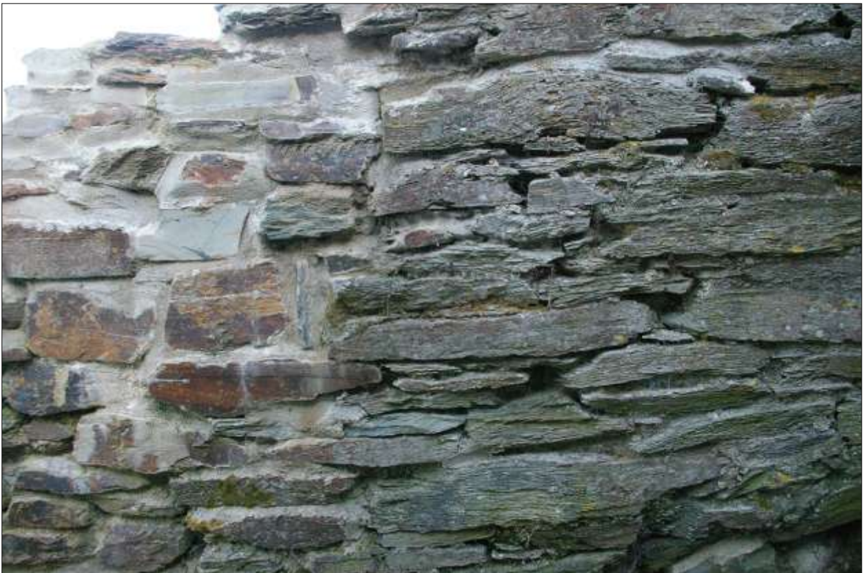
THE VISUAL COMPARISON BETWEEN WEATHERED/TEXTURED HISTORIC STONWORK, AND MORE RECENT, UNWEATHERED STONE.
