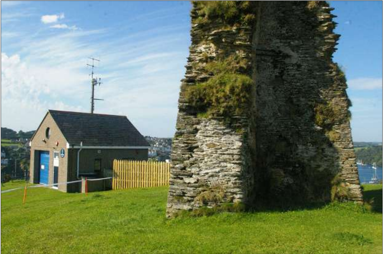
AS ABOVE, VIEWED FROM THE SOUTH-EAST.
