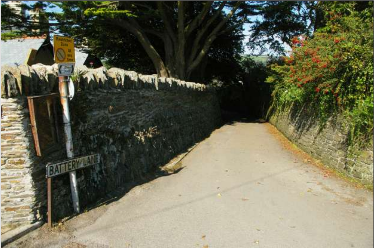
AS ABOVE, LOOKING DOWN BATTERY LANE; VIEWED FROM THE SOUTH.
