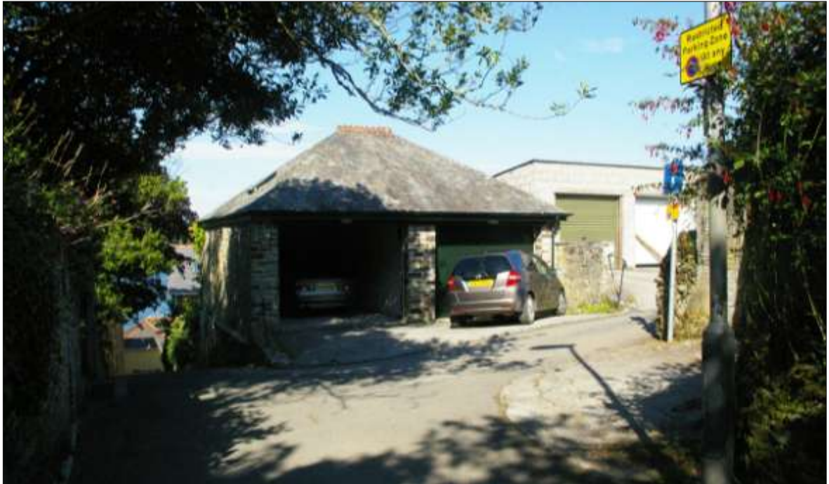
FIGURE 9: THE CORNER OF BATTERY LANE AND HOCKENS LANE, SHOWING THE NEW GARAGE; VIEWED FROM THE SOUTH.
