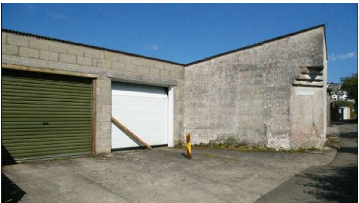
FIGURE 10: THE CONCRETE-BLOCK GARAGE OPPOSITE THE PROPOSED SITE; VIEWED FROM THE SOUTH-WEST.
