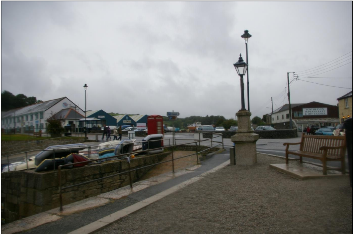
View along the main harbour, showing the existing row of buildings blocking/screening views into the harbour from the boat yard, but also showing the strong visual presence of the boat yard sheds, currently within the harbour; from the east, south-east.
